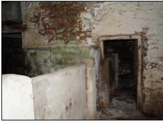
Plate 9. Entrance from one part of the cowhouse to the other. A low concrete partition for additional stalls behind is to the left of the photograph.
