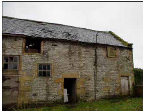
Plate 6. Front elevation of barn/cowhouse, western half.
