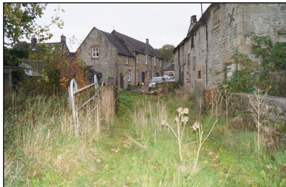
Plate 1. View of the site looking east towards the terraces used as holiday lets by the Charles Cotton Hotel.
