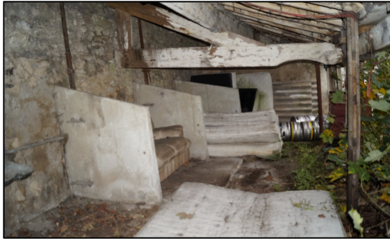
Plate 14. Interior of 'cart shed' looking east. A water feeder is visible to the right of the picture. Discarded mattresses and other debris fill the structure.
