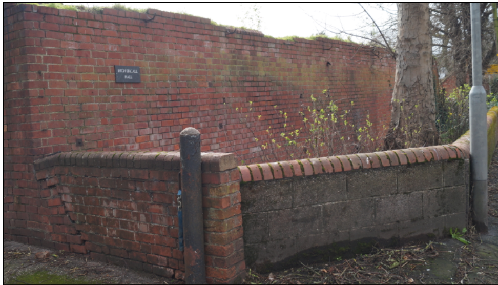
Plate 7. Partial view of boundary to High Ercall Hall on B5062 consisting of concrete blocks capped by brick coping.
