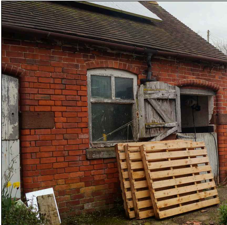
Plate 6. Front elevation of the cowhouse/milking parlour.
