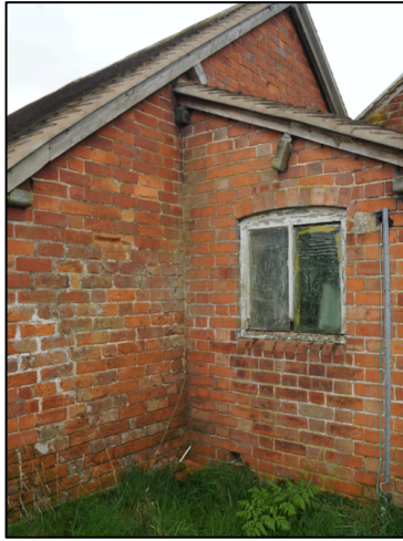
Plate 10. Small power house.
