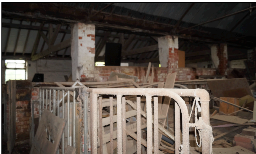
Plate 7. Brick piers to the cowhouse/milking parlour from inside the later cow barn.
