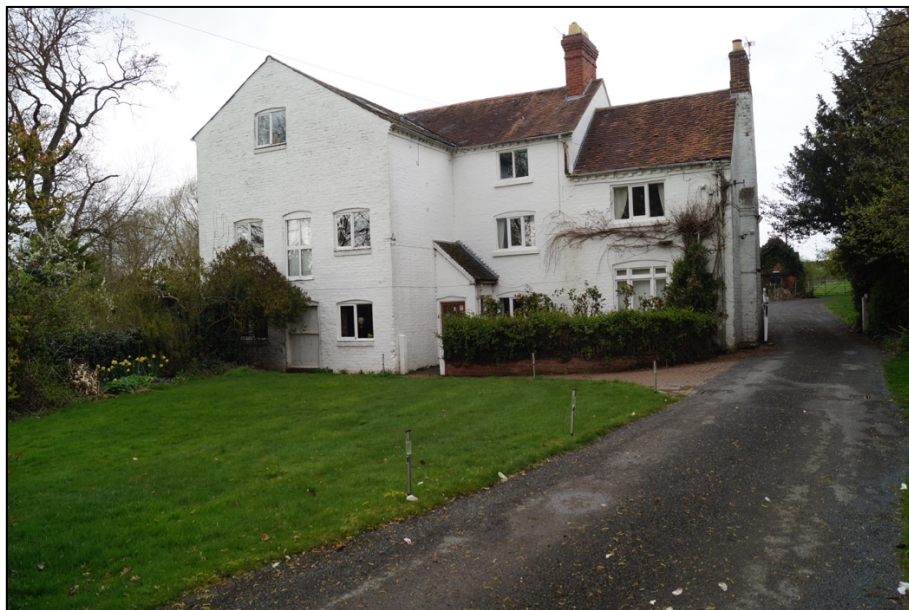
Plate 1. Front elevation of the mill and adjoining Mill House viewed from the Shrewsbury Road.
