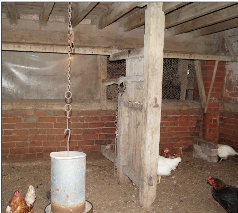
Plate 3. In situ wooden stall partitions.
