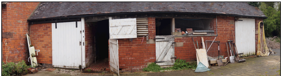
Plate 9. Front elevation of the mid to late 19 th century extension.
