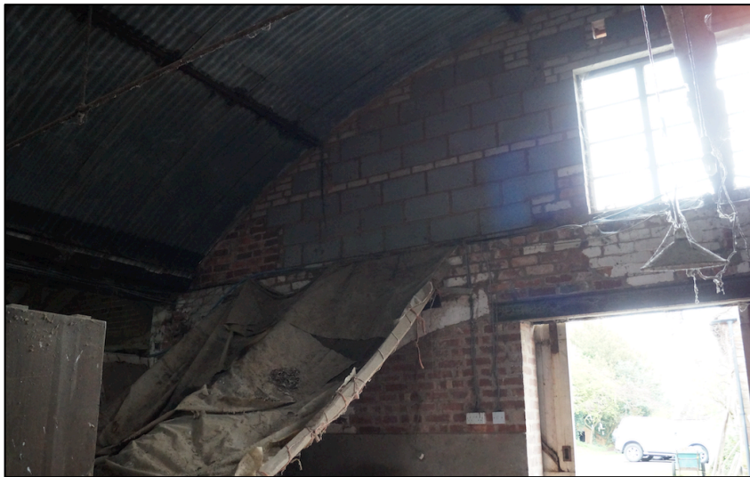
Plate 13. Upper part of the building showing where it was extended upwards.
