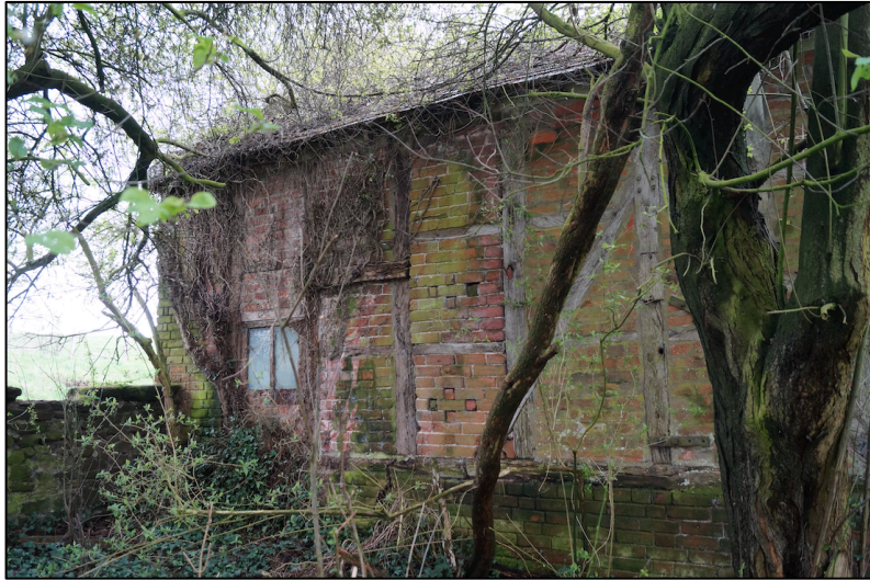
Plate 2. North east facing elevation of the barn.
