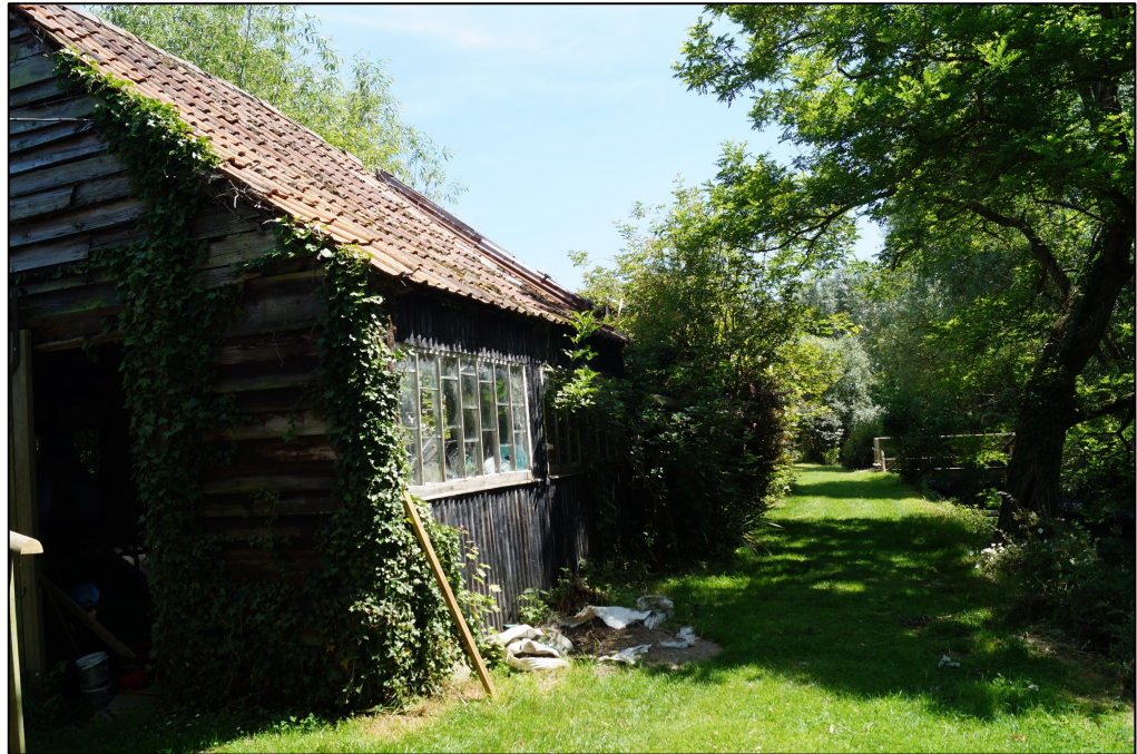
Plate 1. Showing surviving section of a former workshop.
