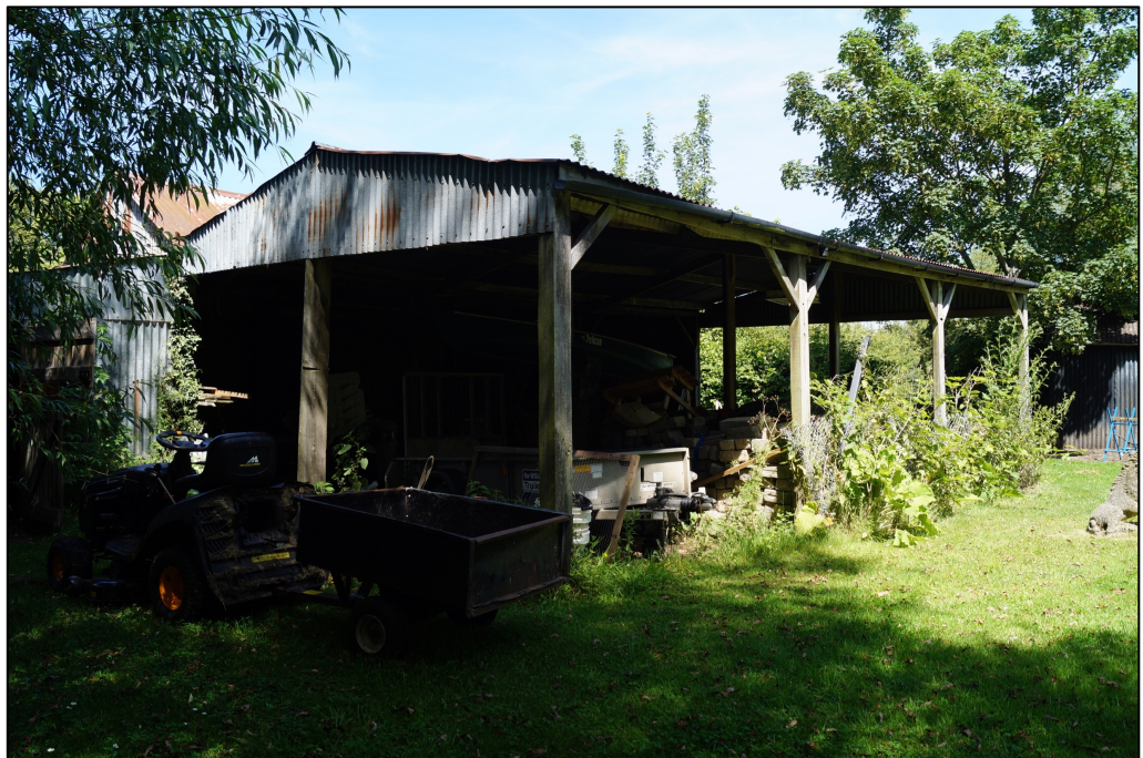
Plate 4. Open fronted store.
