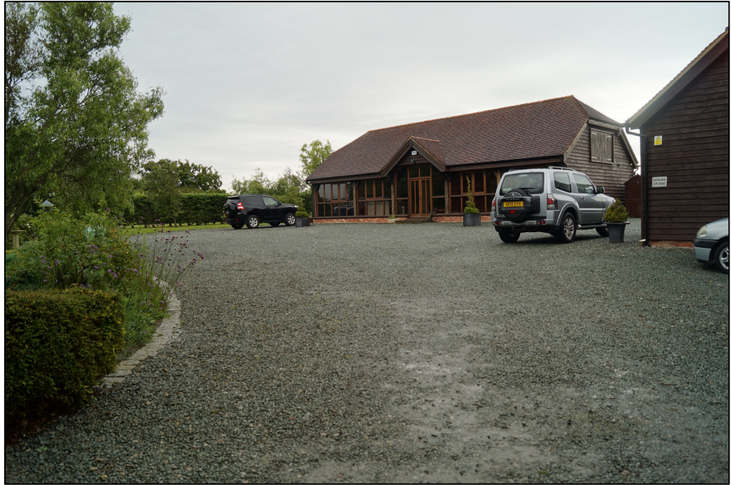
Plate 1. View of the building from the entrance to the property.
