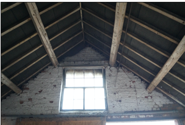
Plate 5. Detail of hopper window in gable end of Barn 2.
