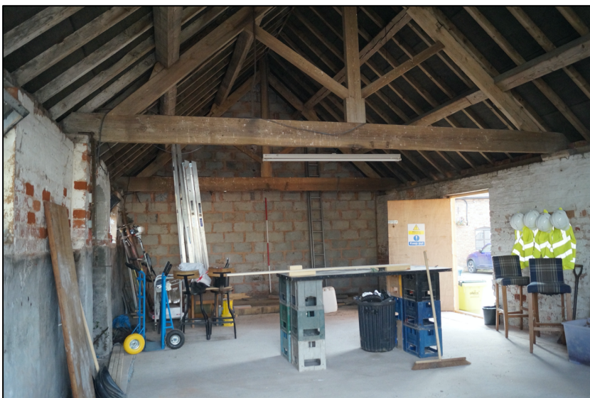
Plate 3. View of interior of Barn 2 looking south.
