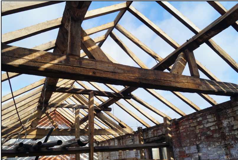
Plate 9. Detail of roof timbers.
