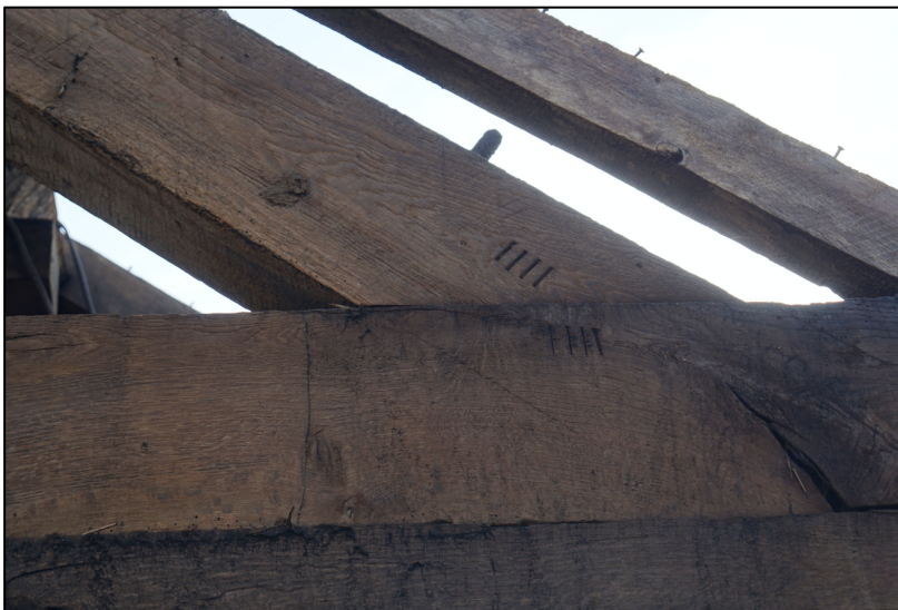
Plate 10. Carpenters marks on two roof timbers.
