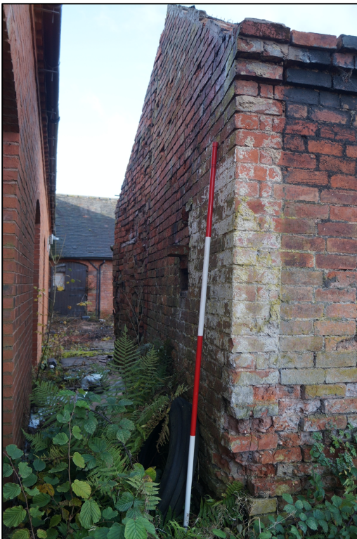
Plate 12. Southern elevation of Barn 3.
