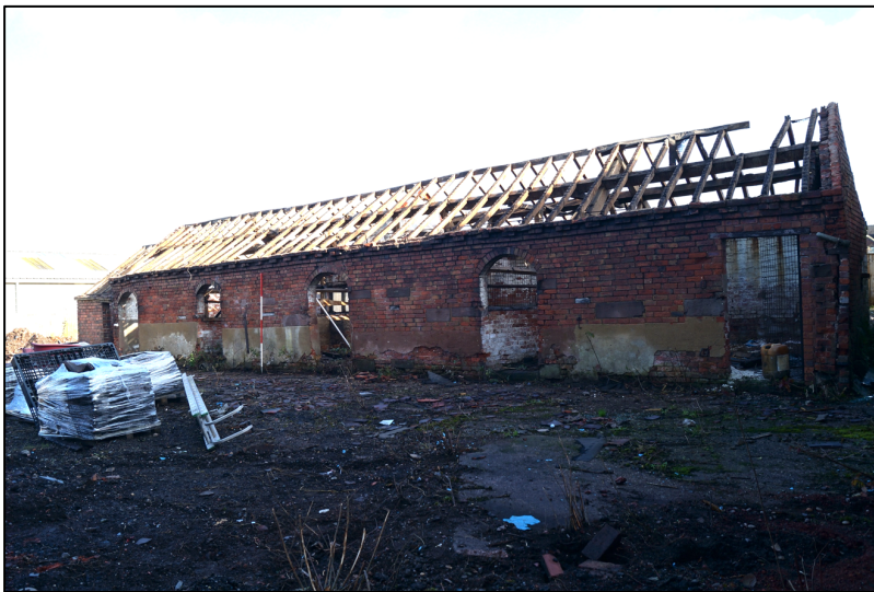
Plate 6. West facing elevation of Barn 3.
