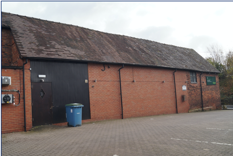
Plate 14. Modified threshing barn showing east facing elevation.
