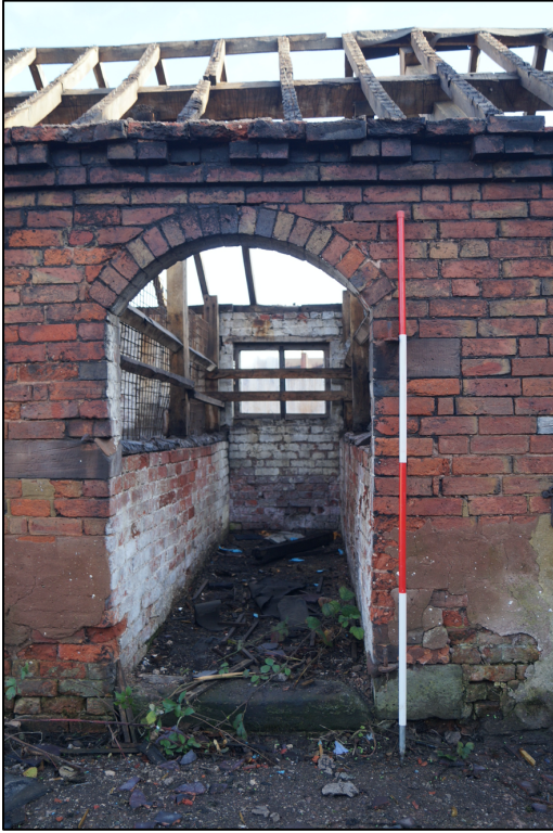
Plate 8. Example of corridor beyond arched opening.
