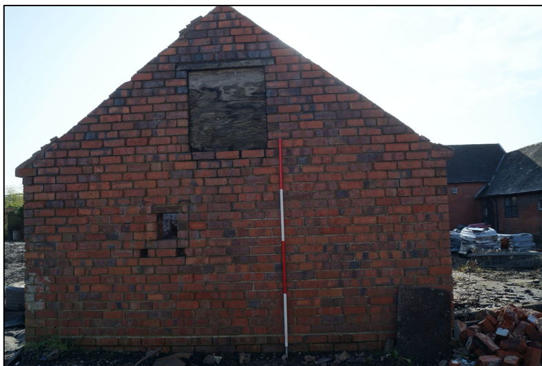
Plate 7. North elevation of extension to Barn 3.
