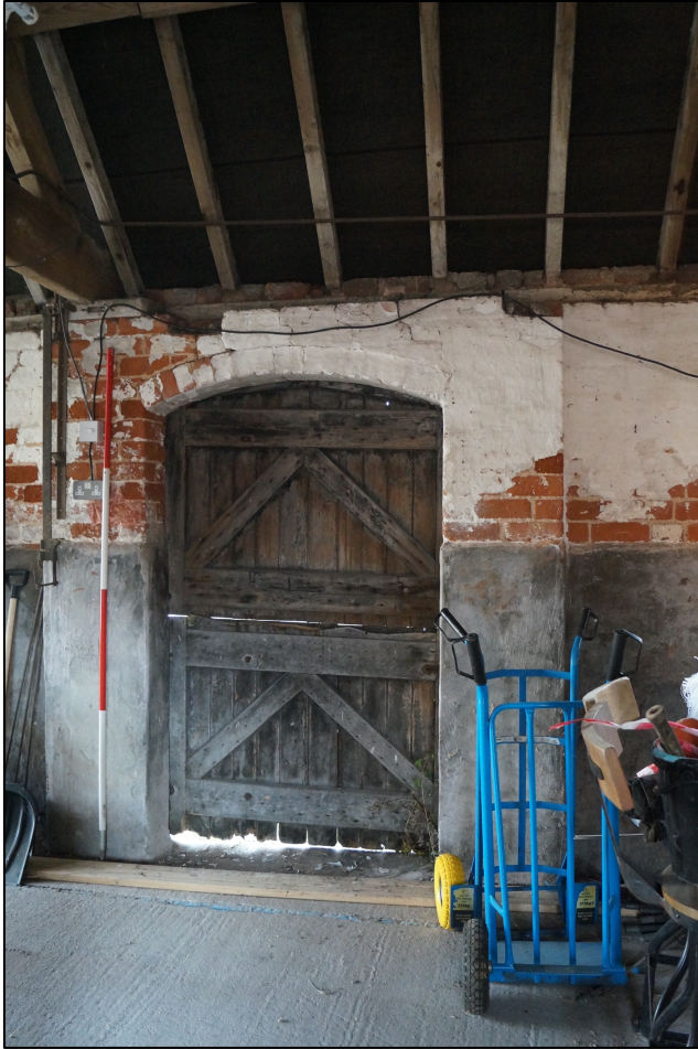
Plate 4. Detail of half rendered east wall with stable door.
