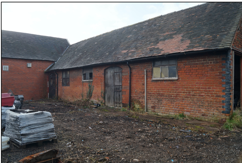
Plate 1. West facing elevation of Barn 2.
