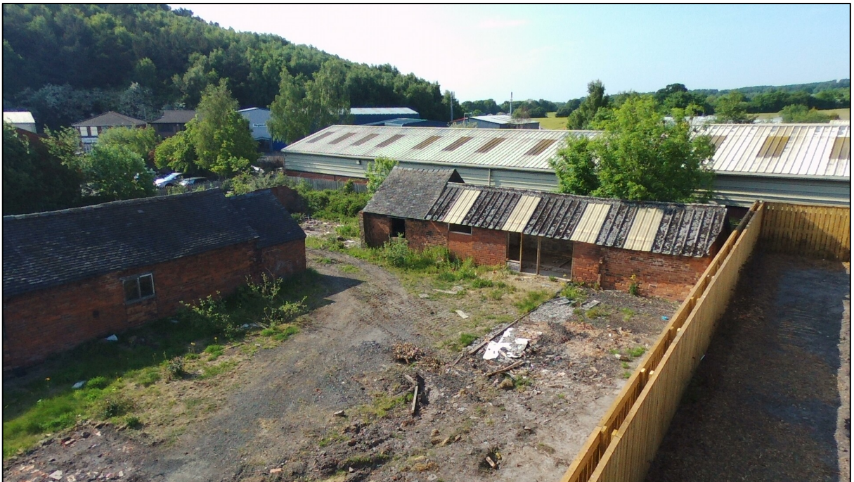
Plate 13. South facing elevation of Barn 1.
