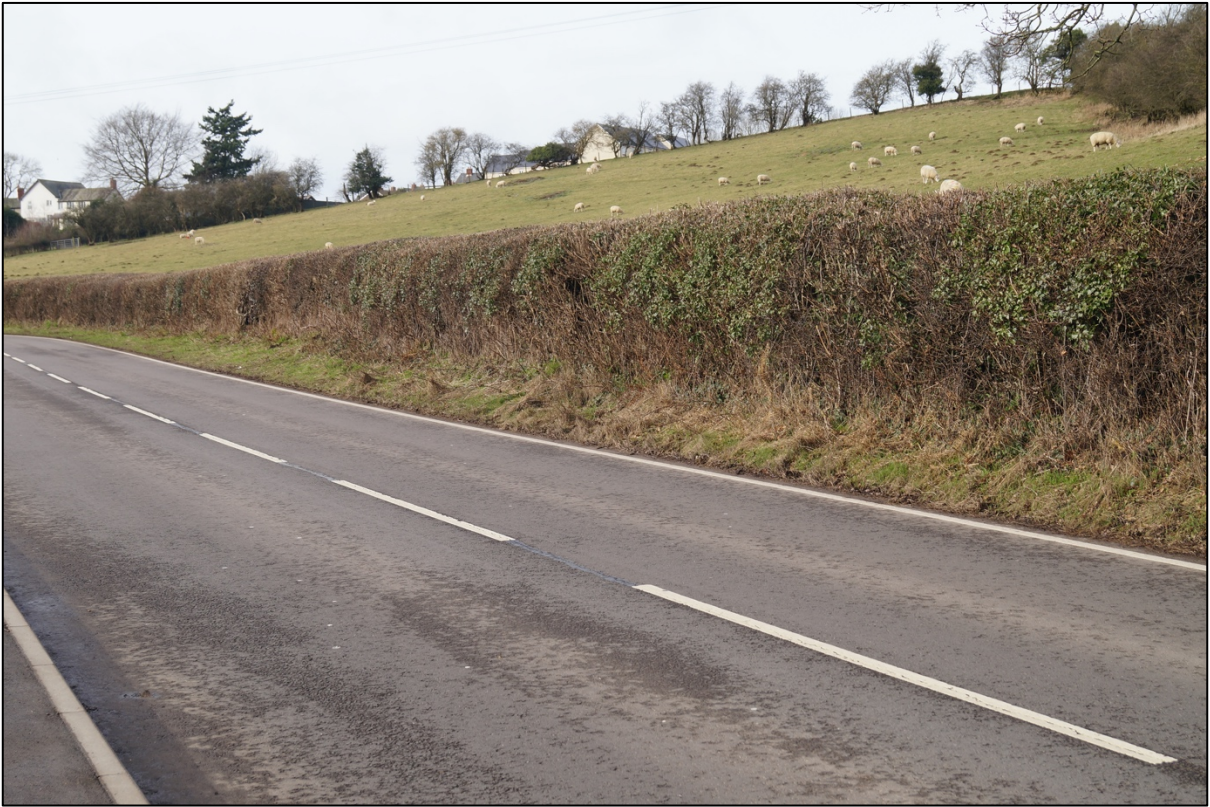
Plate 1. View of the PDA from Schoolhouse Lane.
