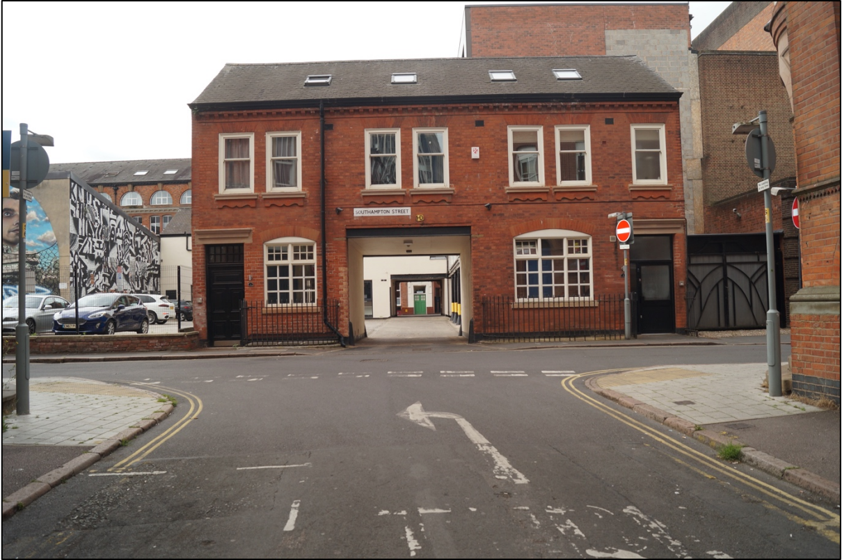
Plate 3. The entrance building into the PDA from Southampton Street.
