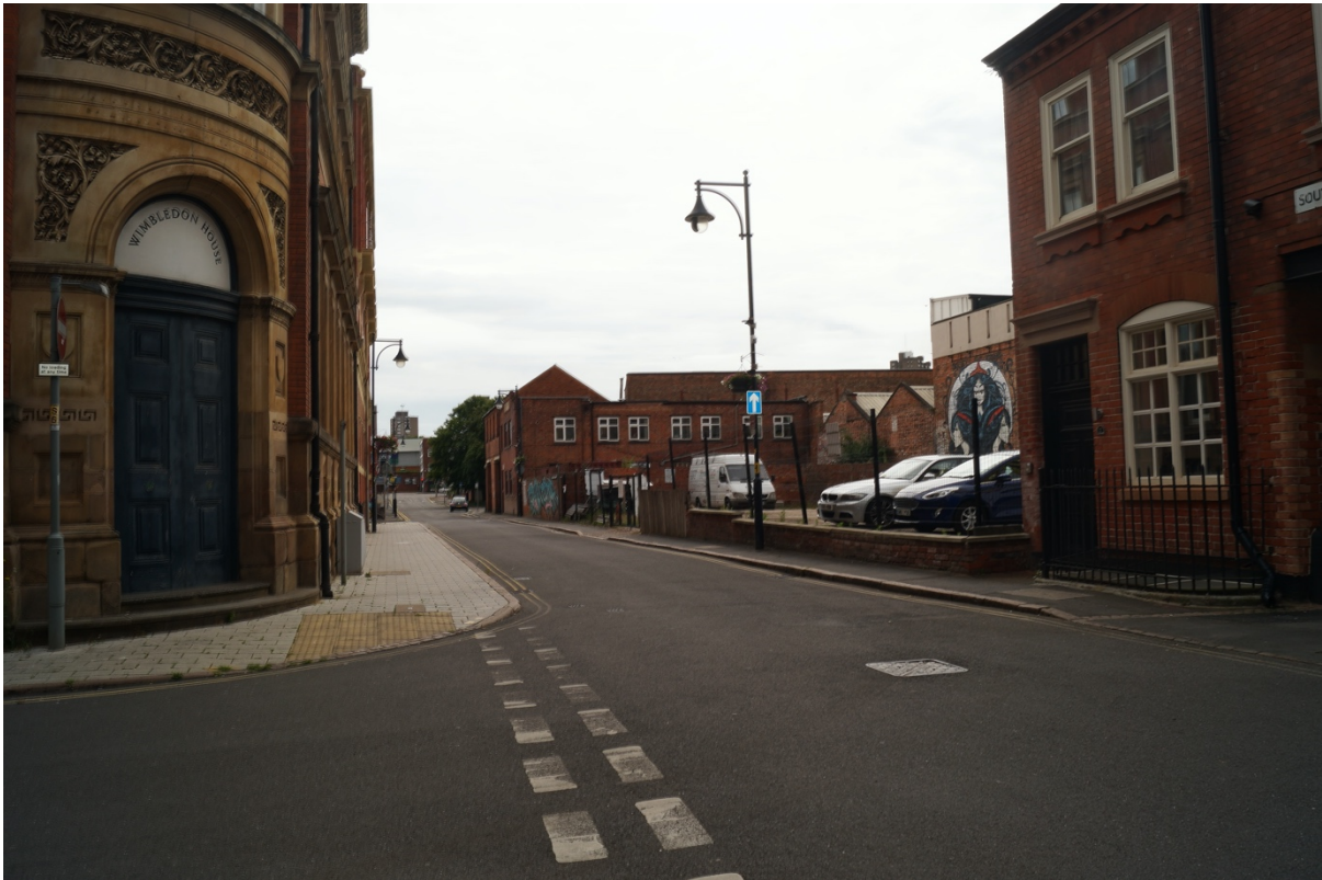
Plate 1. Showing the frontage of the PDA on Southampton Street.
