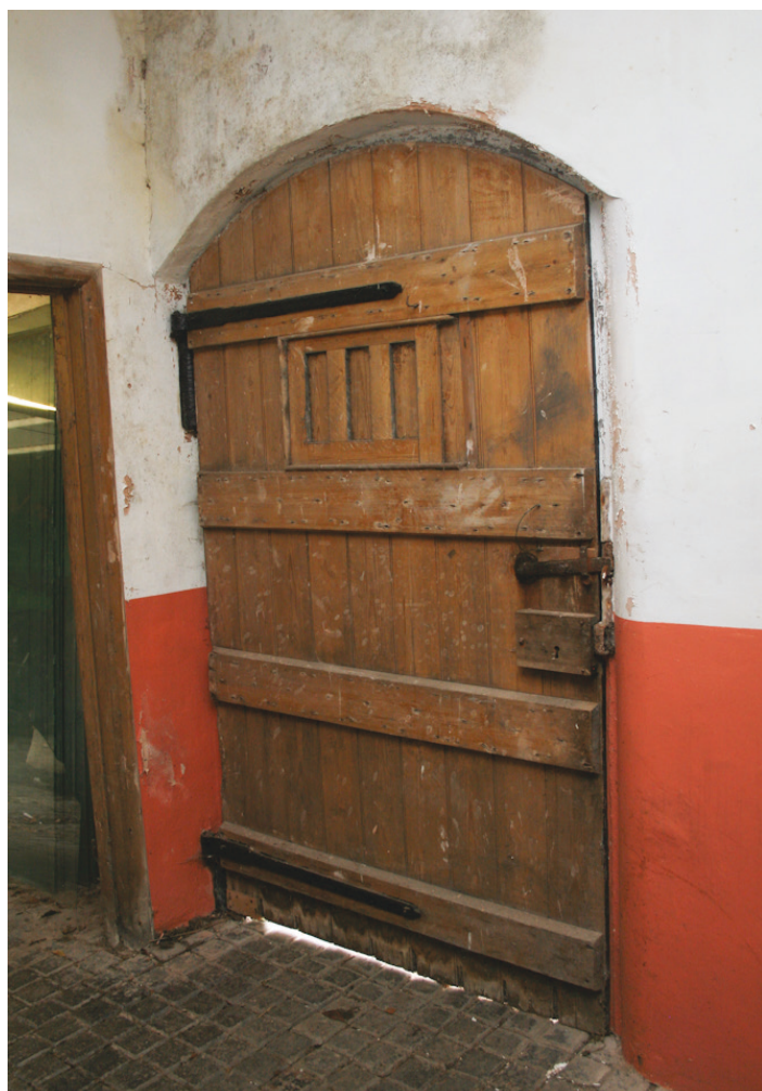
Ground_017 - boarded door to the stable on strap hinges with sliding hatch for ventilation (possibly a late C19 replacement of the original 1820s door)
