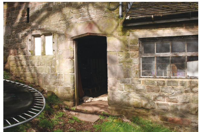
The Tudor-arched stable door and window are coeval with the end wall (left) with its ventilation slots
