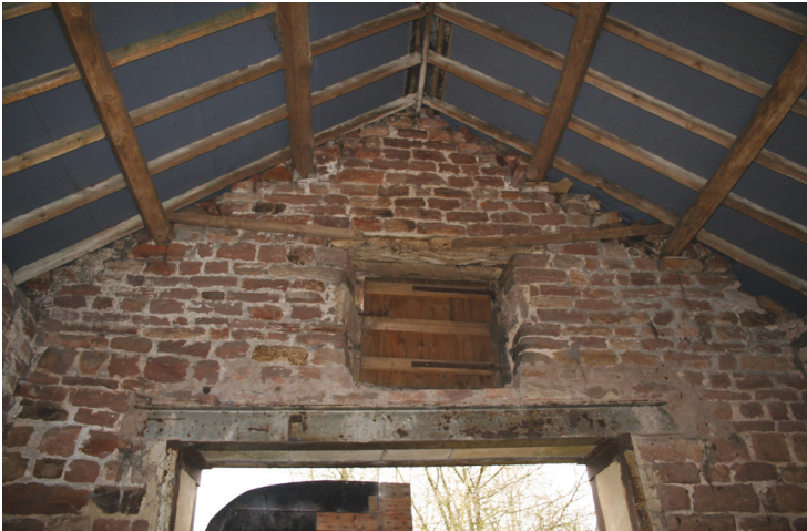
Left - 19th century brick piers inserted to replace oak posts and support the new lowered roof structure of king post trusses and double purlins. Right - imported Baltic timber (Scots pine) inscribed on the purlins with shipping containment / batch numbers
