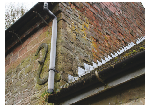
19th century re-roofing comprised inserting king post roof trusses, raising the eastern gable in brick, and lowering the eaves of the barn, remodelling the stable and inserting a new brick dividing wall to form a separate brick gable
