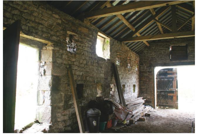
Left - three-bay threshing barn with multiple levels of ventilation for an open internal structure. Right - the door on the left is the main door, the two pitching eyes enable a continual process of adding unthreshed crops into the barn during harvest, until it slowly filled up. The large double-doors opening in the northern gable is a 20th century insertion.
