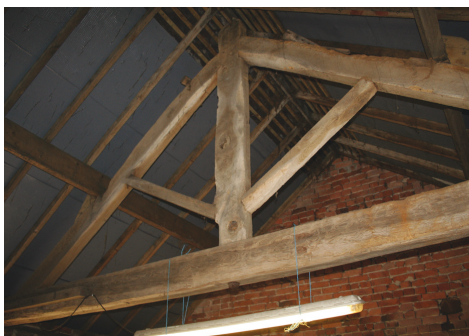
19th century re-roofing comprised inserting king post roof trusses, raising the eastern gable in brick, and lowering the eaves of the barn, remodelling the stable and inserting a new brick dividing wall to form a separate brick gable
