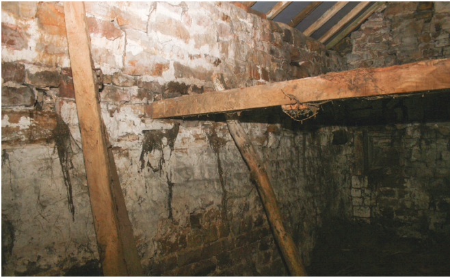
Oak joist re-positioned in wall socket and supported to demonstrate the level of the former hayloft floor. This demonstrates that it would have been efficient and simple to pitch hay and straw into the loft from the barn floor.
