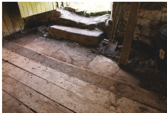
Main door (left) with keeping hole to the right. Above - stone threshing floor and 20th century butted boards, which may have replaced an earlier timber floor. Right - front elevation of wide doorway to threshing barn.
