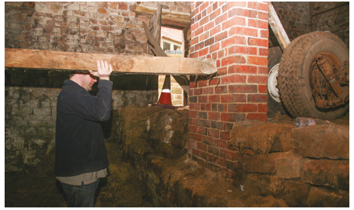
Oak joist re-positioned in wall socket and supported to demonstrate the level of the former hayloft floor. This demonstrates that it would have been efficient and simple to pitch hay and straw into the loft from the barn floor.
