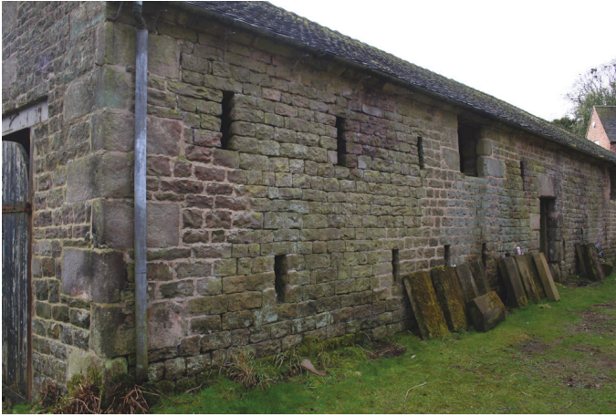
Left - three-bay threshing barn with multiple levels of ventilation for an open internal structure. Right - the door on the left is the main door, the two pitching eyes enable a continual process of adding unthreshed crops into the barn during harvest, until it slowly filled up. The large double-doors opening in the northern gable is a 20th century insertion.
