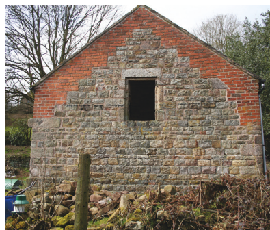
19th century re-roofing comprised inserting king post roof trusses, raising the eastern gable in brick, and lowering the eaves of the barn, remodelling the stable and inserting a new brick dividing wall to form a separate brick gable
