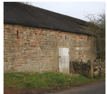
Roadside elevation, with inserted doorway (C18?)
