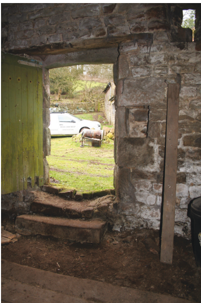
Main door (left) with keeping hole to the right. Above - stone threshing floor and 20th century butted boards, which may have replaced an earlier timber floor. Right - front elevation of wide doorway to threshing barn.
