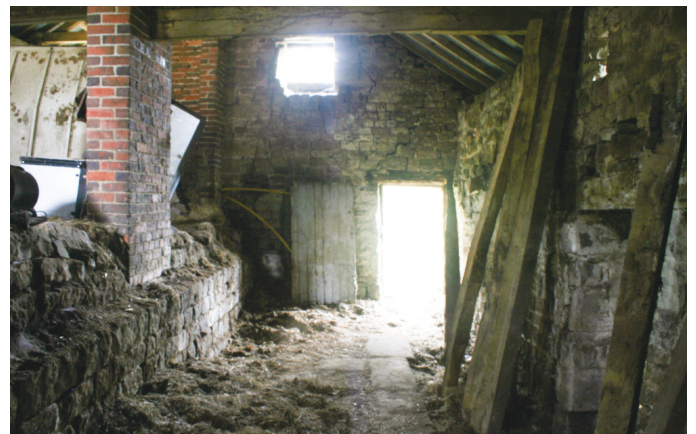
Left - coursed and mortared stone plinth (looking south), which would have supported a short timber-framed structure of posts and horizontal rails; sockets survive in the south wall. Right - the cowhouse looking north, with 19th century brick piers.
