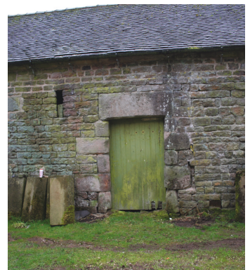
Main door (left) with keeping hole to the right. Above - stone threshing floor and 20th century butted boards, which may have replaced an earlier timber floor. Right - front elevation of wide doorway to threshing barn.
