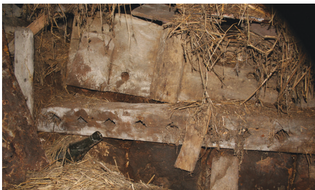
Fragment of oak rack with sockets for staves is part bedded in the lower wall
