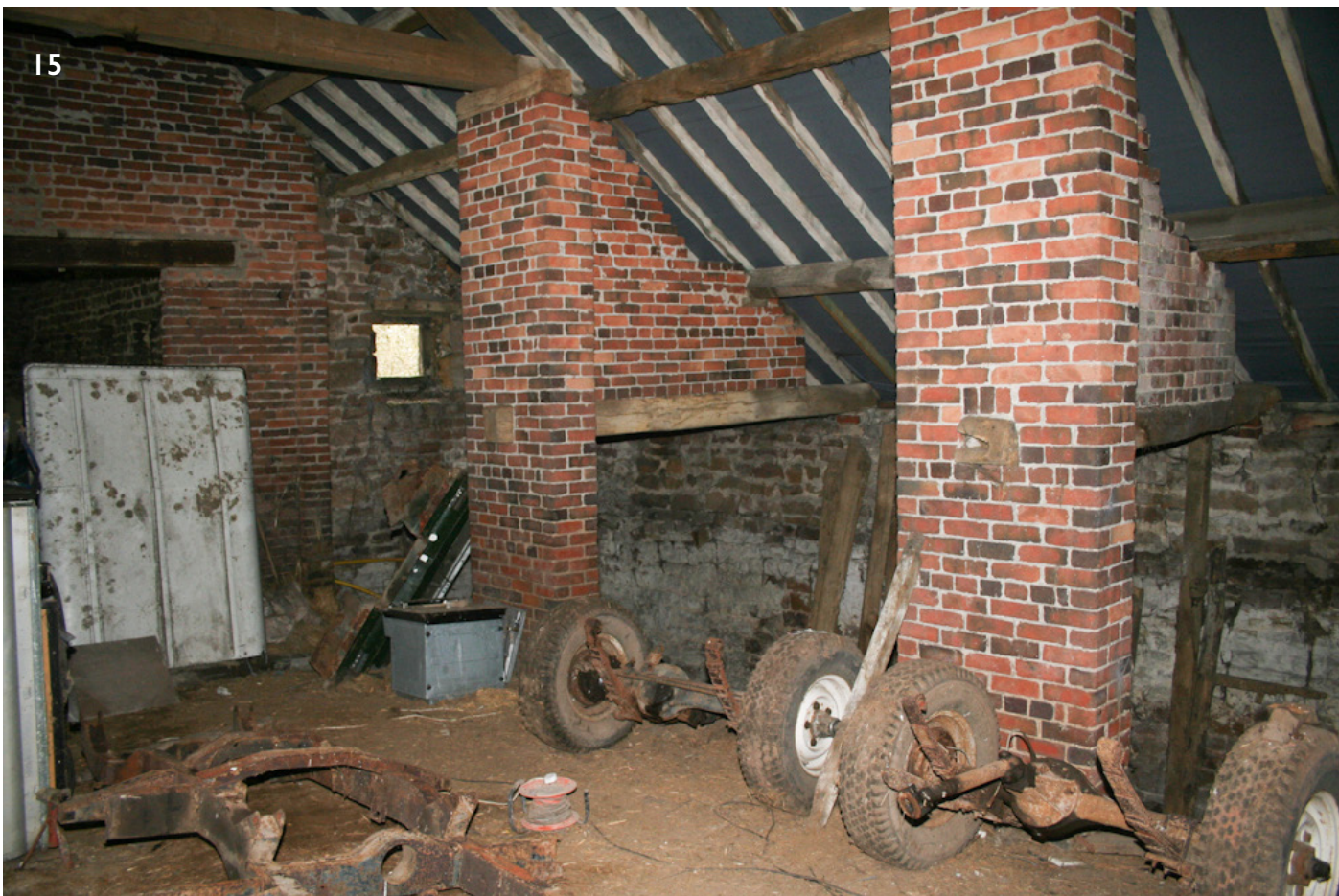
15 - Southern half of the Bank Barn, with view of inserted 19th century brick piers and cross wall to the cowhouse and view through to the cowhouse at the lower level.
