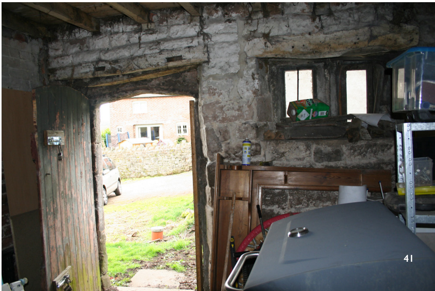
41 - View of front Stable door and chamfered stone mulioned window with oak lintels, 17th century stable 42 - 19th century king post truss with coach bolt threaded between tie beam and main post, and struts to the principal rafters. This is one of two inserted trusses in the Stable Range
