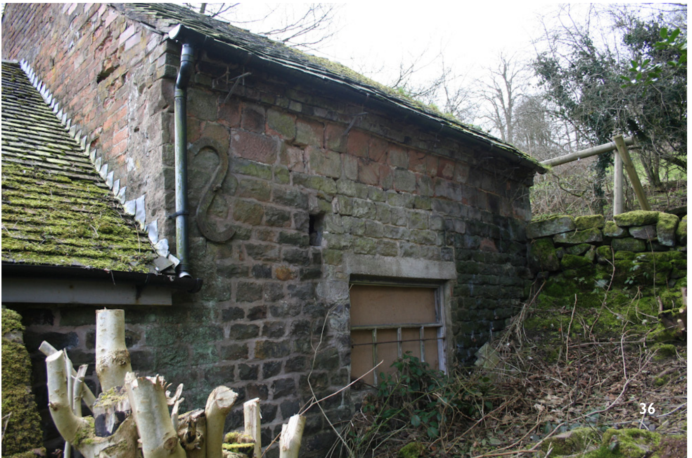
36 - Rear elevation of Stable, altered in the 19th century with coursed stone raised in two courses of pink sandstone, with corbelled brick eaves.
