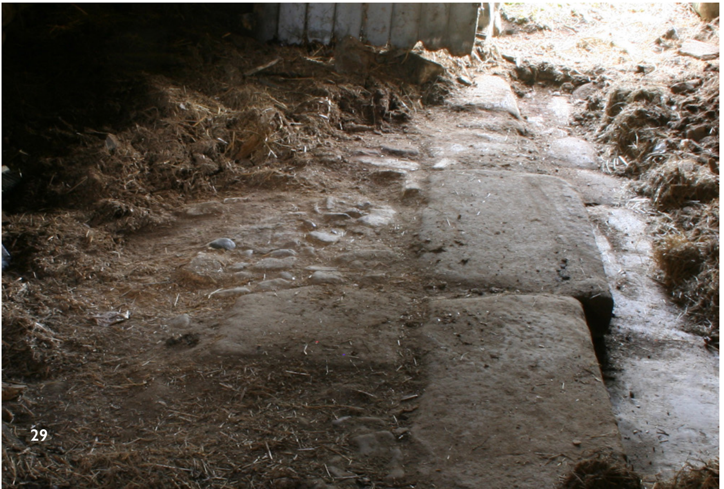
29 - Detail of stone paving flags, kerbs and pitching to cowhouse floor
