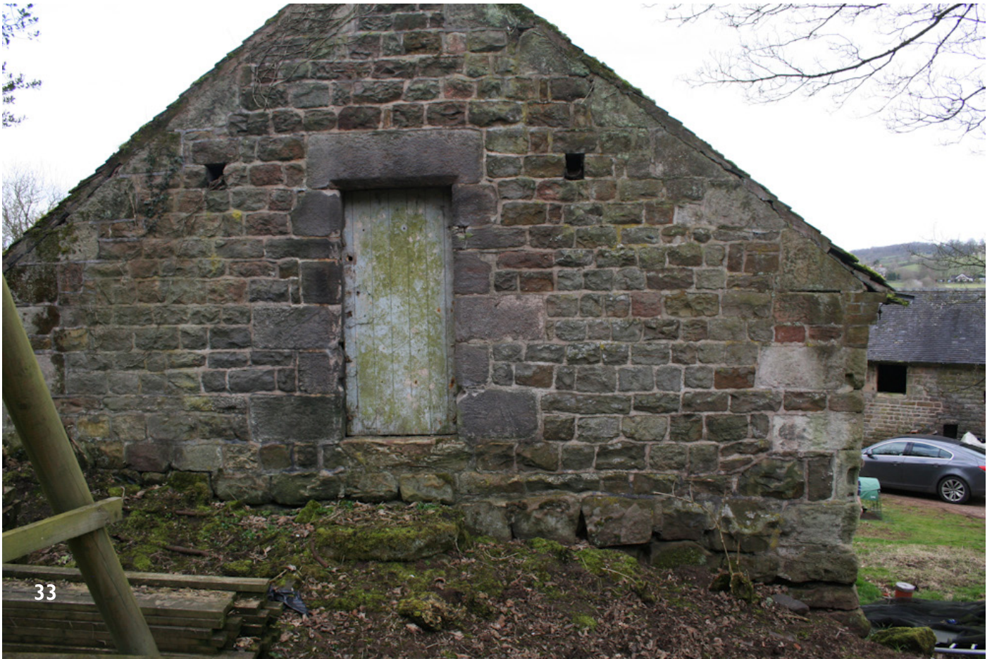
33 - Stable range. Gable end to the west with chamfered door surround and large verge stones; coping to gable removed. The gable was probably heightened when the eaves of the Stable was raised.
