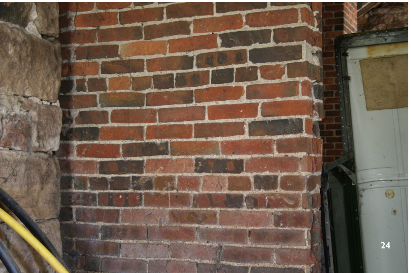
23 - Stone paving flags form the wide threshold in the threshing bay and may have continued across the whole bay. Timber planks are butted up across the former threshing floor and may have replaced an earlier timber floor 24 - brickwork to the dividing wall in English garden wall bond, of mid 18th century date; the wall was chopped back during the late 20th century
