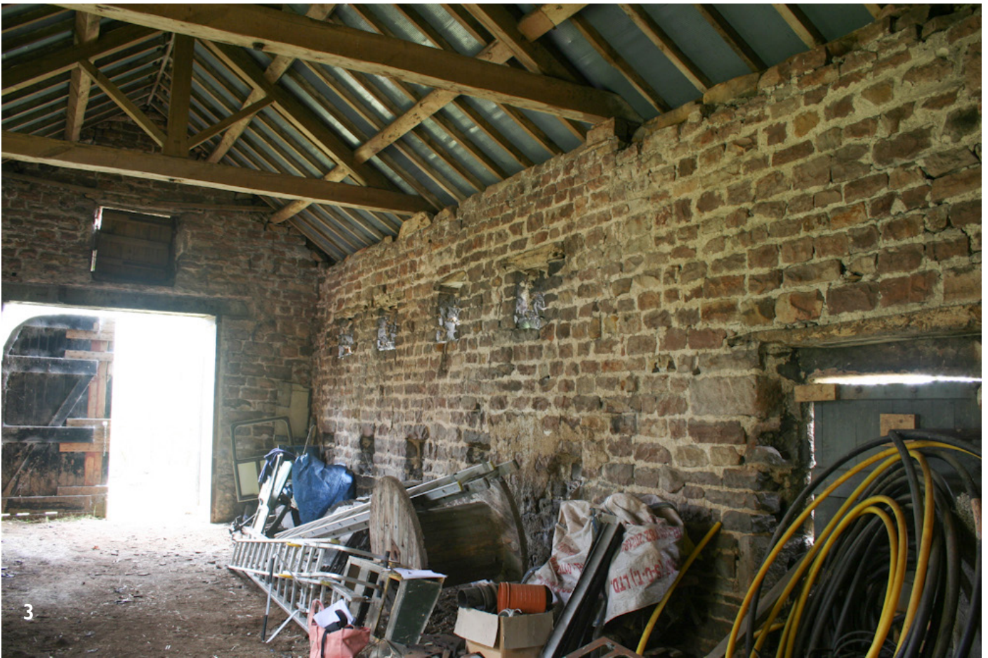
3 - Eastern internal wall of threshing barn with large chamfered ventilation slits, stone lintels to ground level slits and oak lintels to higher level. The door to the right is the "winnowing" door. 4 - Western wall to threshing barn with pitching eyes to upper wall and gable end. The main barn door lies to the left, with heavy dressed chamfered surround. Roof of Scots pine (Baltic timber) inserted in mid 19th century with king post trusses.
