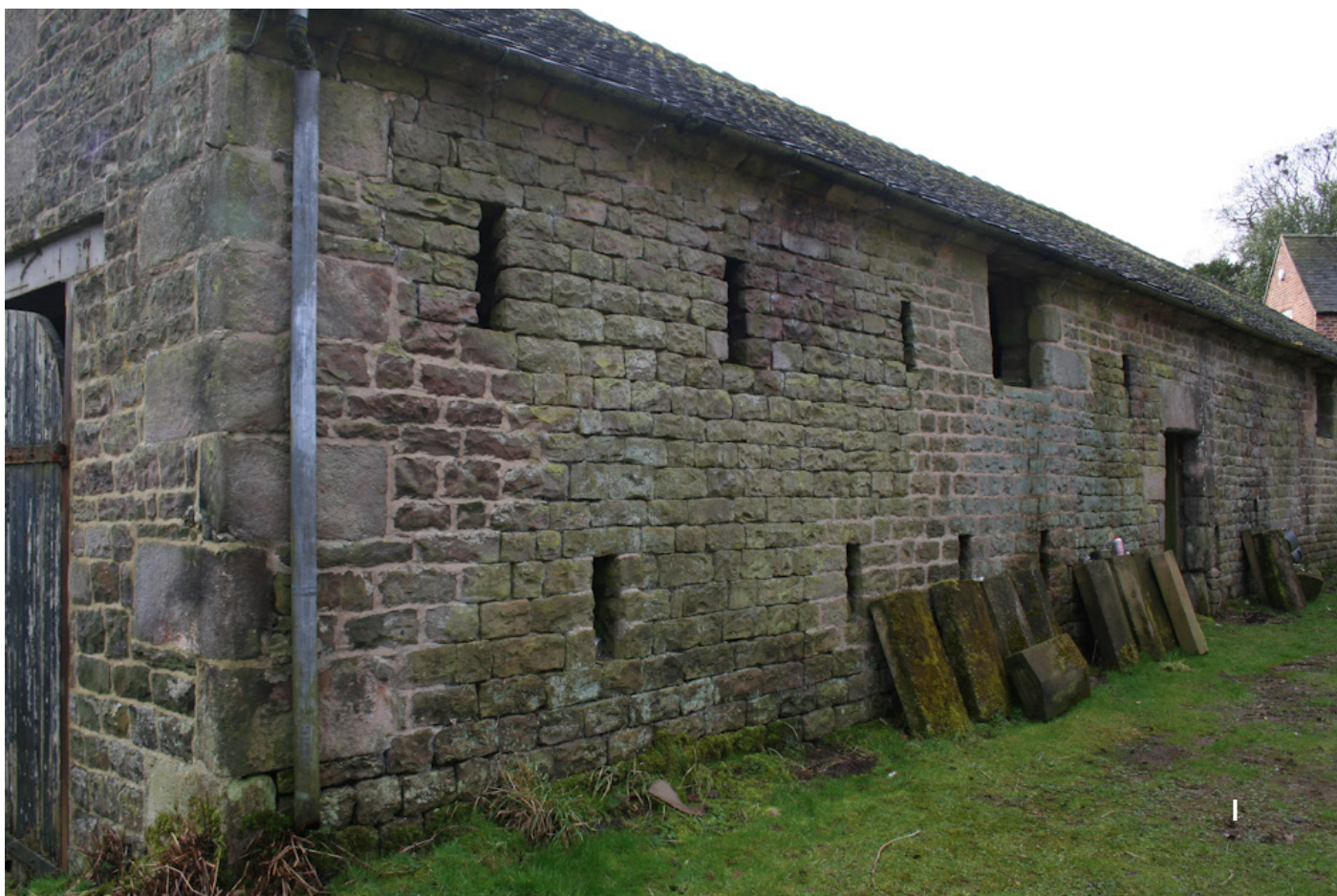
1 - Threshing barn with large ventilation slits, large stone quoins, squared rubble, chamfered surrounds to pitching eyes and doors, and straight chamfered stone eaves. 2 - chamfered surround to quoined pitching eye, with rebated masonry. The split-faced coursed surrounding masonry shows surprisingly few signs of weathering and age, compared with the dressings, but there are no indications that this has been rebuilt and it is entirely consistent, perhaps reflecting a different quarried source.
