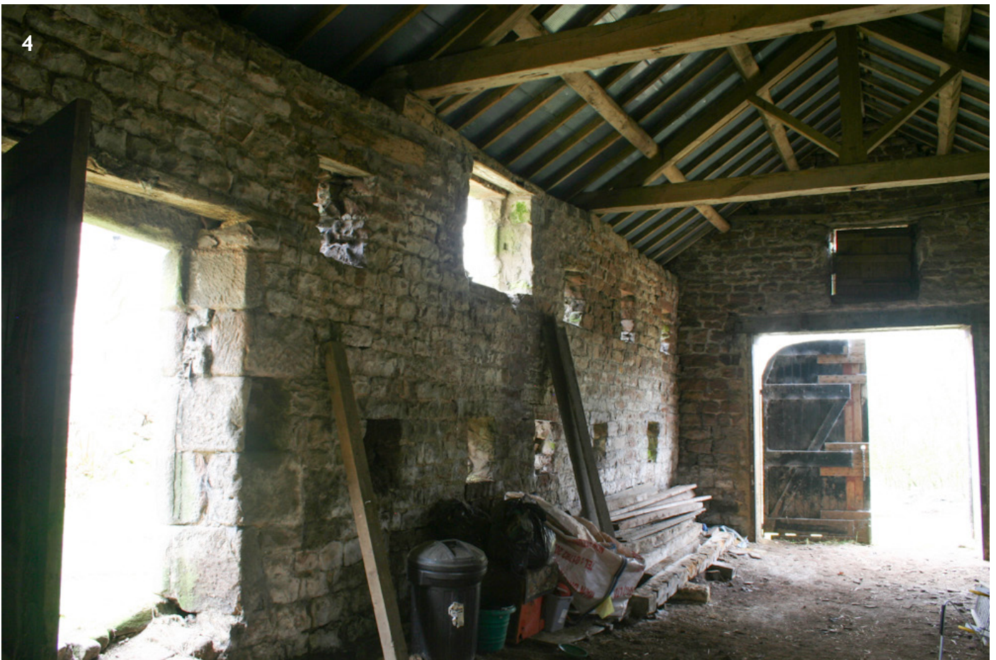
3 - Eastern internal wall of threshing barn with large chamfered ventilation slits, stone lintels to ground level slits and oak lintels to higher level. The door to the right is the "winnowing" door. 4 - Western wall to threshing barn with pitching eyes to upper wall and gable end. The main barn door lies to the left, with heavy dressed chamfered surround. Roof of Scots pine (Baltic timber) inserted in mid 19th century with king post trusses.
