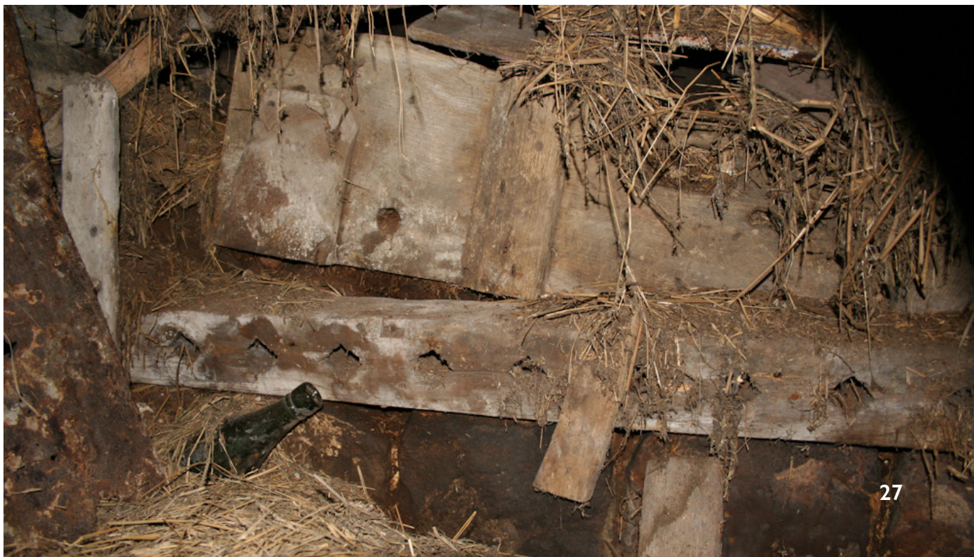
27 - fragments of oak manger, ex-situ, and lodged in the base of the cowhouse wall, with an old shutter or boarded door. The manger contained diamond-section slots for staves.
