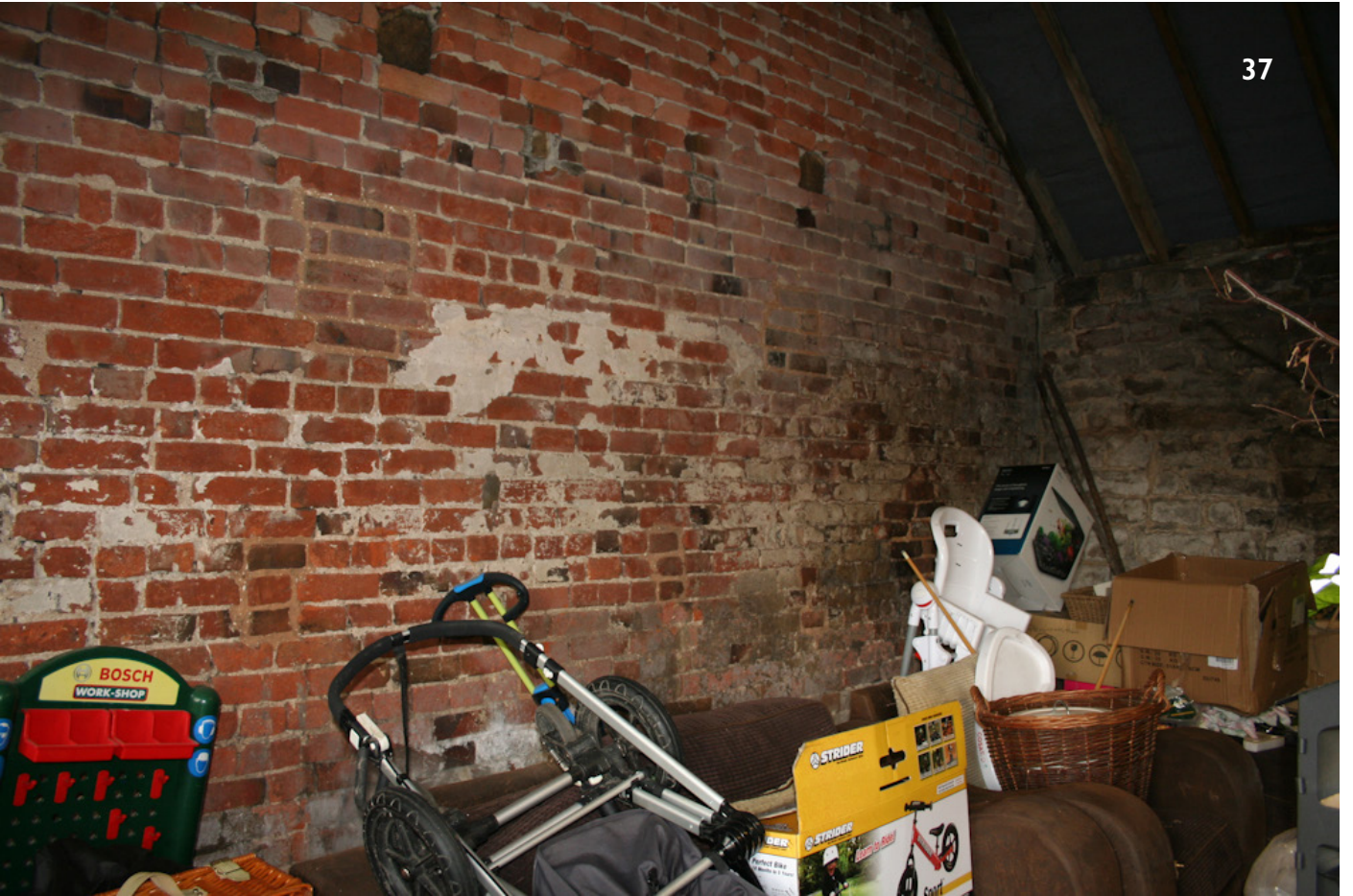
37 - 18th century brick wall dividing upper two bays from lower third bay to former 17th century combination building 38 - Stable with 19th century oak beams, joists and boarded floor to hayloft
