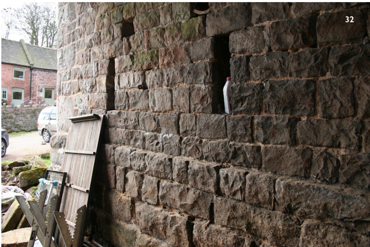
32 - Detail of stone plinth, squared rubble masonry with large courses to plinth, ventilation slits, and sockets for a former inserted floor
