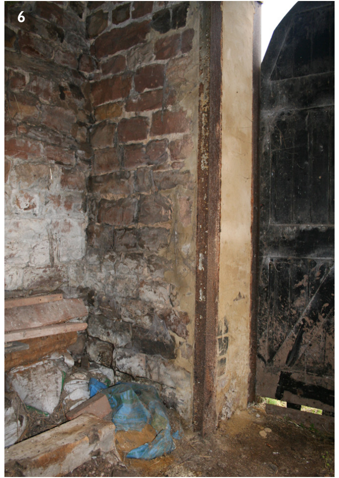
5 - Main door to threshing barn with rebated frame, splayed internal angle, and "keeping hole" to right.
