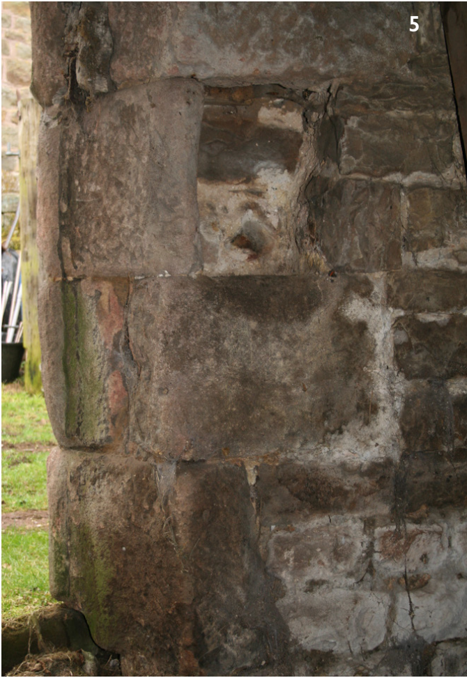
5 - Main door to threshing barn with rebated frame, splayed internal angle, and "keeping hole" to right.
