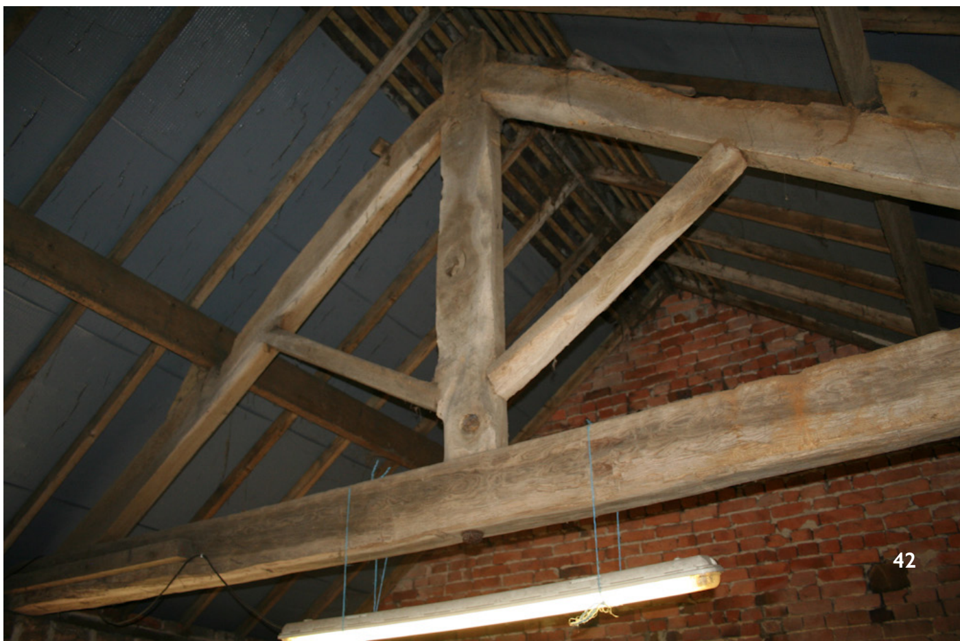
41 - View of front Stable door and chamfered stone mulioned window with oak lintels, 17th century stable 42 - 19th century king post truss with coach bolt threaded between tie beam and main post, and struts to the principal rafters. This is one of two inserted trusses in the Stable Range
