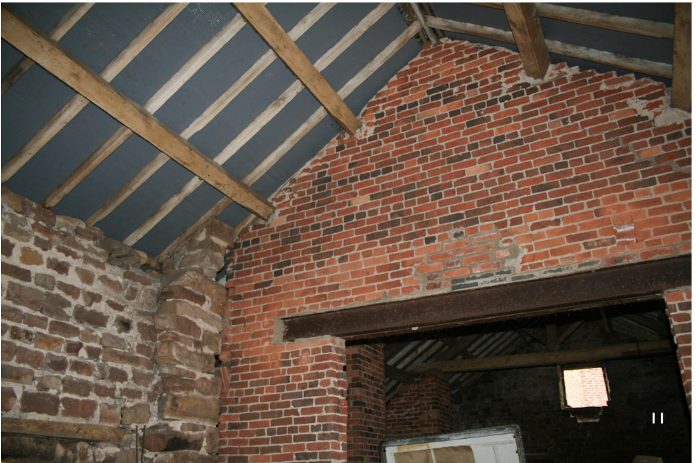
11 - Inserted brick wall, with 18th century brick piers (cut back) and 19th century brickwork at the level of the steel lintel and above. Steel lintel inserted during 20th century. 12 - eastern wall of the threshing barn with regular coursed masonry and two tiers of ventilation holes
