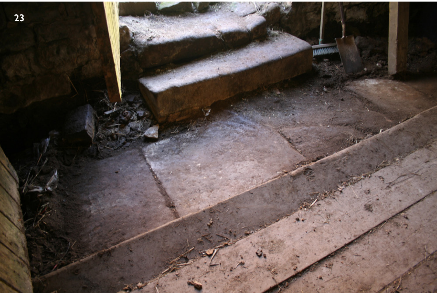
23 - Stone paving flags form the wide threshold in the threshing bay and may have continued across the whole bay. Timber planks are butted up across the former threshing floor and may have replaced an earlier timber floor 24 - brickwork to the dividing wall in English garden wall bond, of mid 18th century date; the wall was chopped back during the late 20th century
