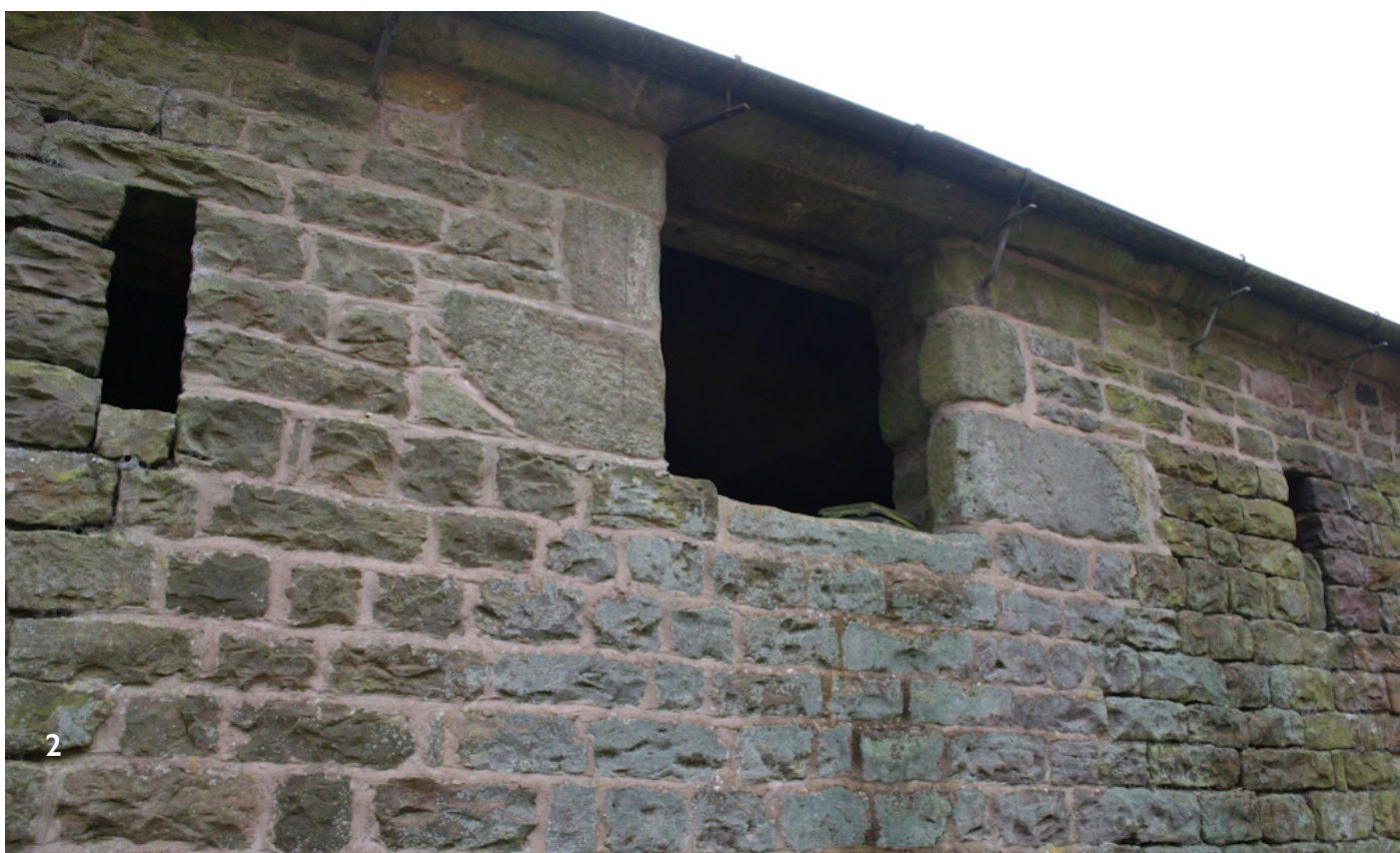
1 - Threshing barn with large ventilation slits, large stone quoins, squared rubble, chamfered surrounds to pitching eyes and doors, and straight chamfered stone eaves. 2 - chamfered surround to quoined pitching eye, with rebated masonry. The split-faced coursed surrounding masonry shows surprisingly few signs of weathering and age, compared with the dressings, but there are no indications that this has been rebuilt and it is entirely consistent, perhaps reflecting a different quarried source.
