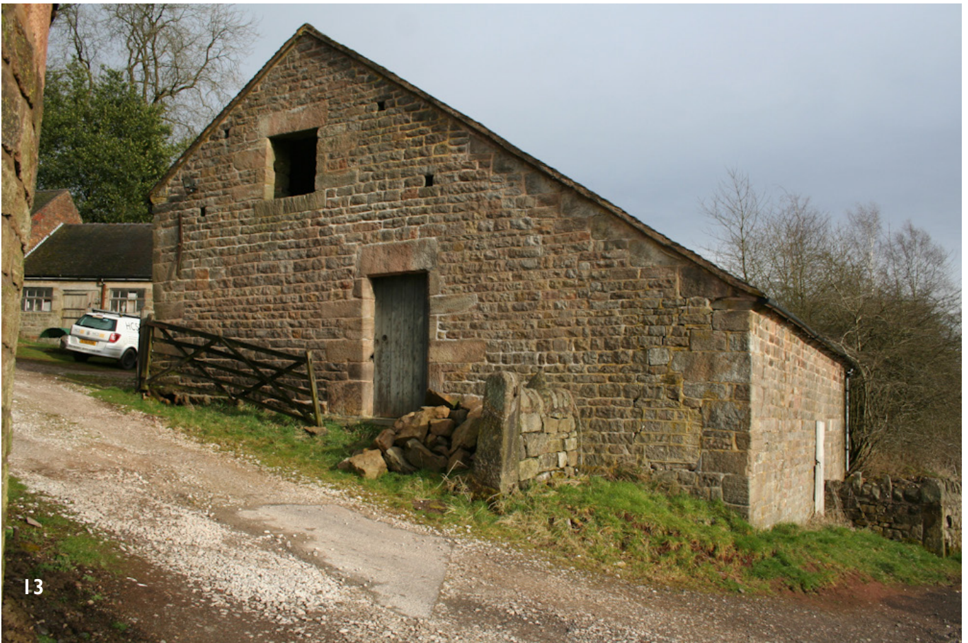
13 - Bank Barn - view from Brook Lane. This view shows the original verge stones to the raised stone coped gables in-situ at the lower level
