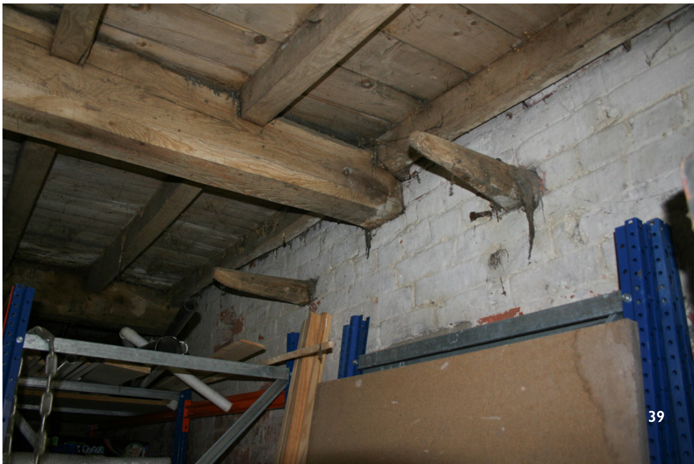
39 - 19th century inserted brick wall to Stable with oak brackets for saddles and tack 40 - horse hay manger to loose-box type stable, Stable Range
