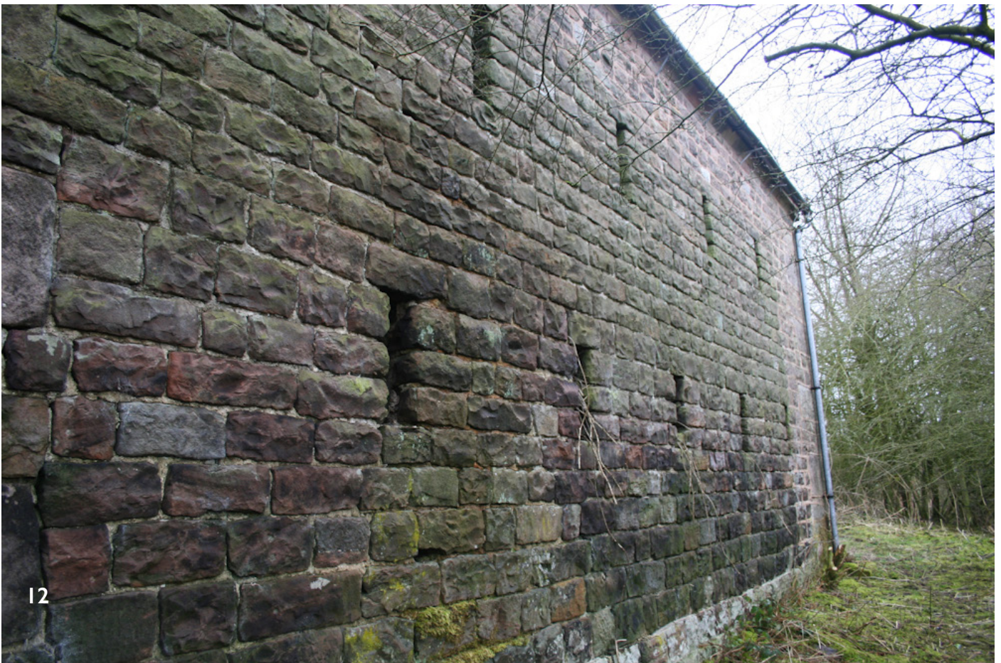
11 - Inserted brick wall, with 18th century brick piers (cut back) and 19th century brickwork at the level of the steel lintel and above. Steel lintel inserted during 20th century. 12 - eastern wall of the threshing barn with regular coursed masonry and two tiers of ventilation holes
