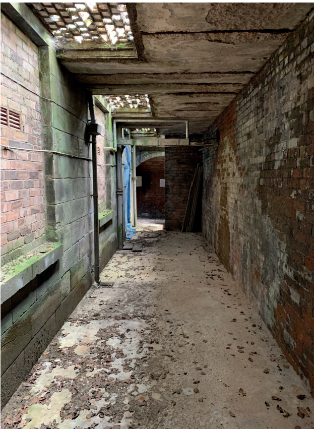
Left - 2020 view within the basement lightwell. The blocked windows to the left formerly lit the servant's hall at basement level. The lightwell is covered over with steel beams, cast-concrete slabs and pavement glazing.
