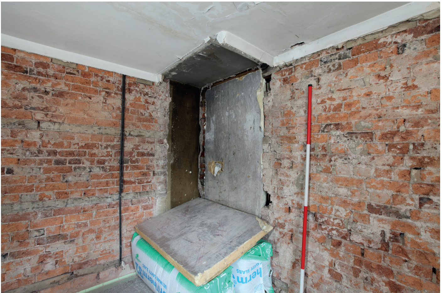
g6_017_14.06.21 Partition for safe and plaster removed
