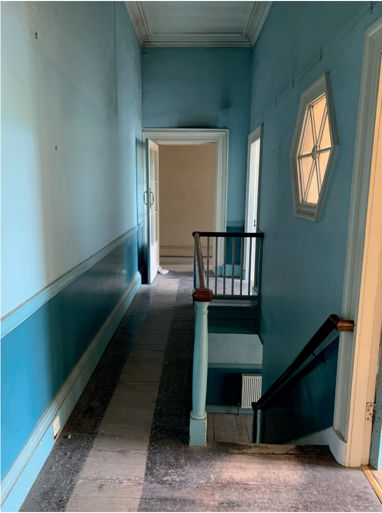
f10_002_14.05.20 first floor service stairs of 1851
