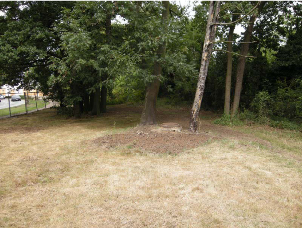
Fig 5 Disturbed surface scar following the removal of the Camp Bling structure shown above which originally enclosed the manhole (looking N)
