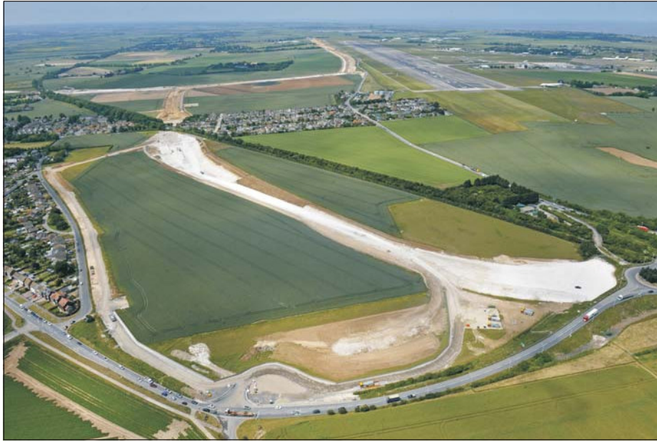
Plate 3: Aerial photograph: Zones 13 – 15 and 26 (view from east)
