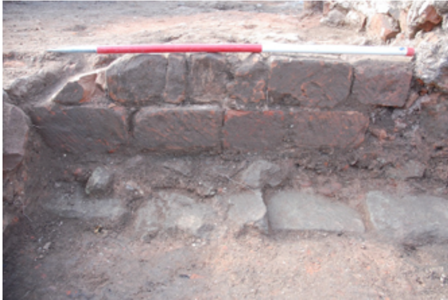
Figure 31: Medieval wall CG36, facing south
