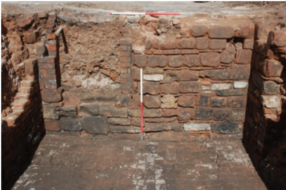
Figure 27: Sandstone cellar walls CG58, facing north
