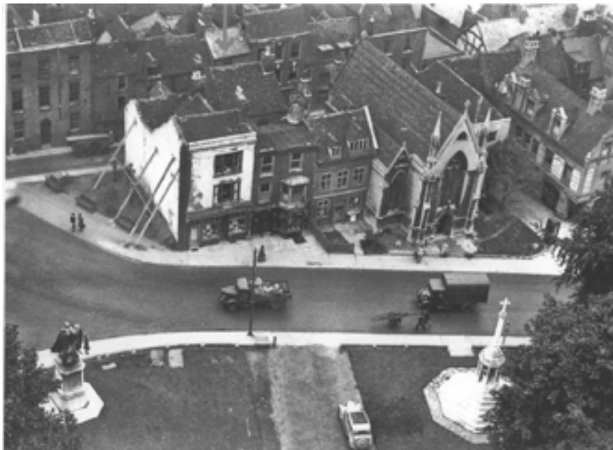
Figure 10: No. 2 Lich Street and No. 3 College Street supported by props (WAAS)
