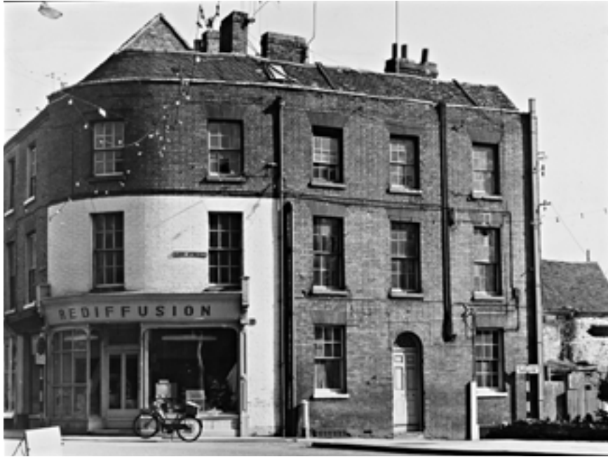
Figure 15: No. 1 High Street/No. 1 Lich Street in the 1960s (WAAS).
