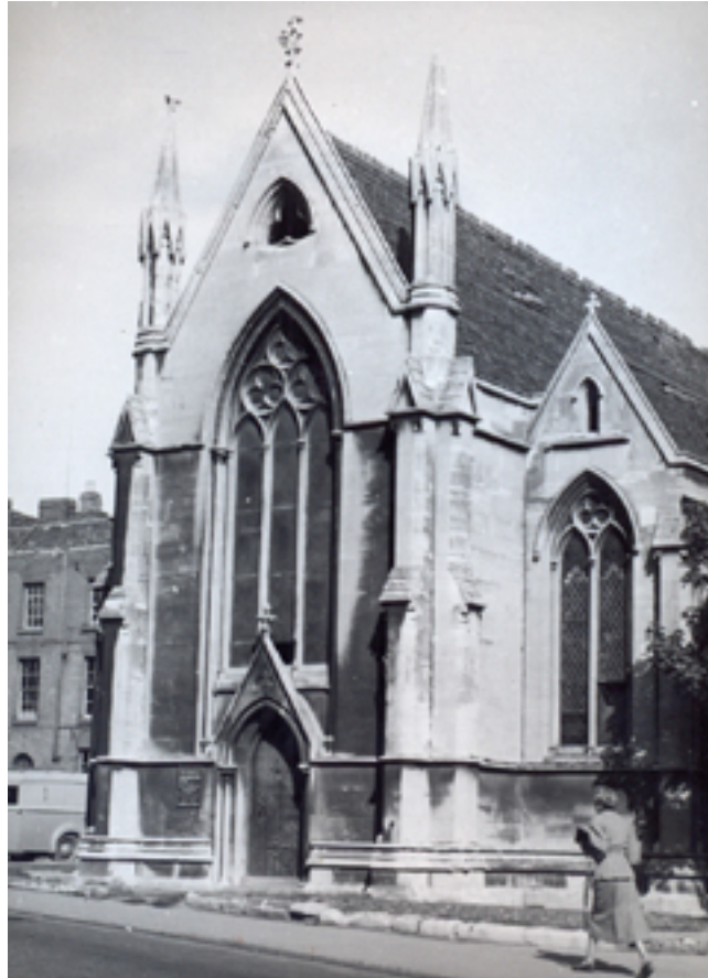
Figure 9: The new St Michael's church with College Street in the foreground (WAAS)
