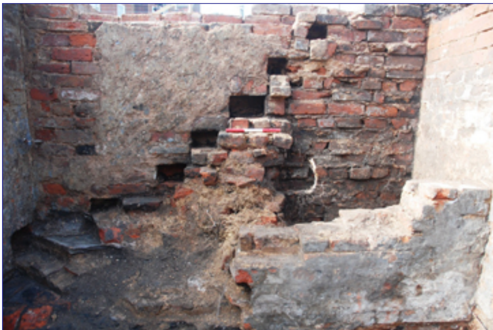
Figure 18: Staircase in No. 3 cellar (ecclesiastical stonework was in space behind wall in foreground)
