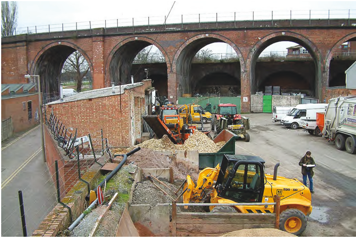
Plate 192: Railway viaduct running across the site, west to the left
