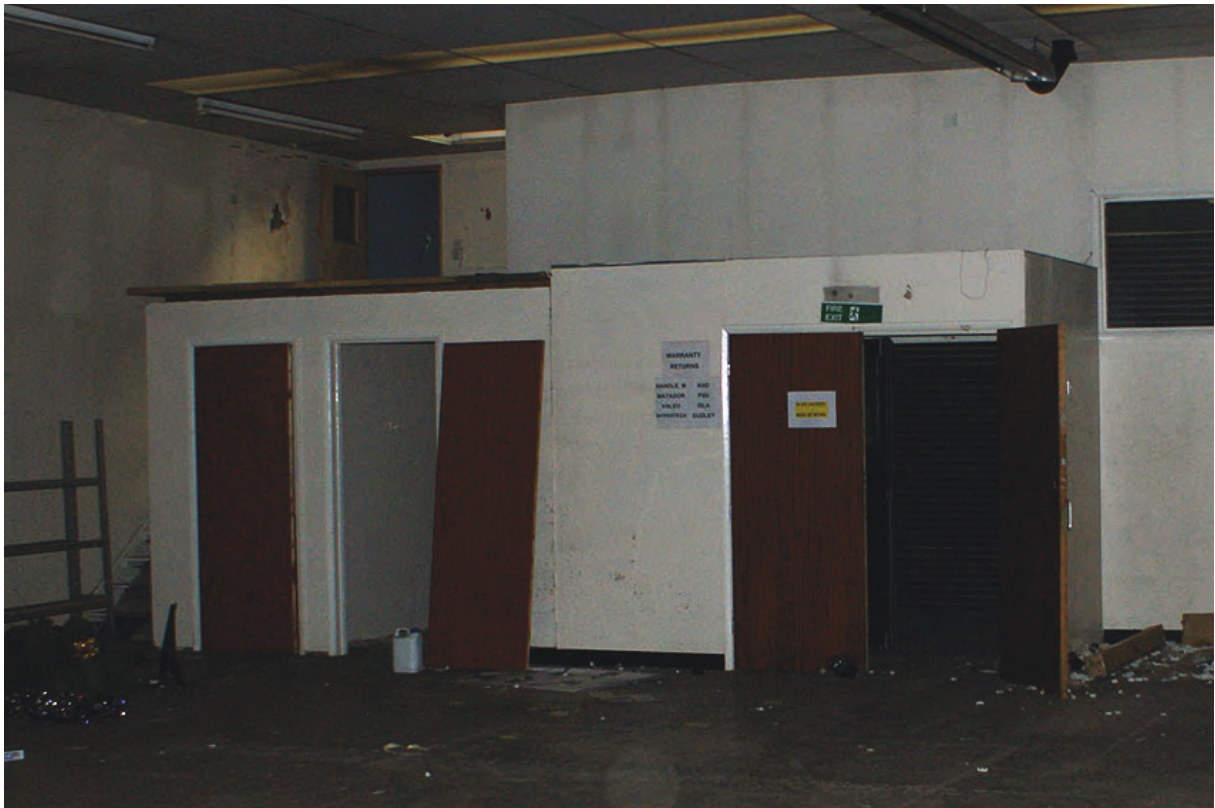
Plate 30: New breeze block utility rooms
