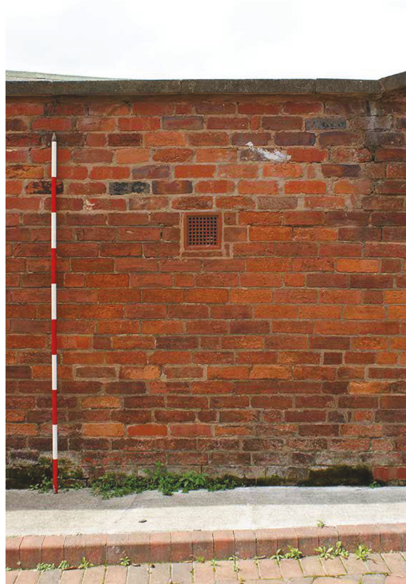
Plate 53: Flemish Bond brickwork of Netherton Lane wall
