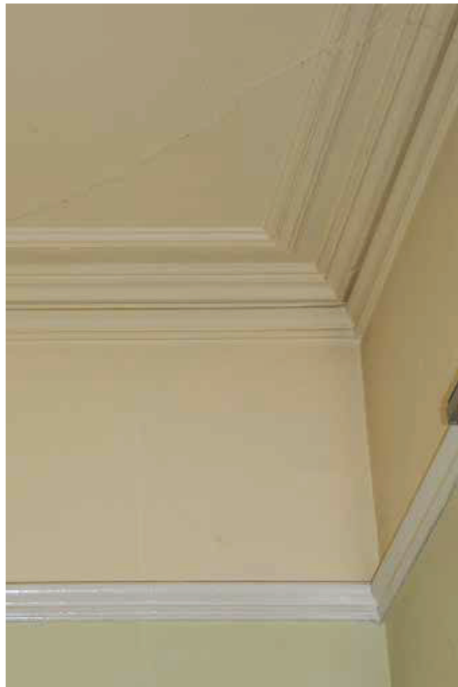
Plate 121: Cornice and picture rail, Room F1
