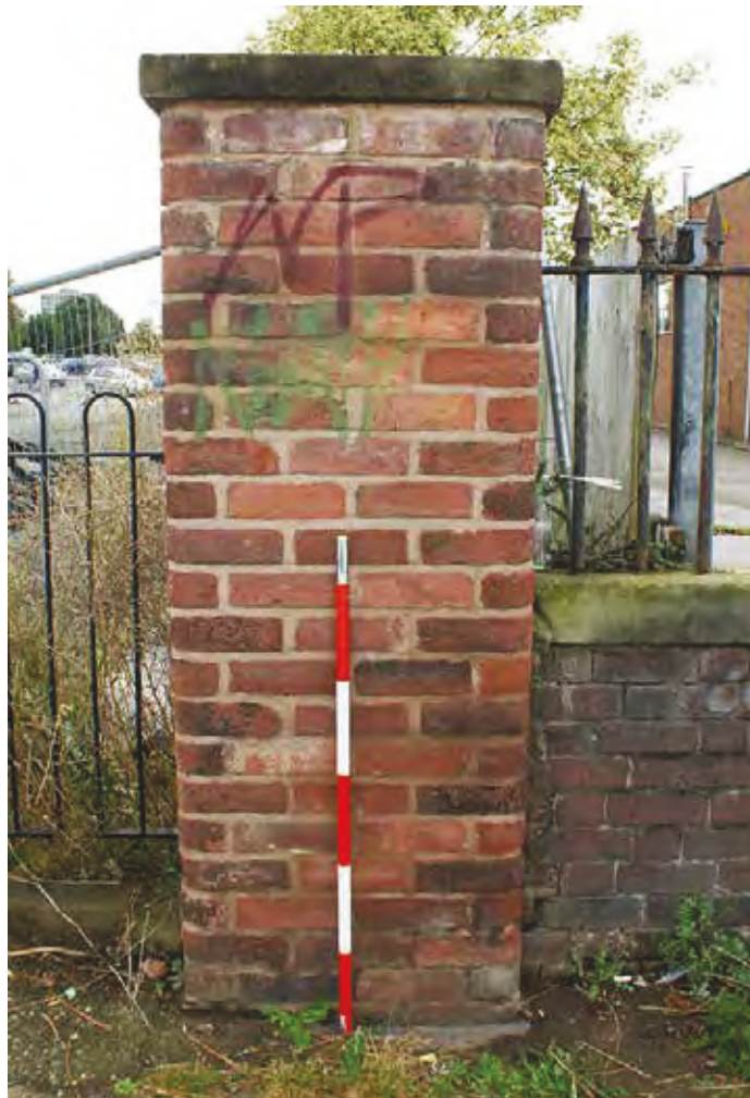
Plate 78: South pier of Coomber's boundary wall
