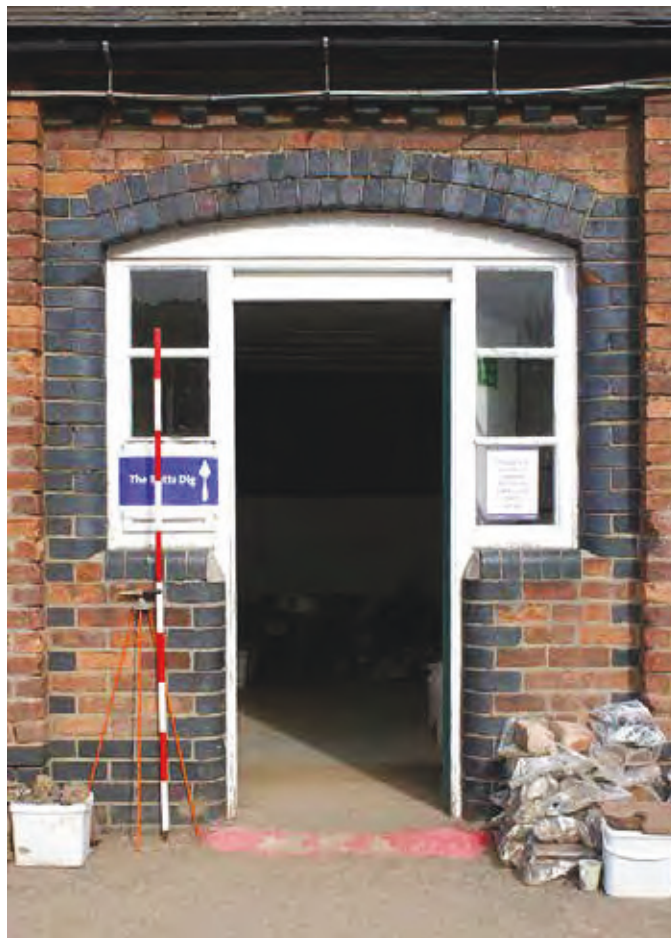
Plate 103: Door way of single-storey range showing blue brick detail
