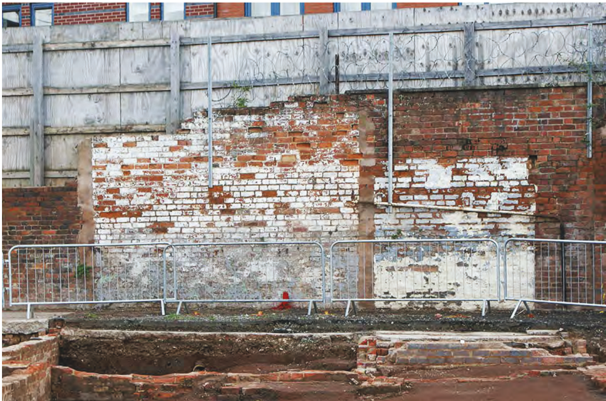
Plate 64: Foundations of range of buildings and the corresponding building scars on the wall
