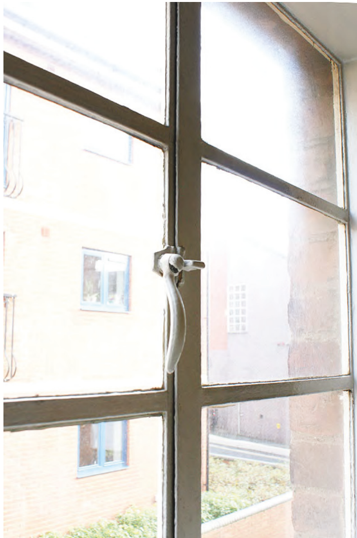
Plate 132: Curved turnbuckle window catch
