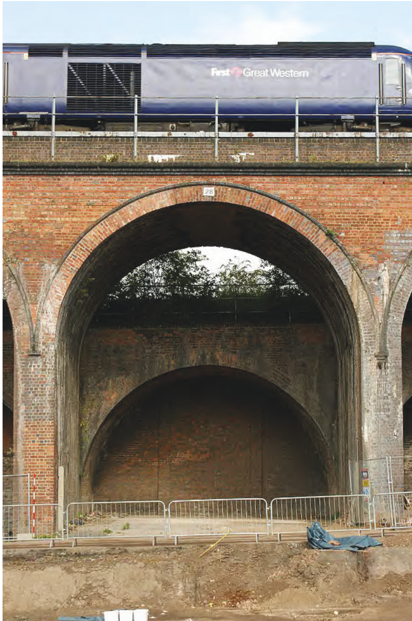
Plate 195: Viaduct arch showing stepped cornice and parapet
