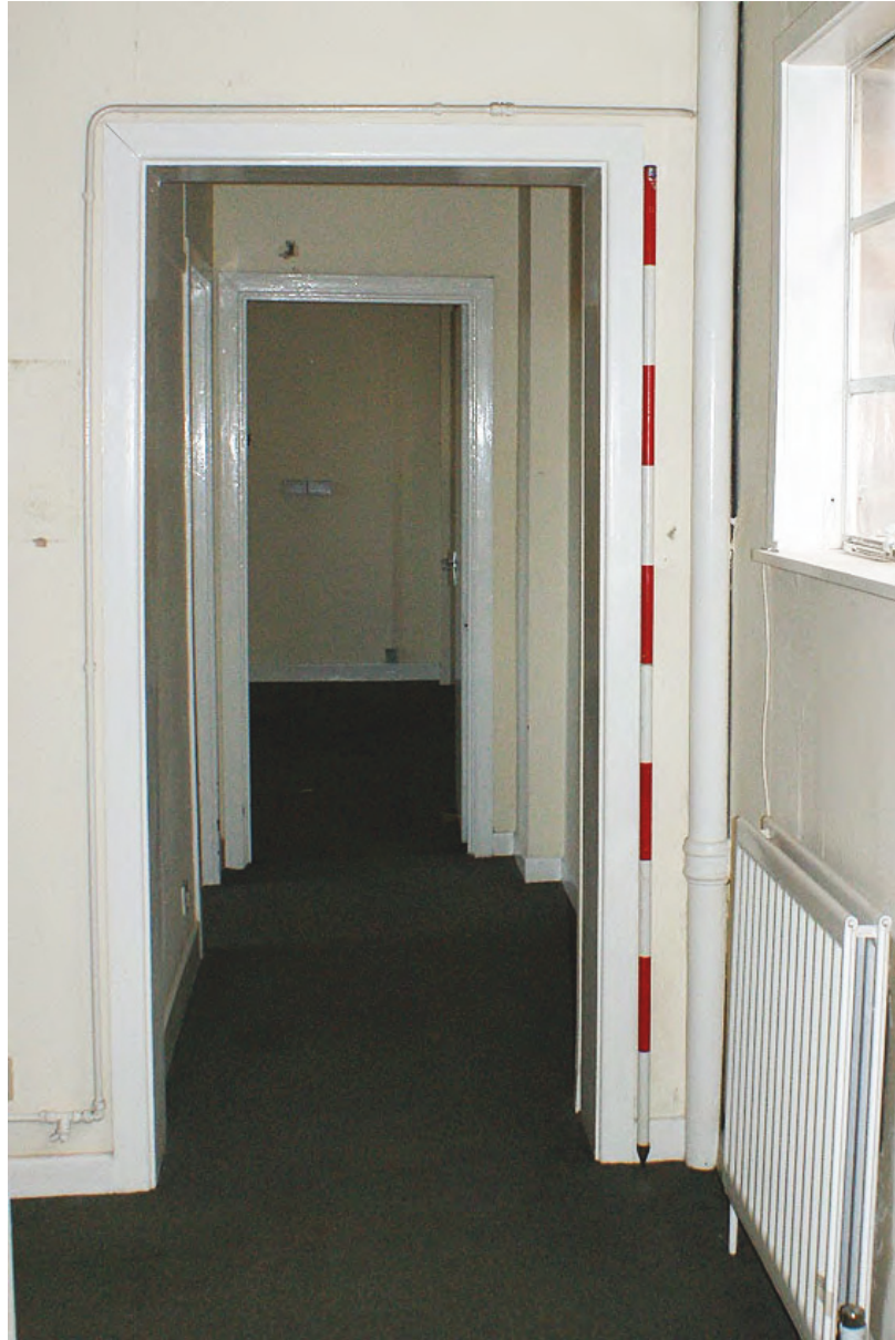
Plate 150: 1980s passage space
