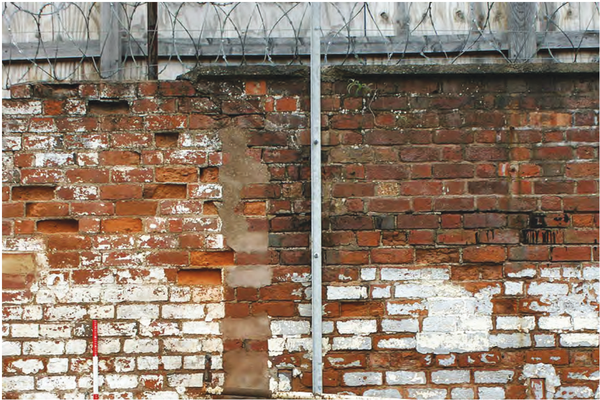
Plate 66: Roofline of former structure on wall section 5
