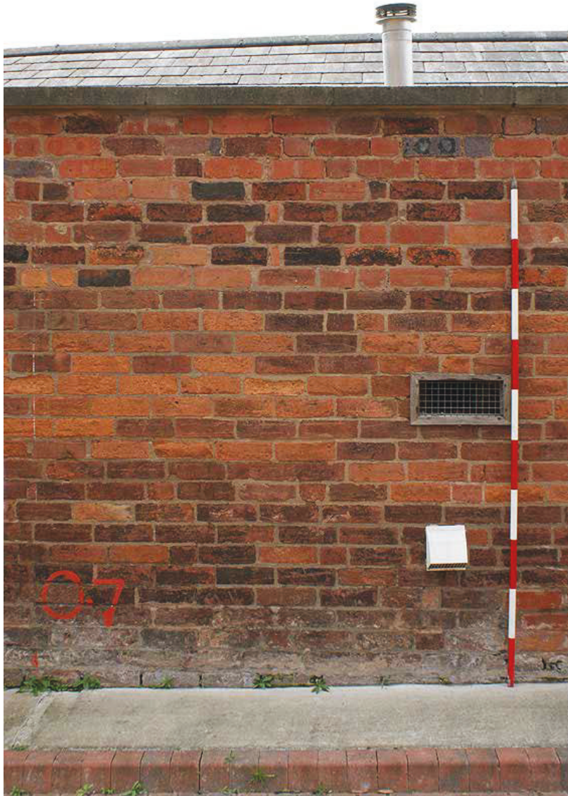
Plate 52: Three phases of brickwork of Netherton Lane wall
