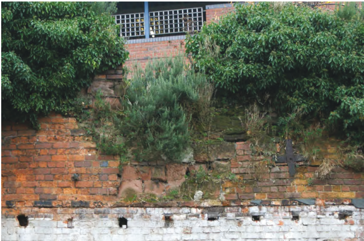
Plate 33: Stonework at top of the city wall
