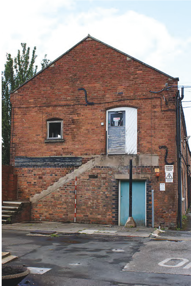
Plate 164: South elevation of sawmill building from south
