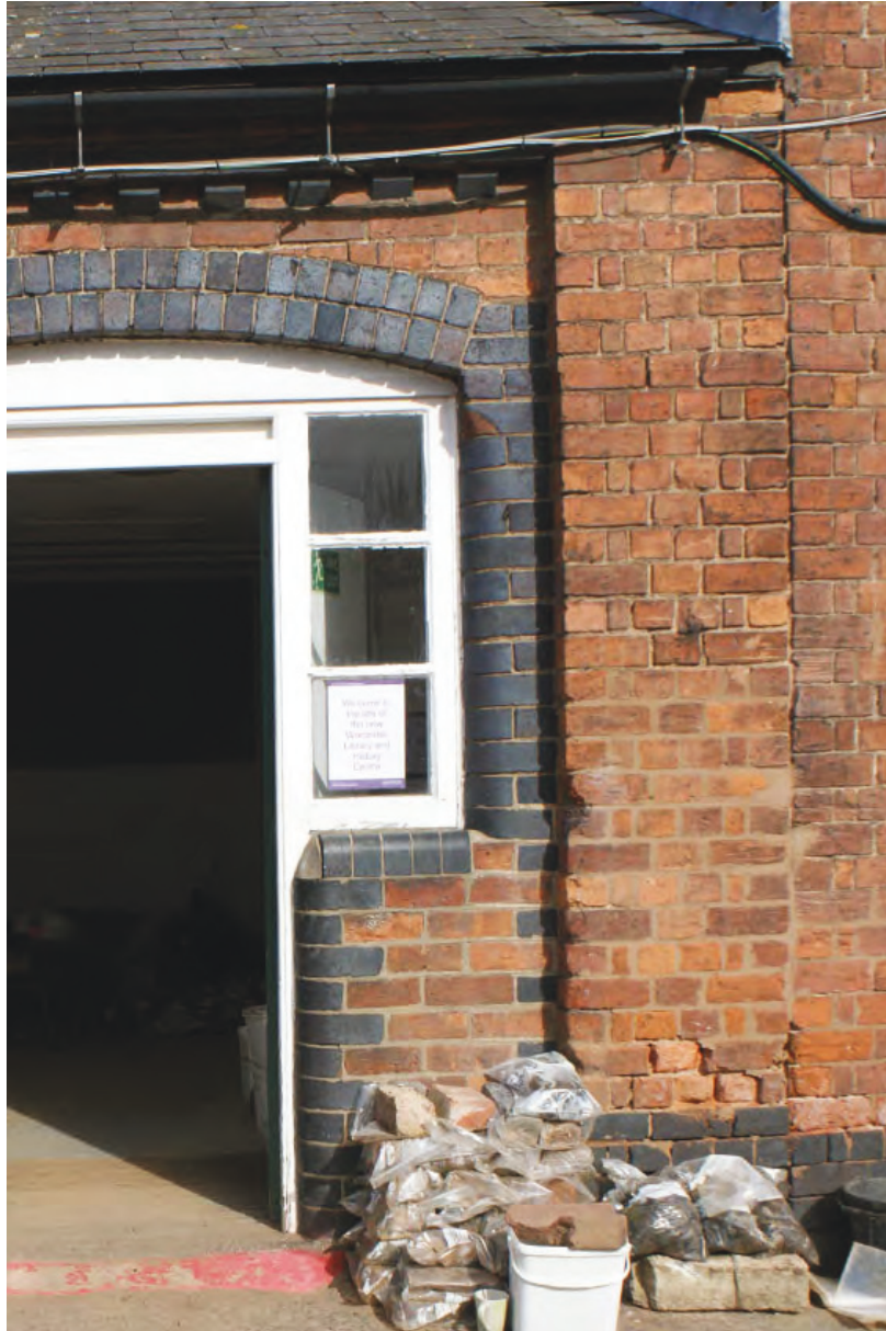
Plate 140: Building break between middle and rear sections
