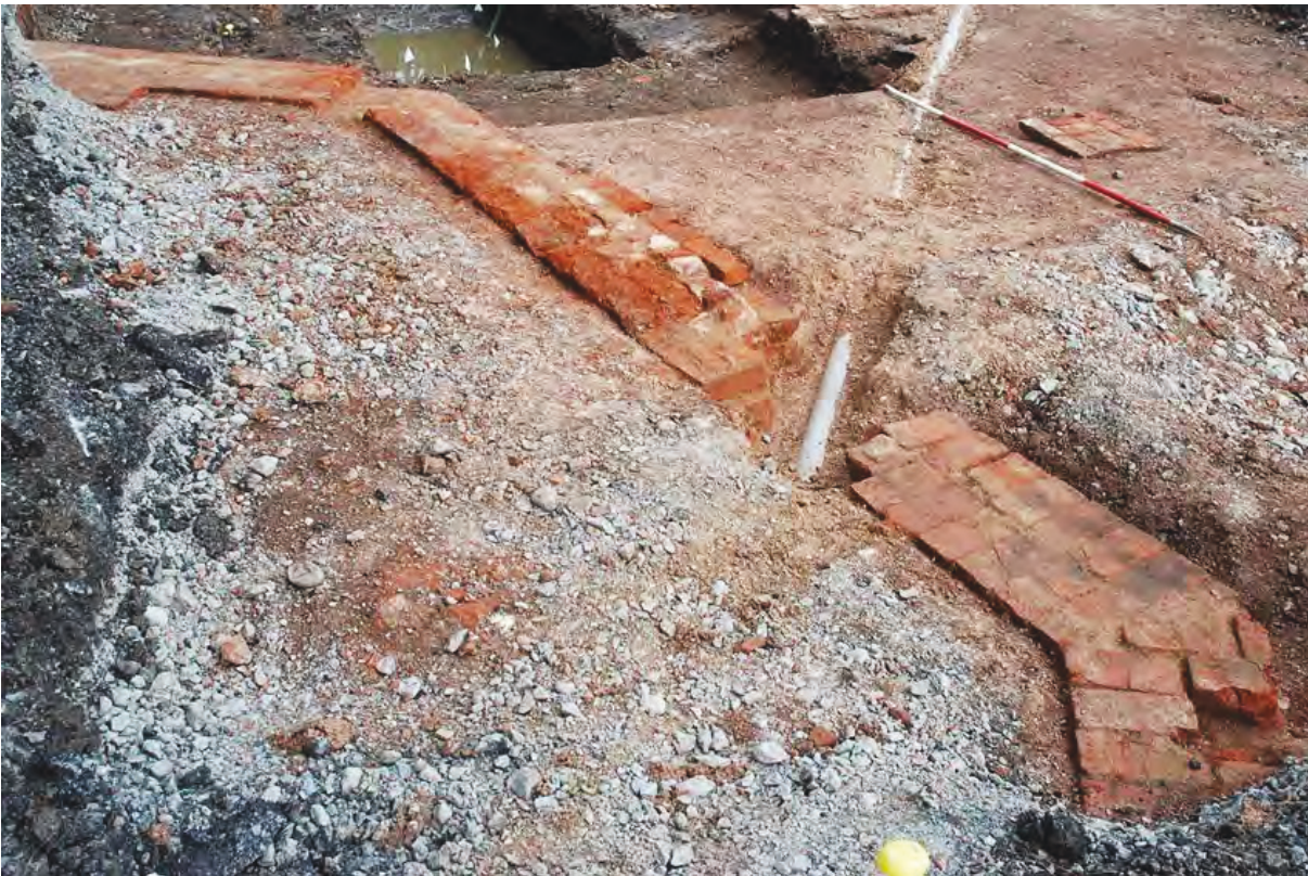
Plate 38: Foundations of octagonal cattle market counting house
