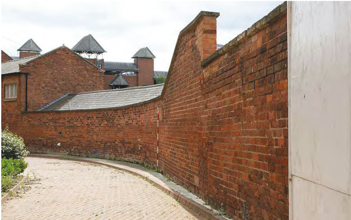
Plate 51: Netherton Lane boundary wall from the north
