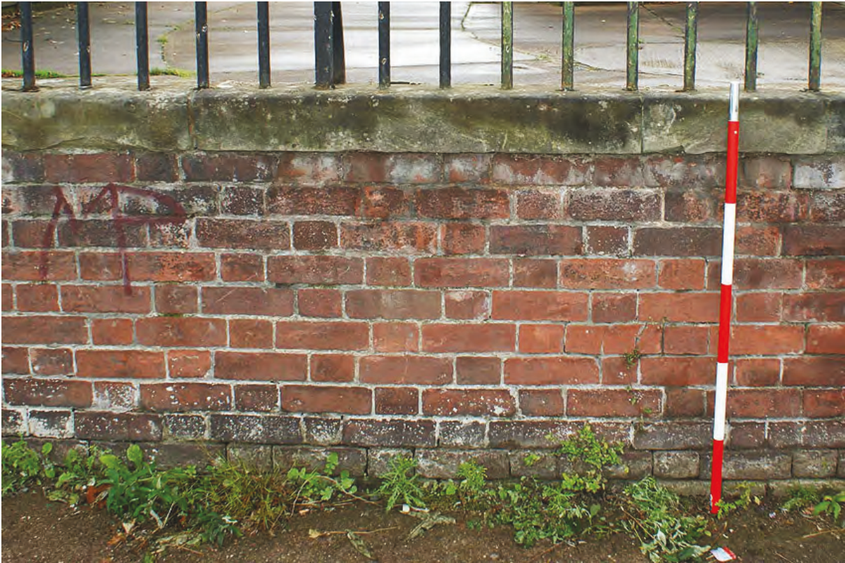
Plate 72: Coomber's boundary wall brickwork and sandstone top
