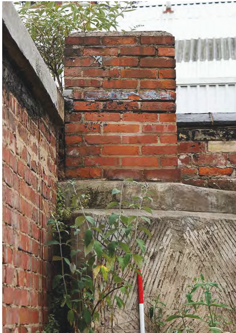
Plate 87: Chimney from demolished structure to west of air raid shelter
