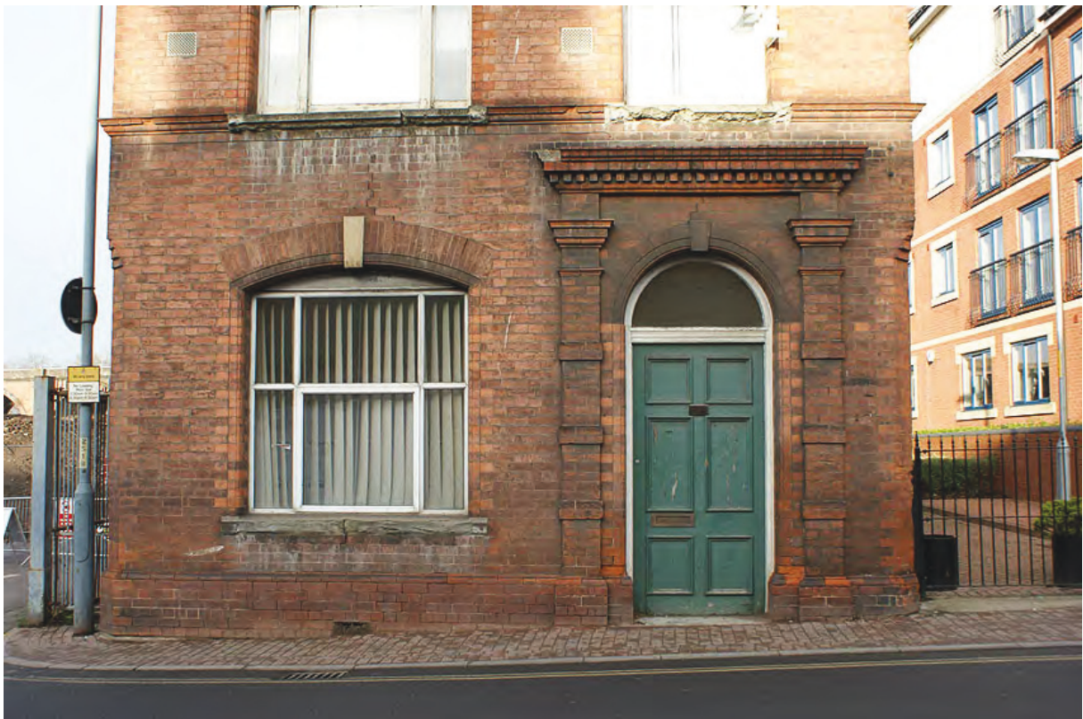
Plate 105: Ground floor, south elevation of the 'office building' fronting The Butts, showing door surround, window surround and string course
