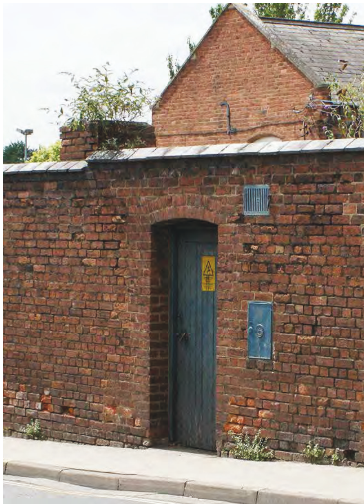
Plate 82: Entrance to air raid shelter on The Butts
