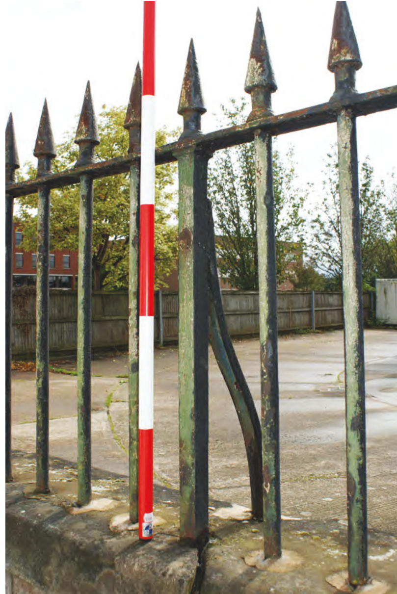
Plate 74: Square post and bracket of railings
