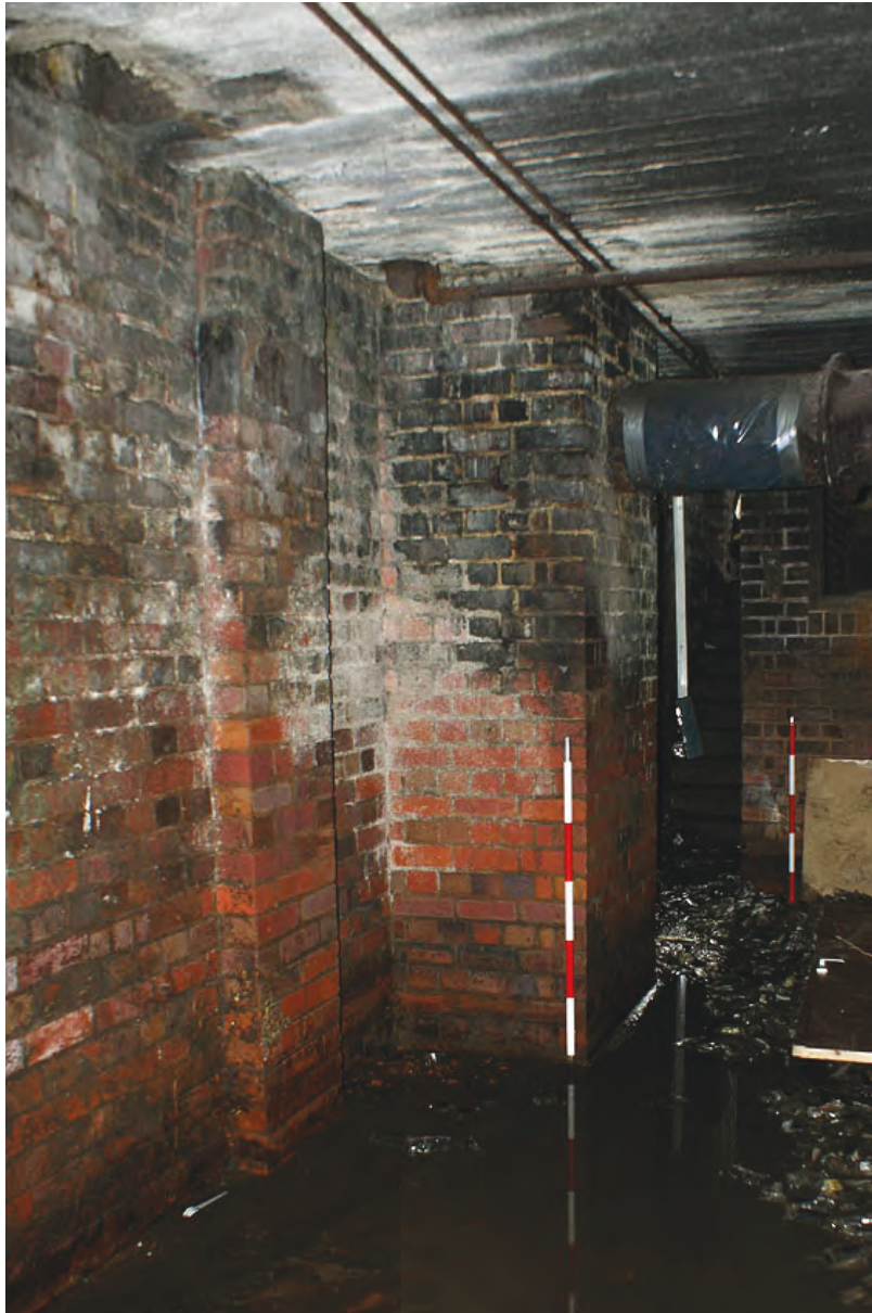
Plate 11: Base of chimney stack from the south
