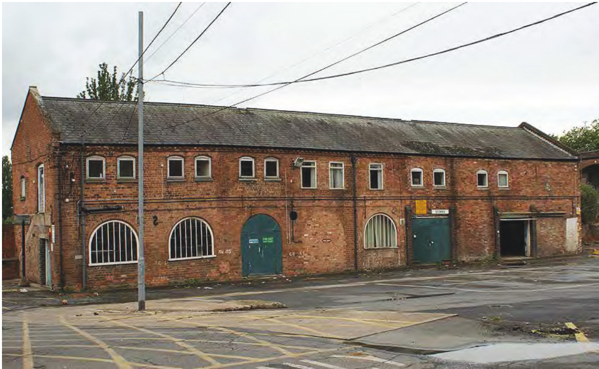
Plate 162: Sawmill building from the south-east, east elevation from the depot
