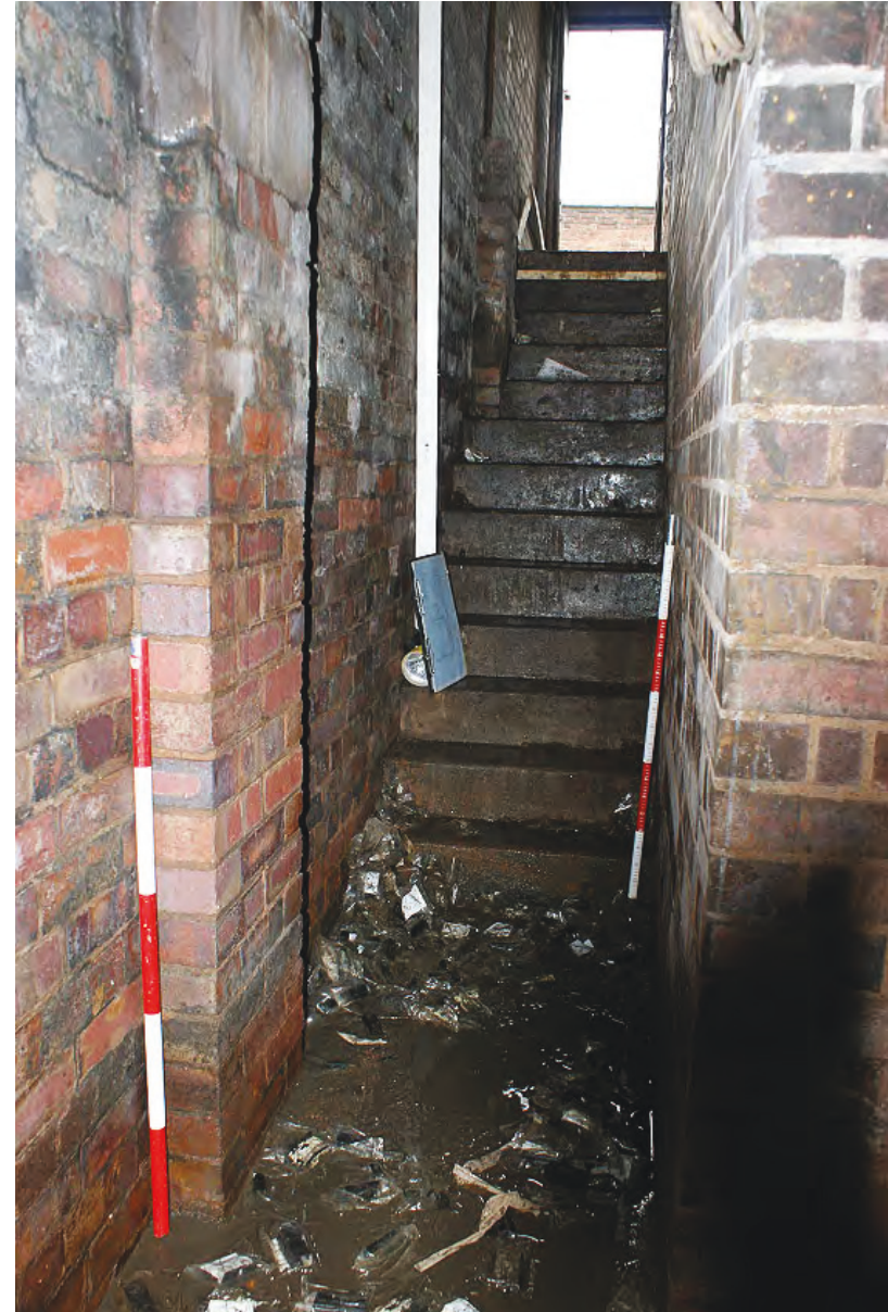
Plate 10: Corridor and stairs into cellar
