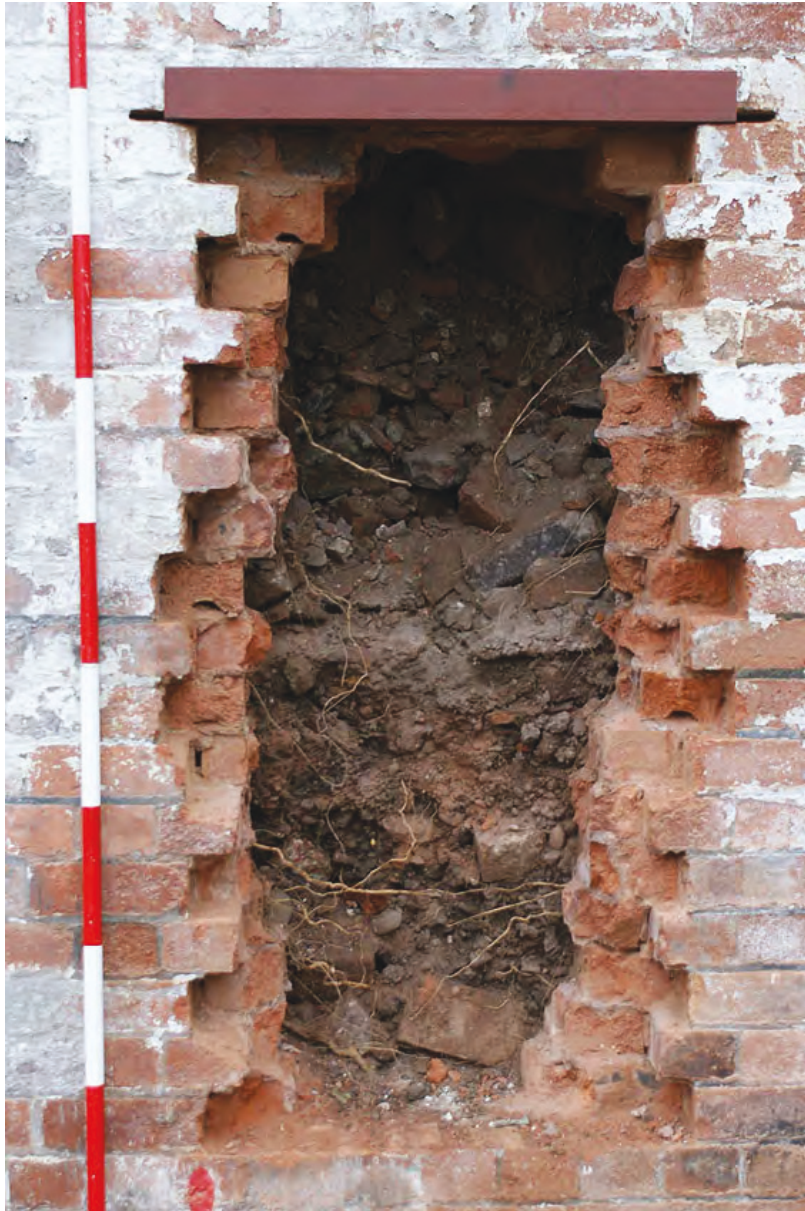
Plate 36: West side hole cut into city wall
