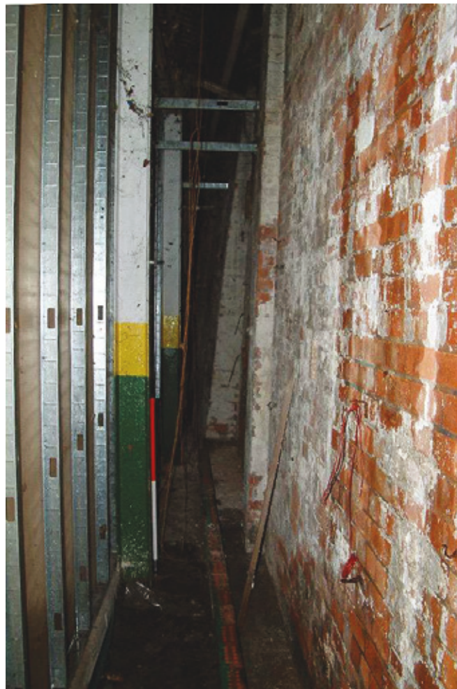
Plate 6 Transwipers interior stanchion structure from thh west
