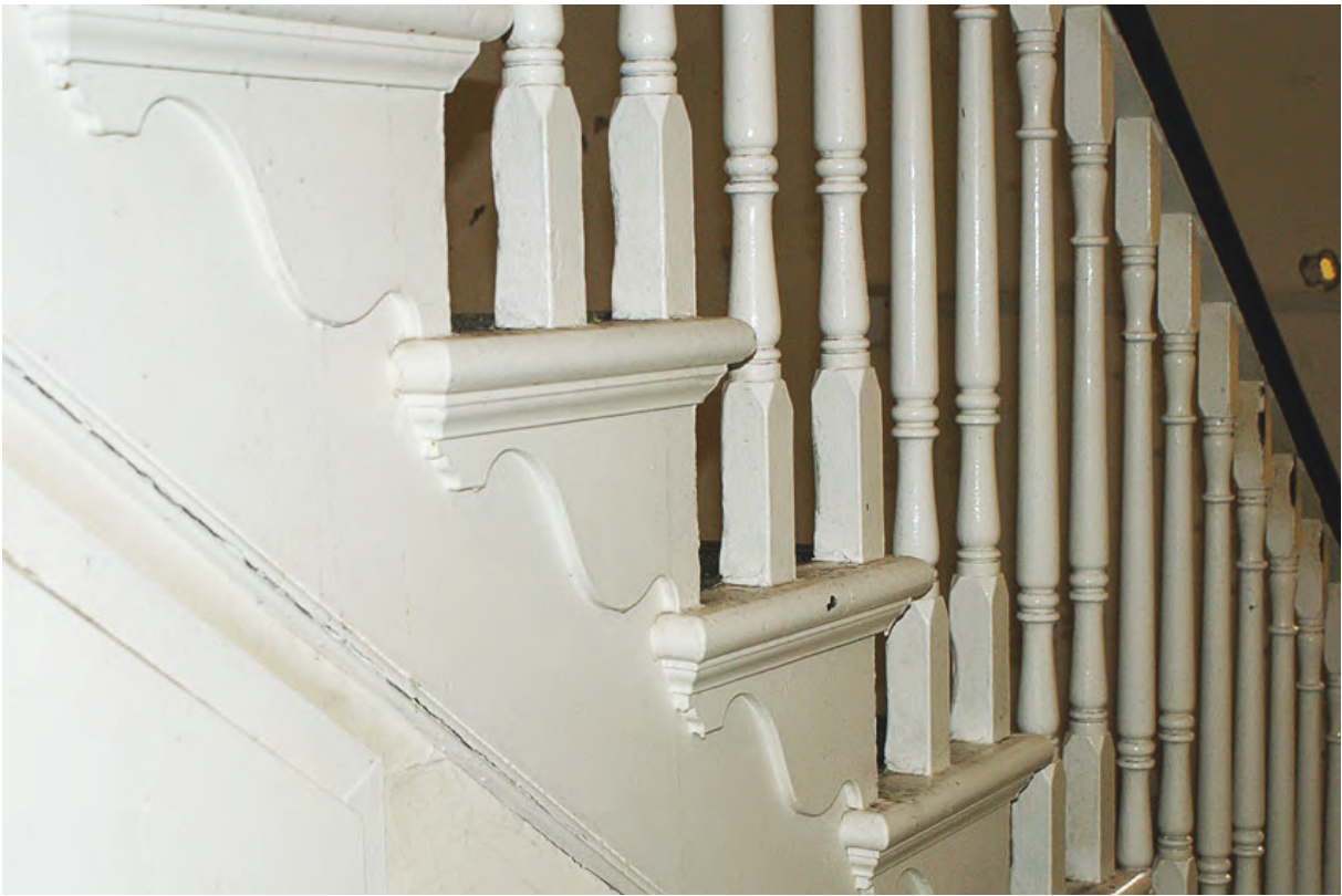
Plate 118: Open string with decorated scroll type brackets
