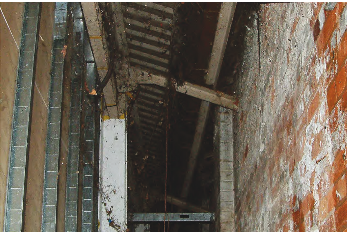
Plate 8: Transwipers interior roof structure tied into city wall from the west
