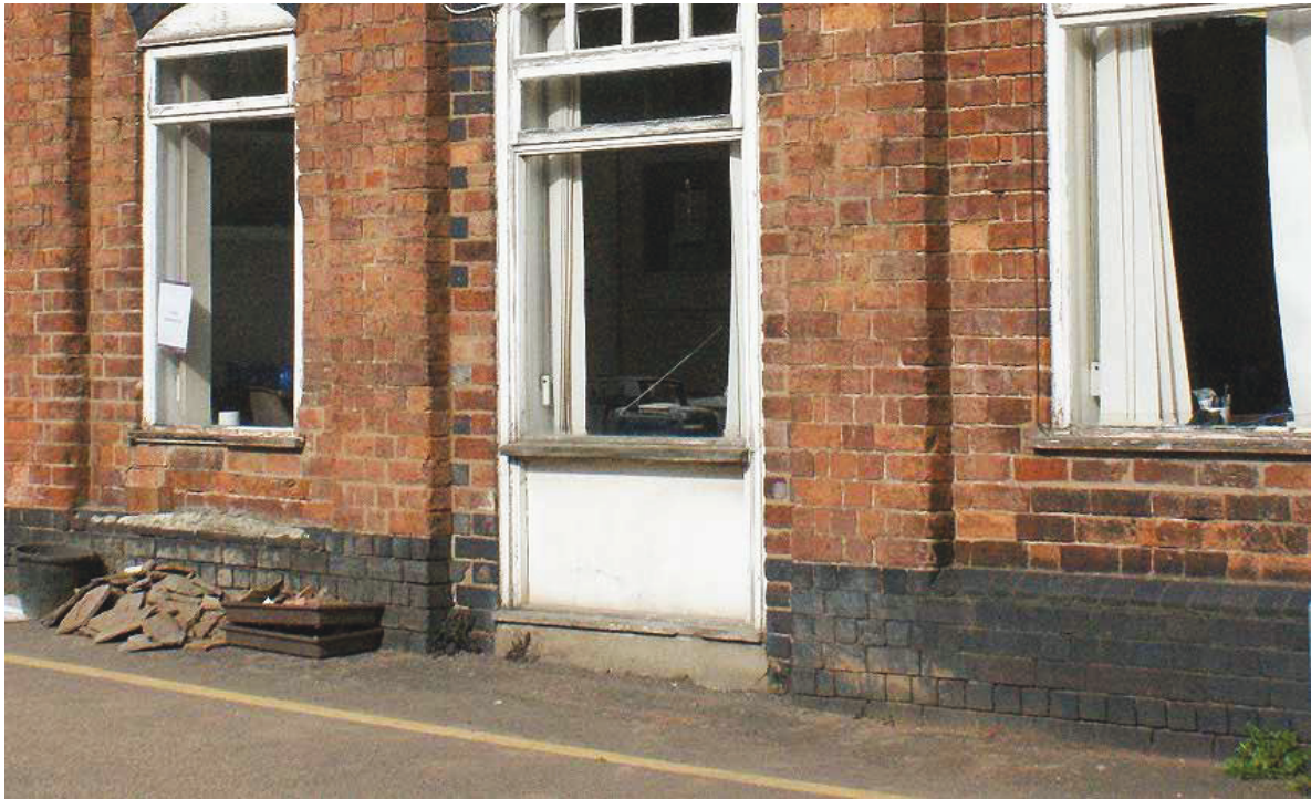
Plate 102: Plinth of two-storey range
