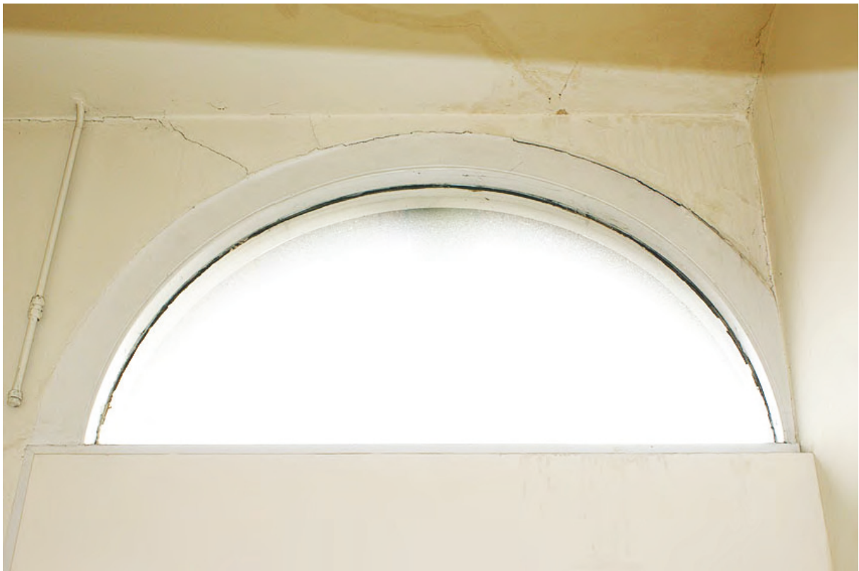
Plate 113: Plain fanlight above front door, Room G5
