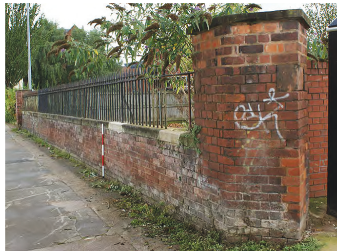
View south along Croft Walk
