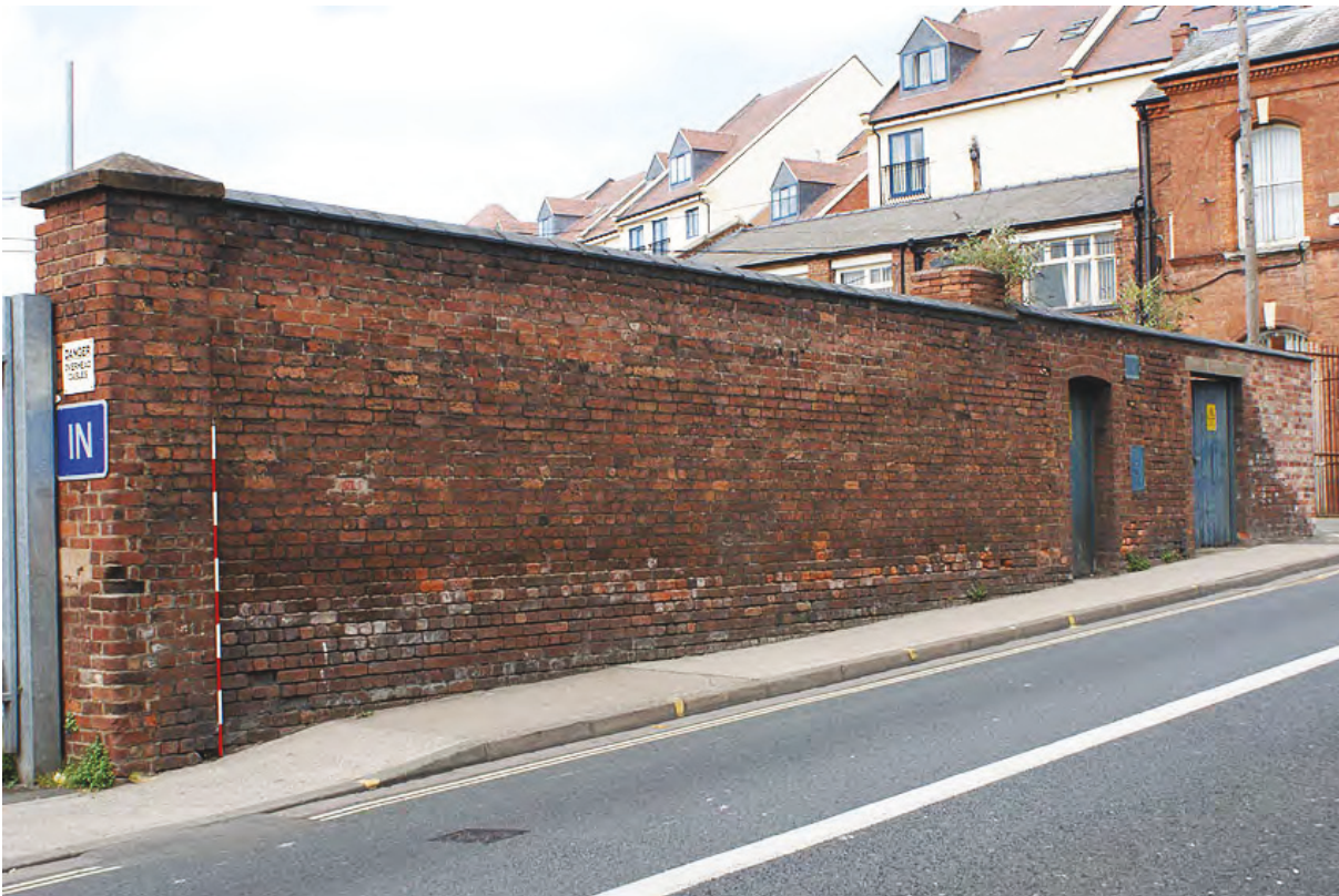
Plate 41: The Butts boundary wall to the former City Council depot from the south-west
