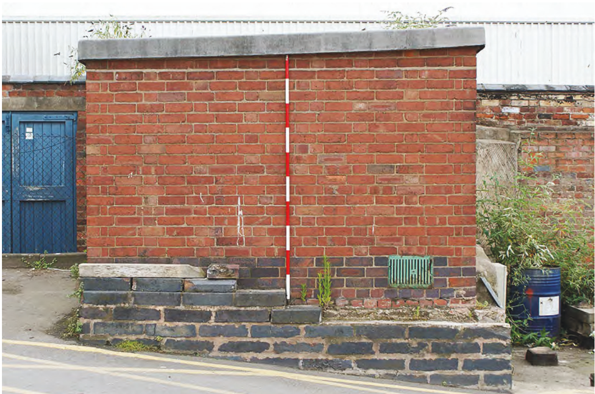
Plate 80: North elevation of air raid shelter
