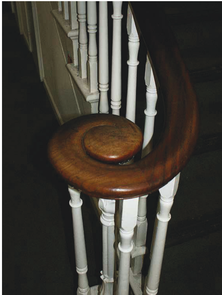
Plate 136: Gently curved flat top stair handrail
