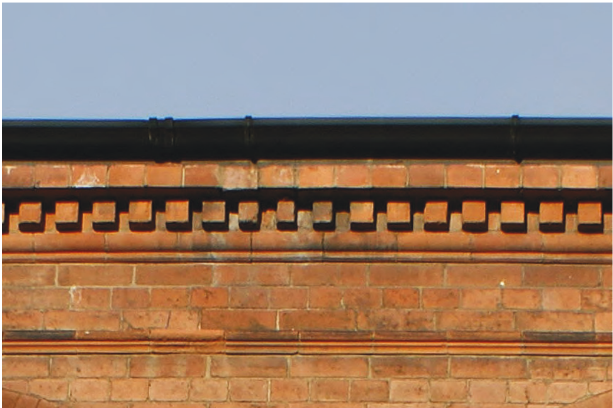
Plate 99: Moulded terracotta and brick eaves cornice
