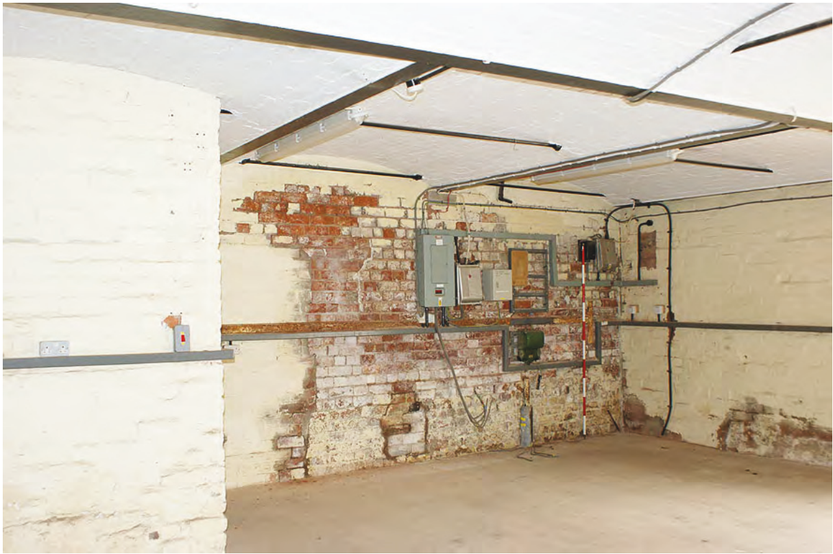
Plate 172: Vaulted ceiling of ground floor of sawmill building
