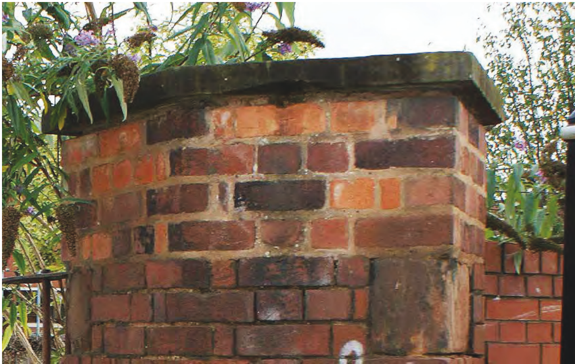
Plate 77: Modern bricks at top of north pier of Coomber's Wall
