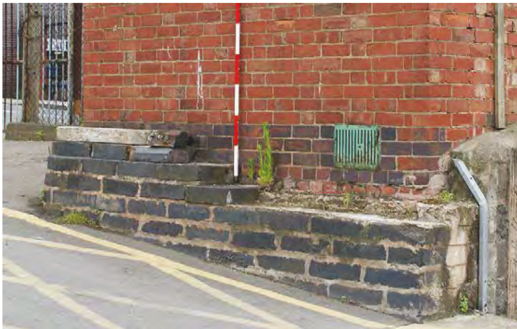
Plate 88: Low level wall constructed of engineering brick
