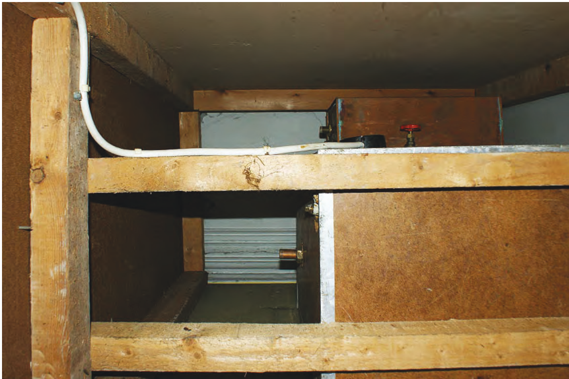
Plate 120: Looking up to ceiling showing surviving cornice, Room F3 cupboard
