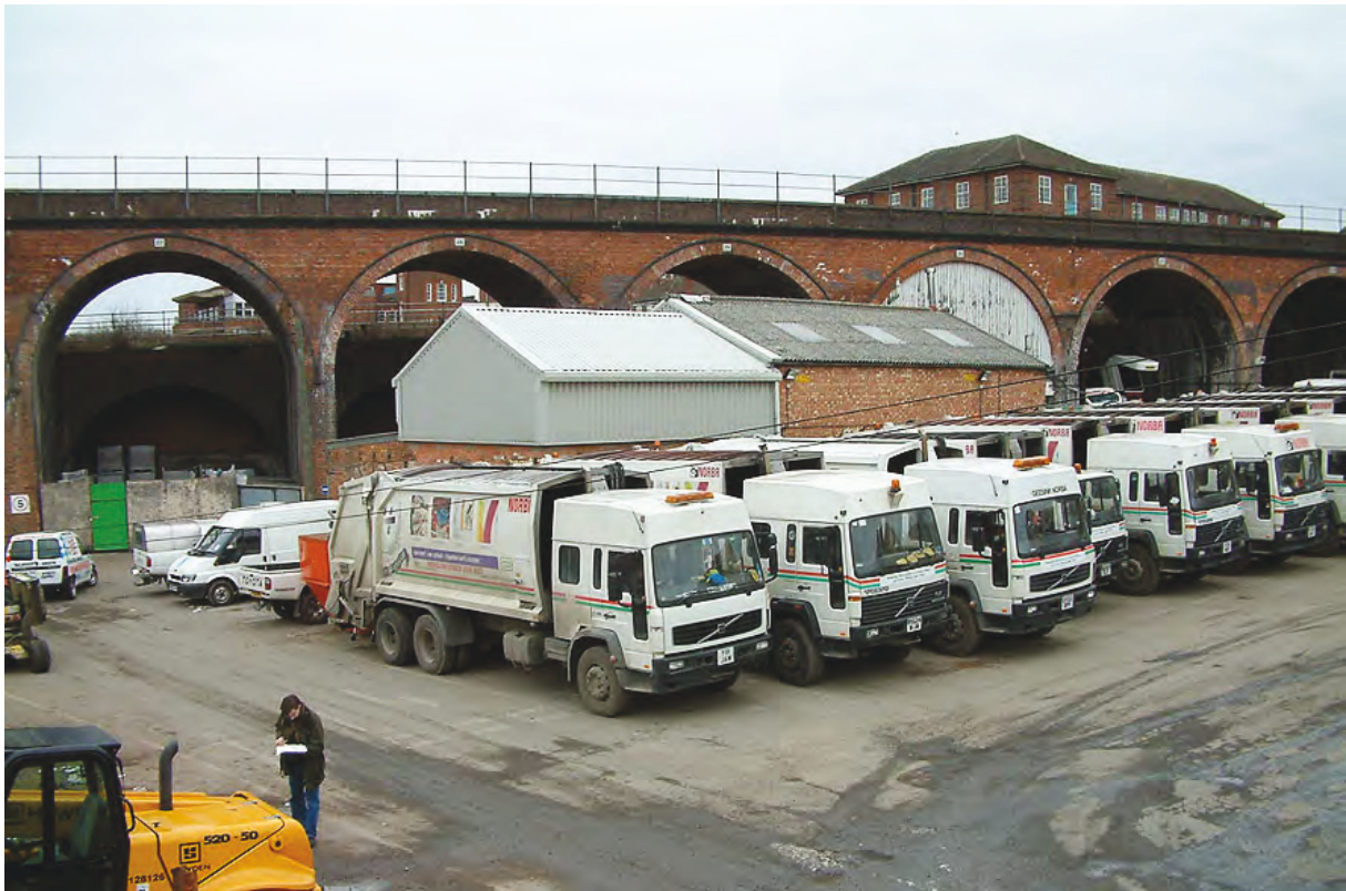
Plate 193: Railway viaduct running across the site, west to the left
