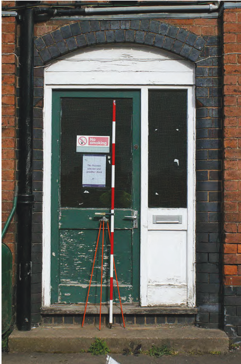
Plate 100: Blue brick door surround of two-storey range
