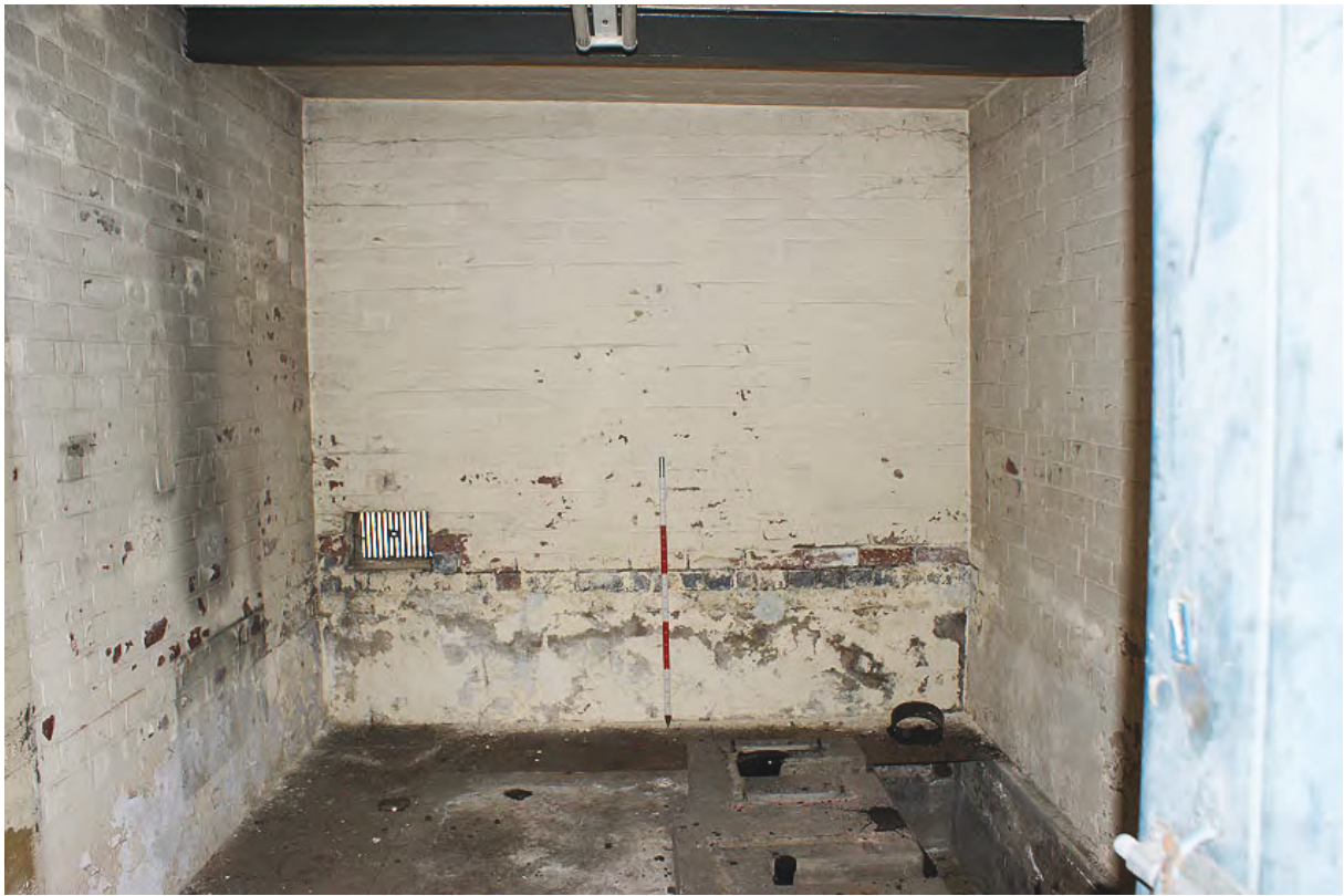
Plate 89: Interior of air raid shelter
