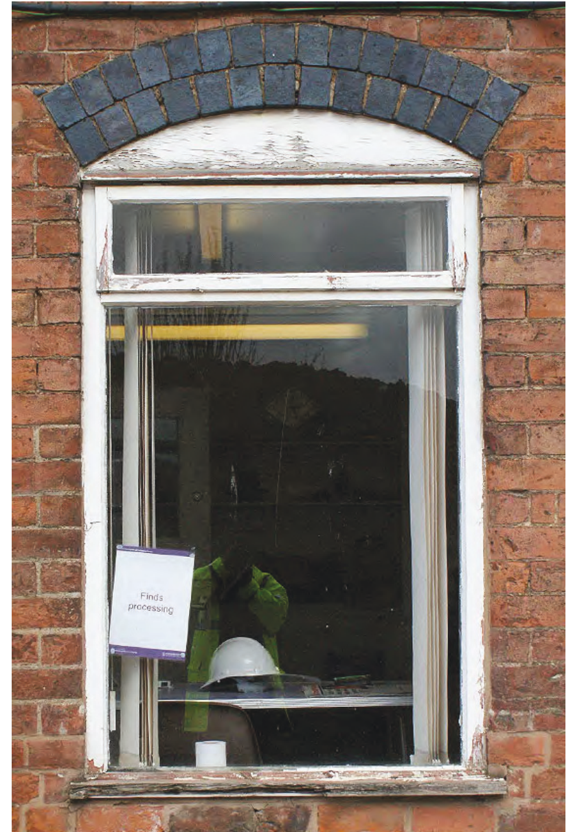
Plate 101: Blue brick window arch on two-storey range
