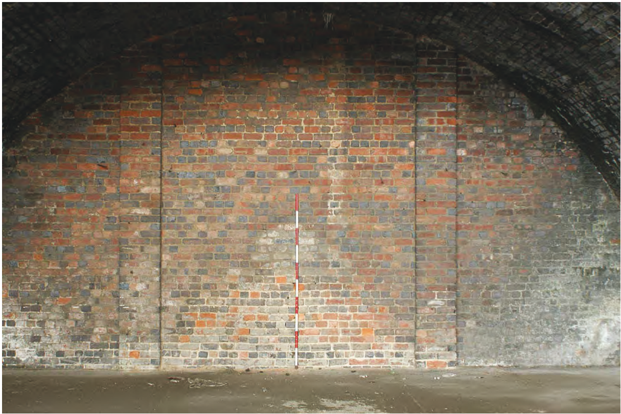
Plate 202: Blocking of The Butts siding arch
