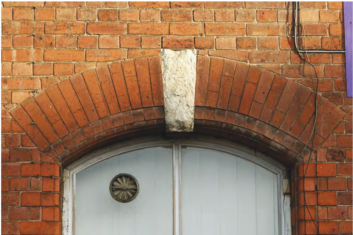
Plate 96: Example of window arches showing decorated brickwork and limestone keystone
