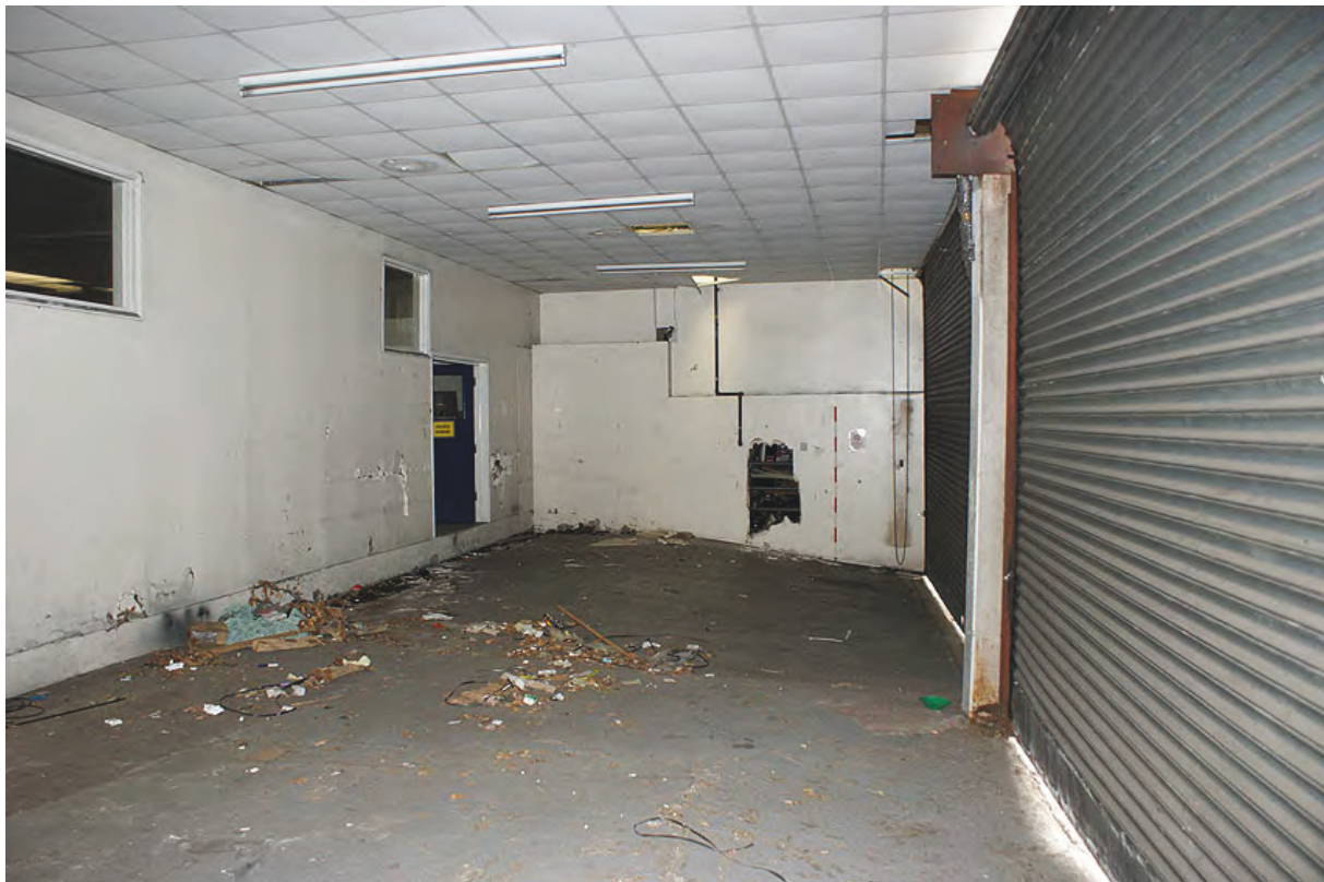
Plate 27: Interior, roadside, space of Transwipers from the east
