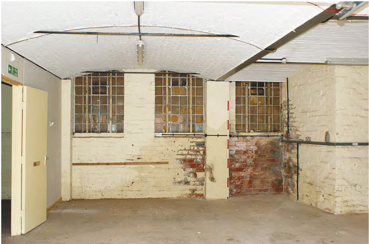
Plate 169: Interior ground floor of sawmill building from the east
