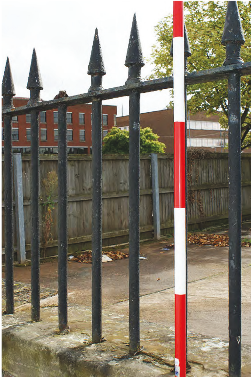
Plate 73: Tubular railing posts and spiked tops
