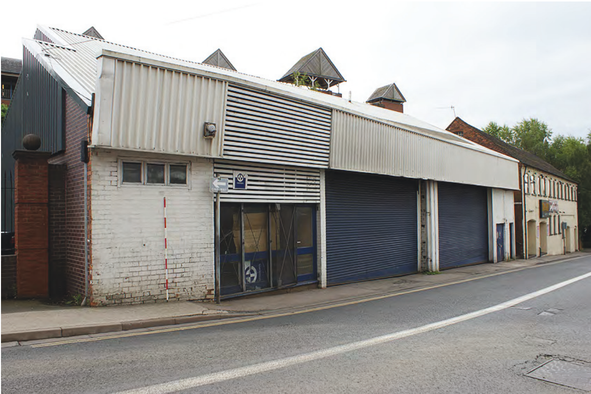
Plate 2: Transwipers building from the north-east
