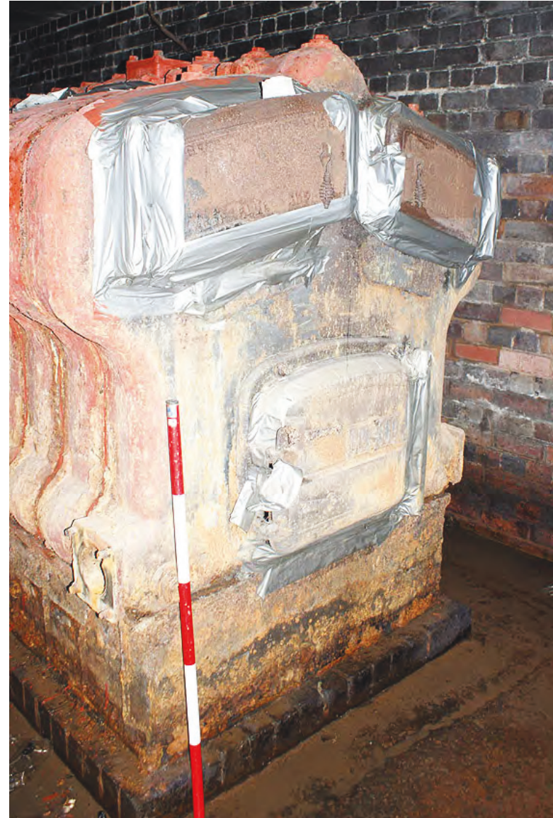
Plate 14: Cast iron boiler with Transwipers cellar, from the south
