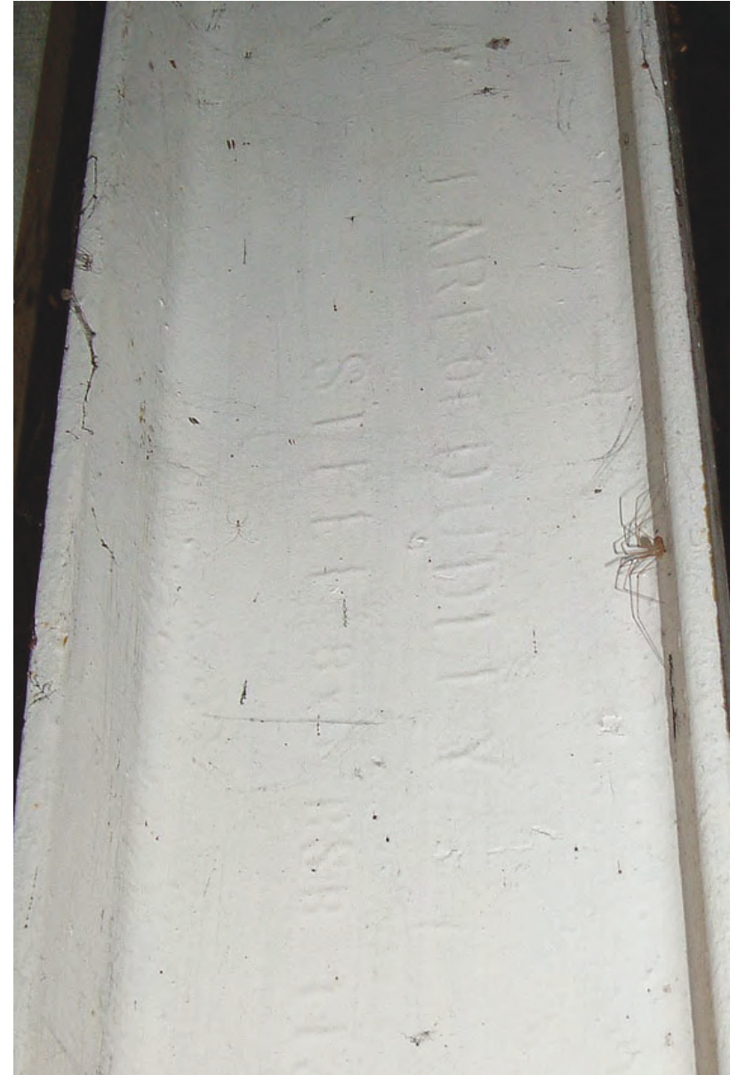
Plate 23 Earl of Dudley Steel stanchion
