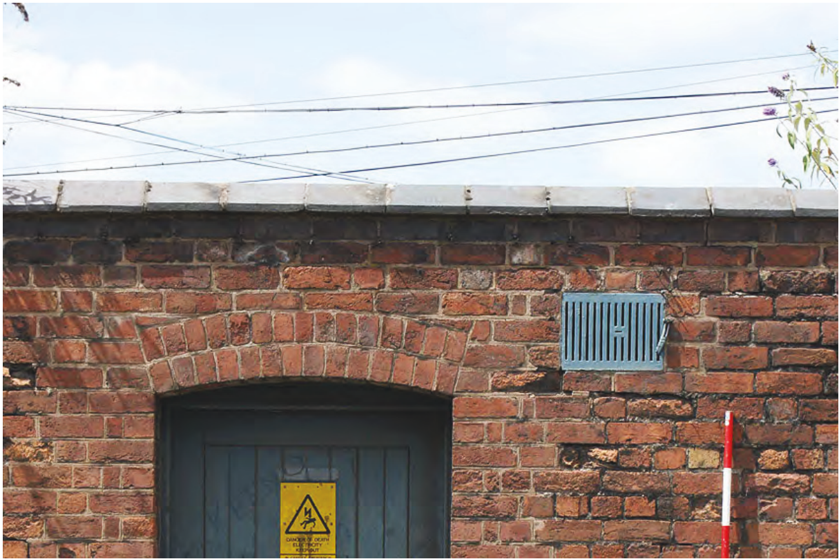
Plate 83: Air vent at top of wall of air raid shelter
