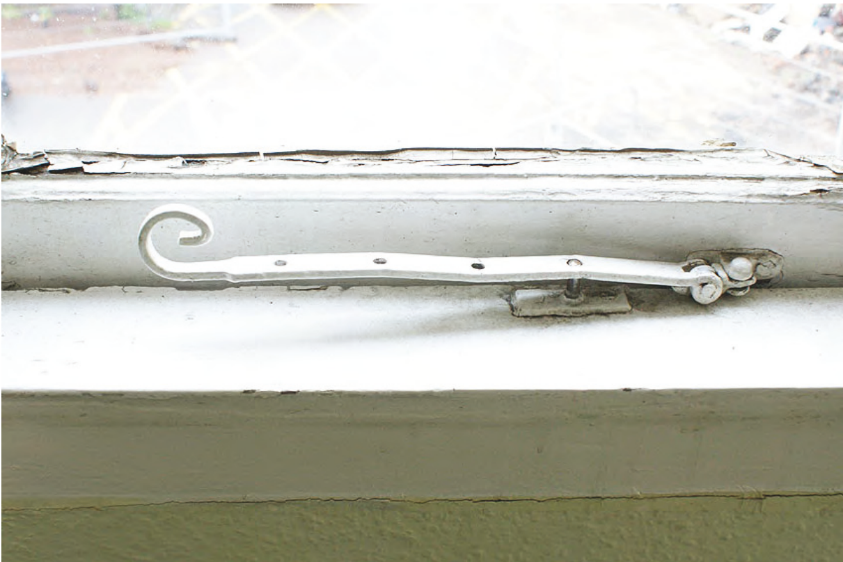
Plate 135: Spiral window stay and handle
