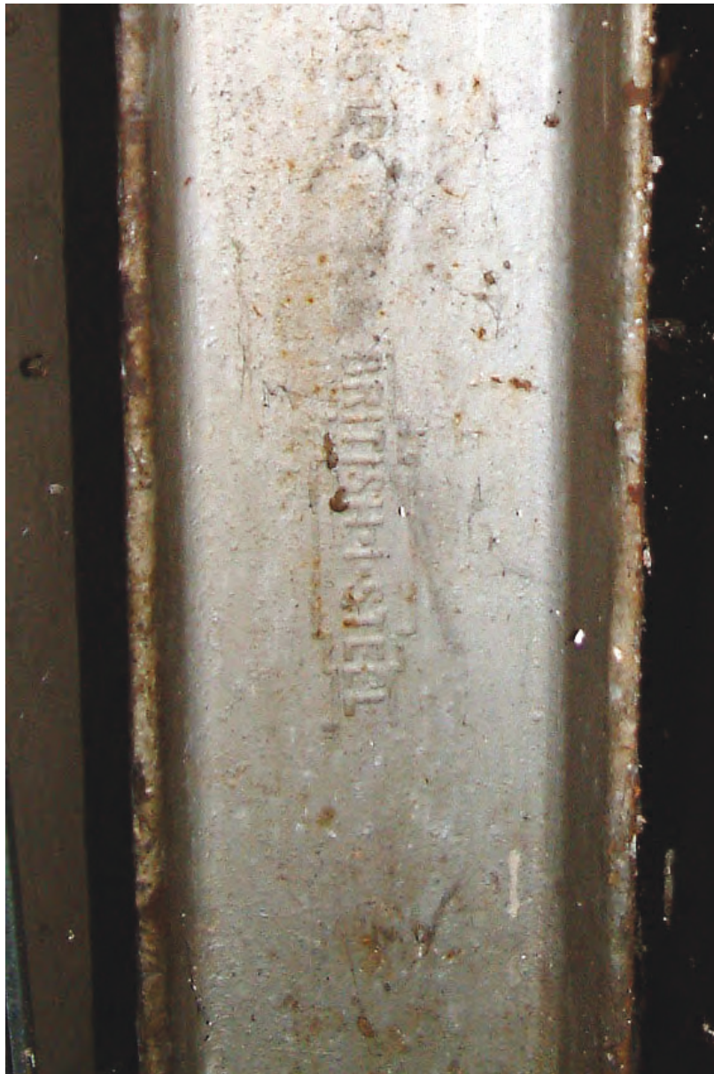
Plate 25: British Steel stanchion
