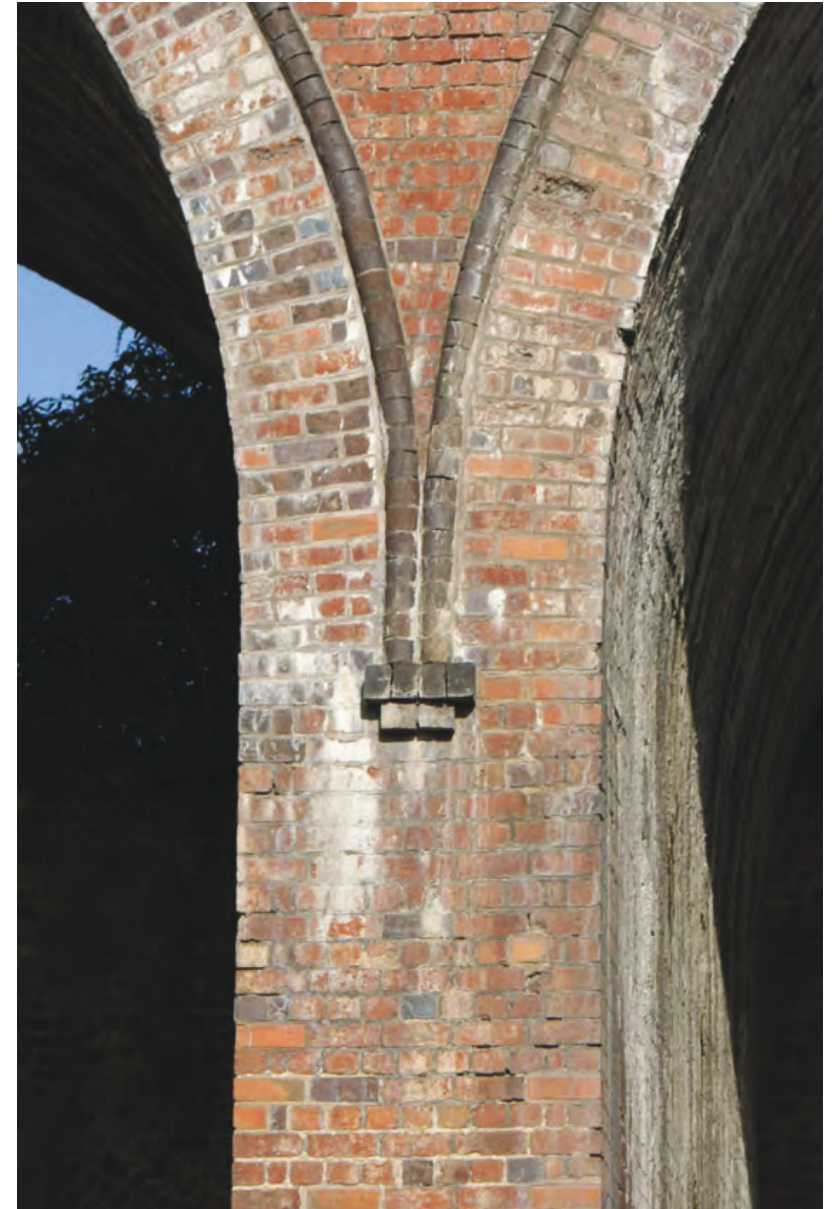
Plate 196: Viaduct arch hoodmould and stop of brick
