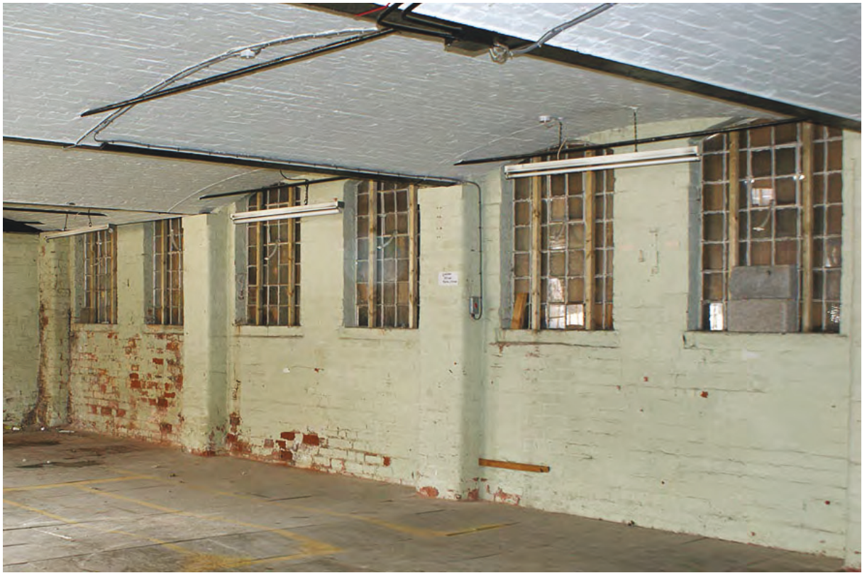
Plate 170: Interior ground floor of sawmill building showing windows of west elevation
