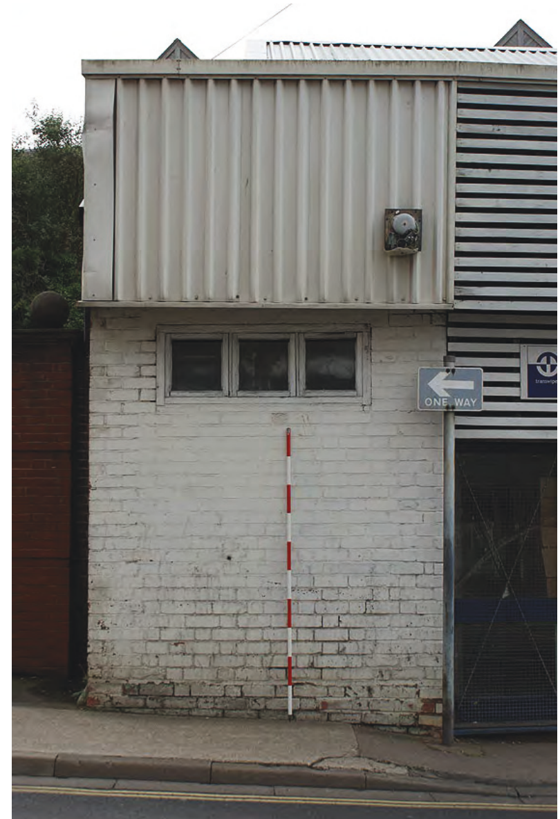
Plate 21: 19 th century brickwork on The Butts elevation, from the north
