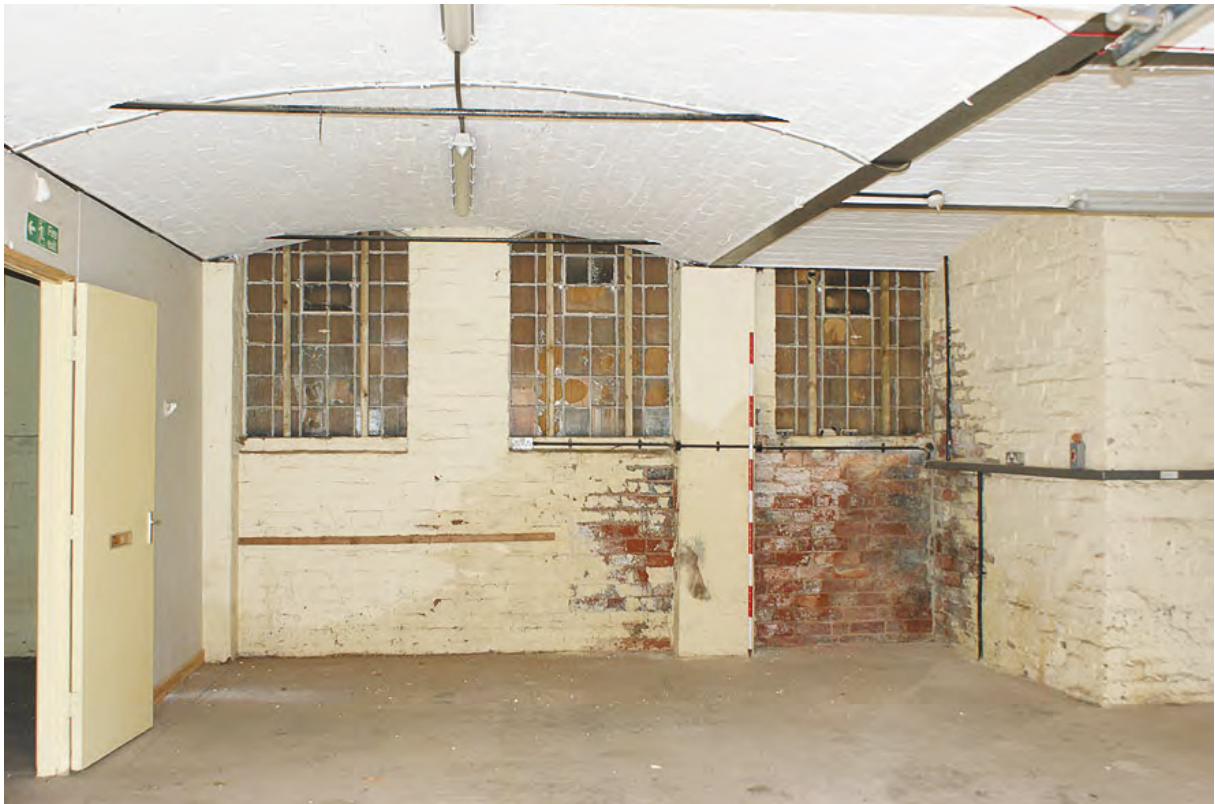
Plate 171: Vaulted ceiling of ground floor of sawmill building
