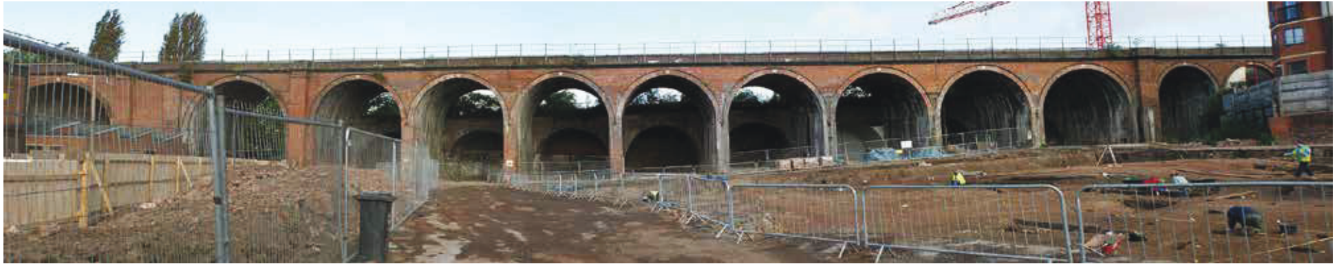
Plate 194: Viaduct arches 25 to 33 during excavation
