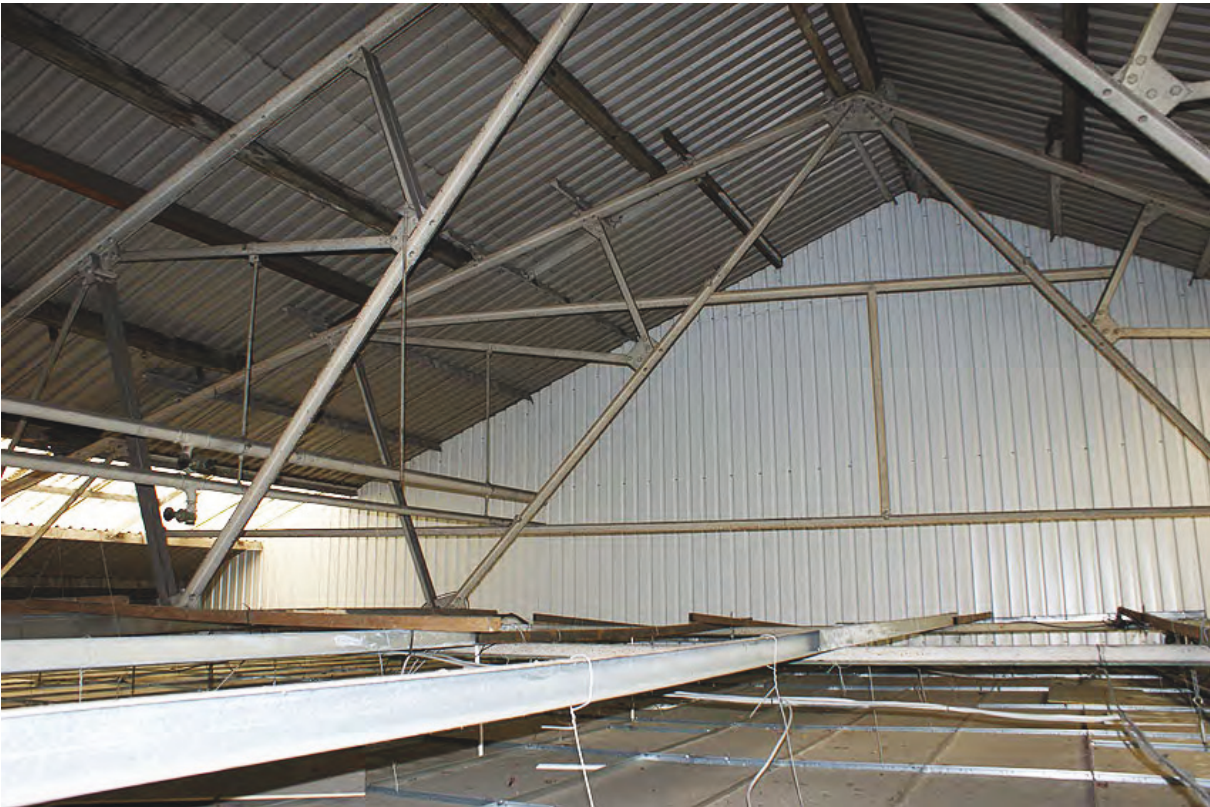
Plate 7: Transwipers interior roof structure building from the east
