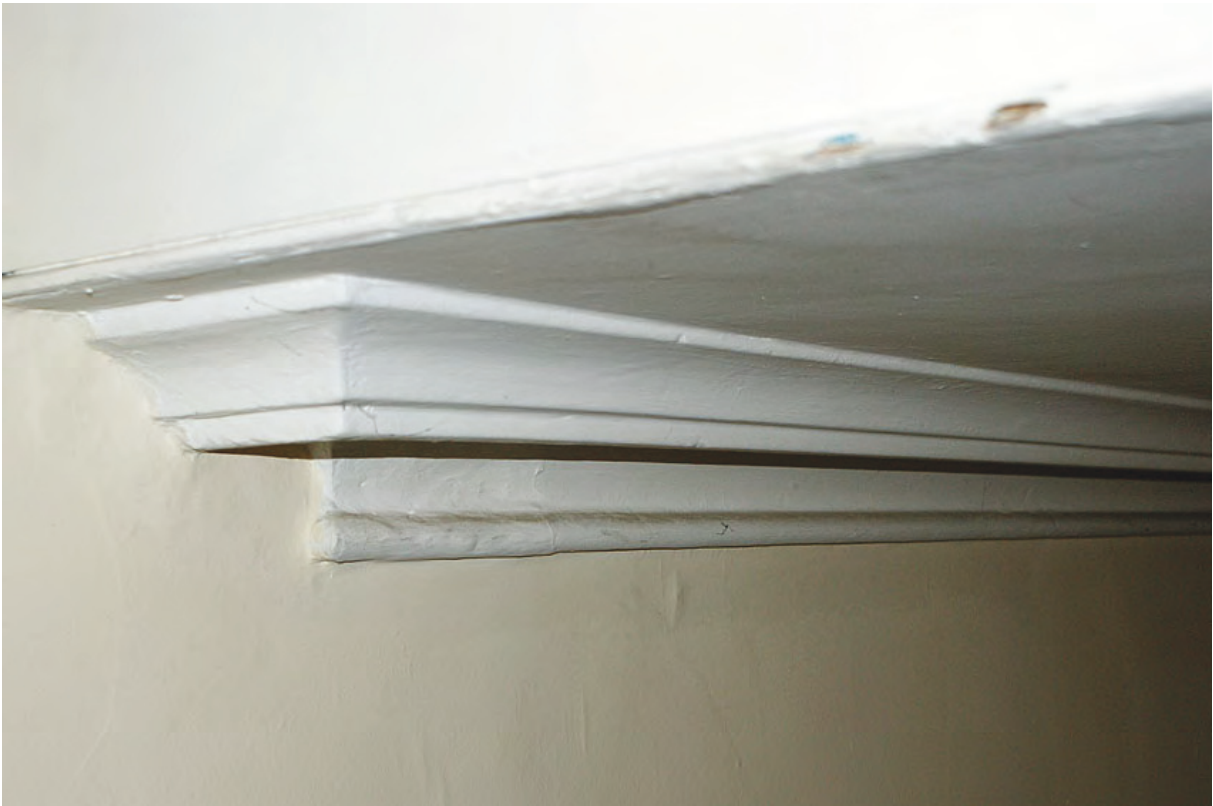
Plate 119: Example of plaster moulded cornice on staircase
