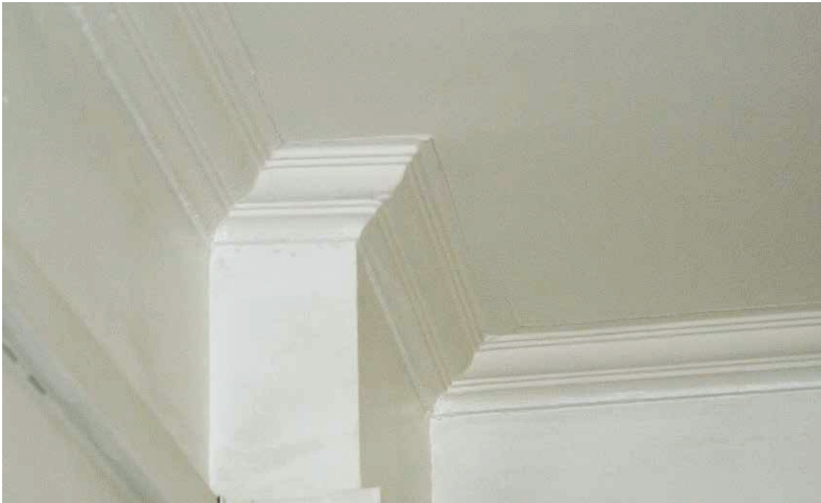
Plate 137: Example of moulded plaster cornice in two-storey range, Room G6
