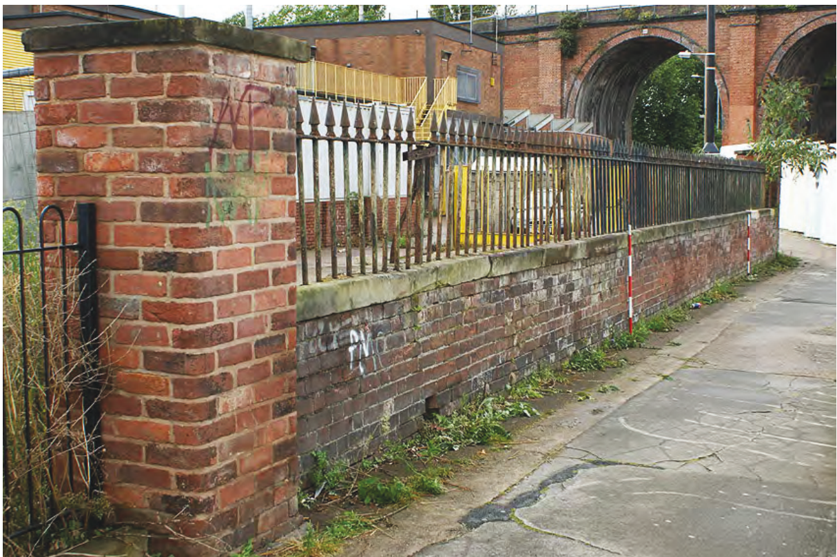
Plate 71: Coomber's boundary wall from the south
