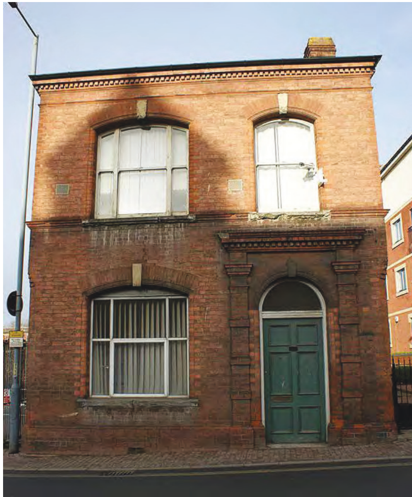
Plate 91: The Butts frontage of the Joseph Wood office building
