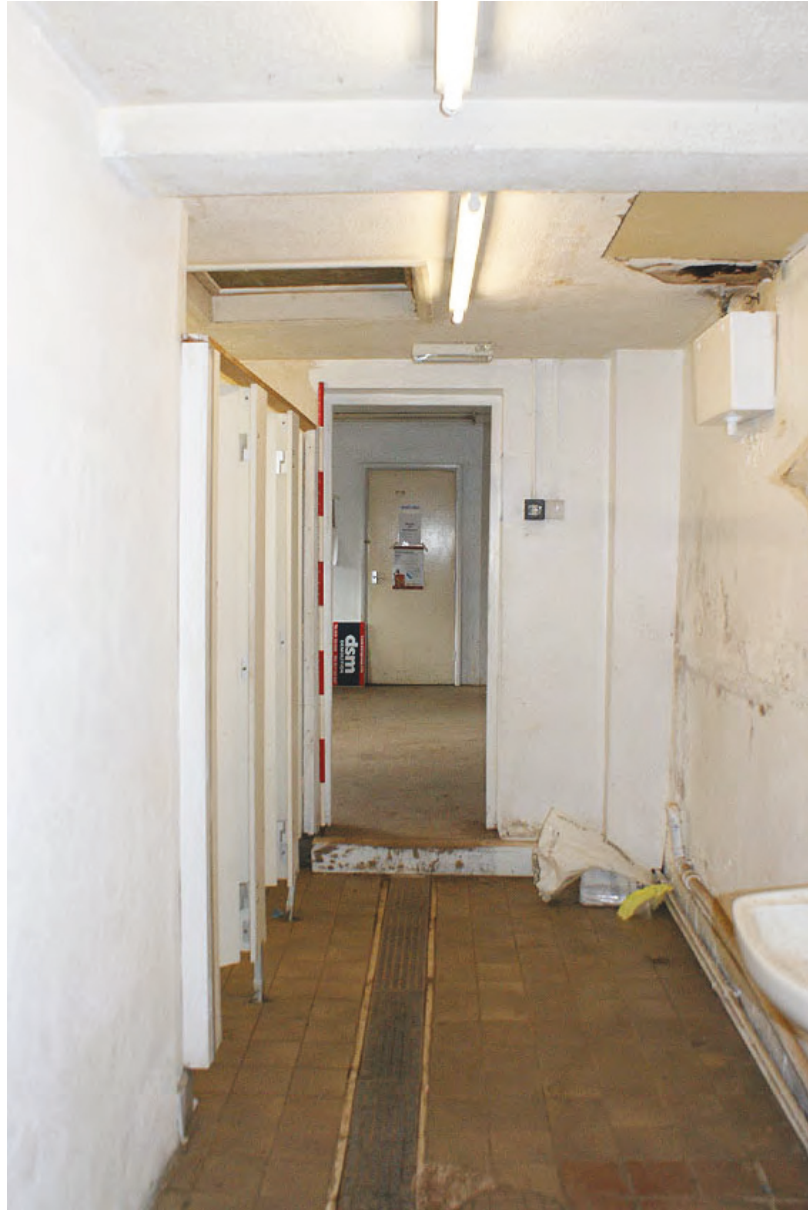
Plate 144: 1970s toilet area
