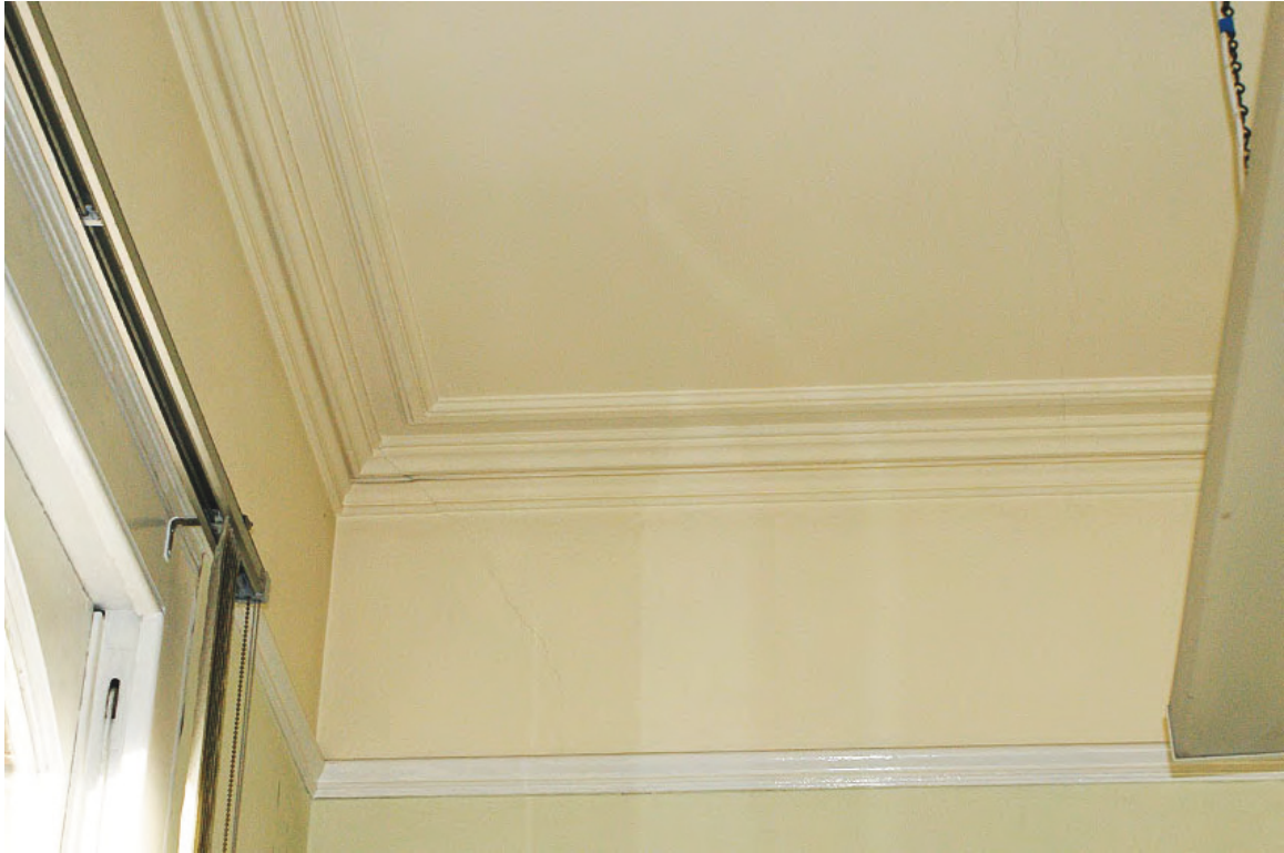
Plate 124: Cornice and picture rail in building fronting The Butts
