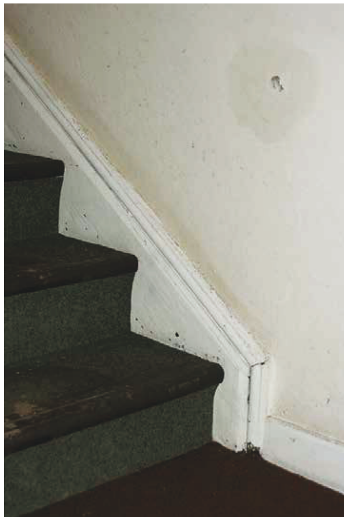
Plate 116: Roll beaded skirting on staircase
