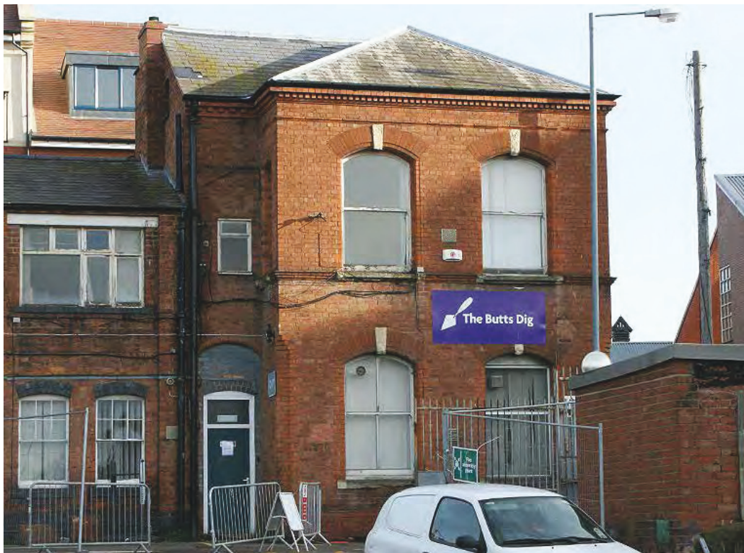
Plate 92: Depot (west) elevation of Joseph Wood office building
