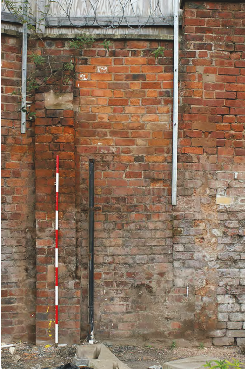
Plate 60: Wall section 4, blocked gateway
