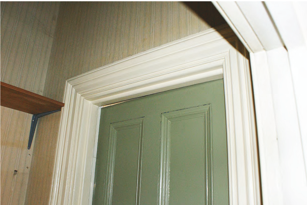
Plate 127: Surviving bolection moulded door surround, Room F4a
