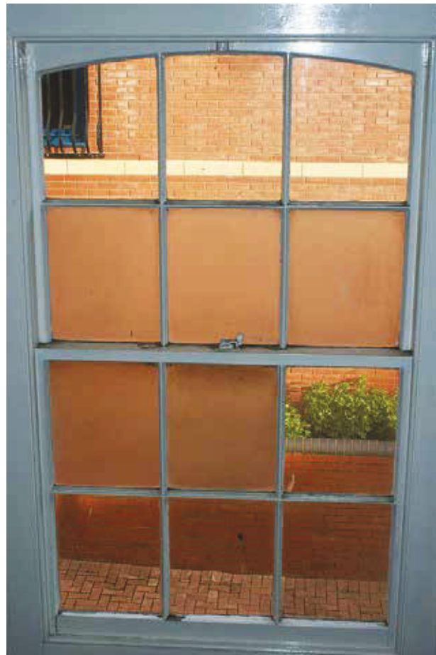
Plate 125: Staircase window, Room F3
