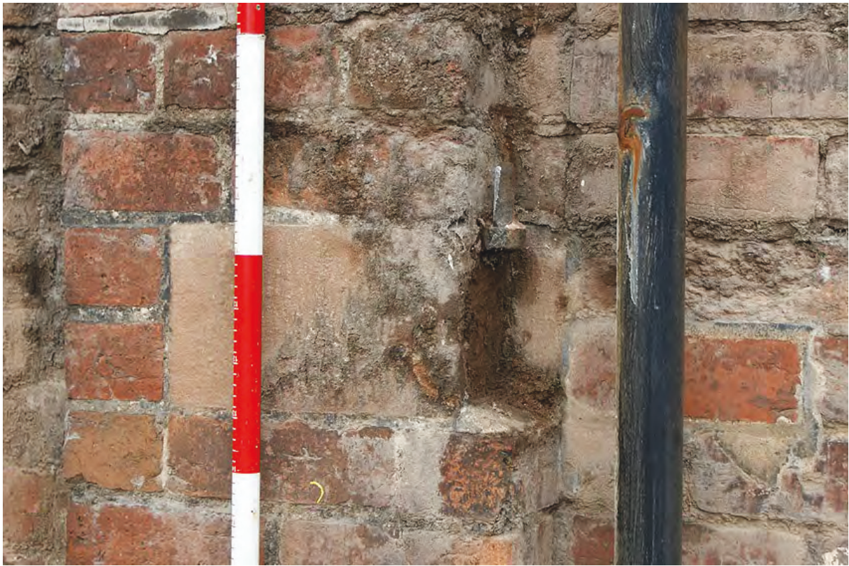
Plate 61: Hook for holding hinges of a gate
