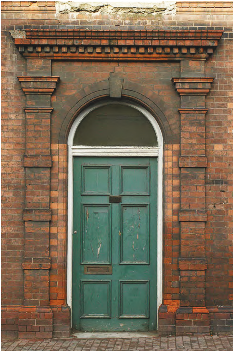
Plate 97: Decorative brickwork and terracotta around front door with bolection moulded panels
