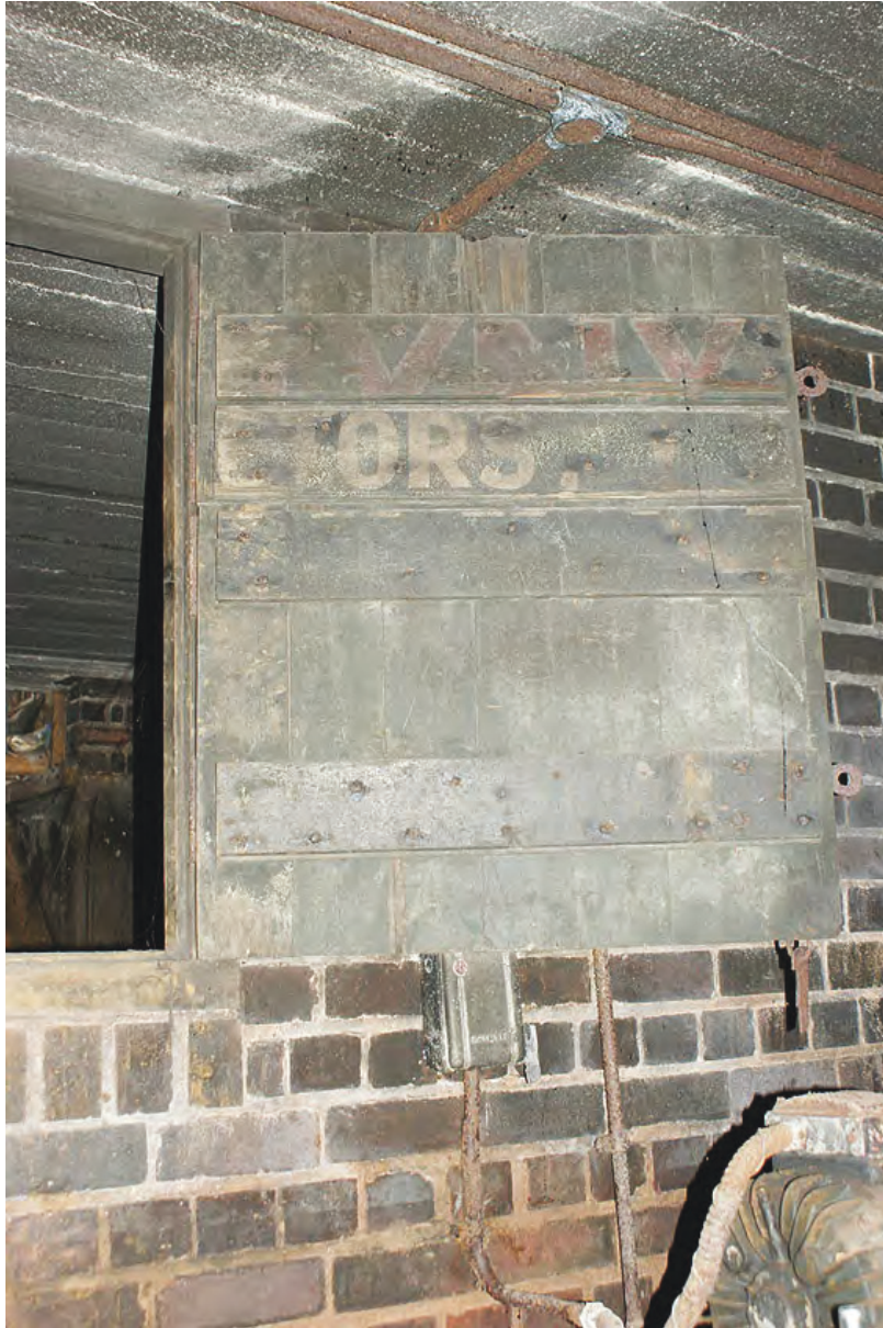
Plate 20: Coal cellar hatch from the south
