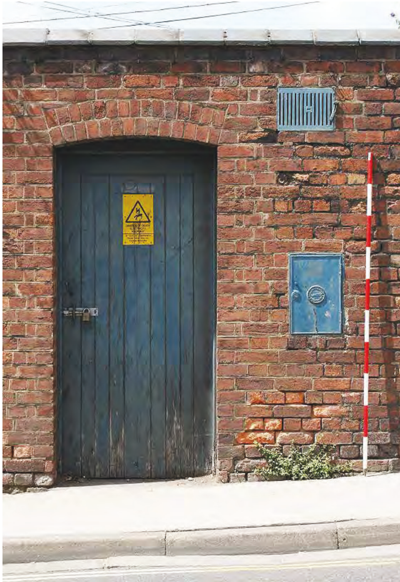
Plate 46: 1930s/40s inserted door, box and air vent
