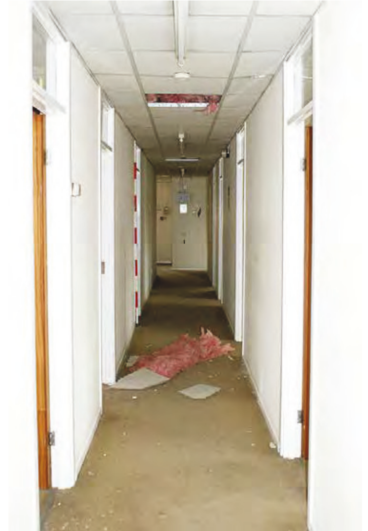
Plate 176: Corridor on sawmill building first floor
