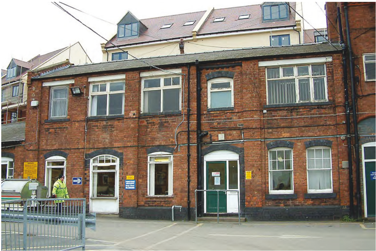
Plate 93: Middle, two-storey range of Joseph Wood building
