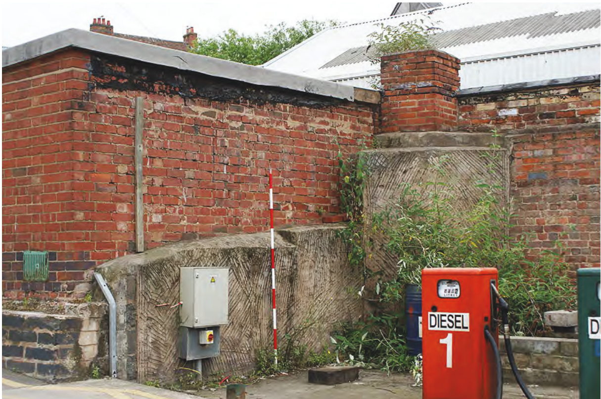
Plate 86: Remains of demolished structure to west of air raid shelter
