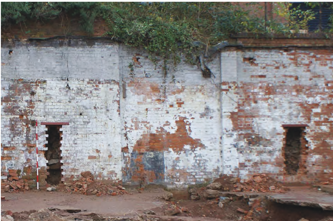
Plate 35: Holes cut into city wall to test the make-up of the wall
