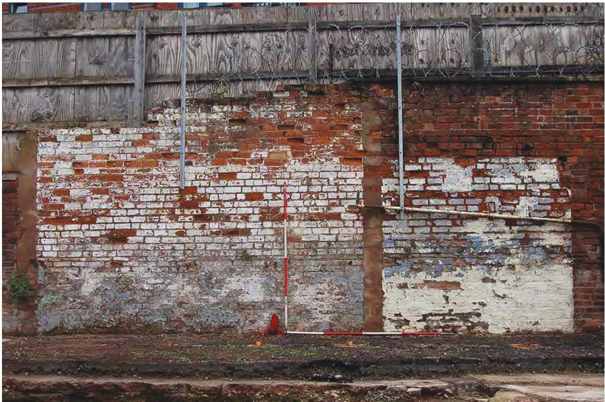
Plate 62: Wall section 5 of Netherton Lane wall, depot side
