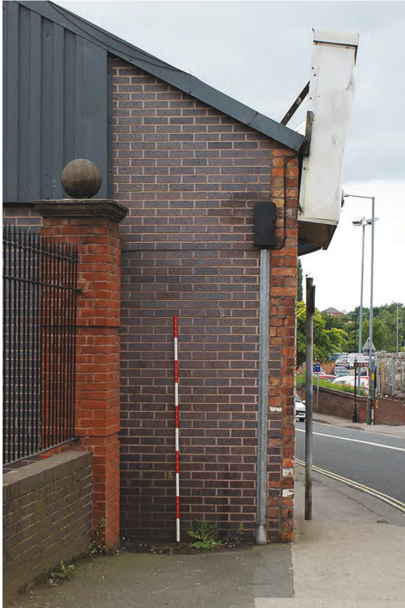
Plate 22 East elevation of Transwipers
