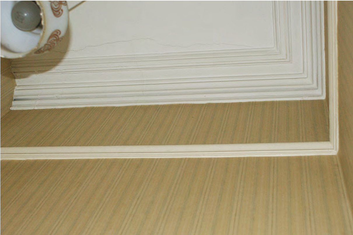
Plate 126: Looking up to ceiling cornice and picture rail, Room F4a
