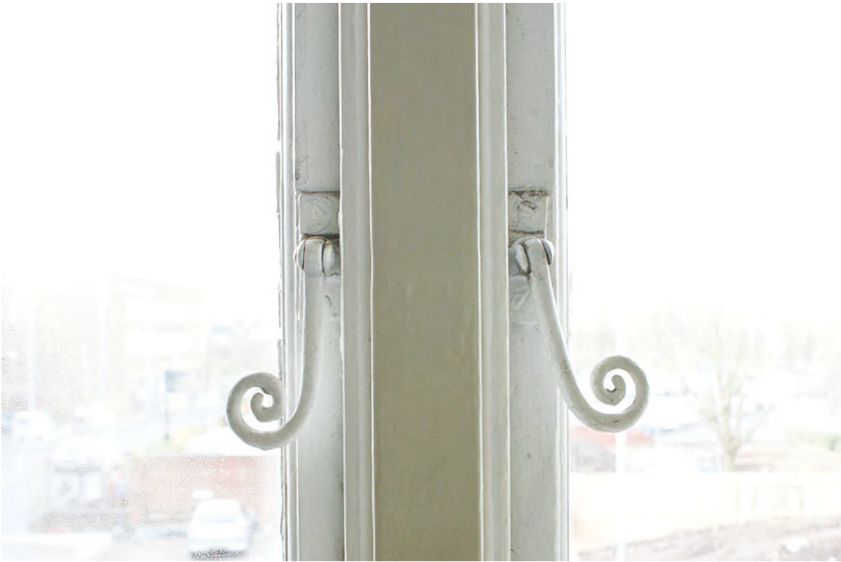
Plate 134: Spiral turnbuckle window catches
