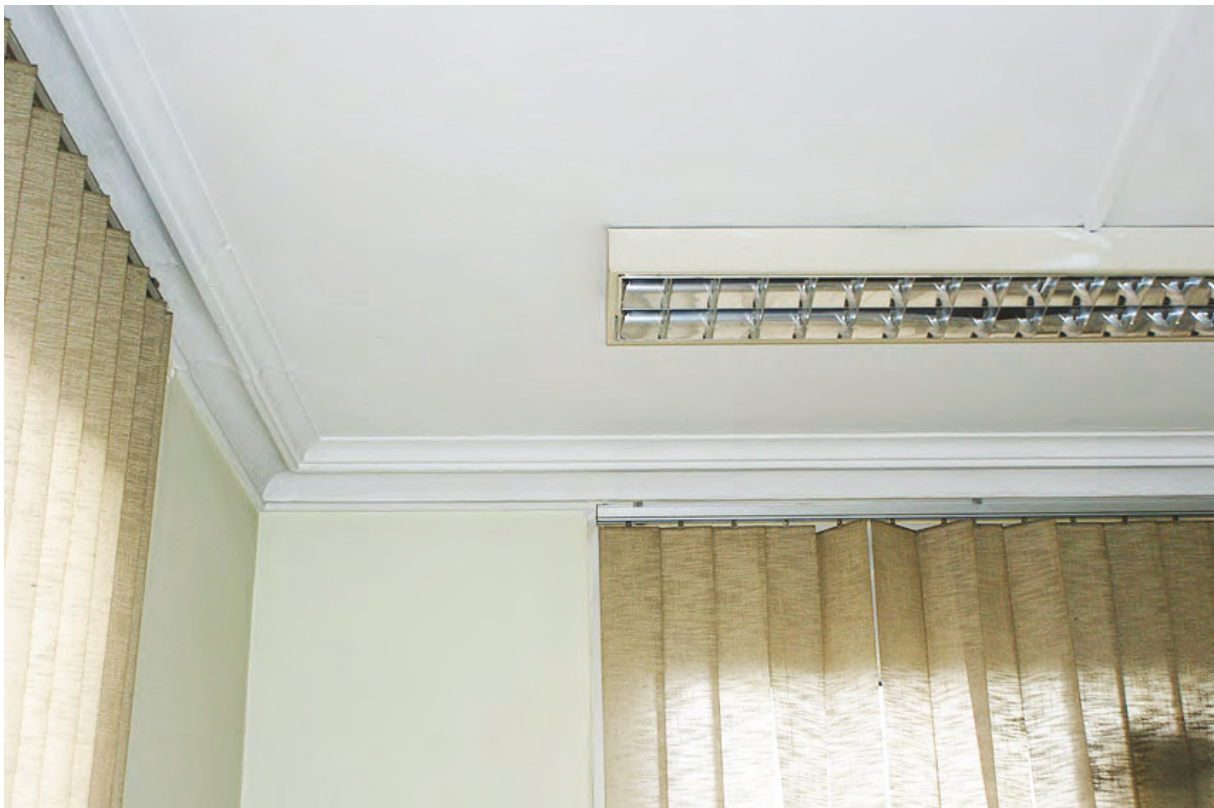
Plate 111: Moulded plaster corncing within the main building
