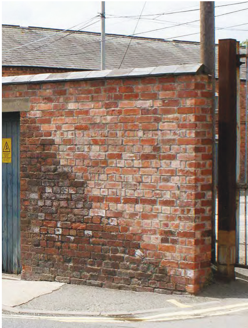
Plate 44: The Butts boundary wall rebuilt east section
