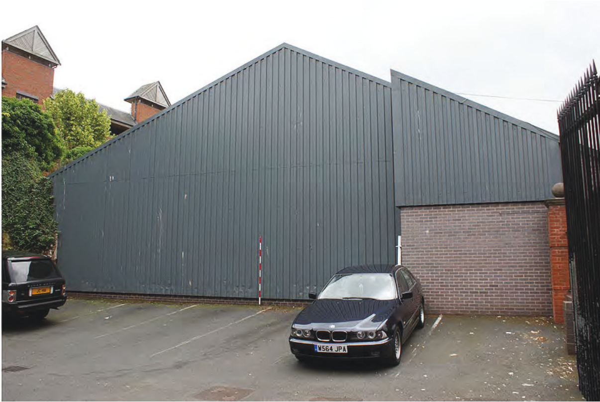
Plate 3: Transwipers building from the east
