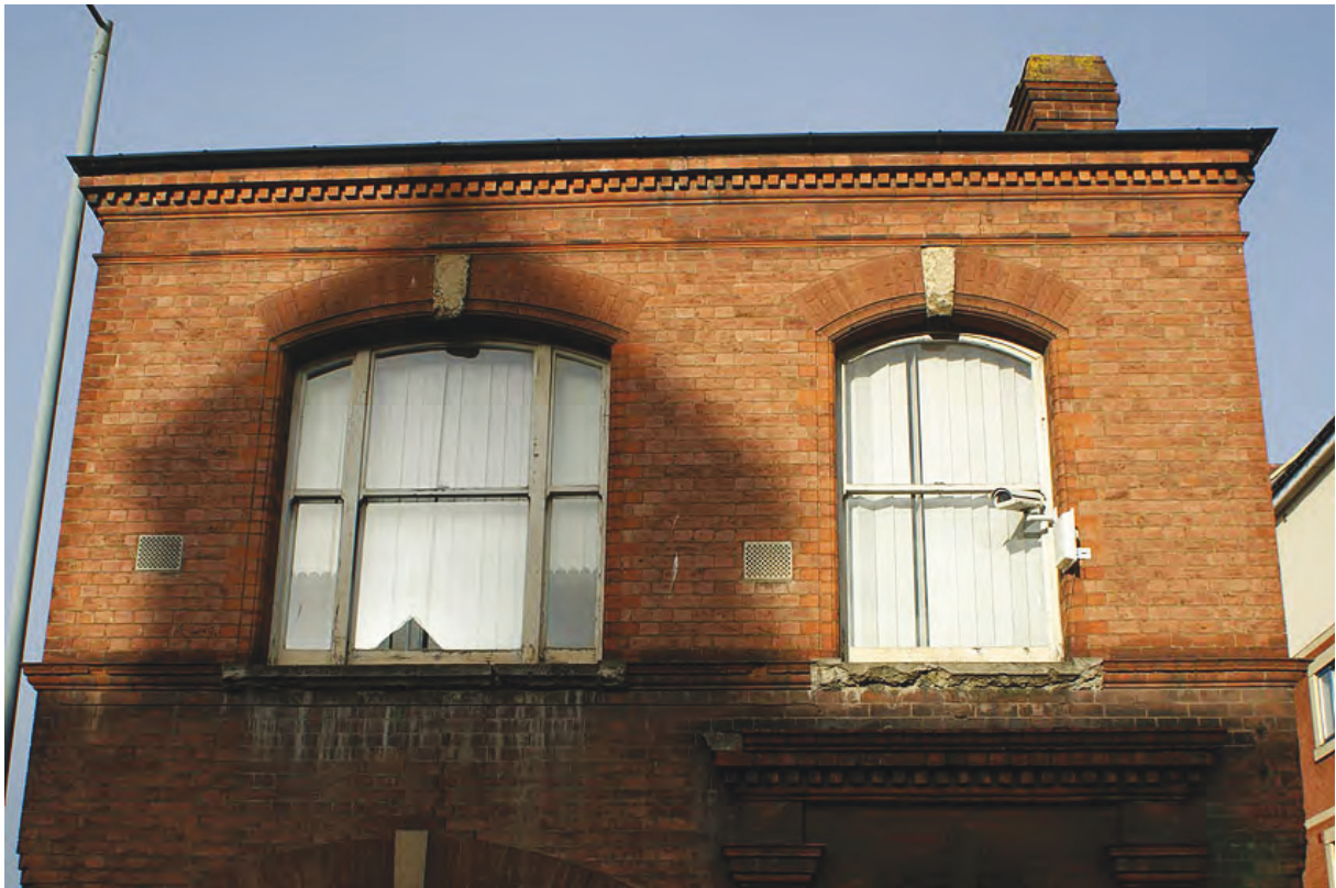
Plate 106: First floor, south elevation of the 'office building' fronting The Butts, showing the eaves cornice, window surrounds and string courses
