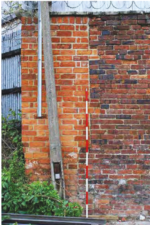
Plate 69: Wall section 6 of Netherton lane wall, depot side
