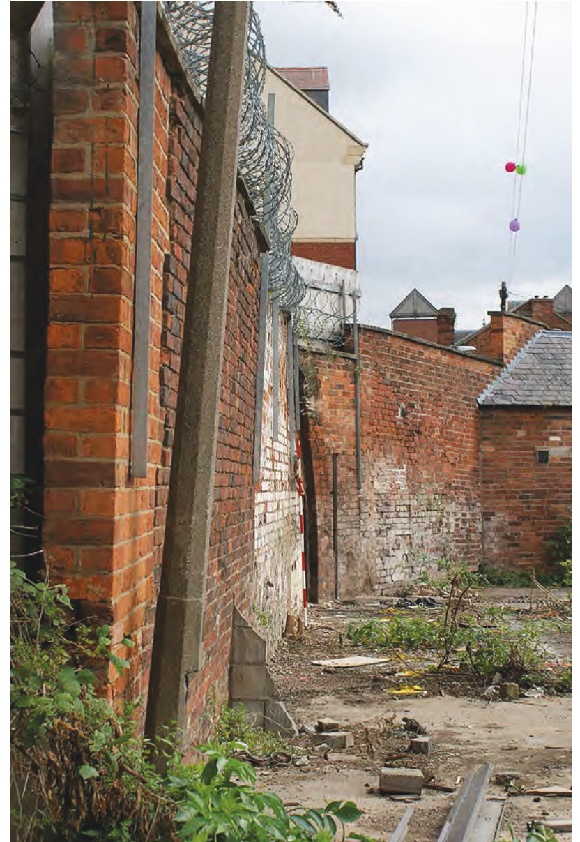
Plate 57: Depot side of Netherton Lane wall
