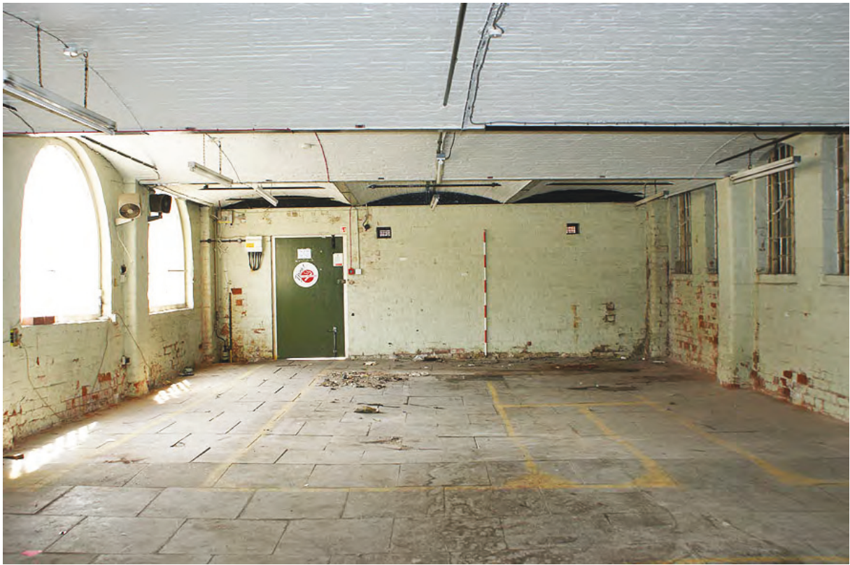
Plate 168: Interior ground floor of sawmill building from the north
