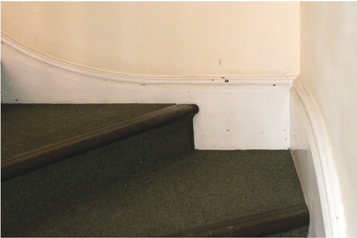
Plate 129: Roll beaded skirting on staircase, Room F3
