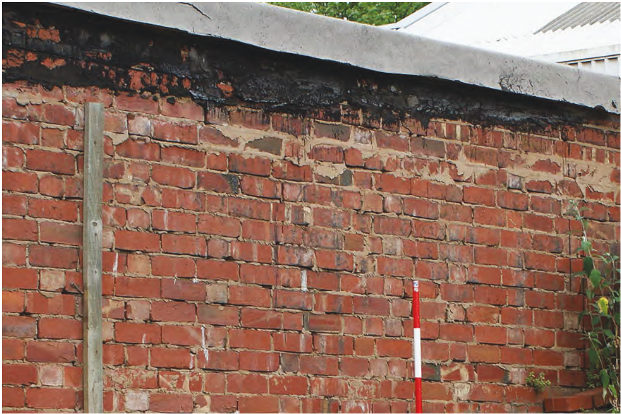
Plate 85: Unfinished mortar on air raid shelter west elevation
