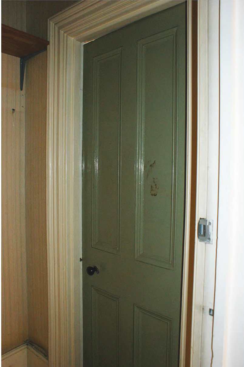
Plate 128: Example of surviving bolection panelled door, Room F4a
