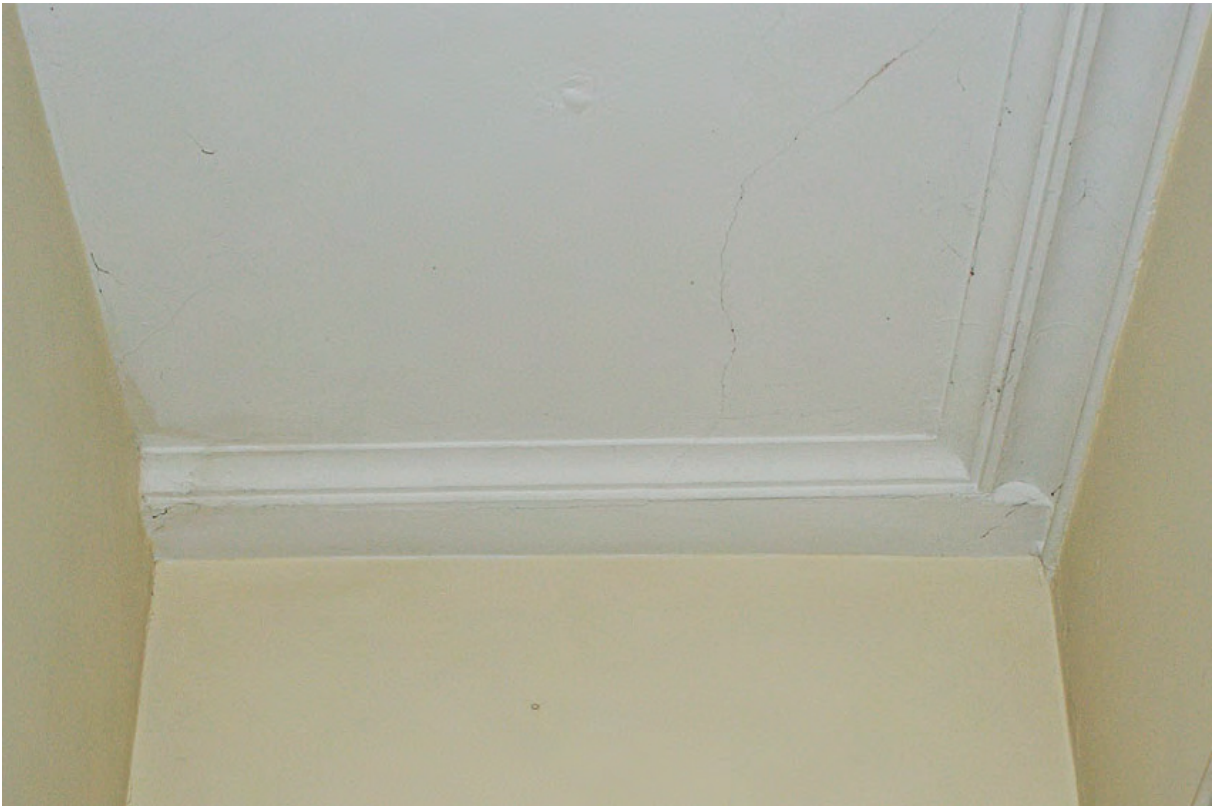
Plate 109: Moulded plaster corncicing, Room G3
