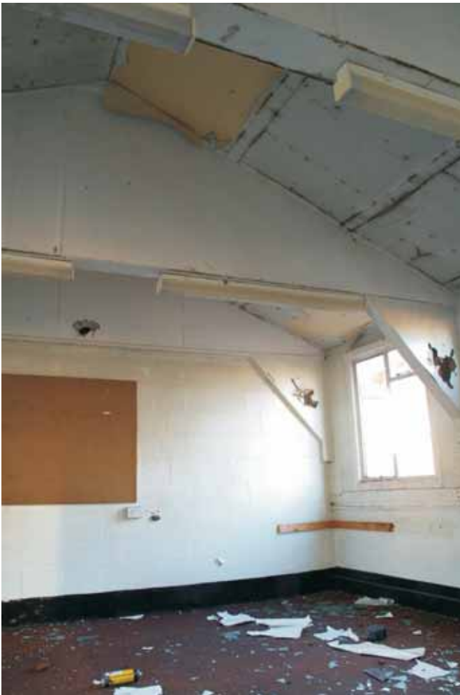
Plate 3.6: Building 3 – detail of internal roof structure, view to the northeast
