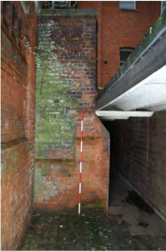
Plate 36.5: Building 36 – easternmost part of southern elevation, view to the north
