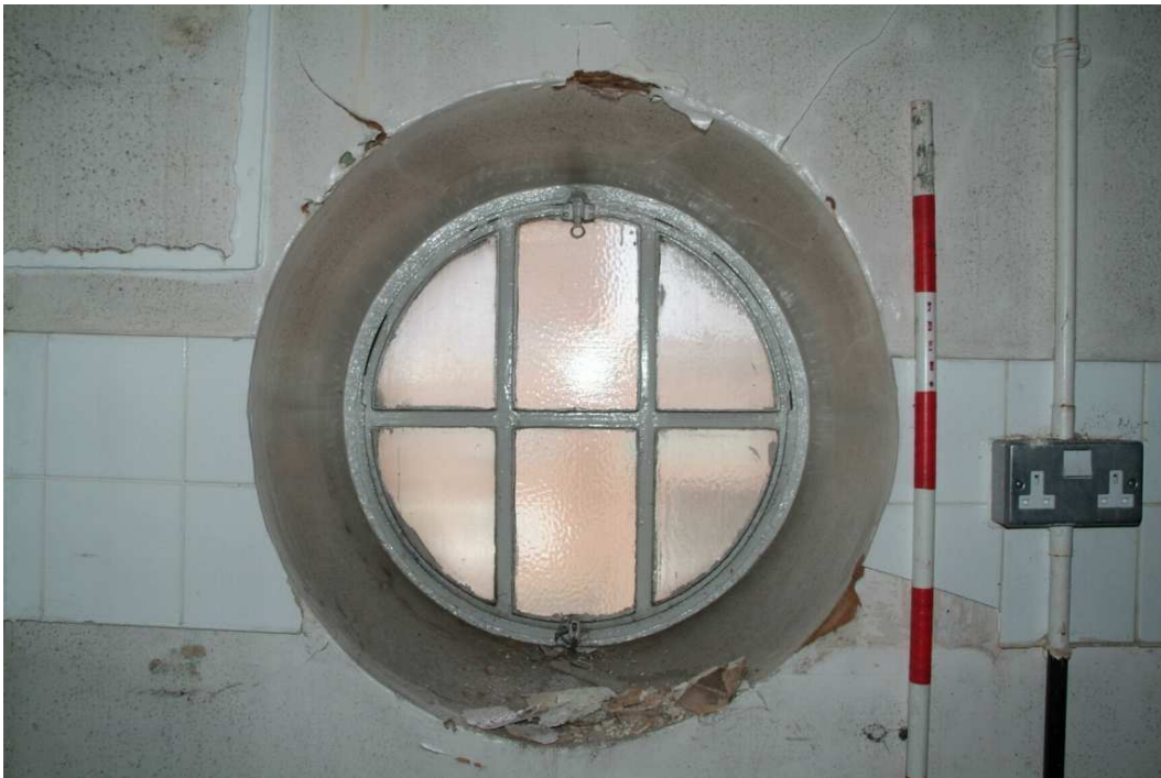
Plate 40.24: Building 40 (UGF): detail of oculus window, view to the north
