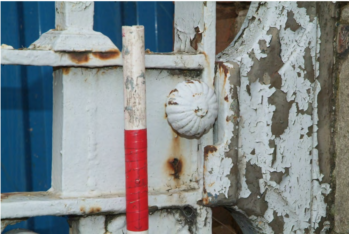
Plate 42.7: Building 42 –detail of lock in pedestrian gate
