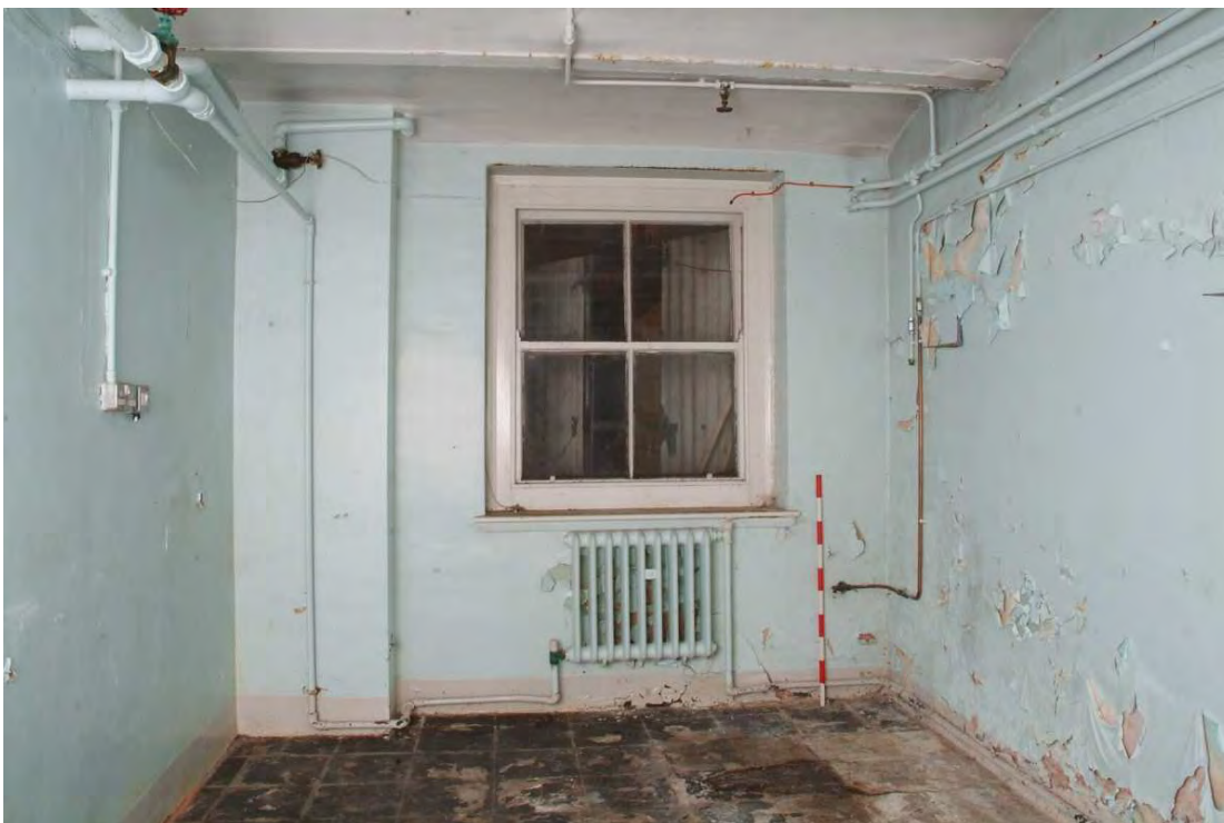
Plate 43.46: Building 43 – basement: former boiler room, view to the north
