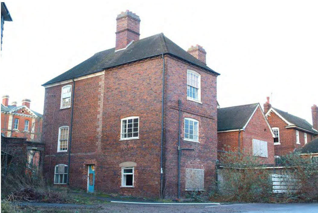
Plate 30.6: Building 30: western elevation, view to the northeast
