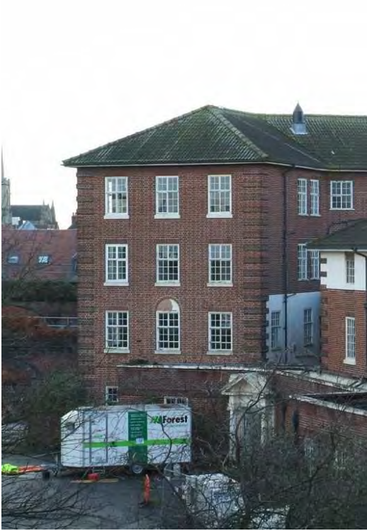
Plate 27.41: Building 27b – northeast elevation showing ground floor connecting corridor from building 27a
