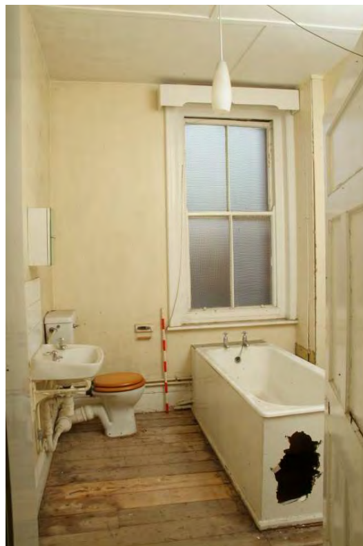
Plate 43.58: Building 43 - first floor: bathroom in central range, view to the east
