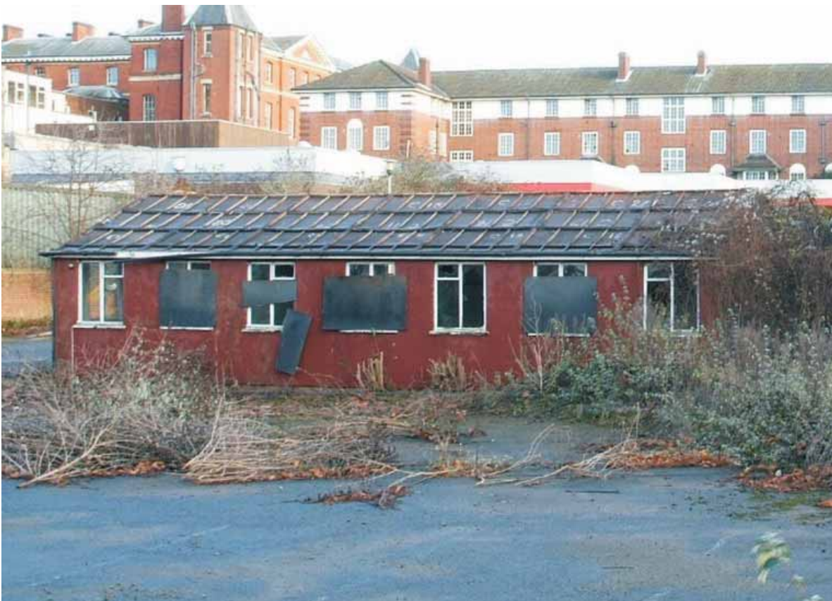
Plate 3.3: Building 3 – western elevation
