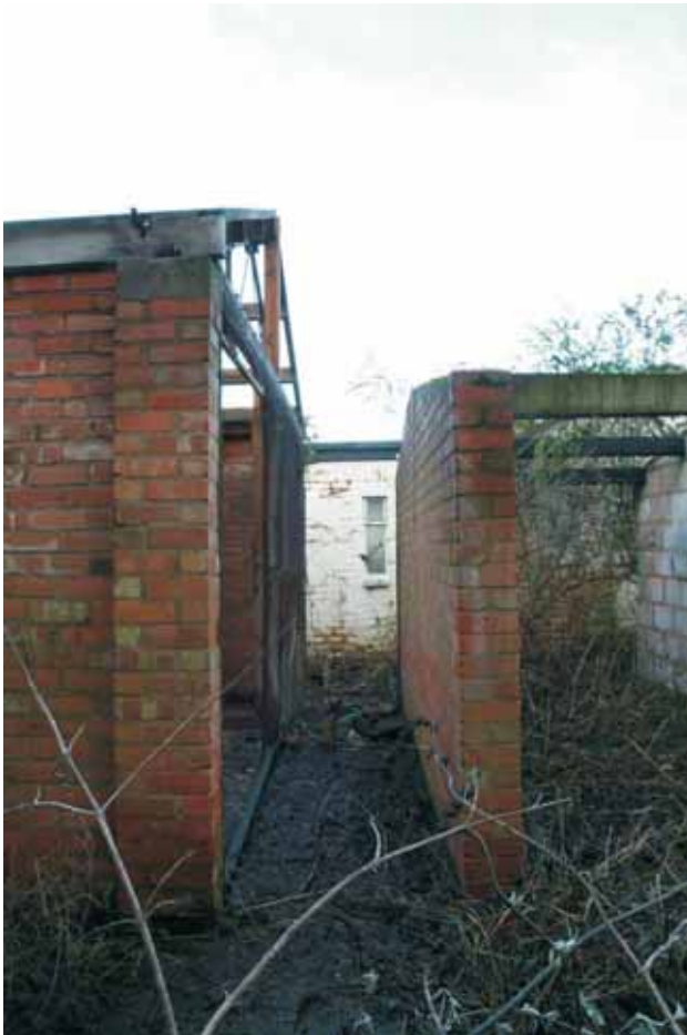
Plate 1.4: Building 1 – eastern elevation against Building 4
