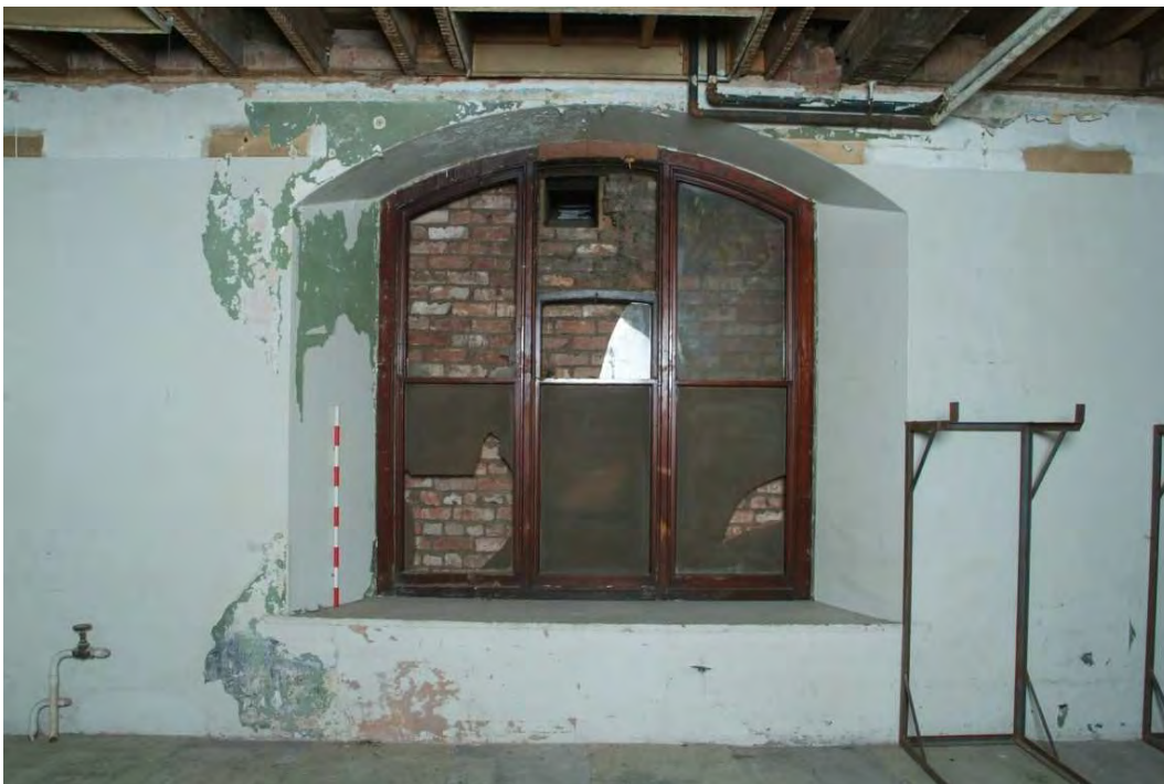
Plate 24.134: Building 24 (LGF): detail of northern original window and blocking of Building 24e [Room 91], view to the north
