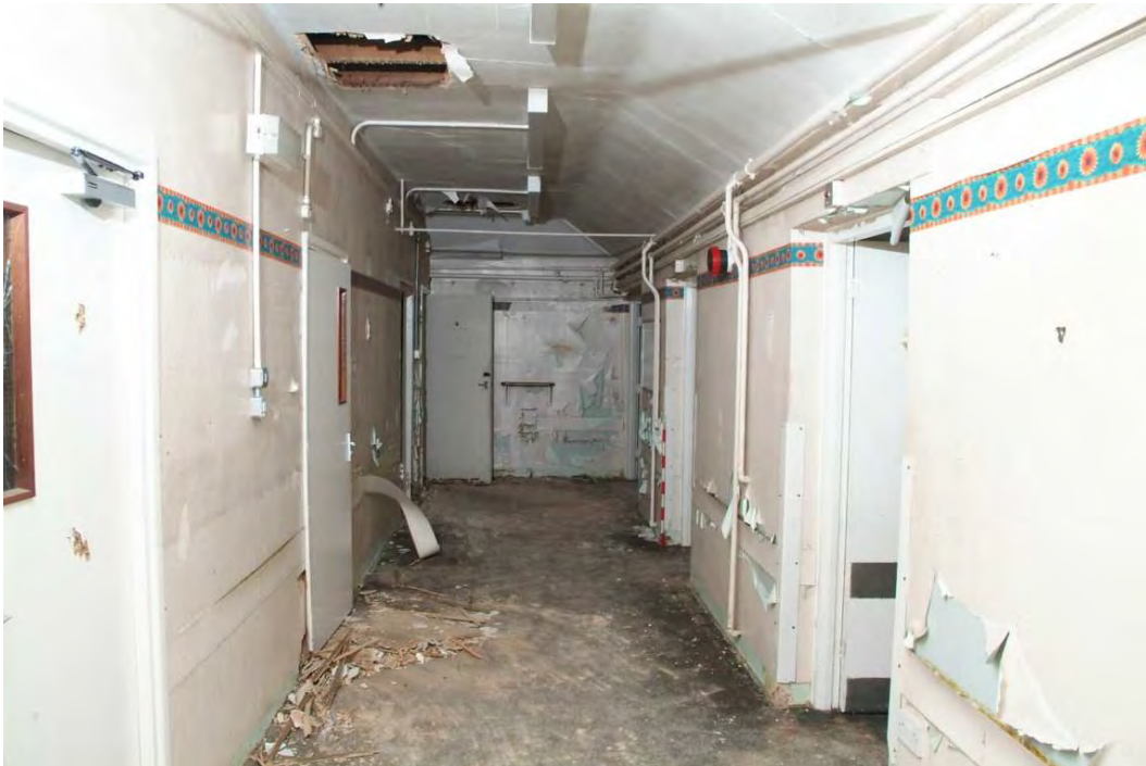
Plate 40.20: Building 40 (UGF): main east-west corridor [Room 1.5], view to the east
