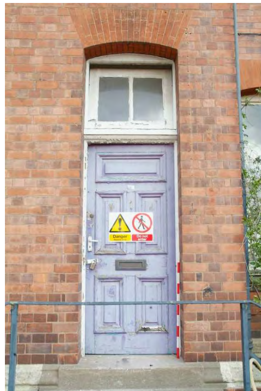
Plate 43.16: Building 43 – side door on the left of the western elevation
