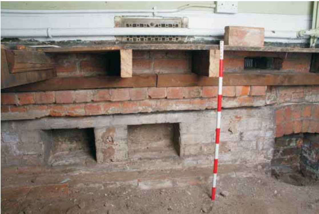
Plate 18.25: Building 18 – ground floor: interior of northern elevation showing openings to vertical shafts below the ground floor, view to the north
