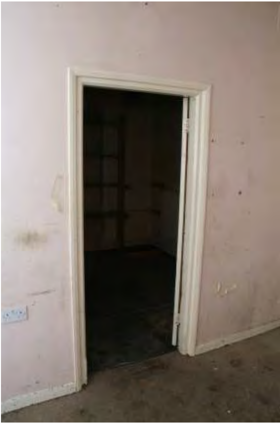
Plate 35.9: Building 35 – internal partition, view to the southwest
