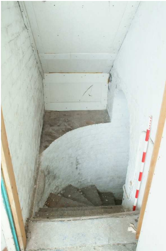
Plate 24.123: Building 24 (LGF): stairs to basement, view to the east
