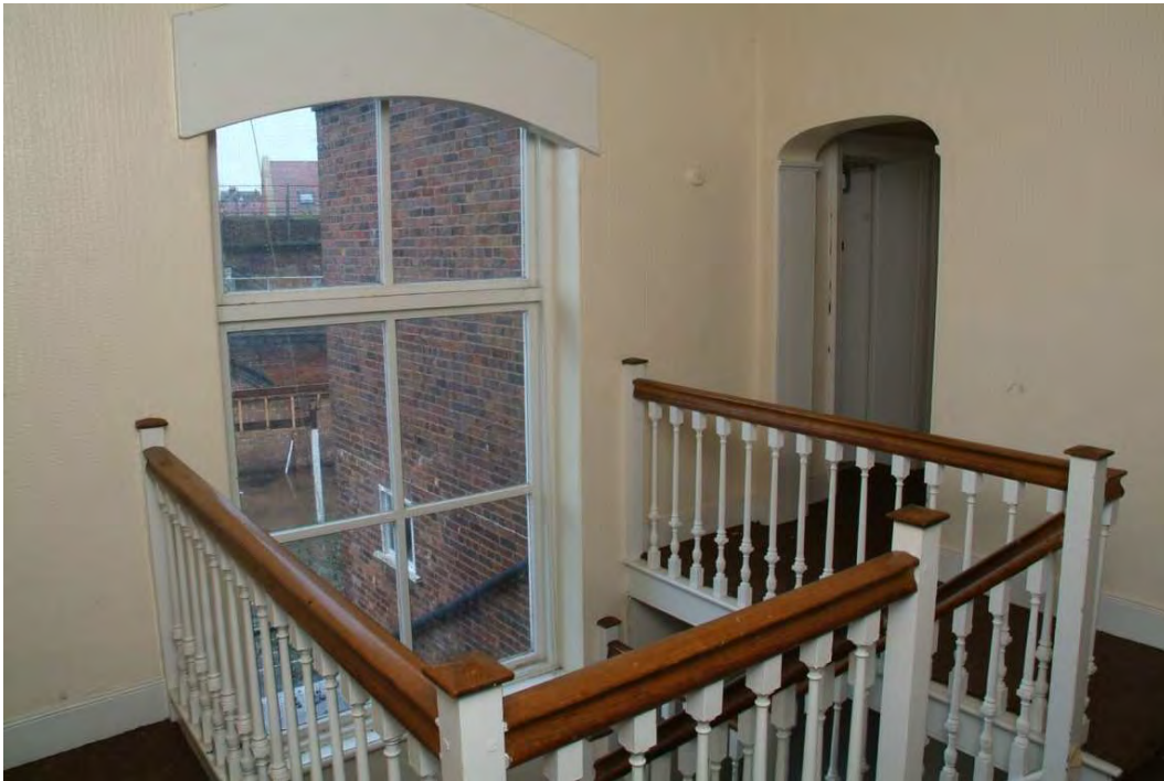
Plate 30.37: Building 30 (FF): landing showing inserted door beyond, view to the southwest
