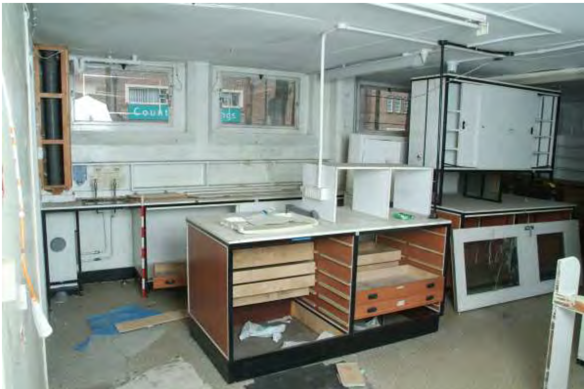
Plate 41.21: Building 41 – ground floor - dispensary, view to the northeast
