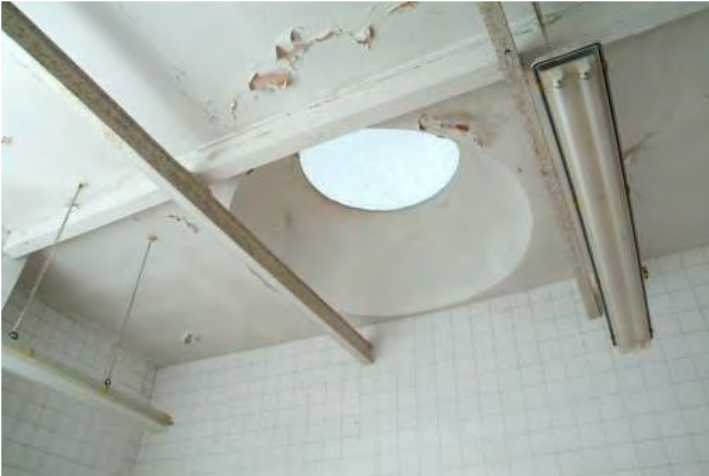
Plate 34.8: Building 34 – detail of c.1950s roof light
