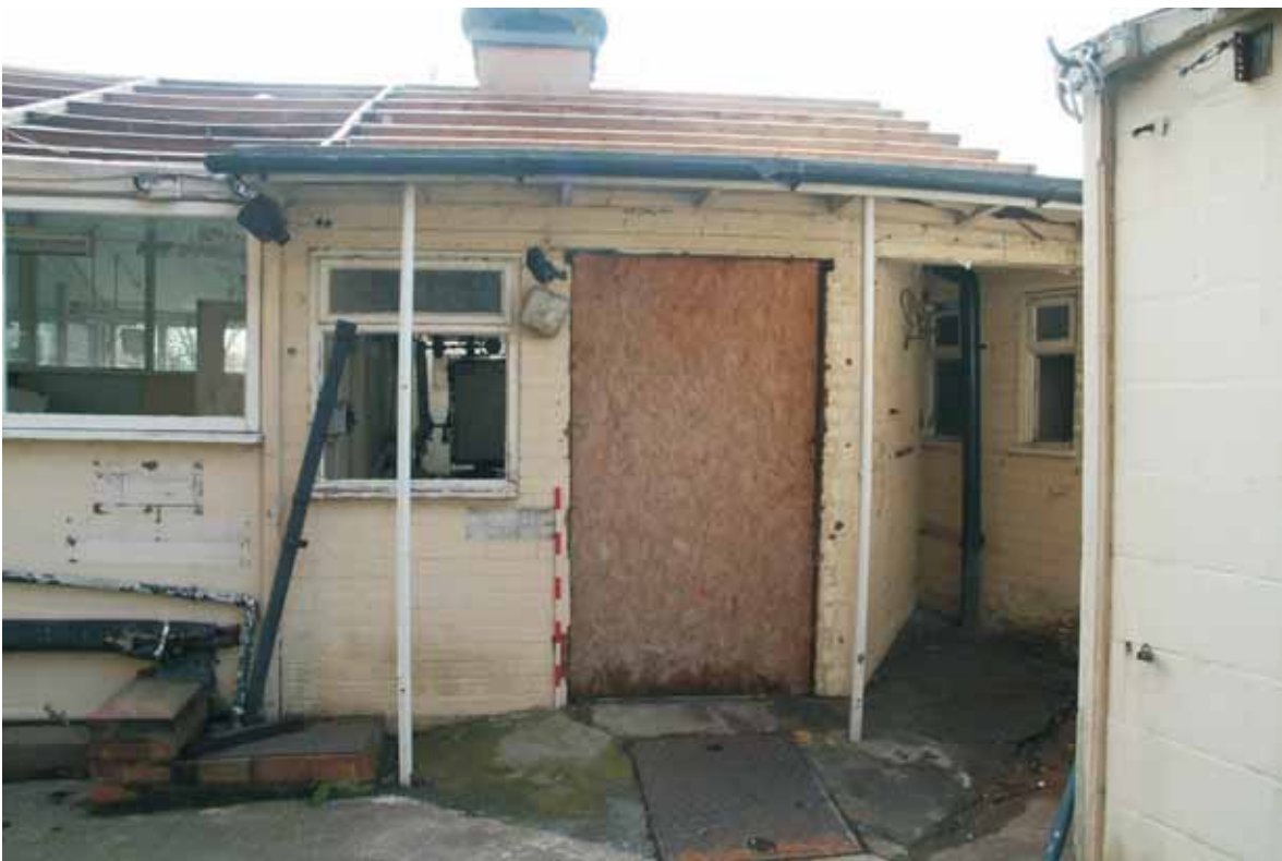
Plate 20.3: Building 20 – east elevation of linking range
