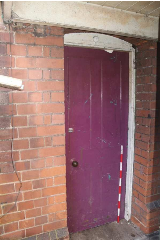
Plate 43.9: Building 43 – detail of basement entrance on north elevation
