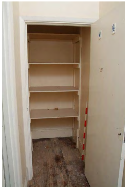
Plate 43.60: Building 43 - first floor: inserted cupboard on east side of central corridor, view to the east
