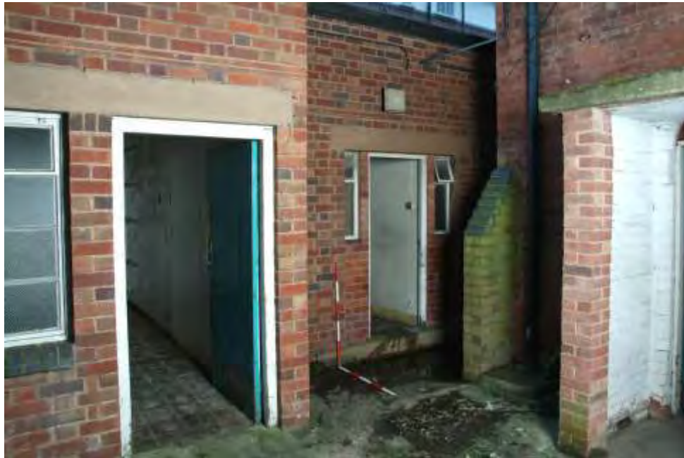
Plate 33.5: Building 33 – northern elevation of eastern part, view to the southeast
