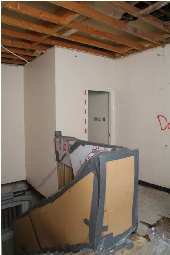
Plate 24.187: Building 24 (SF): top of northern staircase, view to the northwest
