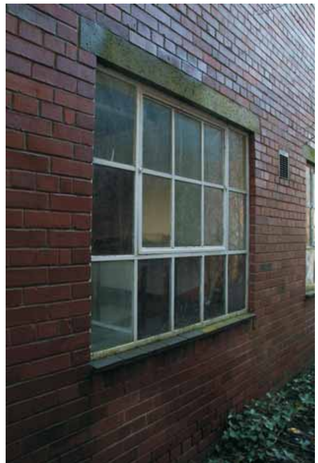
Plate 6.6: Building 6 - detail of typical window
