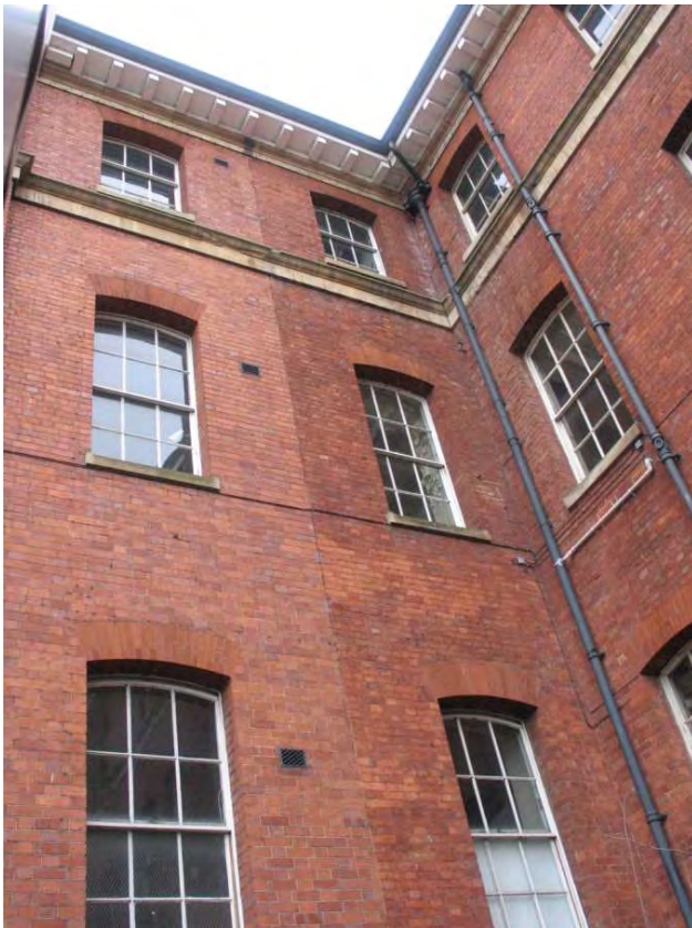
Plate 24.3: Building 24: detail of north facing elevation of SE wing showing point of extension
