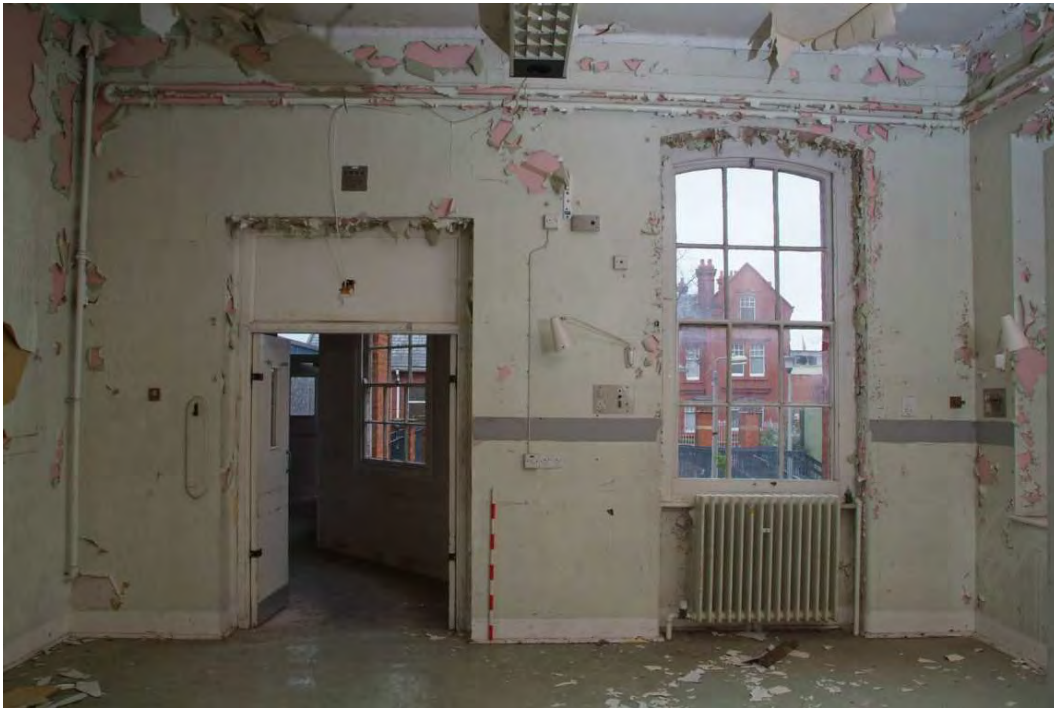
Plate 24.59: Building 24: Rushout Ward [Room 1.11], view to the east
