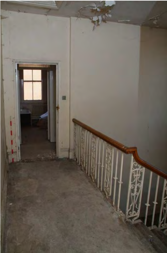
Plate 43.67: Building 43 – second floor: landing, view to the north
