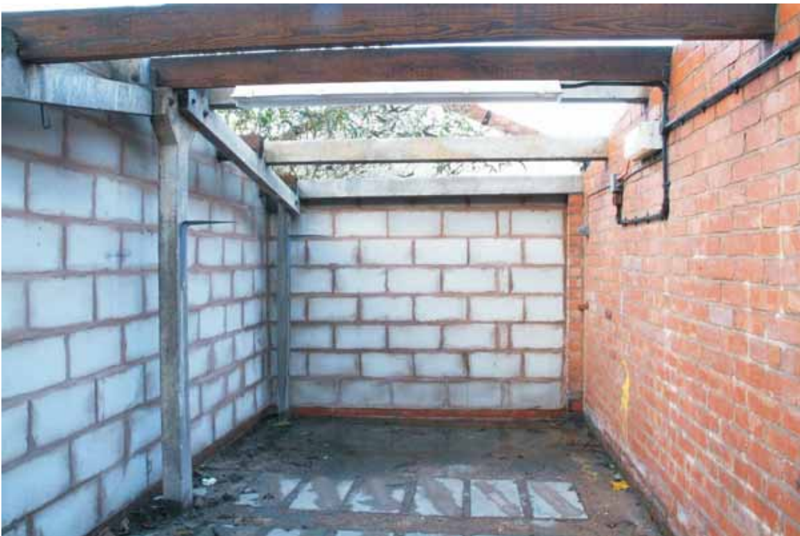
Plate 4.3: Building 4 – interior of western part
