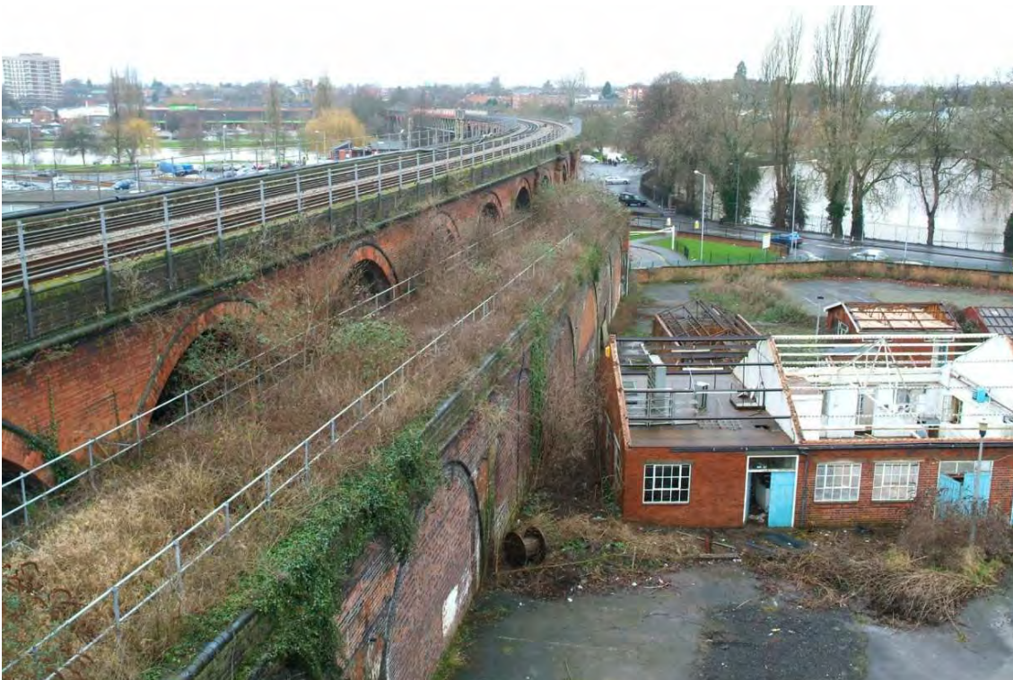
Plate 44.6: Building 44 – general view of carriage way, view to the west
