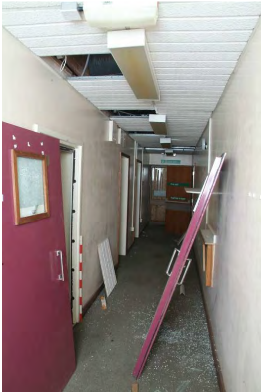
Plate 39.15: Building 39 – lower ground floor eastern corridor view to the south
