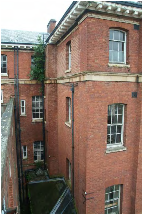
Plate 24.23: Building 24: detail of right hand part of central western elevation, view to the east
