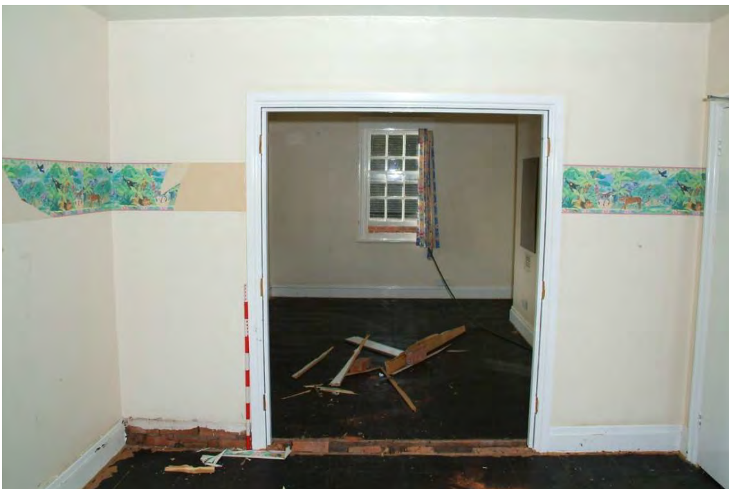
Plate 31.20: Building 31 (FF): principal bedrooms, view to the west
