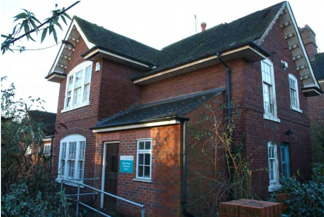
Plate 31.3: Building 31: eastern elevation, view to the southwest
