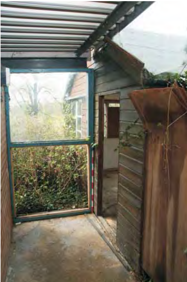
Plate 19.3: Building 19 – passage along north side leading to Building 21
