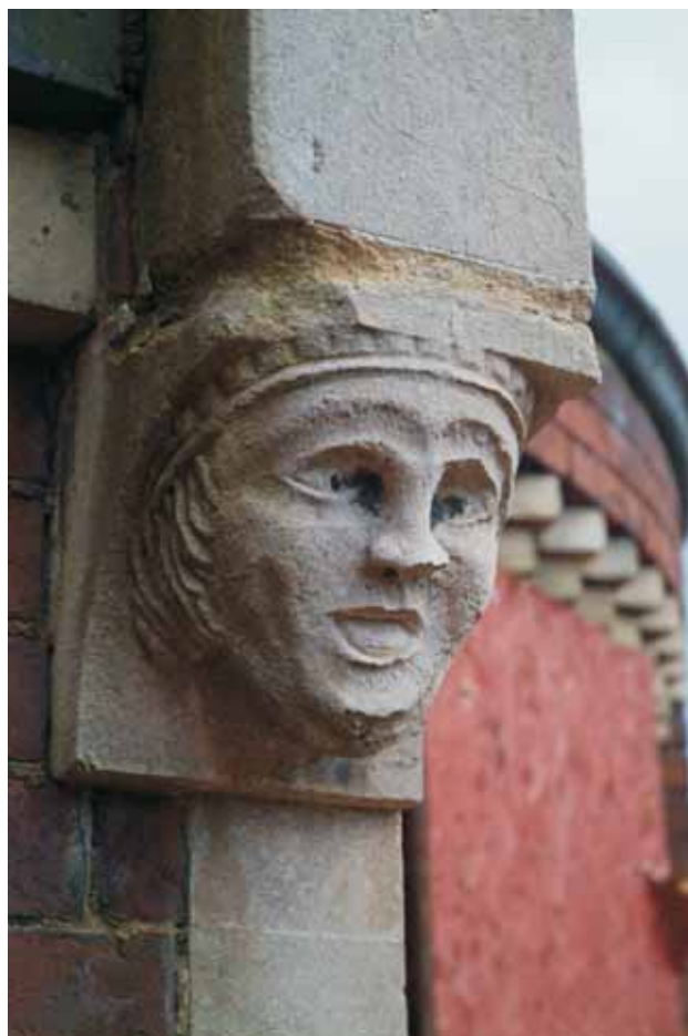
Plate 22.10: Building 22 – detail of carved head kneeler on northern elevation, view to the southwest
