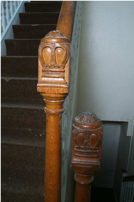
Plate 30.13: Building 30 (GF): entrance hall showing carved newel to staircase
