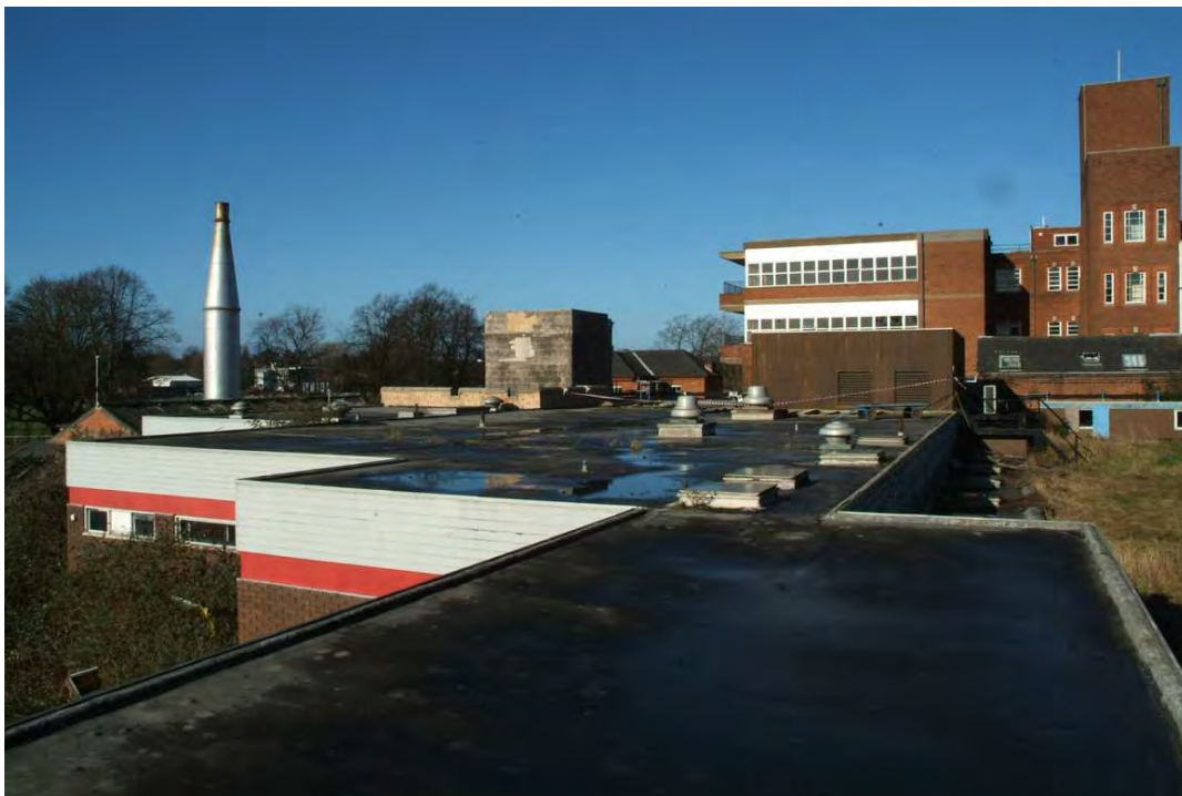
Plate 26.2: Building 26: flat roof, view to the north
