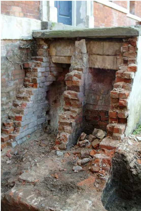
Plate 24.9: Building 24: exterior of barrel vault supporting central platform, view to the northwest
