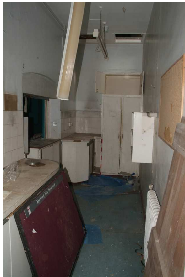
Plate 40.10: Building 40 (LGF): outpatients buffet [Room 0.32]. view to the north
