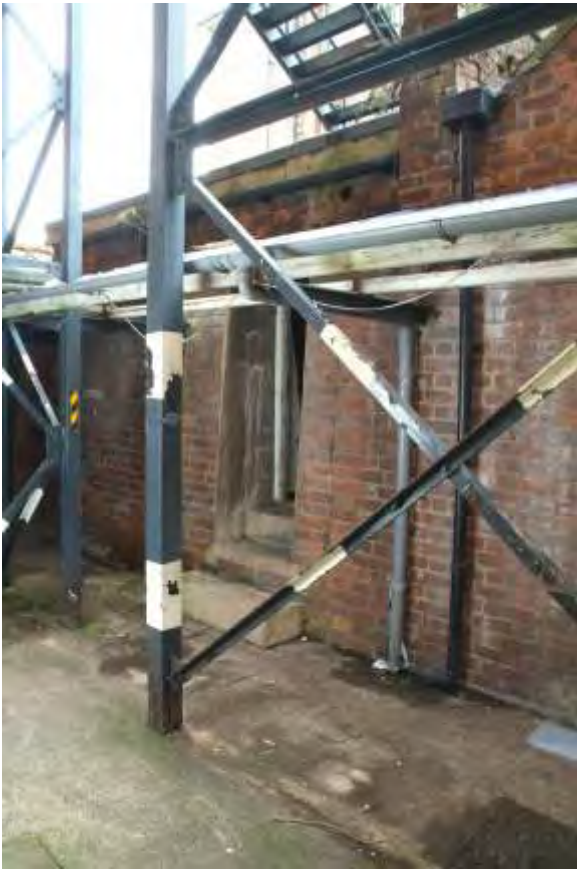
Plate 36.1: Building 36 – general view of north elevation, view to the southeast
