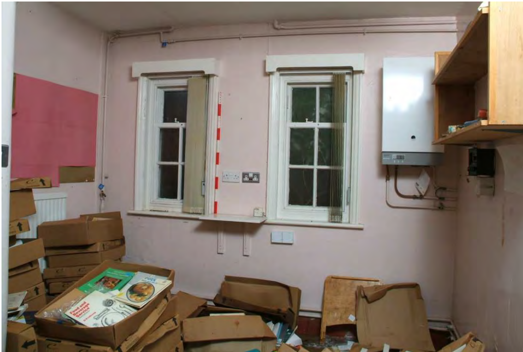
Plate 31.11: Building 31 (GF): interior of former kitchen, view to the southwest
