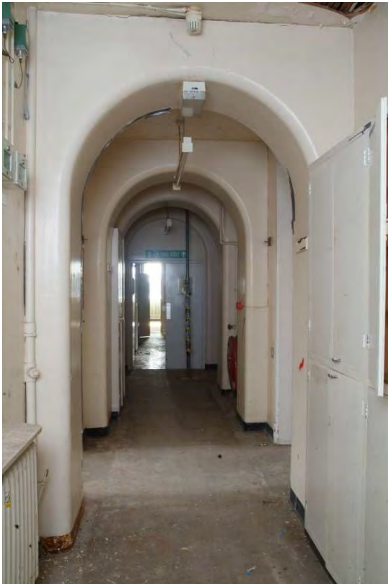
Plate 24.185: Building 24 (SF): central corridor, view to the south
