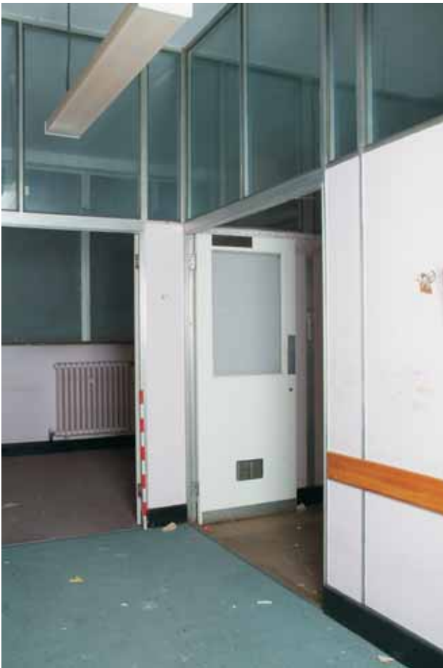
Plate 17.29: Building 17a – ground floor: refurbished treatment rooms, view to the east
