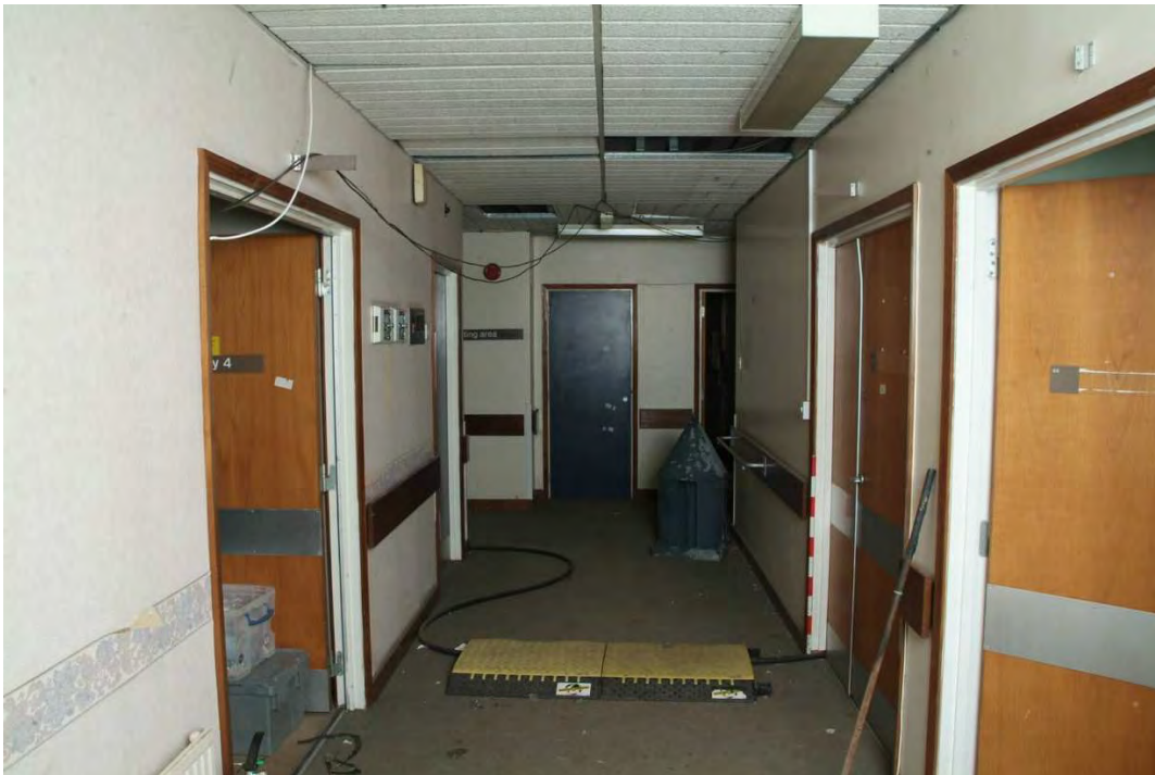
Plate 39.8: Building 39 – upper ground floor main corridor, view to the east
