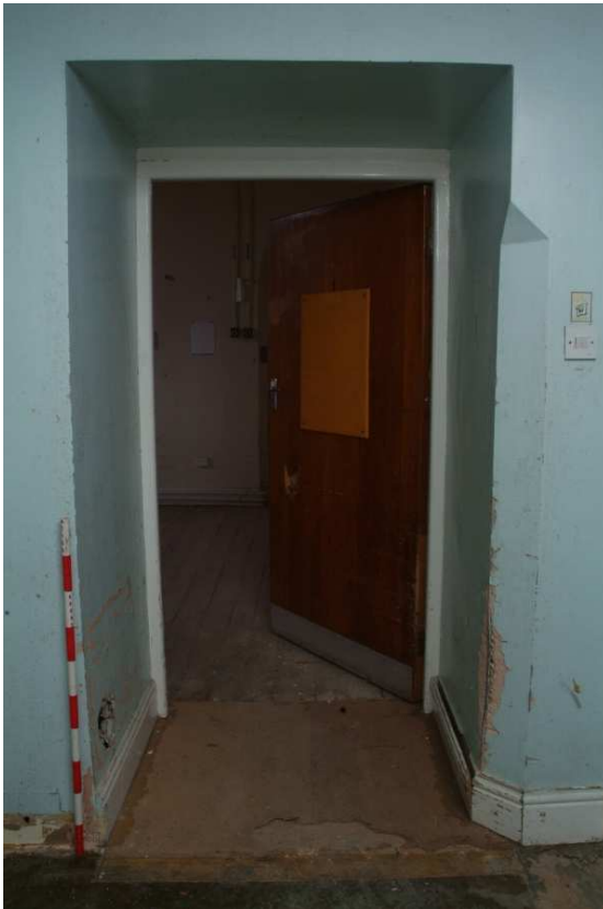
Plate 24.175: Building 24 (FF): inserted opening between Room 2.25 and ward [Room 2.26], view to the south
