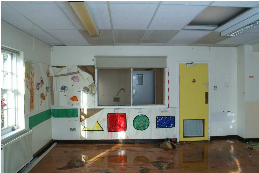
Plate 31.16: Building 31 (GF): west side of extension, view to the north
