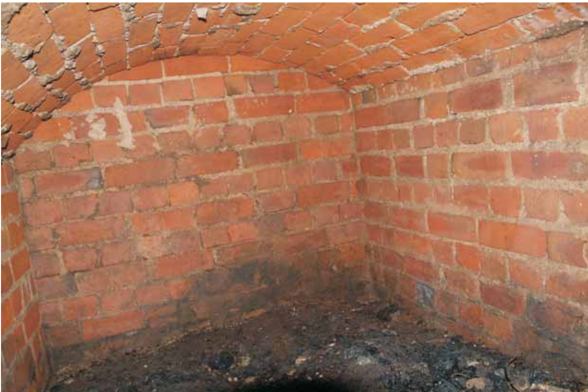
Plate 18.32: Building 18 – basement: interior, view to the south
