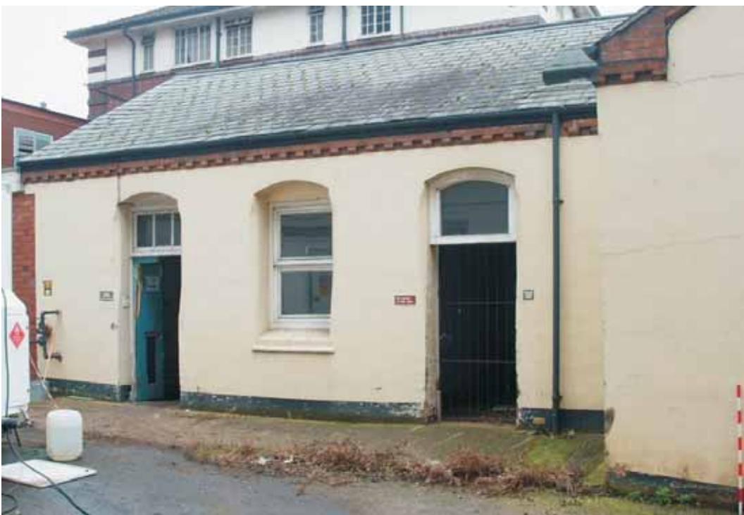
Plate 14.6: Building 14 – eastern wing showing modified windows, view to the southeast
