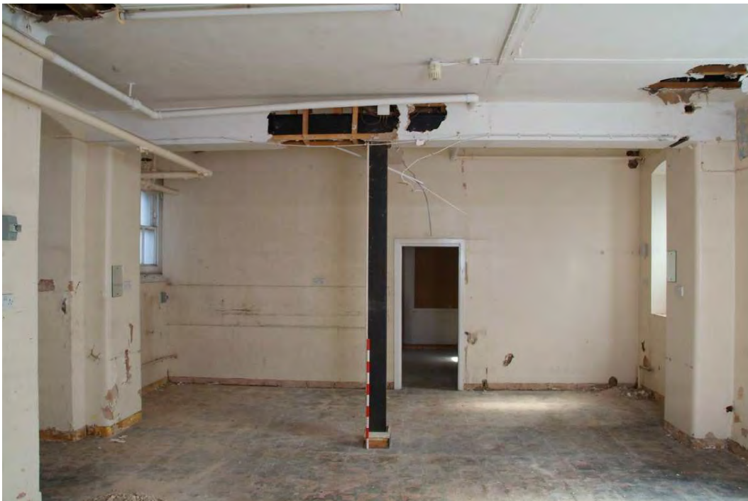
Plate 24.98: Building 24 (LGF): nursing staff changing area [Room 109], view to the east
