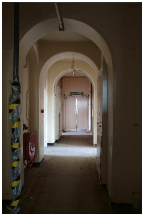
Plate 24.186: Building 24 (SF): central corridor, view to the north
