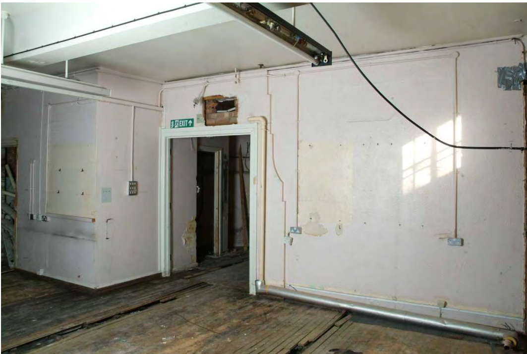
Plate 27.60: Building 27b – lower ground floor: eastern wall of archive room showing blocked projection aperture
