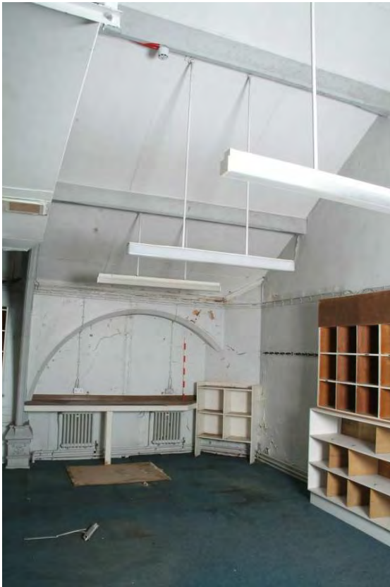
Plate 41.19: Building 41: mezzanine floor (west end), view to the south
