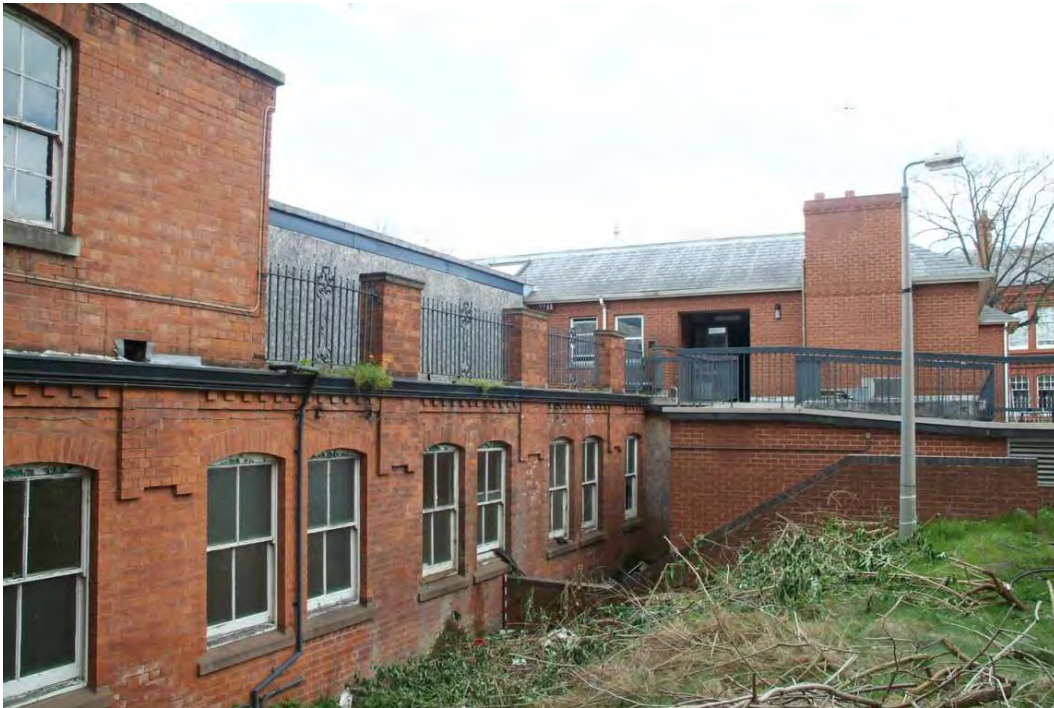
Plate 40.7: Building 40: eastern part of southern elevation, view to the northeast
