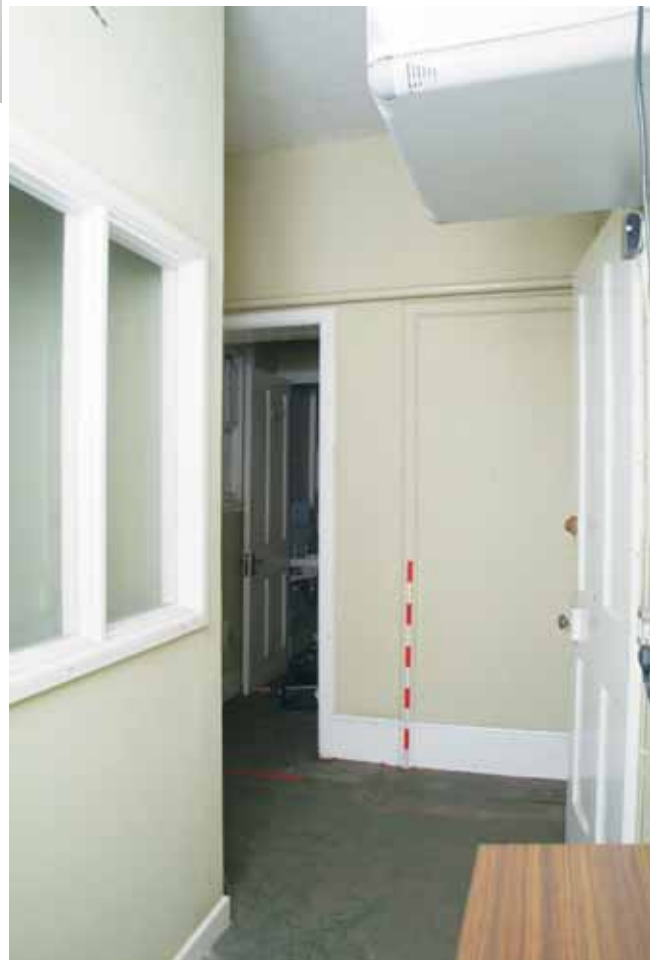
Plate 18.36: Building 18 – first floor: interior of comms room showing lobby area, view to the south
