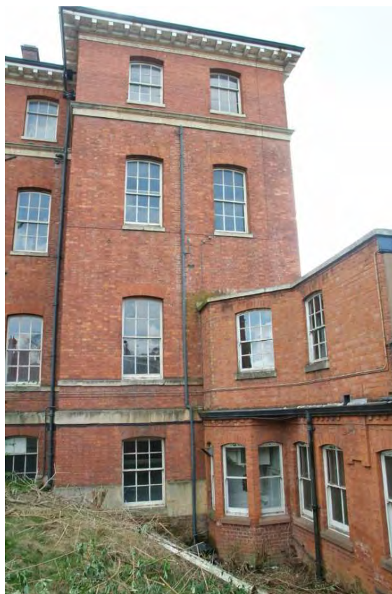
Plate 24.16: Building 24: northern wing, view to the west
