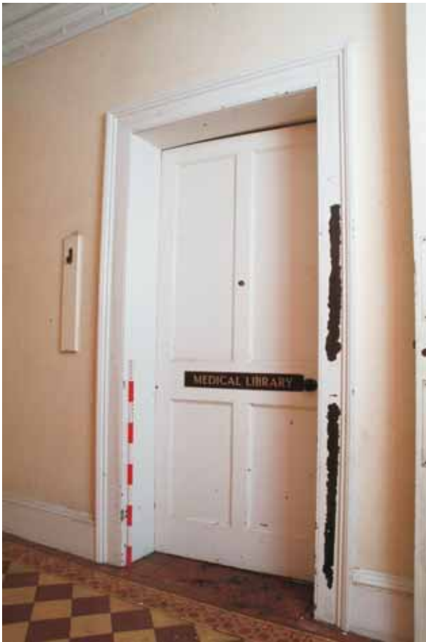
Plate 22.39: Building 22 – connecting range: central corridor on upper ground floor showing doorway on north side, view to the northwest
