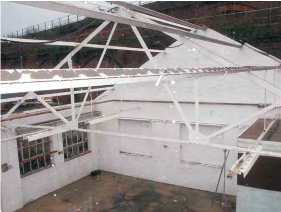
Plate 6.17: Building 6 – roof trusses over former southernmost workshop, view to the southeast
