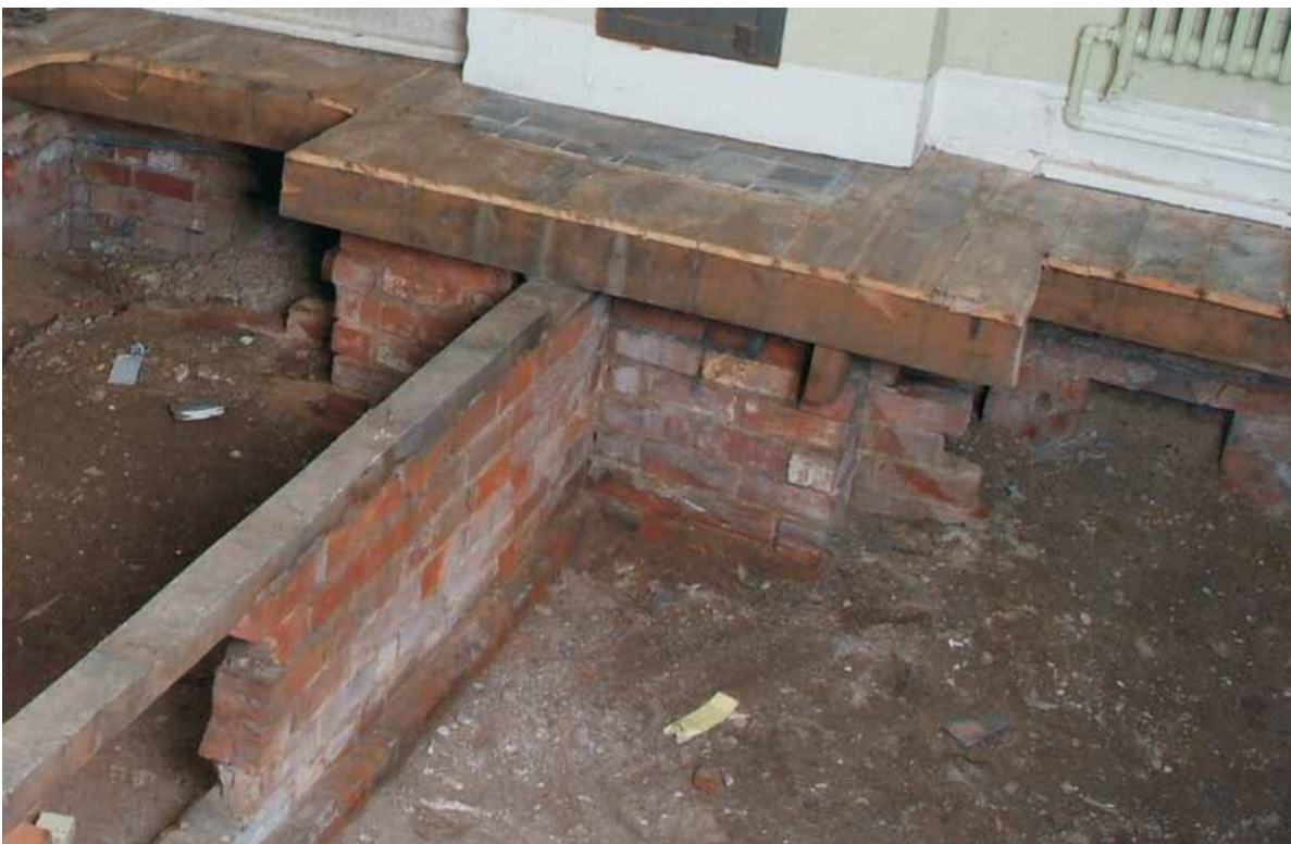
Plate 18.24: Building 18 – ground floor: eastern chimney showing stubs of brick ducting projecting from the chambered hearth plinth, view to the northeast
