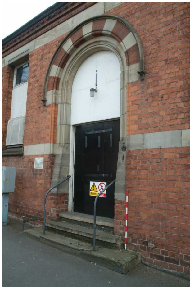
Plate 41.2: Building 41: detail of former main entrance, view to the southeast
