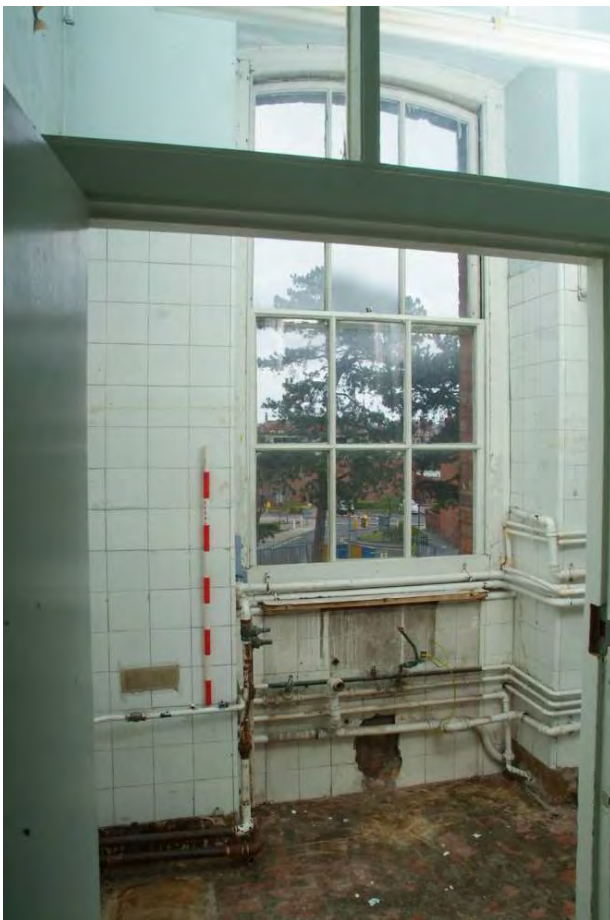
Plate 24.174: Building 24 (FF): interior of sluice room, view to the southeast
