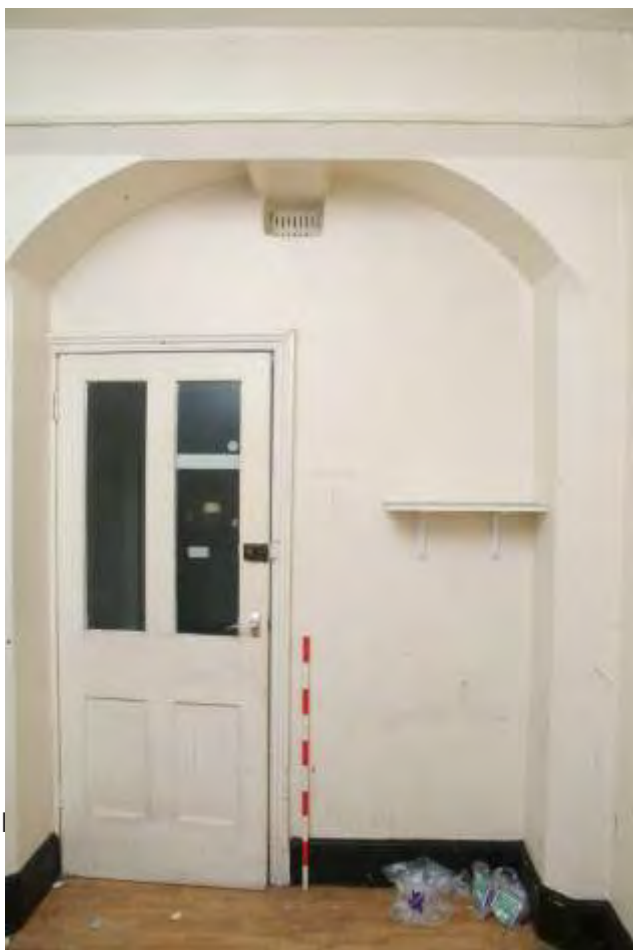
Plate 22.63: Building 22 (LGF): interior of 'Porters Changing Room' showing entrance from central corridor and high level ducts, view to the south
