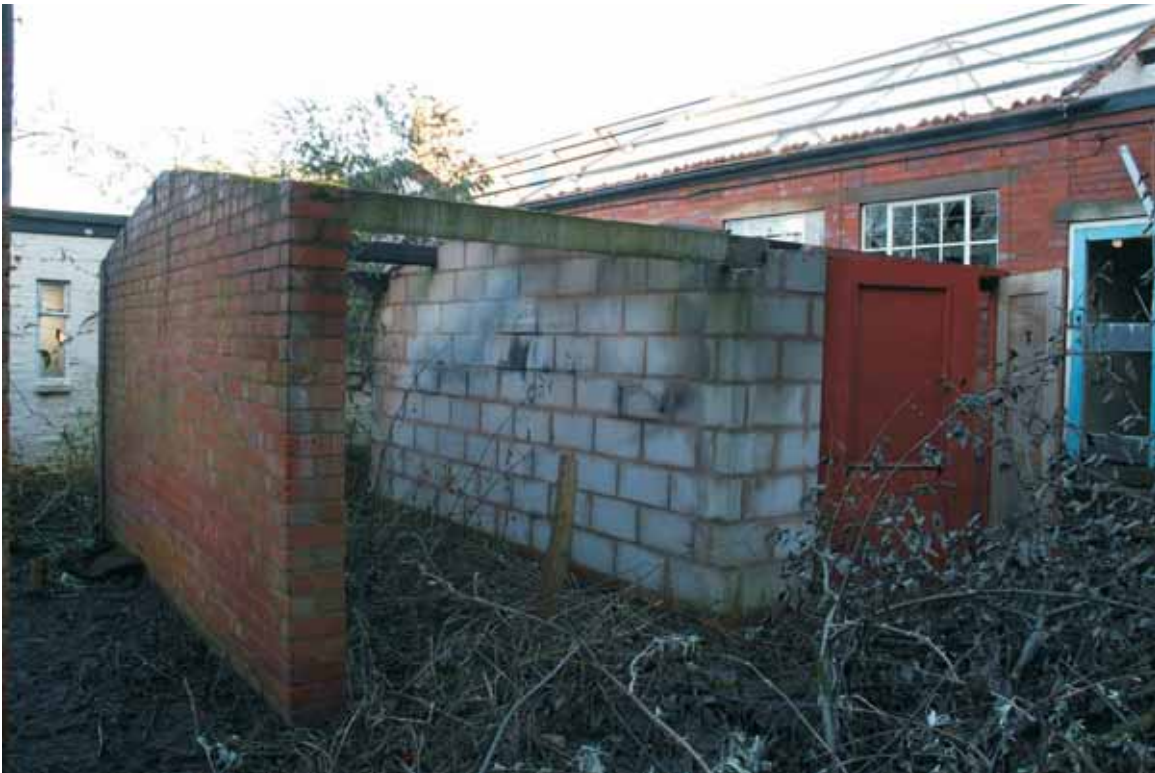
Plate 4.2: Building 4 – southern and western elevations
