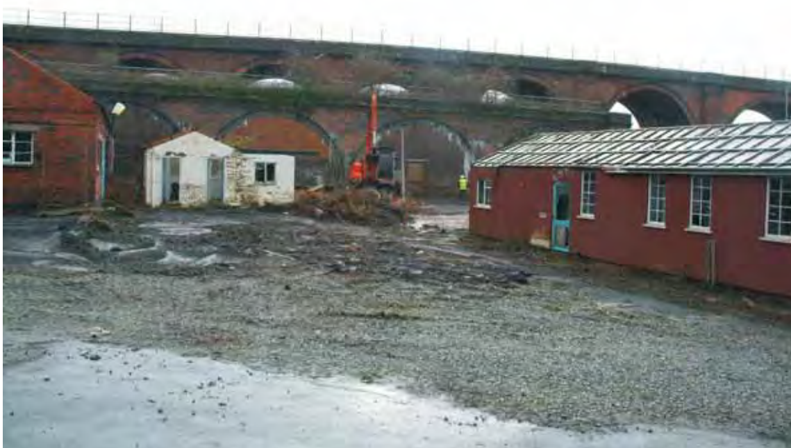
Plate 5.4: Building 5 – northern elevation during demolition
