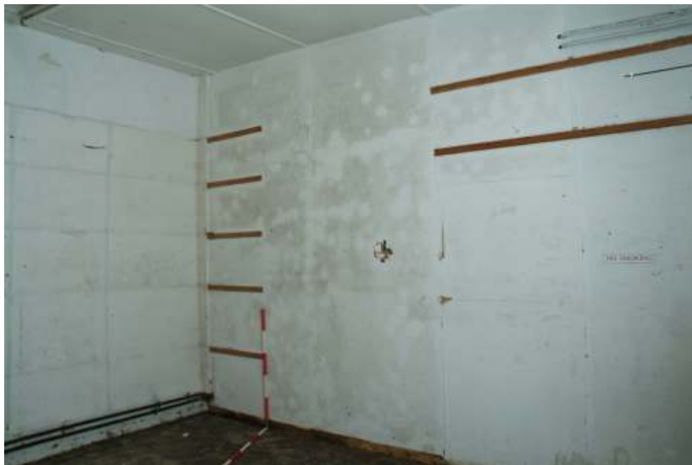
Plate 33.10: Building 33 - interior of northern part, view to the southwest
