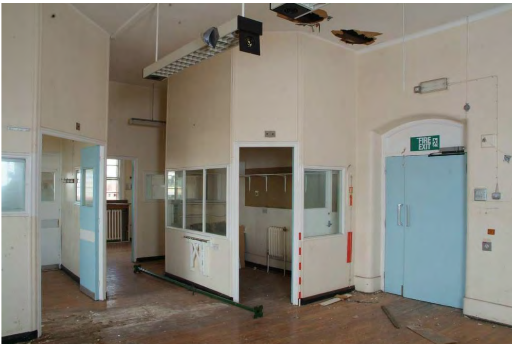
Plate 24.194: Building 24 (SF): subdivision of the eastern part of Maddox Ward, view to the southeast
