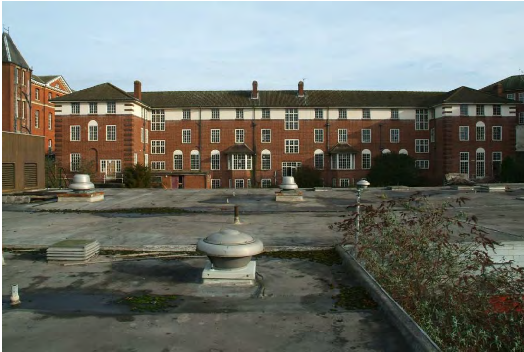
Plate 27.9 : Building 27a - western elevation
