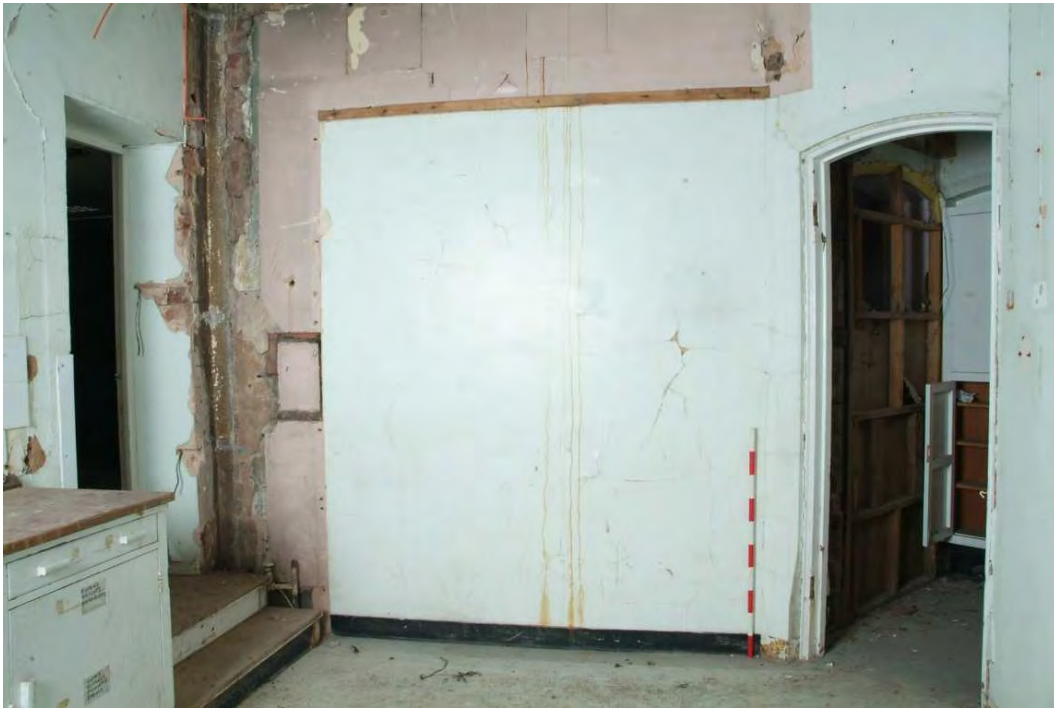
Plate 24.149: Building 24 (LGF): original (right) and inserted (left) doorways in pharmaceutical store, view to the east
