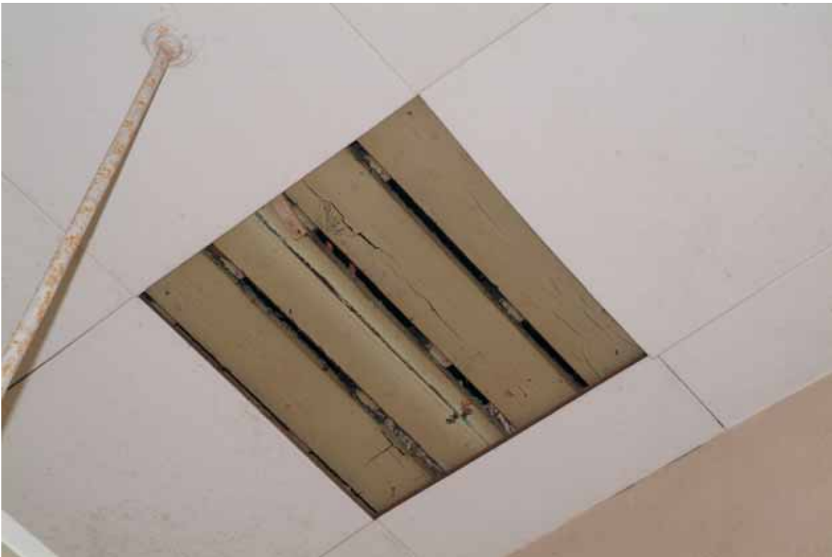
Plate 14.23: Building 14 – detail of original ceiling boarding, view up
