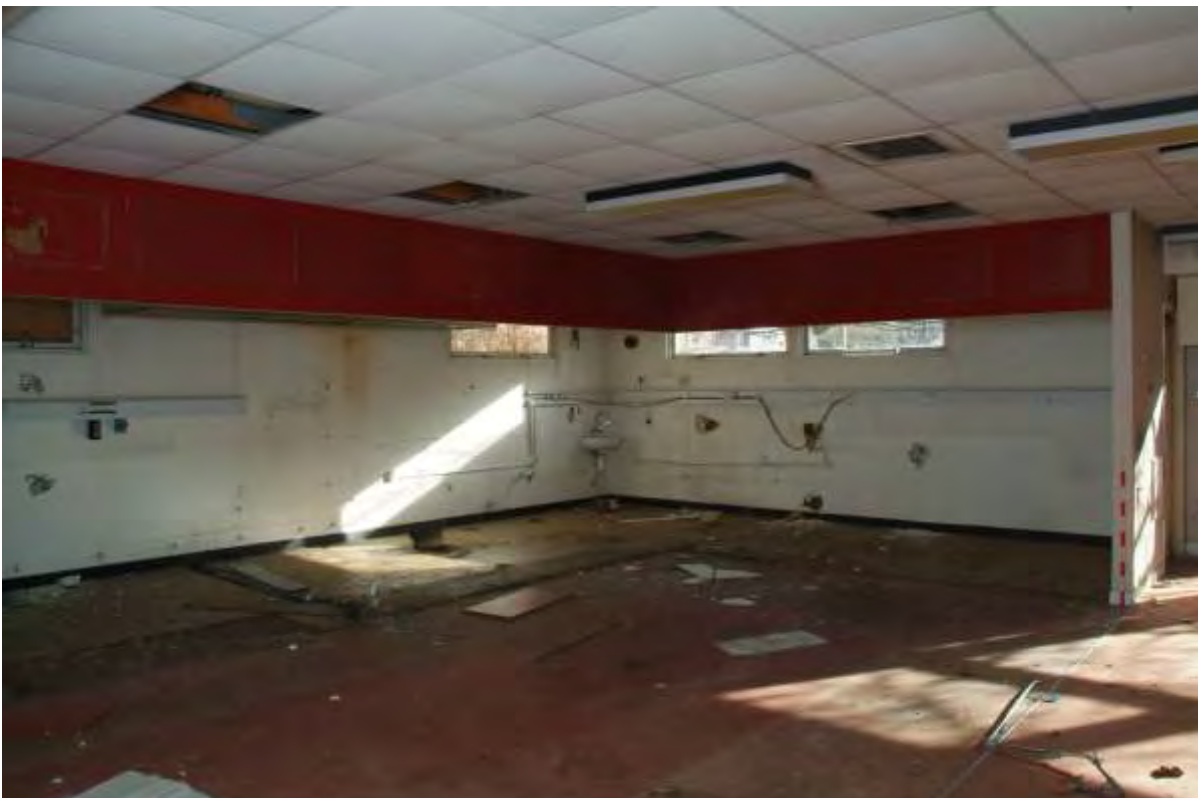
Plate 49.3: Building 49 – interior of northern dining area, view to the southwest
