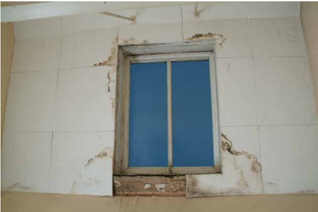
Plate 14.24: Building 14 – detail of historic roof light, view up
