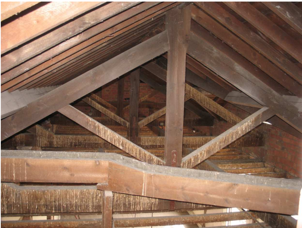
Plate 43.74: Building 43 – roof space: typical roof truss, view to the north
