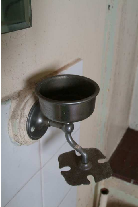
Plate 27.39: Building 27a - second floor: detail of original toothbrush holder, view to the west
