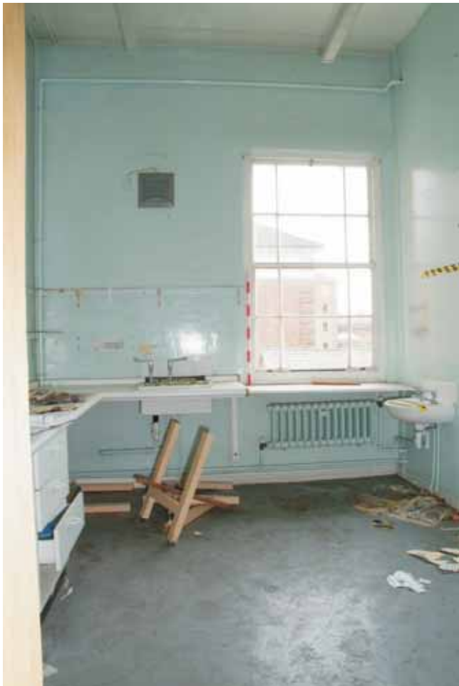
Plate 16.6: Building 16 – typical first floor consulting room, view to the south
