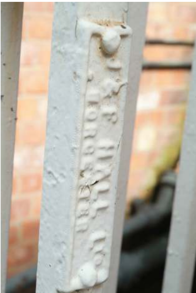
Plate 48.3: Building 48: detail of railings around stairwell to basement
