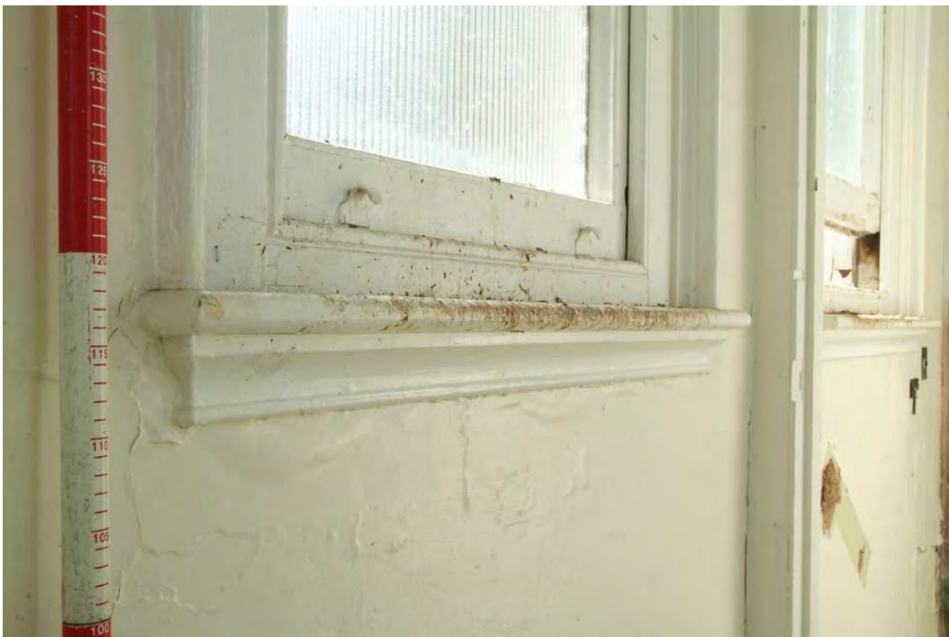
Plate 24.166: Building 24 (FF): detail of typical sill in northwest corner tower
