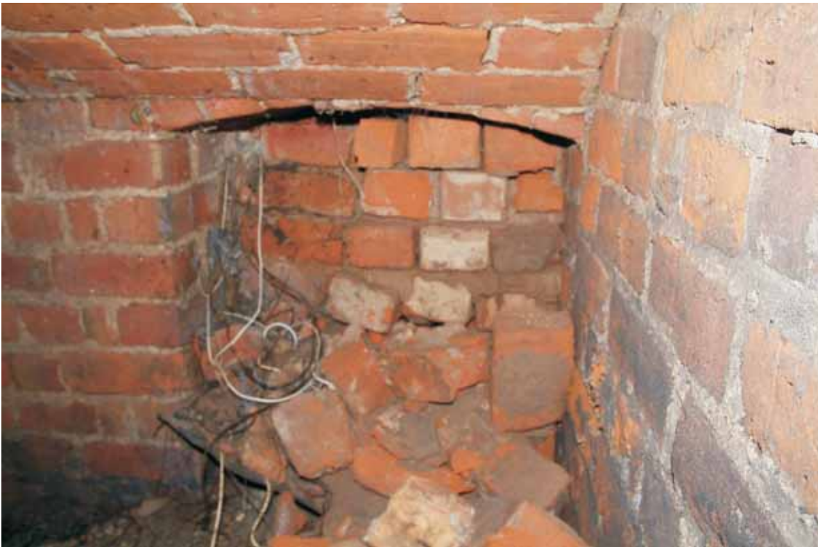
Plate 18.33: Building 18 – basement: interior showing blocked former entrance, view to the west
