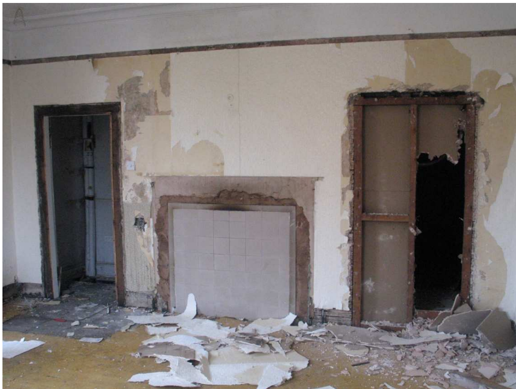
Plate 30.60: Building 30 (GF): blocked openings to former wardrobes in northeast room
