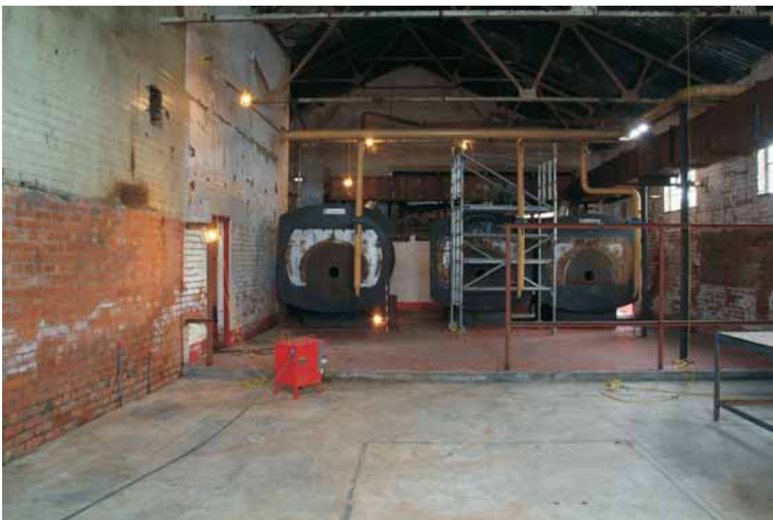
Plate 10.13: Building 10 – interior of main shed, view to the south
