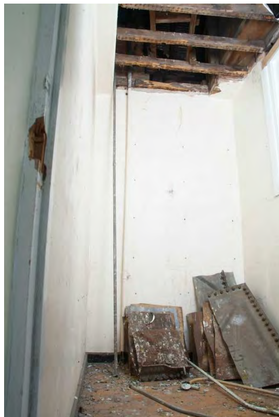
Plate 24.198: Building 24 (SF): closet wing in original form, view to the east
