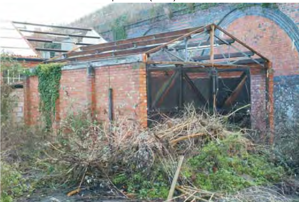
Plate 1.1: Building 1 – northern and western elevations
