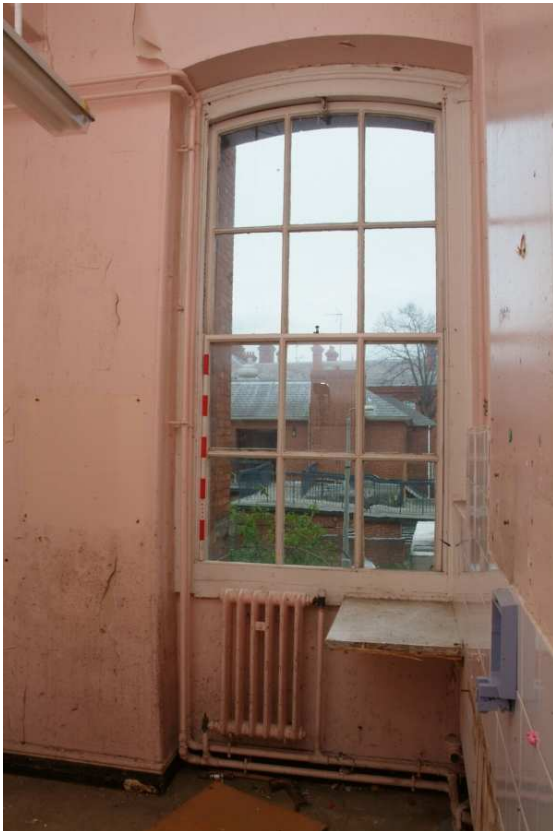
Plate 24.57: Building 24: Room 1.18, view to the east
