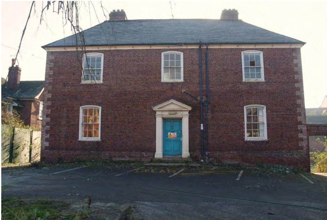
Plate 30.1: Building 30: northern elevation
