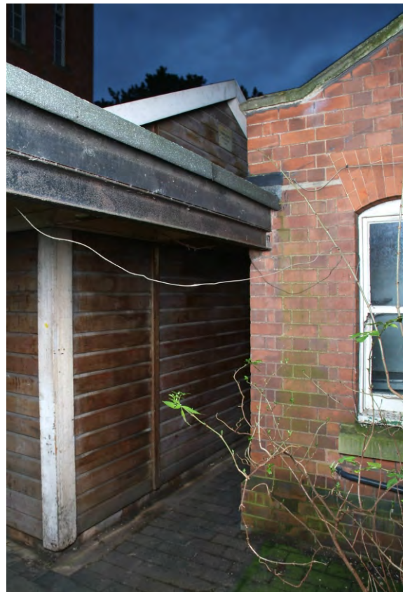
Plate 37.4: Building 37 – south elevation, view to the northeast
