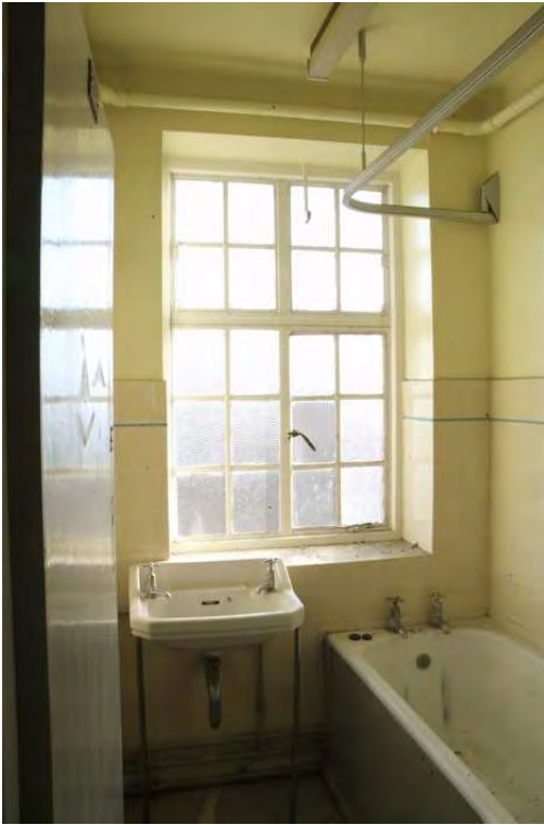
Plate 27.73: Building 27b – second floor: original bathroom, view to the north
