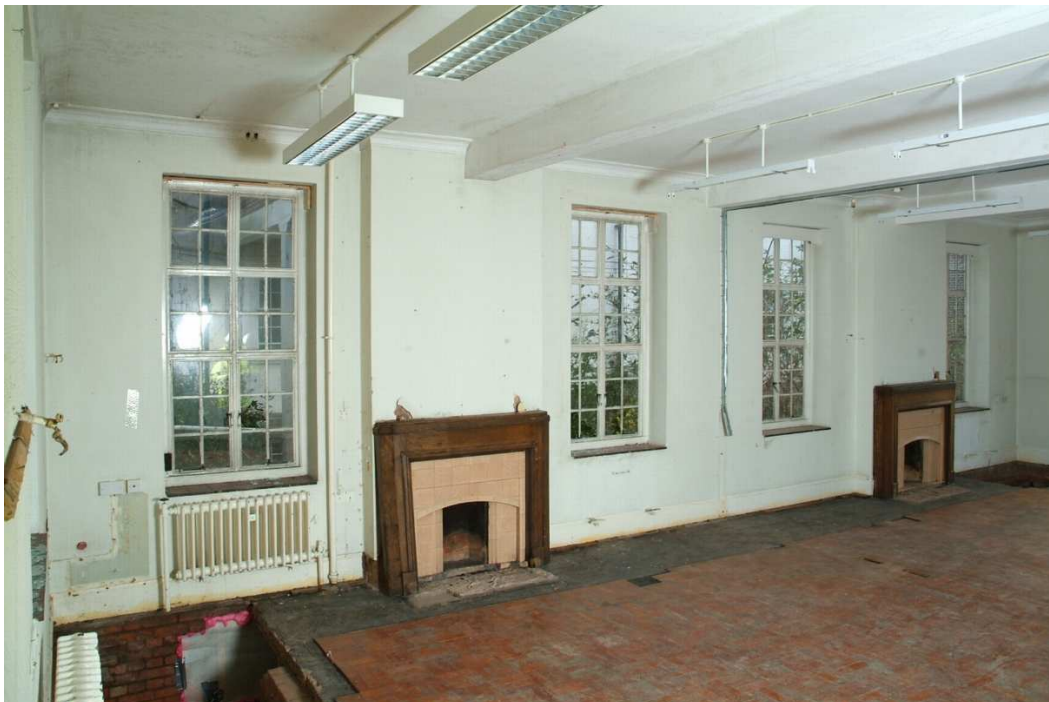
Plate 27.24: Building 27a – ground floor: nurses' sitting room, view to the southwest
