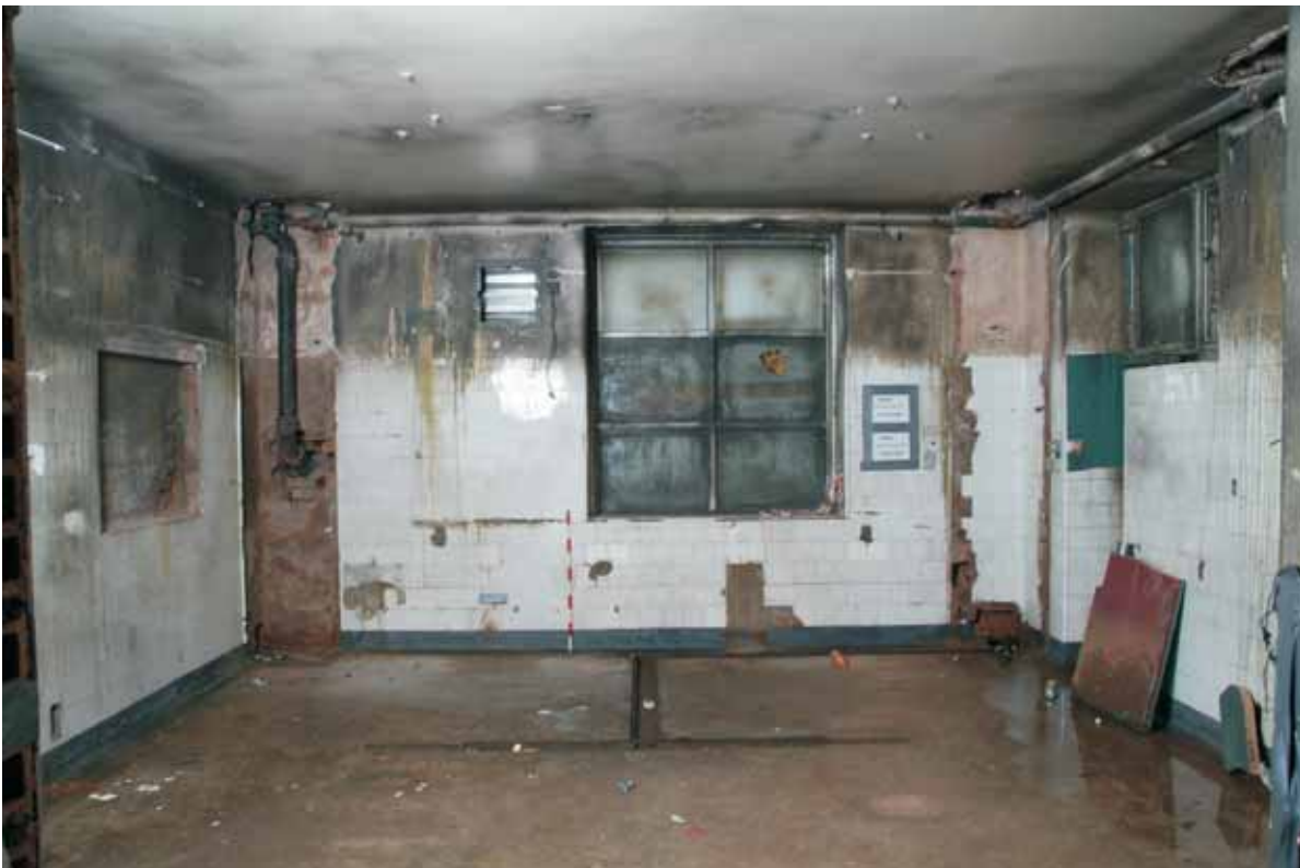
Plate 17.18: Building 17a – basement: tiled post mortem room, view to the south
