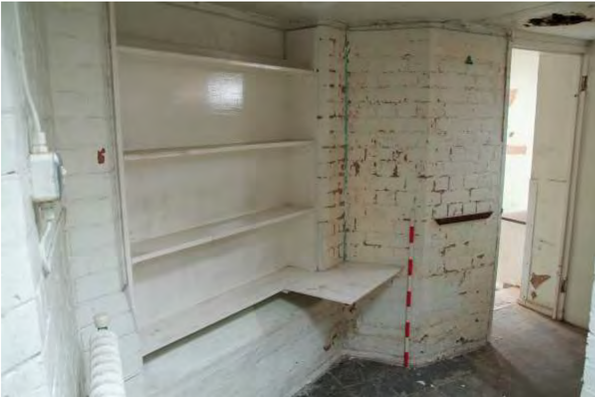
Plate 48.8: Building 48: access to northern part, view to the southwest
