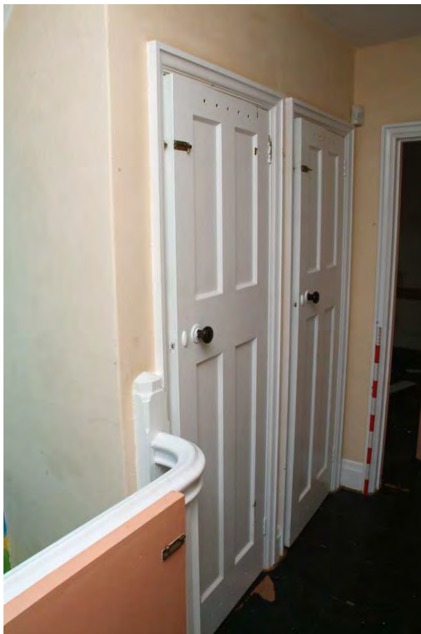
Plate 31.18: Building 31: first floor landing, view to the southeast
