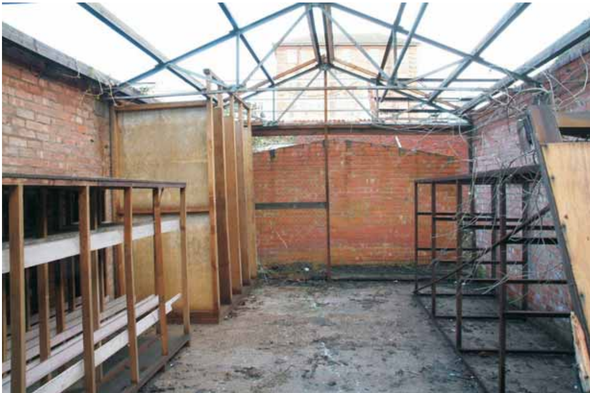
Plate 1.5: Building 1 – interior, view to the southwest
