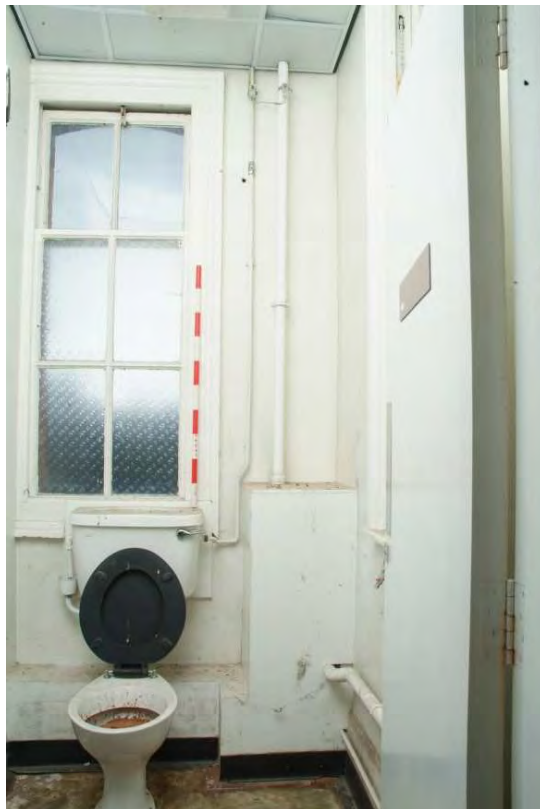
Plate 24.210: Building 24 (SF): interior of southeast corner tower, view to the south
