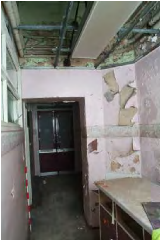
Plate 41.24: Building 41 – corridor along south, view to the east
