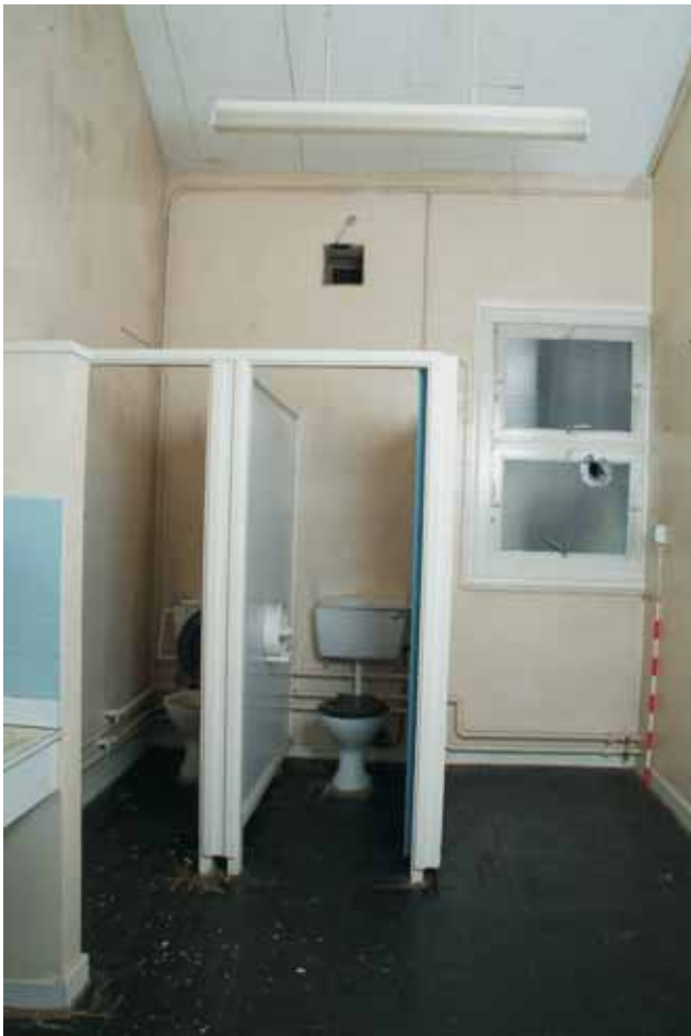
Plate 14.11: Building 14 – female WC, view to the east
