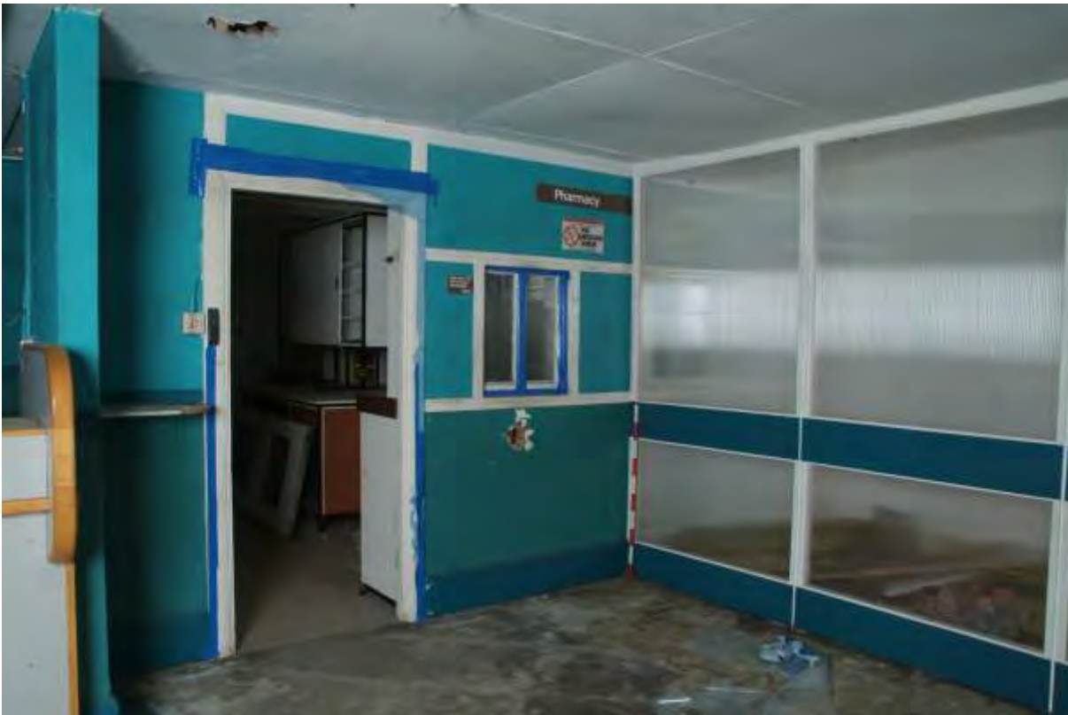
Plate 41.20: Building 41 – ground floor - dispensary counter, view to the west
