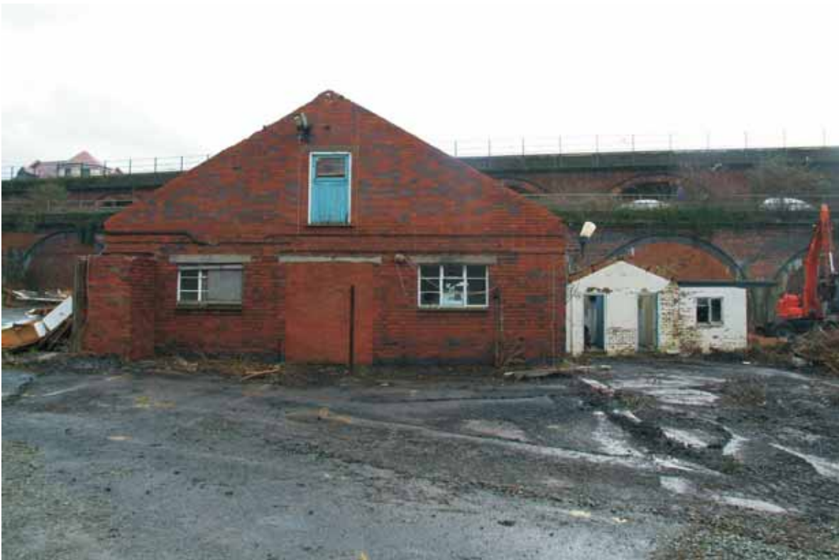
Plate 6.2: Building 6 – northern elevation
