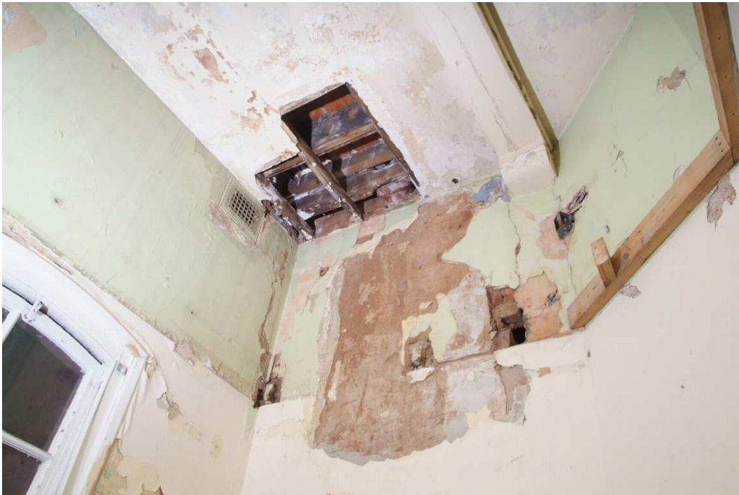
Plate 24.81: Building 24: Wheeley Lea Ward [Room 1.35], view up and to the east
