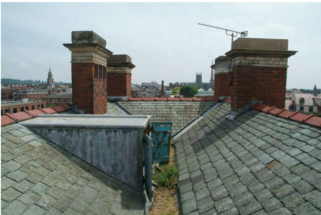
Plate 43.2: Building 43 – roof, view to the south
