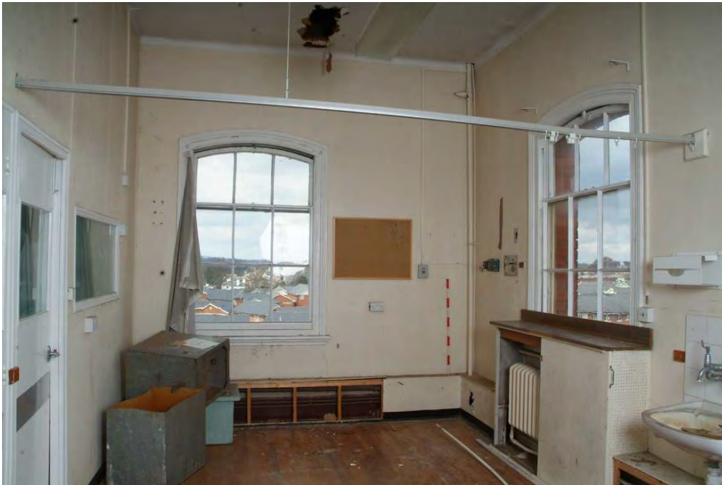
Plate 24.195: Building 24 (SF): easternmost area of Maddox Ward, view to the north
