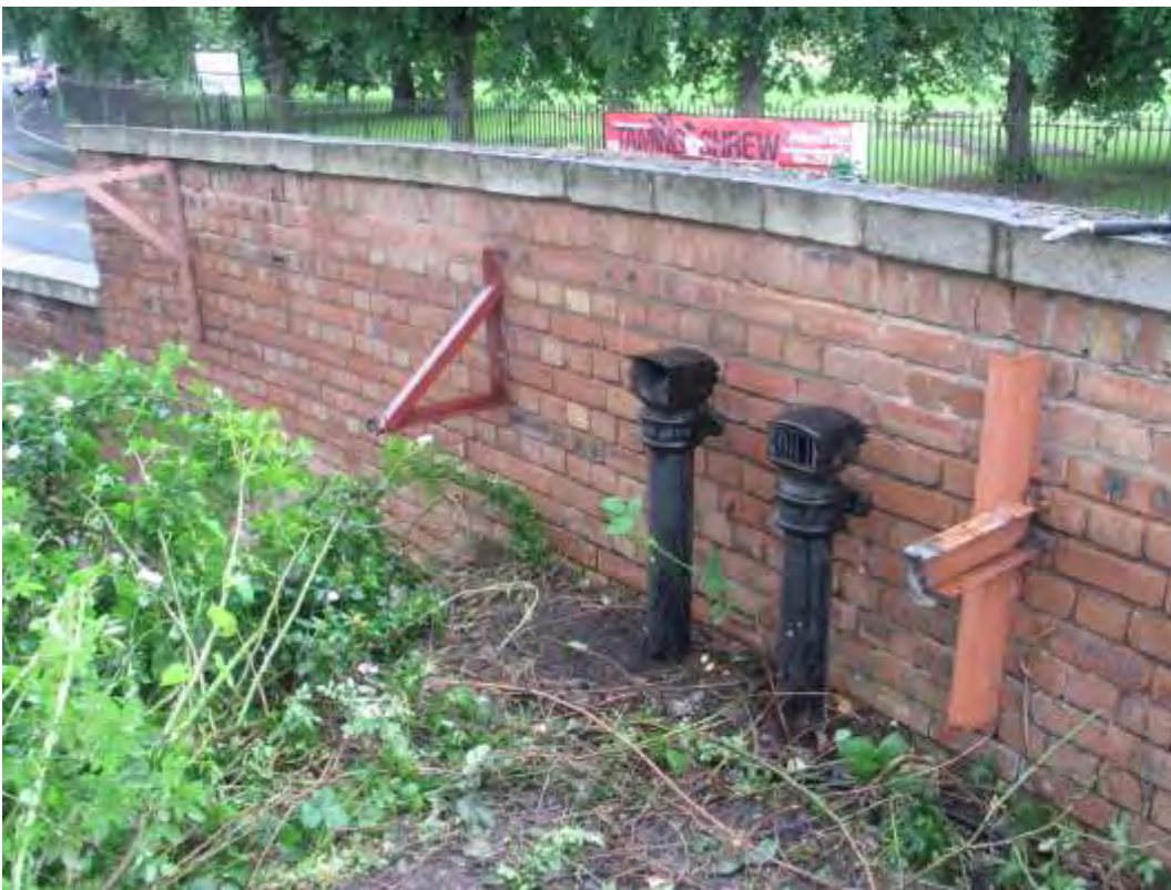
Plate 47.13: Building 47: hospital elevation 04
