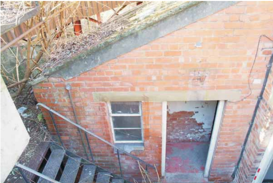
Plate 10.2: Building 10 – southern end of the eastern elevation, view to the east
