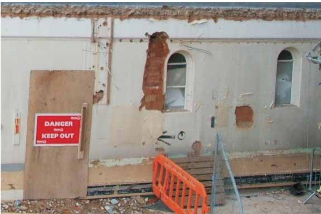
Plate 22.12: Building 22 – original basement windows in southern elevation, view to the northeast
