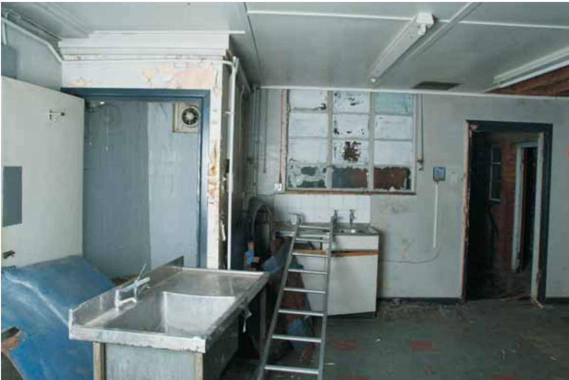
Plate 10.20: Building 10 – interior of mess room in eastern range, view to the south
