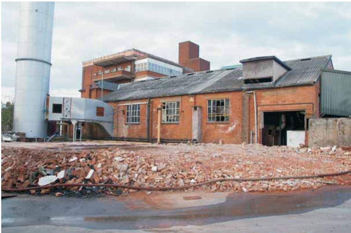
Plate 10.7: Building 10 – western elevation following the demolition of Building 7
