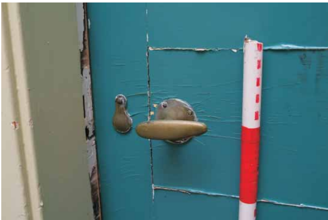
Plate 22.8: Building 22 – upper ground floor: detail of early 20th century fittings on modified original door, view to the northwest
