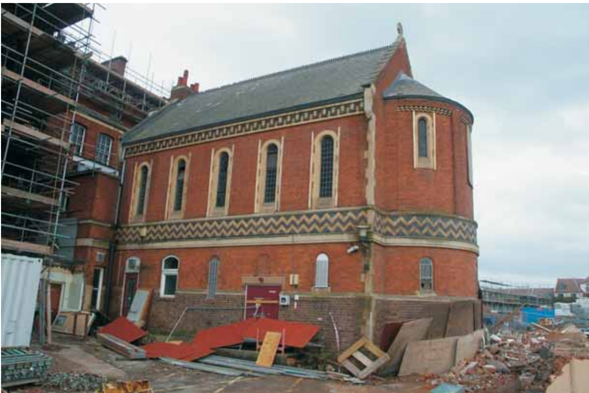
Plate 22.2: Building 22 – northern elevation
