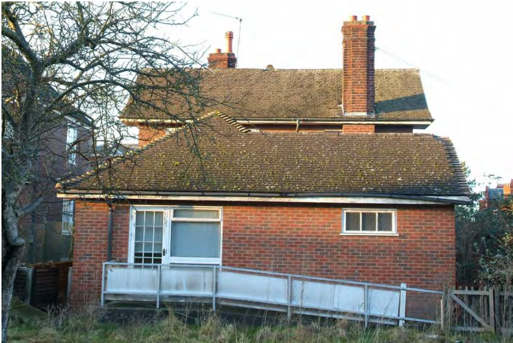
Plate 31.9: Building 31: southern elevation, view to the north
