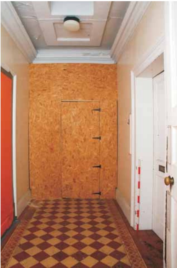
Plate 22.35: Building 22 – connecting range: central corridor on upper ground floor, view to the west
