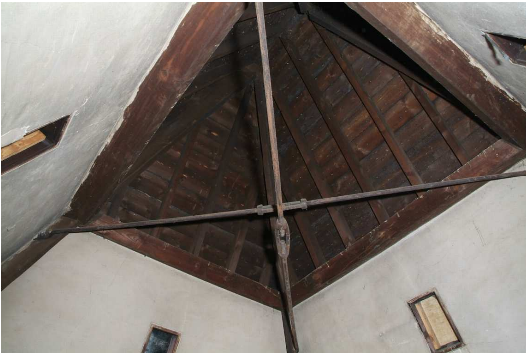
Plate 24.212: Building 24 (SF): structure of roof apex over southeast corner tower
