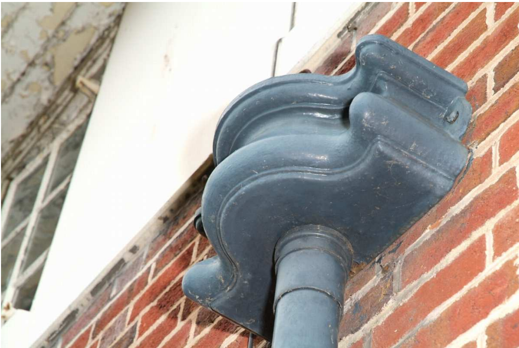
Plate 27.12: Building 27a - detail of typical rainwater head, view to the southwest
