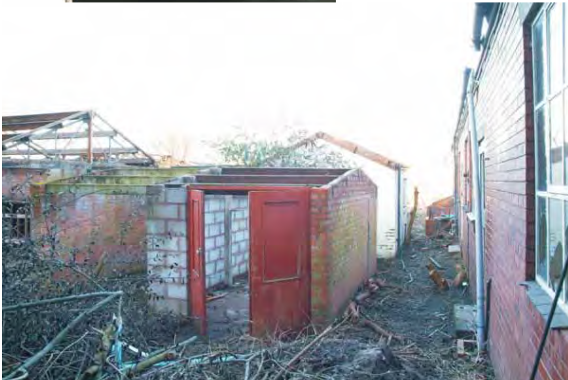
Plate 4.1: Building 4 – southern and eastern elevations
