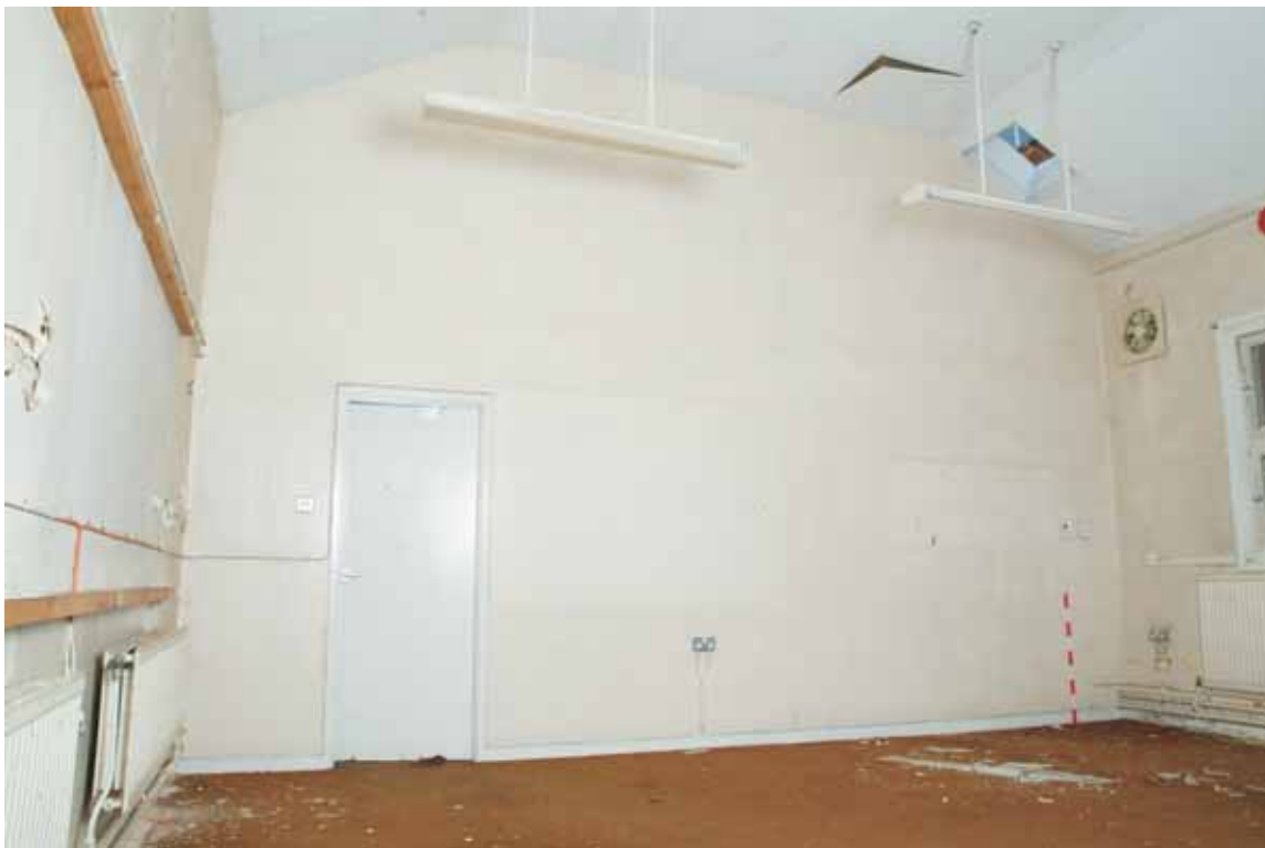
Plate 14.12: Building 14 – western seminar room, view to the northwest
