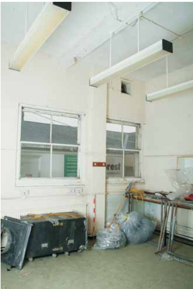
Plate 16.5: Building 16 – typical ground floor room, view to the northeast
