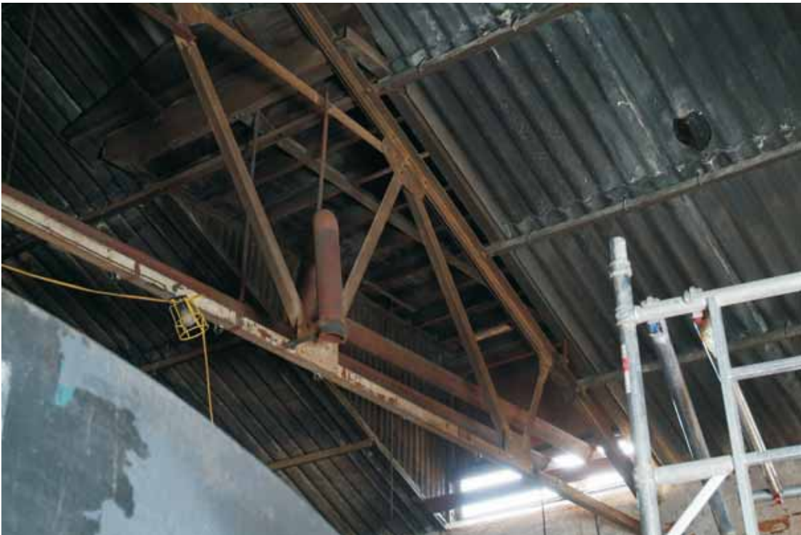
Plate 10.16: Building 10 – detail of roof trusses
