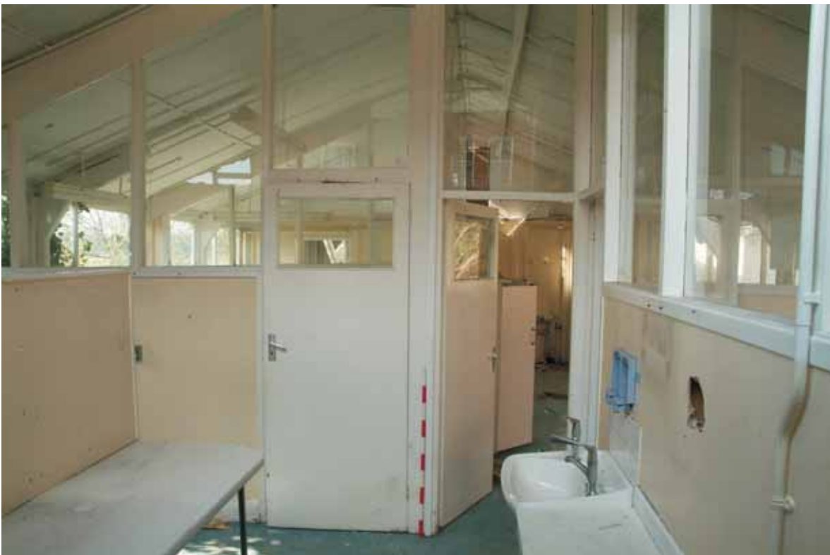
Plate 20.4: Building 20 – Interior of southern hut showing half glazed partitions, view to the north
