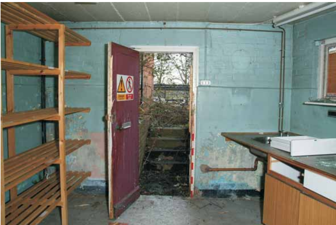
Plate 13.5: Building 13 – interior of basement, view to the west
