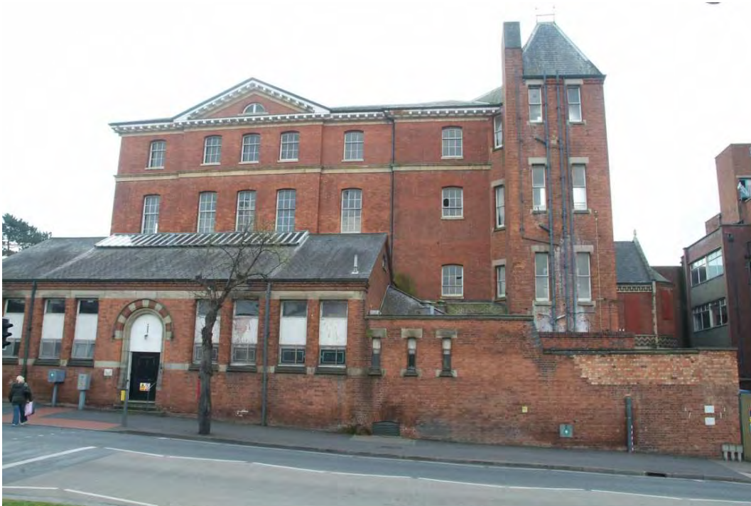
Plate 24.17: Building 24: north elevation above Building 40
