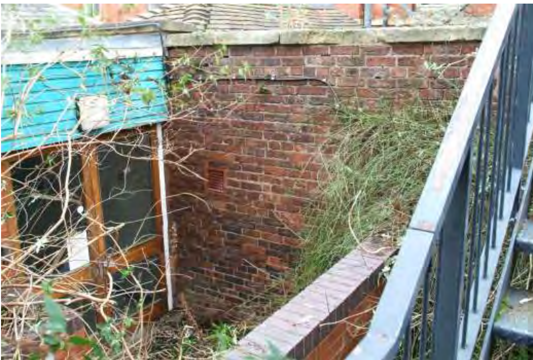
Plate 36.6: Building 36 – westernmost part of southern elevation, view to the northwest
