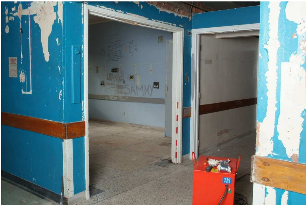
Plate 26.8: Building 26: typical level of survival of fittings, view to the northwest
