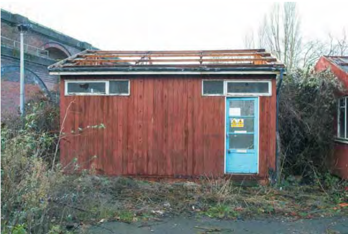
Plate 2.3: Building 2 – eastern elevation
