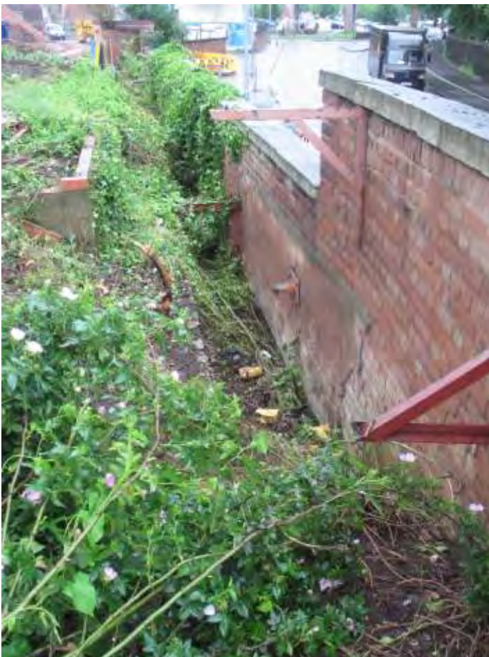
Plate 47.14: Building 47: hospital elevation 05
