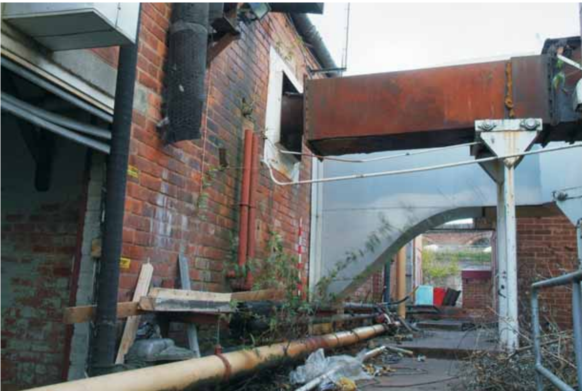
Plate 10.6: Building 10 – western elevation
