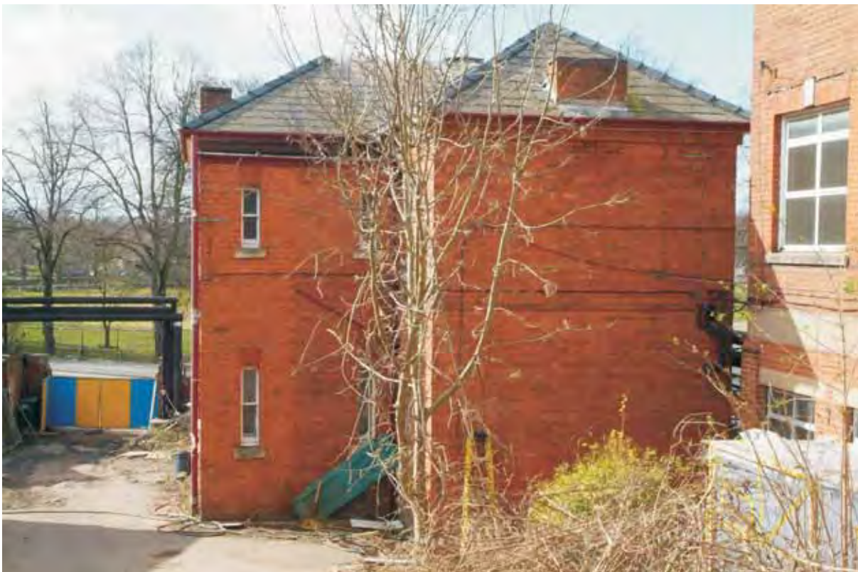
Plate 18.4: Building 18 – east elevation
