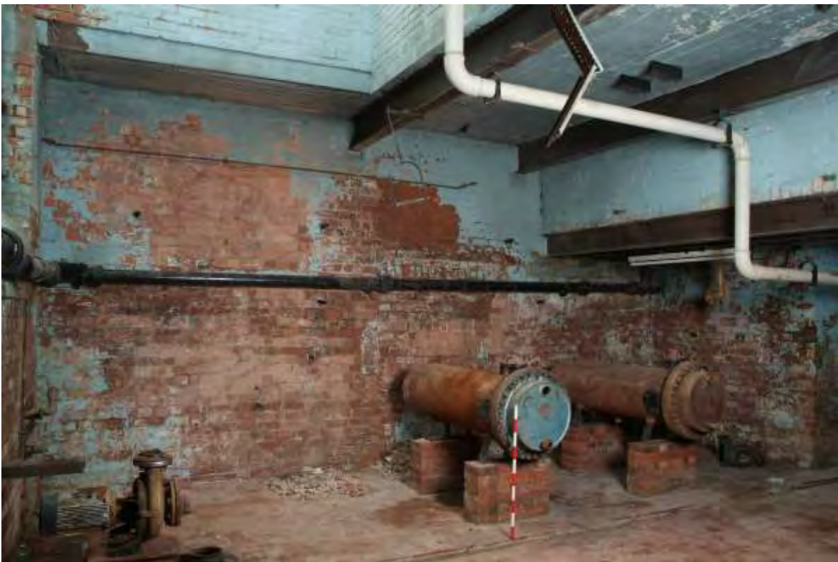
Plate 48.10: Building 48: basement –internal north wall, view to the northeast
