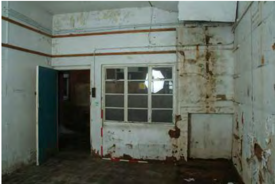
Plate 33.9: Building 33 – interior of northern part, view to the north
