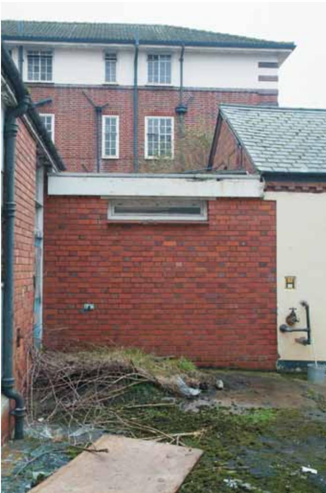
Plate 15.6: Building 15a –northern elevation
