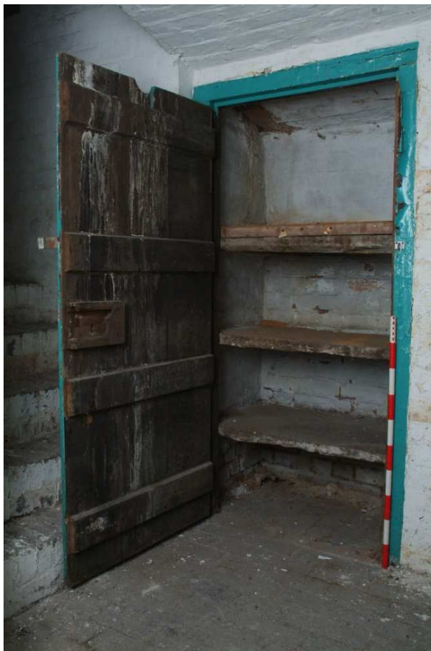
Plate 24.126: Building 24 (basement): detail of cupboard door, view to the northeast
