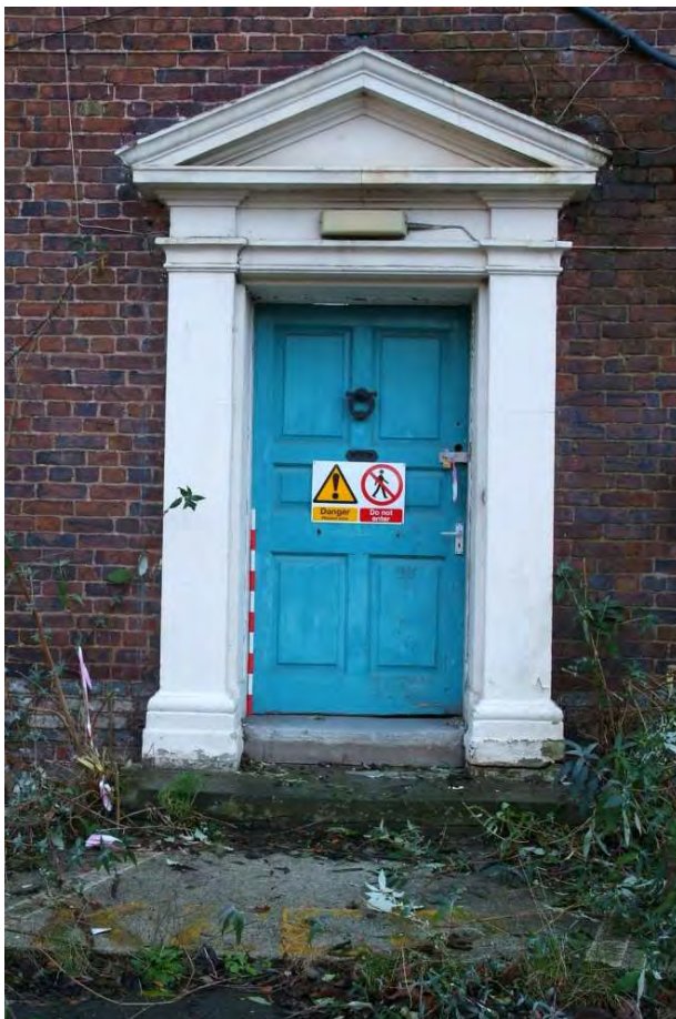
Plate 30.2: Building 30: doorcase to principal (front) entrance, view to the south
