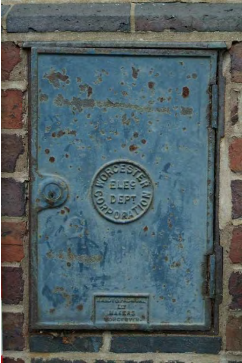
Plate 39.3: Building 39 – detail of 'Hardy and Padmore' electricity box cover, view to the south
