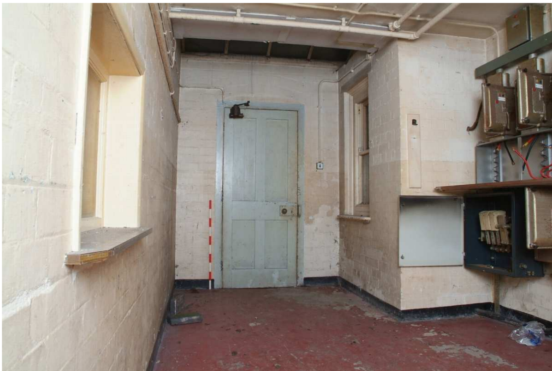
Plate 43.42: Building 43 – basement: entrance hall, view to the north
