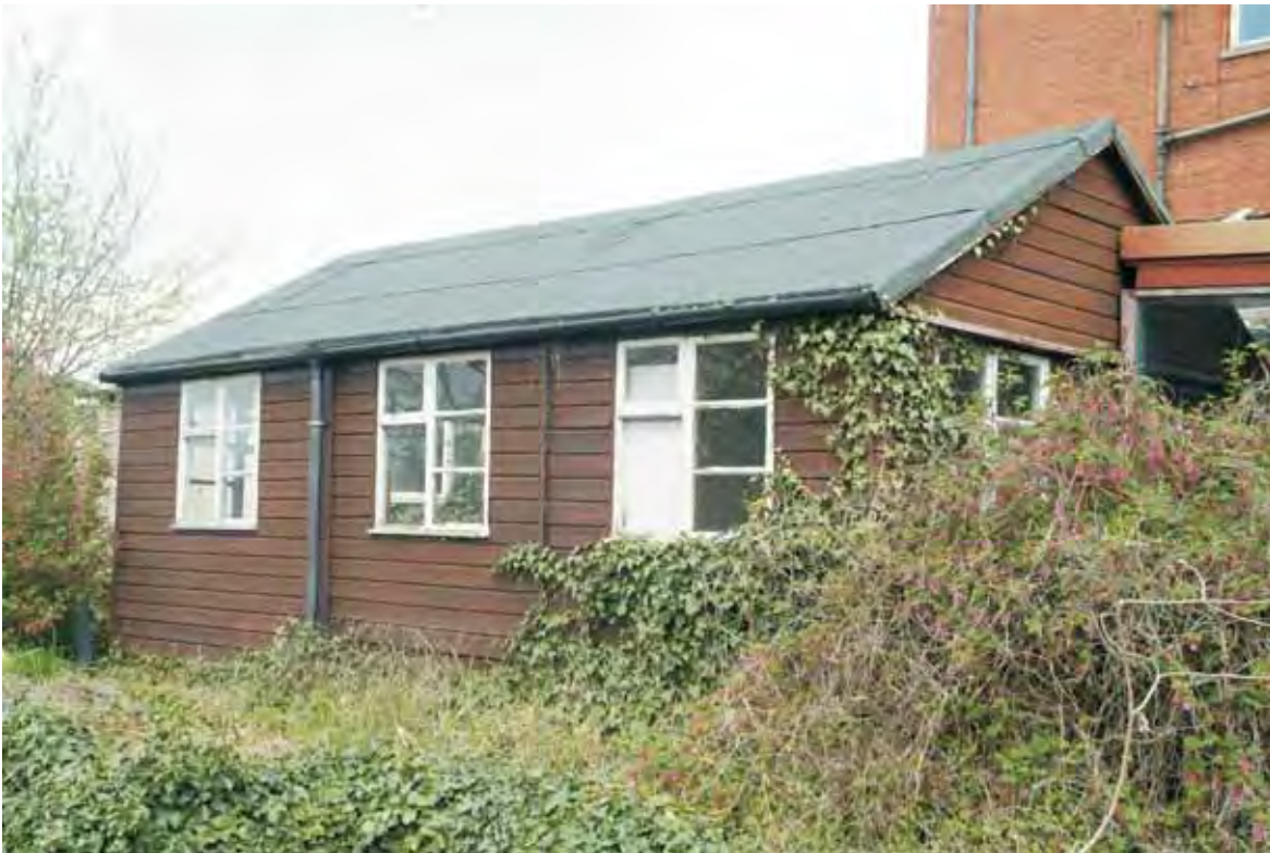
Plate 21.1: Building 21 – south and west elevations
