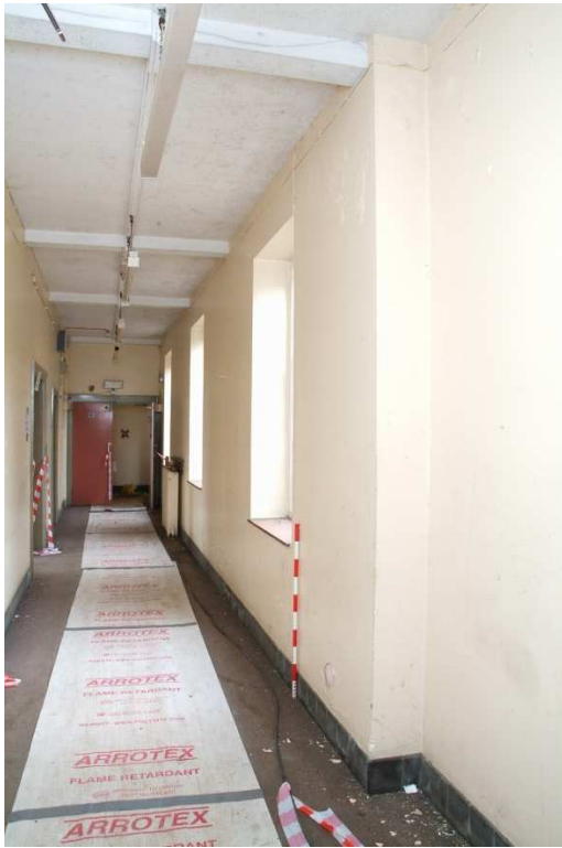
Plate 27.13: Building 27a – ground floor: principal corridor, view to the north
