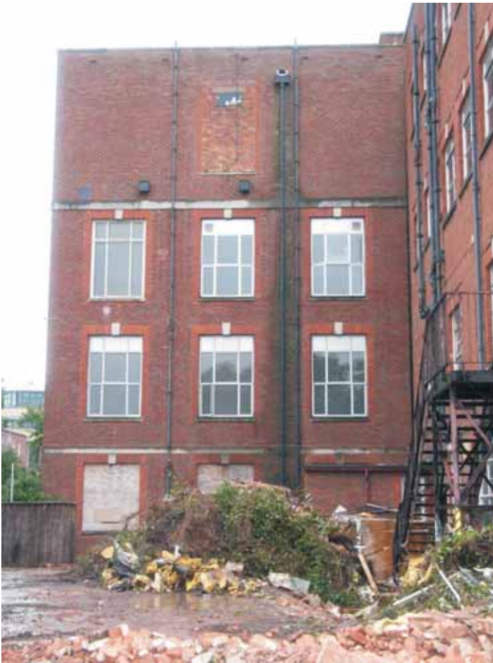
Plate 17.3: Building 17a – west elevation
