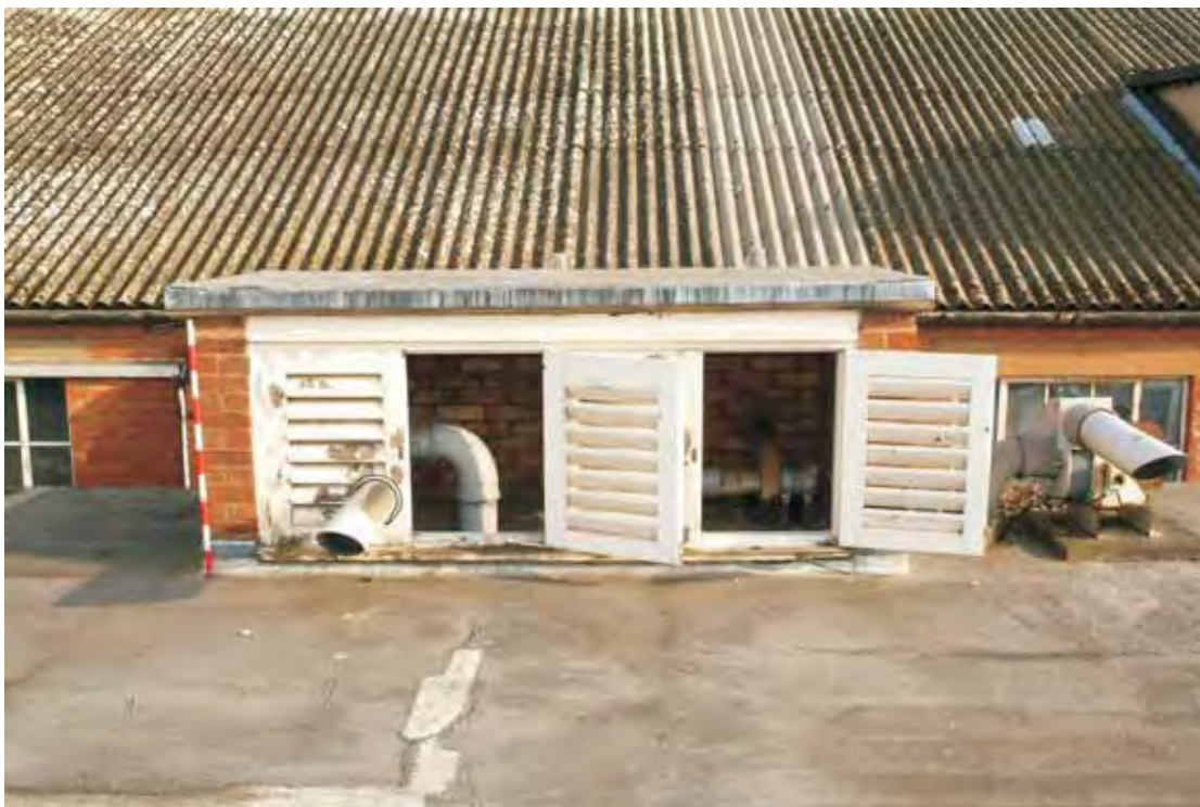
Plate 7.7: Building 7 – plant room on roof, view to the east
