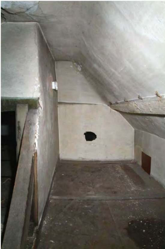
Plate 30.51: Building 30 (attic floor): interior of former store room, view to the west
