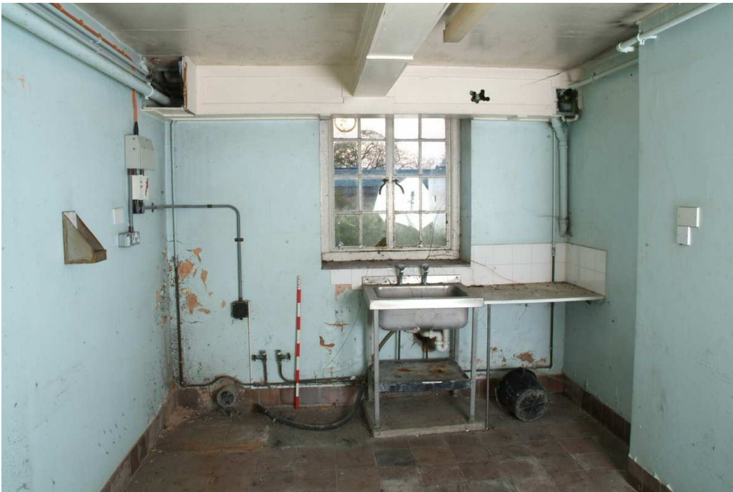
Plate 27.30: Building 27a - basement: former domestic laundry room, view to the west
