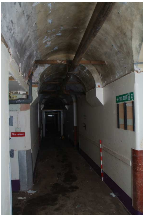
Plate 24.93: Building 24 (LGF): central corridor [Room 90] central section, view to the north
