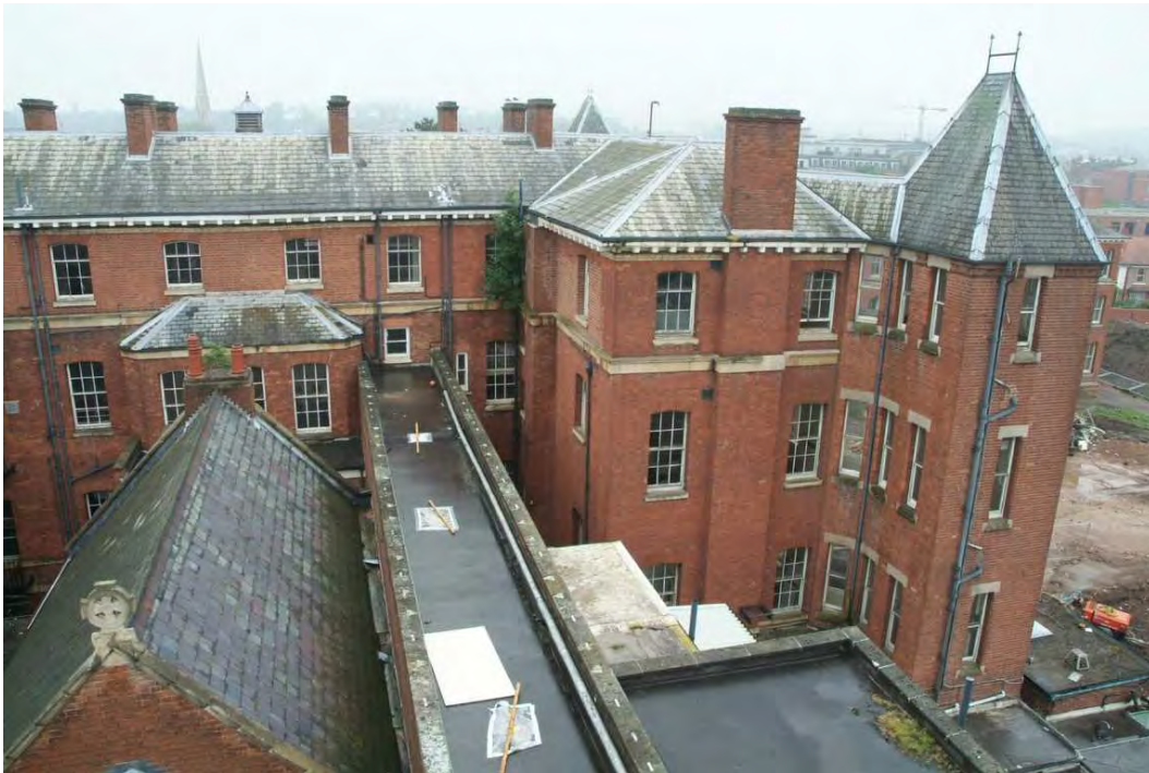
Plate 24.25: Building 24: southwest wing, view to the southeast
