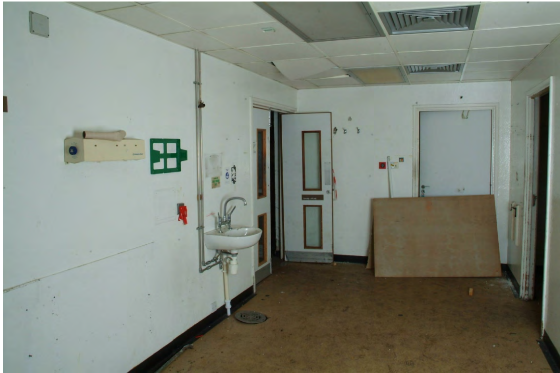
Plate 32.5: Building 32: plating room, view to the west
