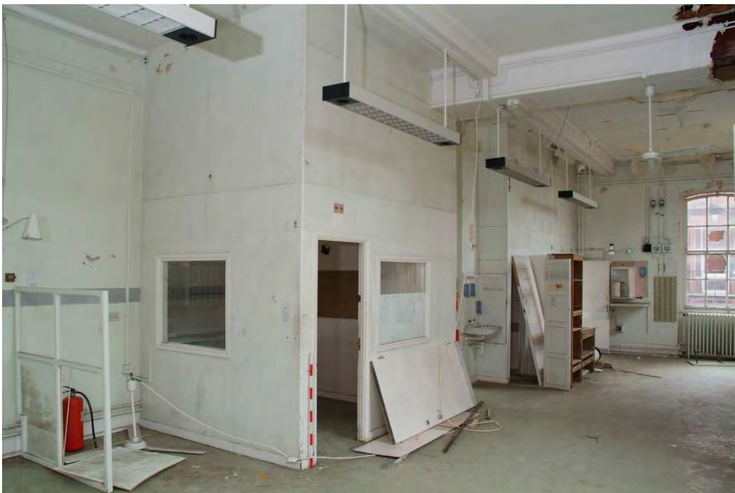
Plate 24.62: Building 24: Rushout Ward [Room 1.11] view to the southwest
