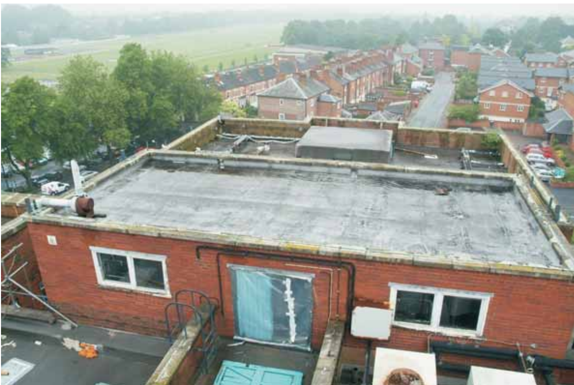
Plate 17.4: Building 17a – roof, view to the northwest
