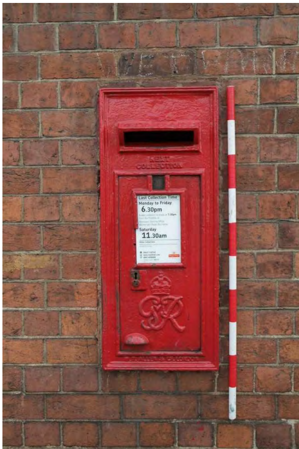
Plate 41.4: Building 41: detail of George VI post box in northern elevation
