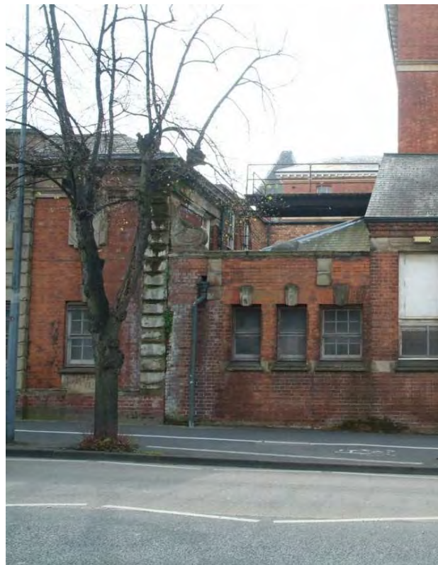
Plate 40.6: Building 40: right hand flanking wing of north elevation, view to the southeast
