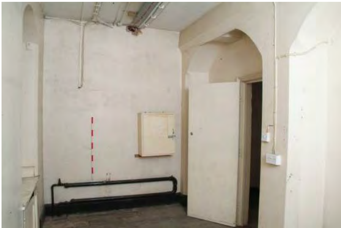
Plate 22.60: Building 22 (LGF): interior of 'Porter's Rest Room' view to the west
