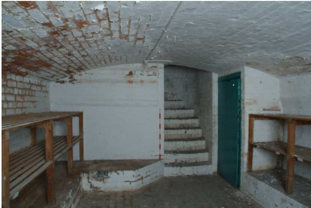
Plate 24.125: Building 24 (basement): interior showing stairs and cupboard
