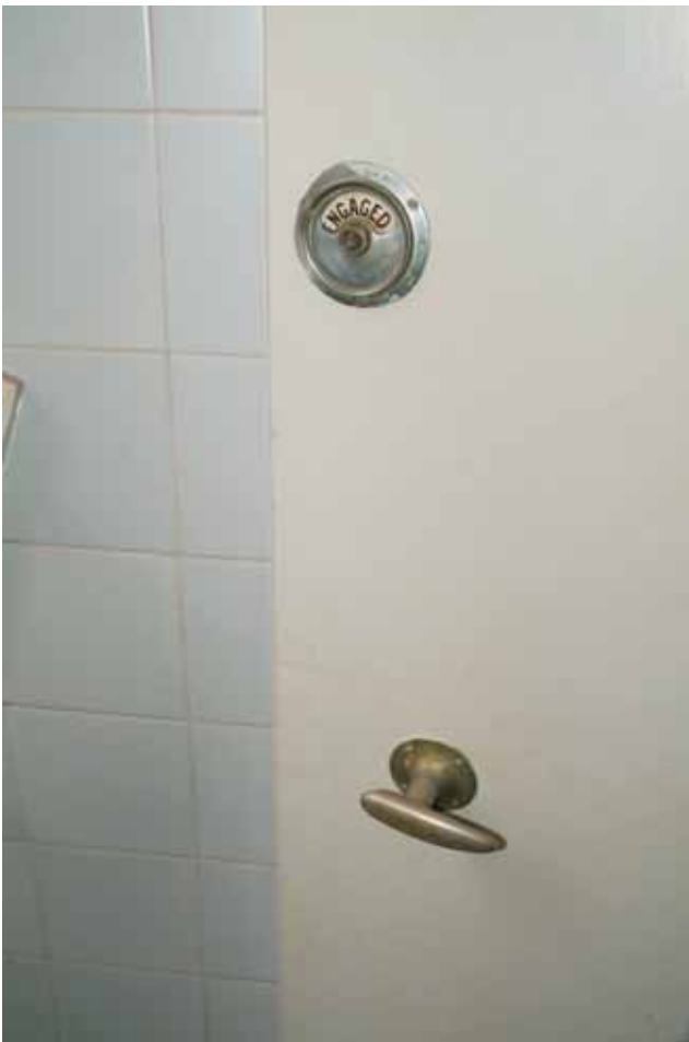
Plate 17.27: Building 17a – ground floor: detail of original door fittings
