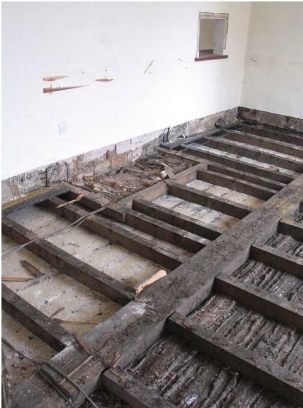
Plate 30.59: Building 30 (GF): exposed floor structure in northwest room
