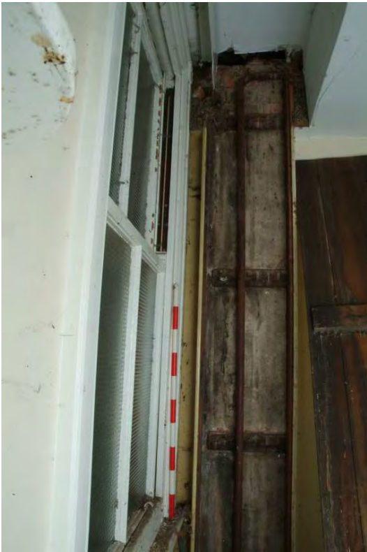
Plate 43.71: Building 43 - second floor: detail of pipe box, view to the south
