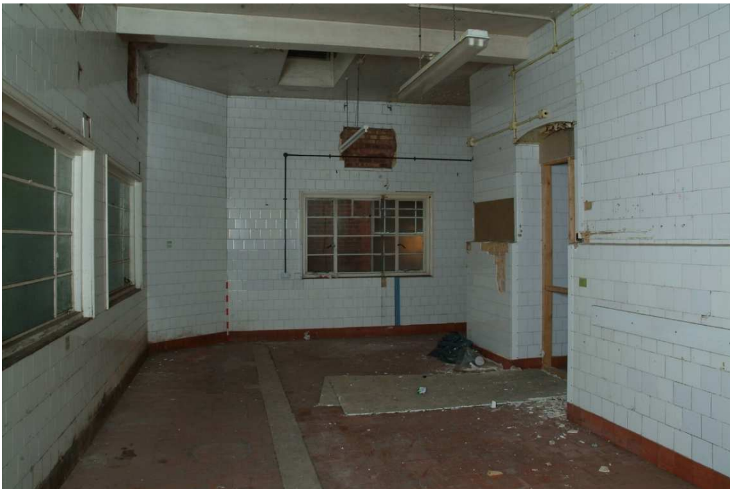
Plate 24.120: Building 24 (LGF): 1920s extension to main kitchens, view to the north
