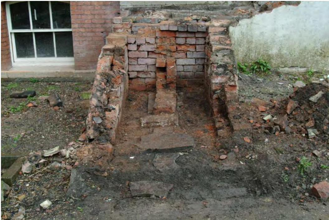
Plate 24.7: Building 24: detail showing structure of tread supports, view to the west
