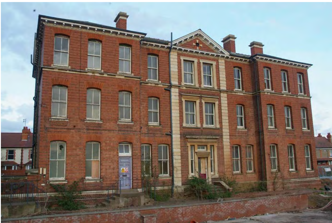
Plate 43.14: Building 43 – western elevation
