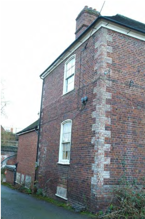
Plate 30.11: Building 30: eastern elevation, view to the southwest
