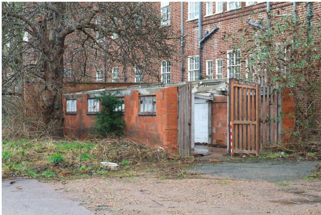
Plate 28.1: Building 28: south and east elevations
