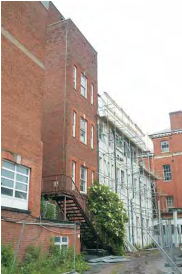
Plate 16.2: Building 16 – southern and eastern elevations
