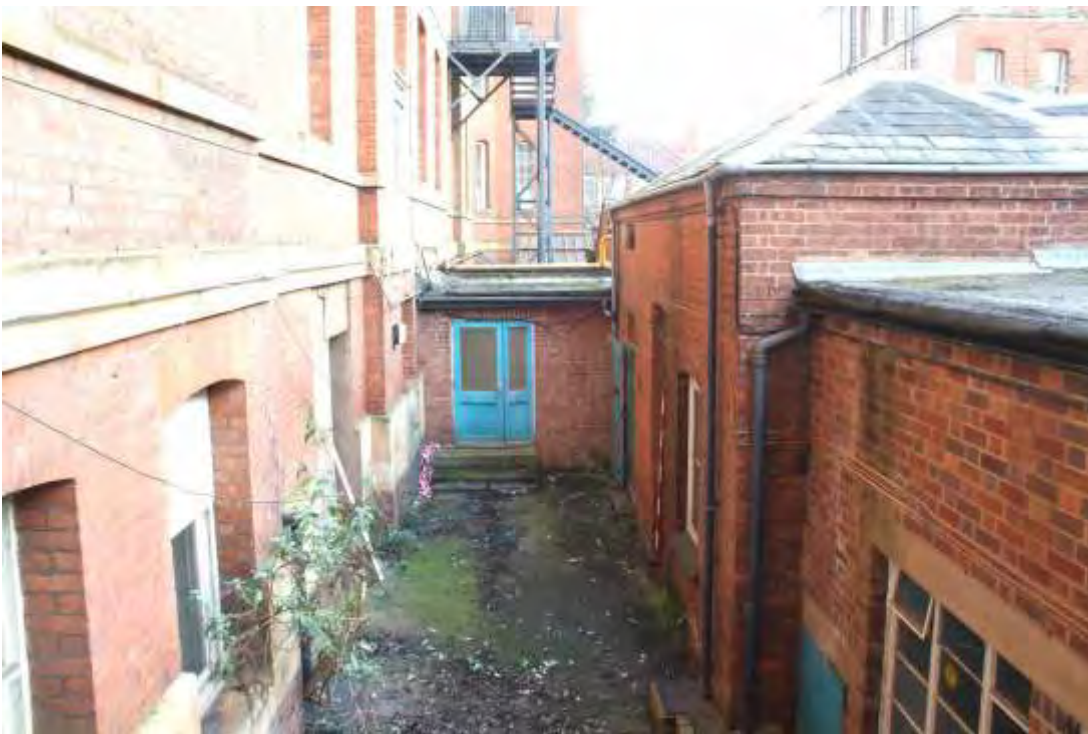
Plate 34.1: Building 34 – North elevation, view to the southeast
