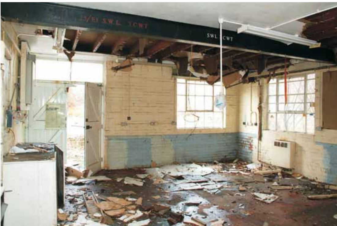
Plate 6.8: Building 6 – interior of southern extension, view to the east
