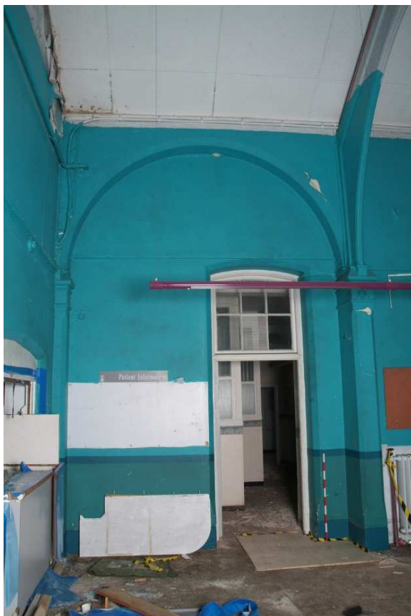
Plate 41.10: Building 41: entrance to the dermatology department, view to the south
