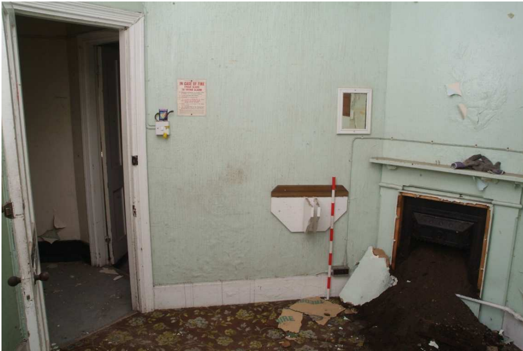
Plate 24.105: Building 24 (LGF): catering office [Room 108], view to the northwest
