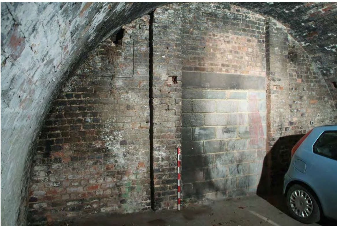
Plate 44.10: Building 44 – detail of blocking wall, view to the northeast
