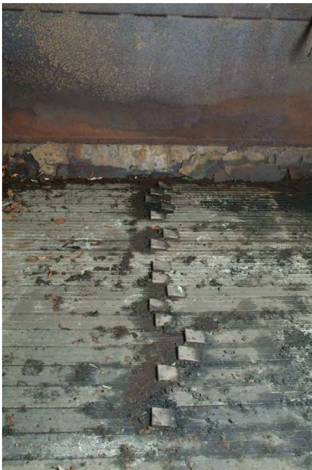
Plate 25.4: Building 25: detail of floor bars and lugs, view to the northwest
