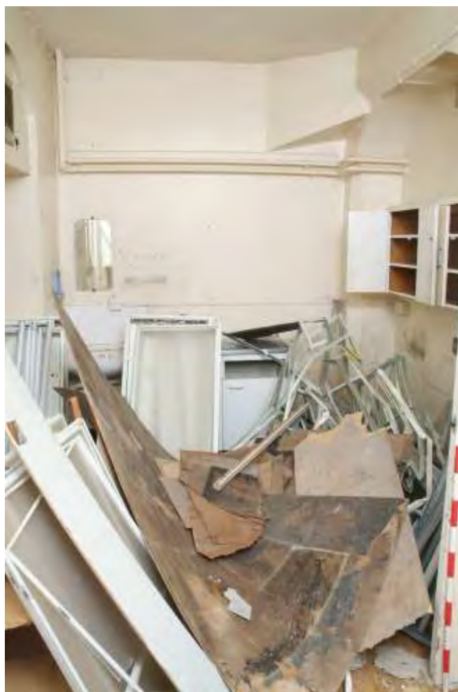
Plate 22.64: Building 22 (LGF): interior of 'Porter's Rest Room', view to the east
