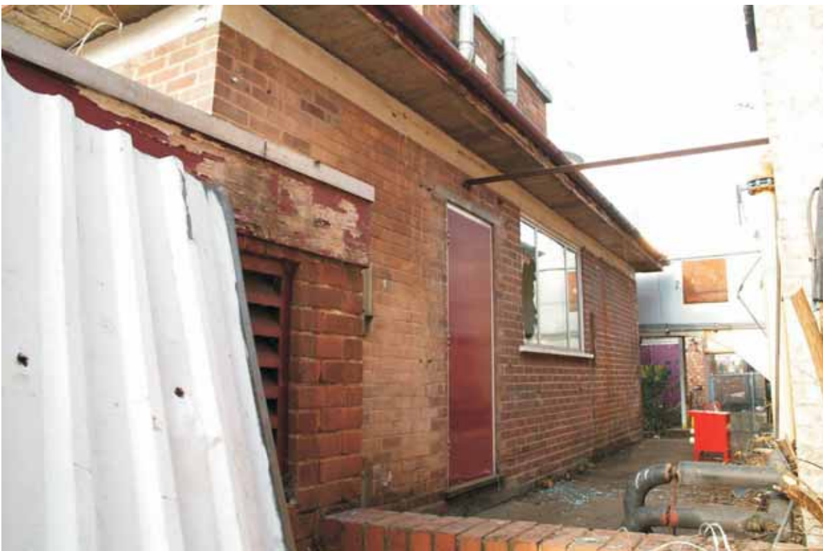
Plate 7.1: Building 7 – eastern elevation
