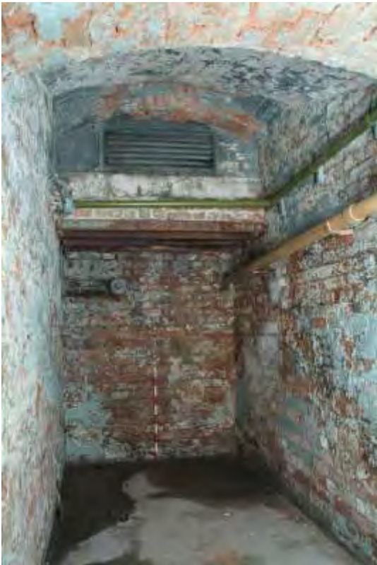
Plate 48.16: Building 48: basement – coal bunker, view to the north
