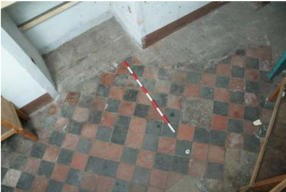
Plate 22.80: Building 22 (LGF): interior detail of historic floor tiles (re-laid)
