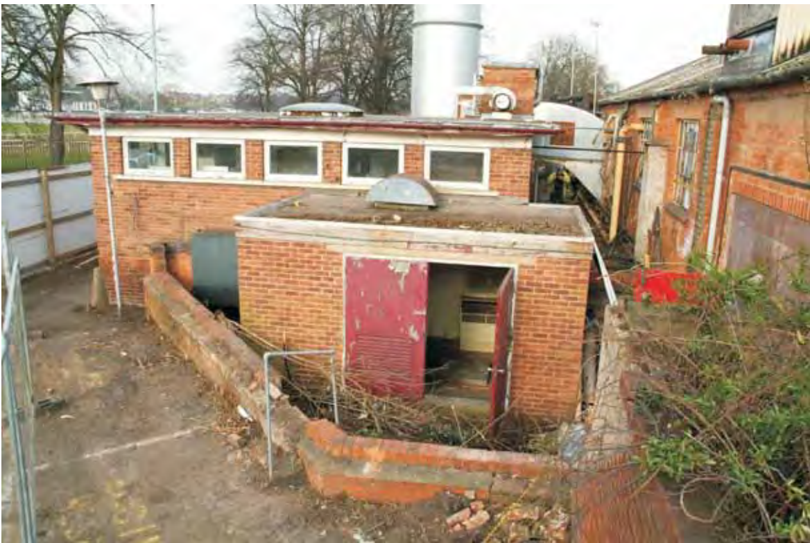
Plate 7.4: Building 7 – southern elevation showing generator room
