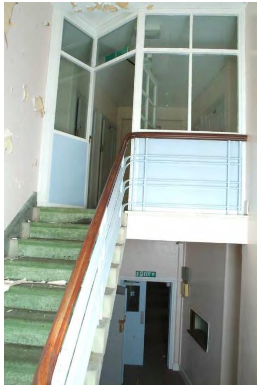
Plate 27.64: Building 27b – first floor: termination of western staircase at first floor level, view to the east
