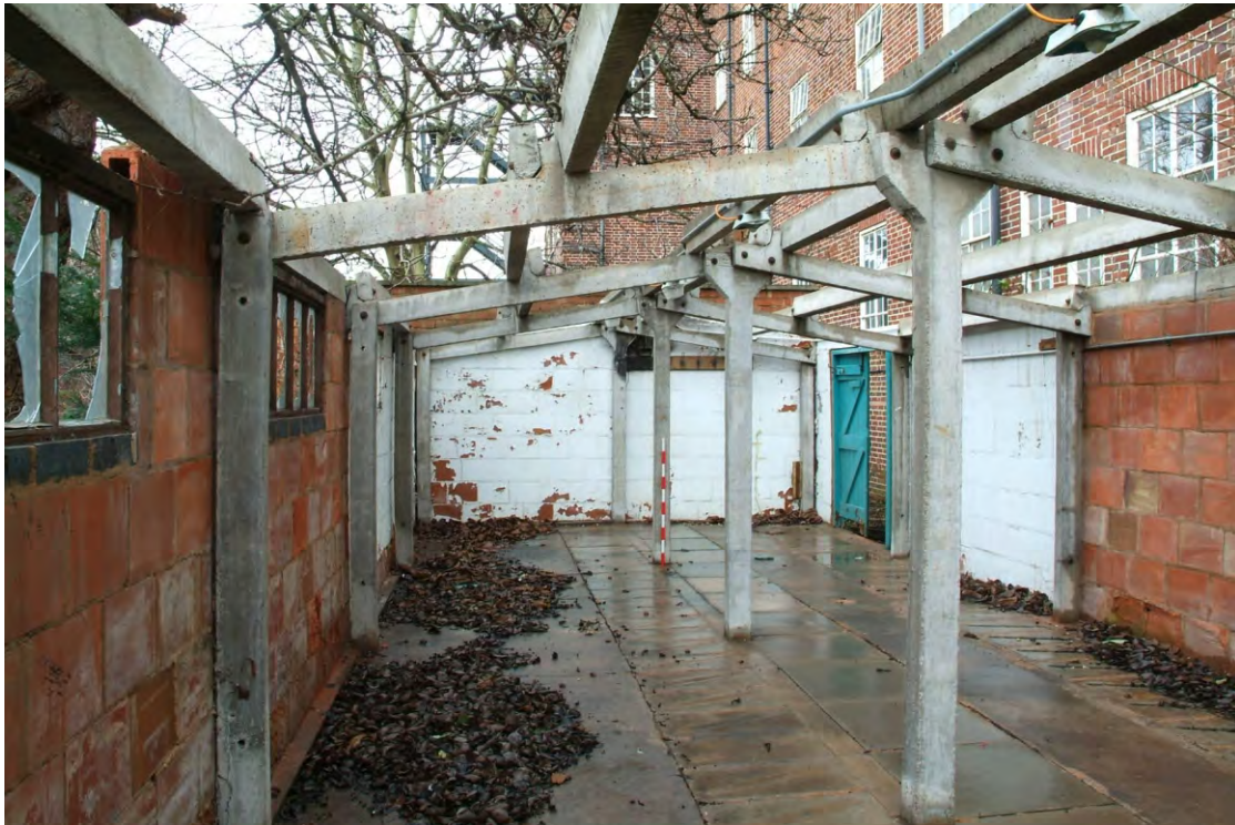
Plate 28.3: Building 28: interior, view to the west
