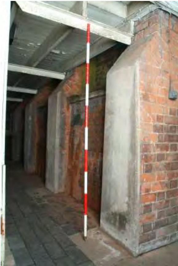
Plate 36.3: Building 36 – eastern elevation showing truncated buttresses, view to the southwest
