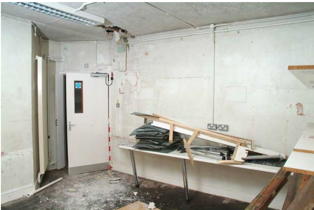
Plate 40.22: Building 40 (UGF): office [Room 1.1] at east end, view to the northwest
