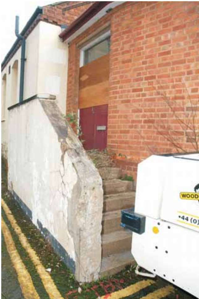
Plate 13.2: Building 13 – principal entrance on the northern elevation, view to the east
