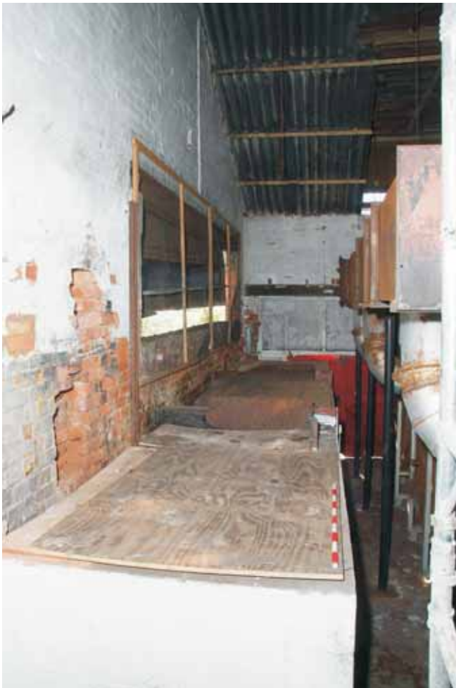
Plate 10.14: Building 10 – coal bins along the southern wall, view to the west
