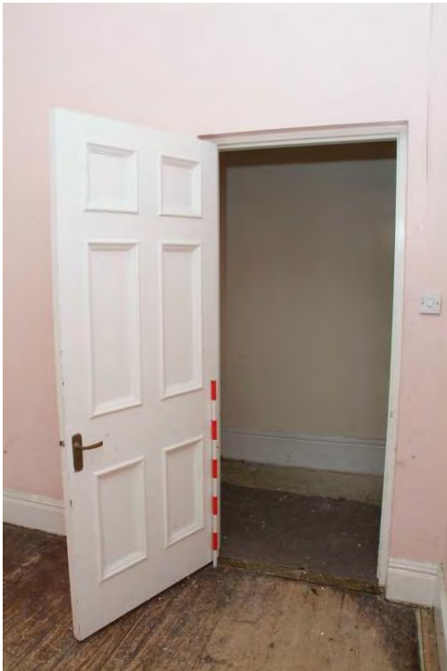
Plate 43.31: Building 43 – ground floor: inserted doorway to eastern central bedroom fitted with reproduction door, view to the south
