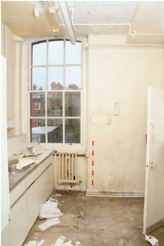
Plate 24.75: Building 24: Room 1.32, view to the southwest
