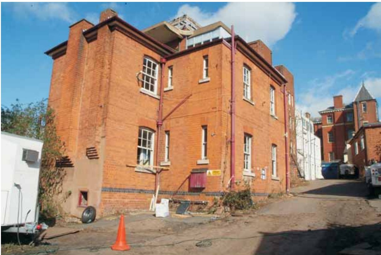
Plate 18.5: Building 18 – west and south elevation, view to the northeast
