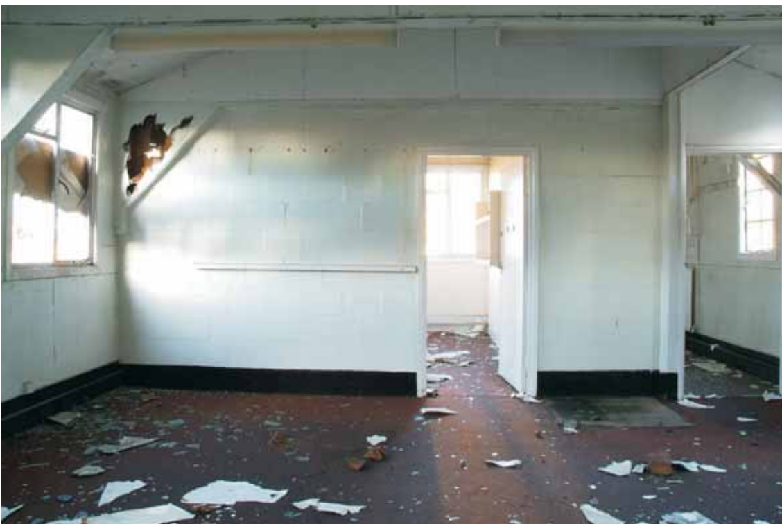
Plate 3.5: Building 3 – typical interior, view to the north
