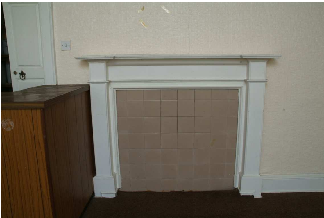
Plate 30.20: Building 30 (GF): northeast principal room showing detail of blocked fireplace, view to the south
