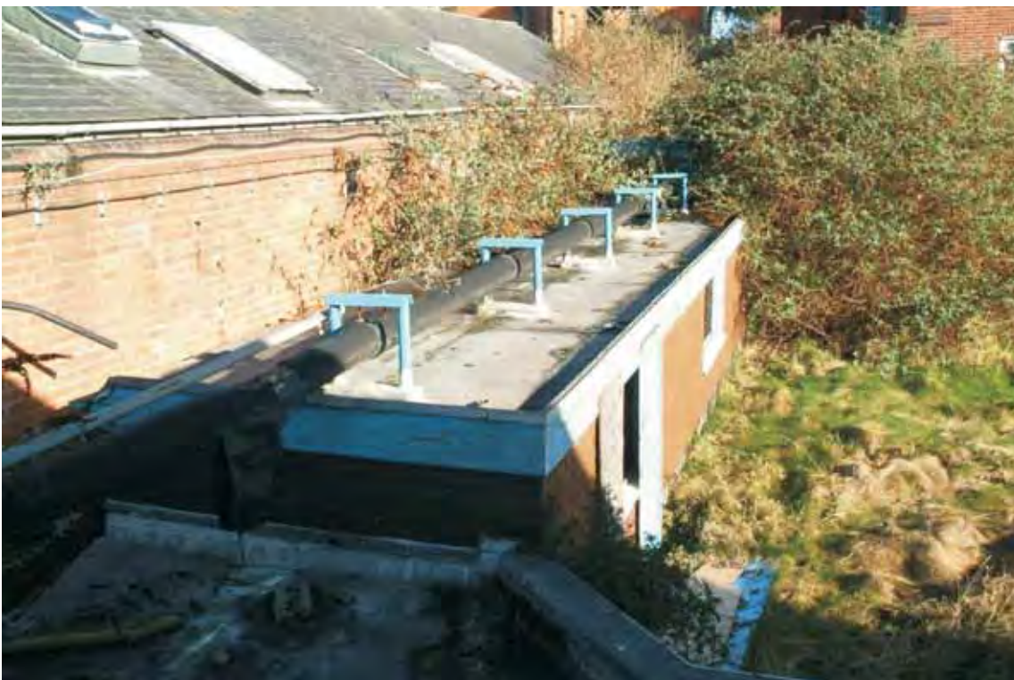
Plate 15.1: Building 15 – roof and south elevation against rear of Building 14
