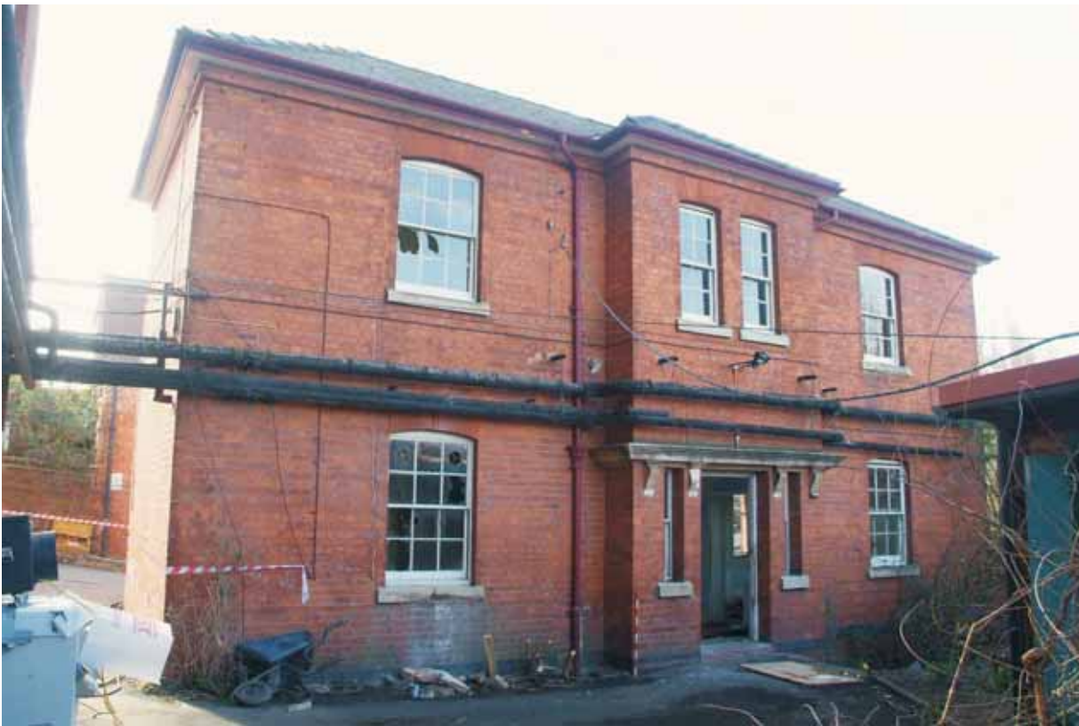
Plate 18.1: Building 18 – north (principal) elevation
