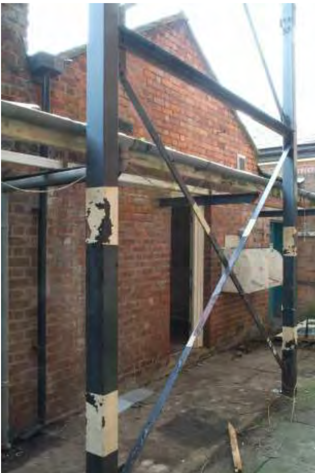
Plate 35.4: Building 35 – interior, view to the southeast
