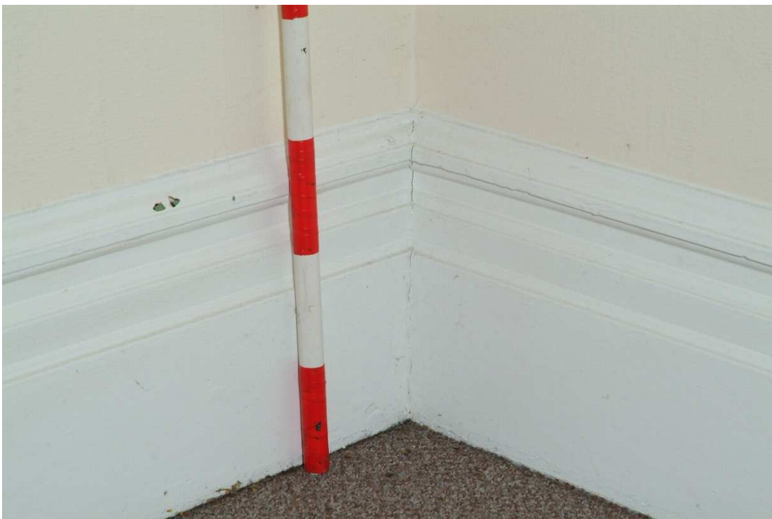
Plate 43.32: Building 43 – ground floor: detail of standard skirting
