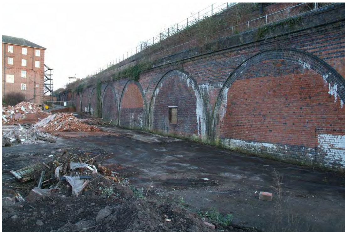
Plate 44.1: Building 44 – general view of northern elevation, view to the southeast
