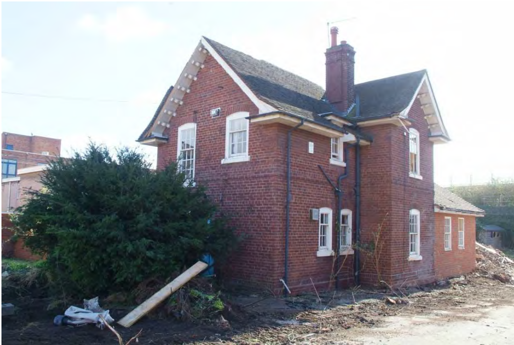
Plate 31.7: Building 31: western elevation, view to the southeast
