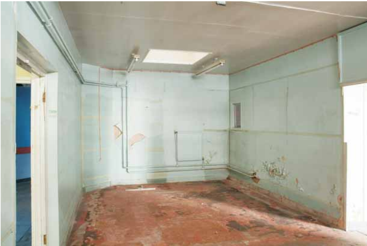
Plate 15.8: Building 15a – interior, view to the north
