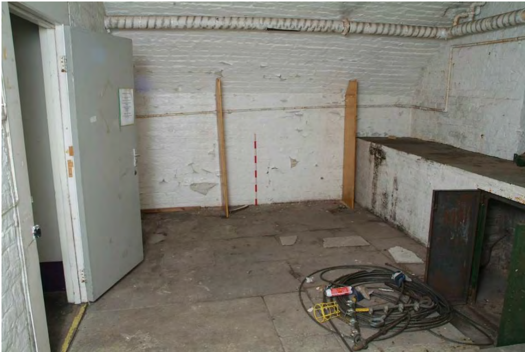
Plate 24.131: Building 24 (LGF): Room 89, view to the north
