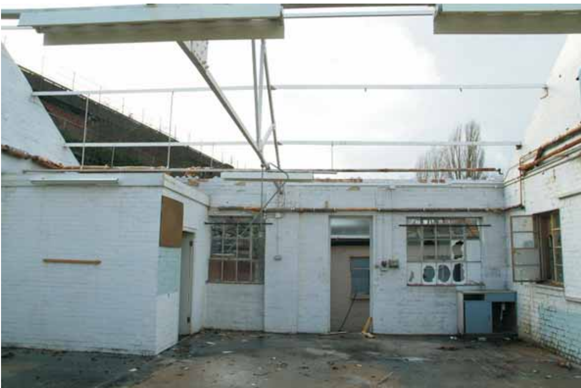
Plate 6.10: Building 6 – interior of former southernmost workshop, view to the southwest
