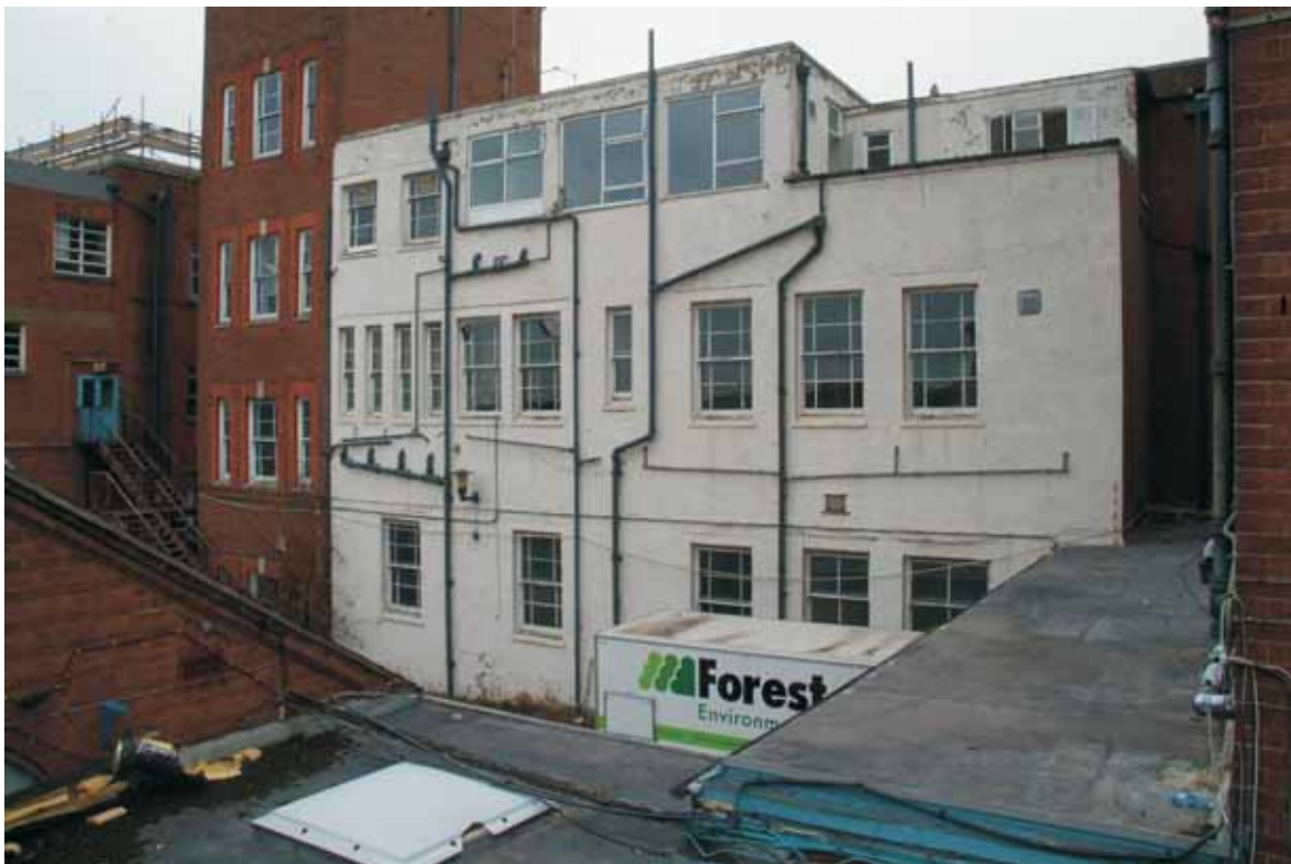
Plate 16.1: Building 16 – southern elevation, view to the northeast
