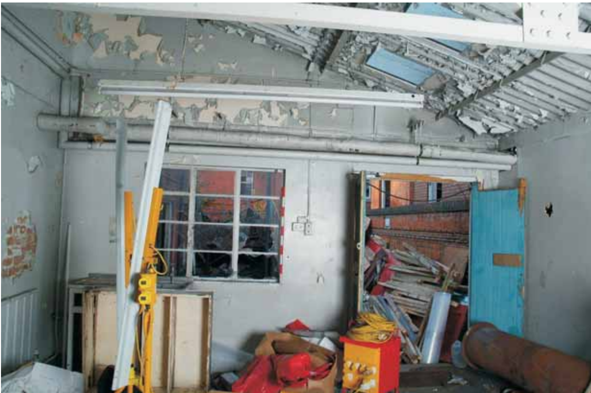
Plate 10.19: Building 10 – interior of workshop in eastern range, view to the north
