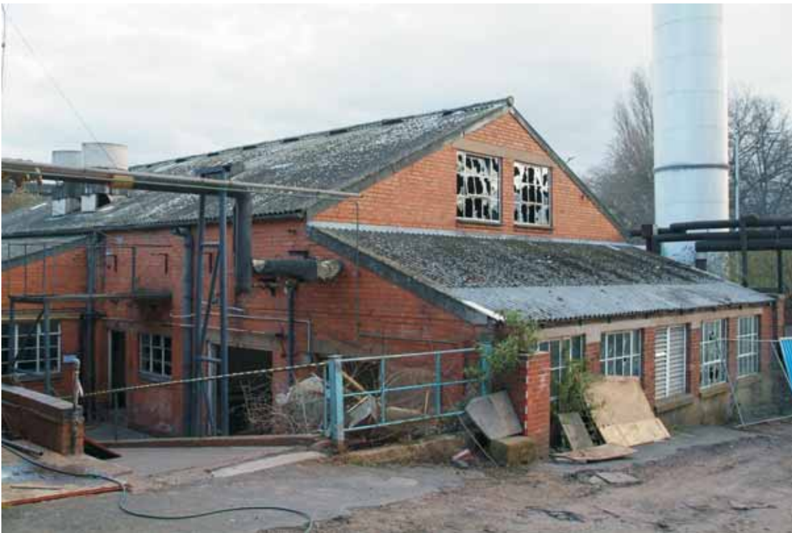
Plate 10.4: Building 10 – northern and eastern elevations, view to the south west
