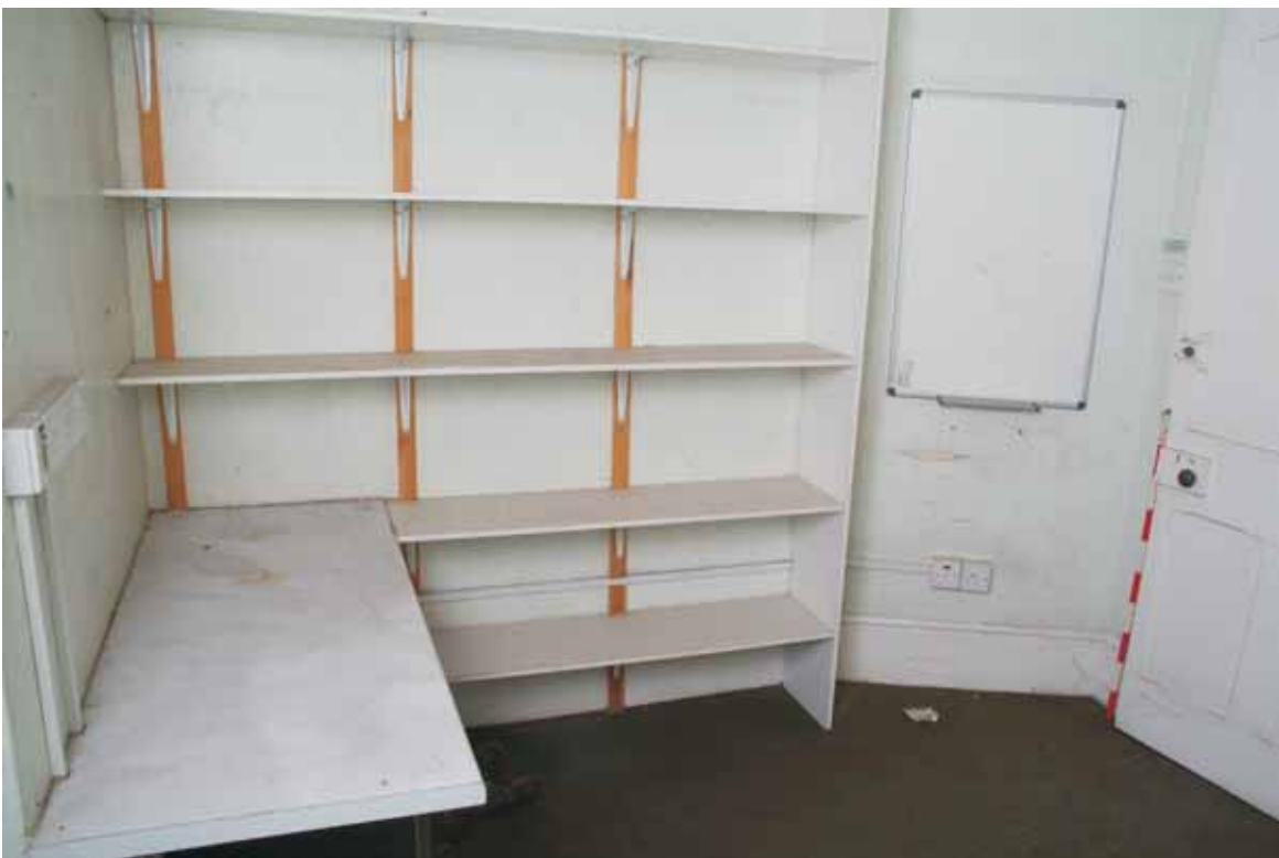
Plate 18.38: Building 18 – first floor: east side of partitioned duty room, view to the northwest
