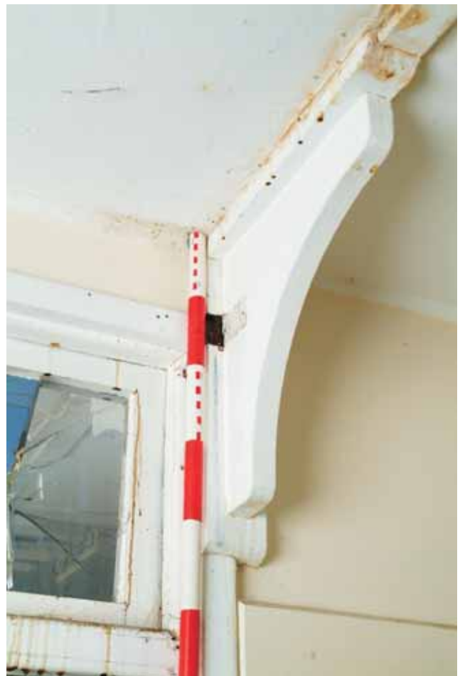
Plate 2.6: Building 2 – detail of roof bracket
