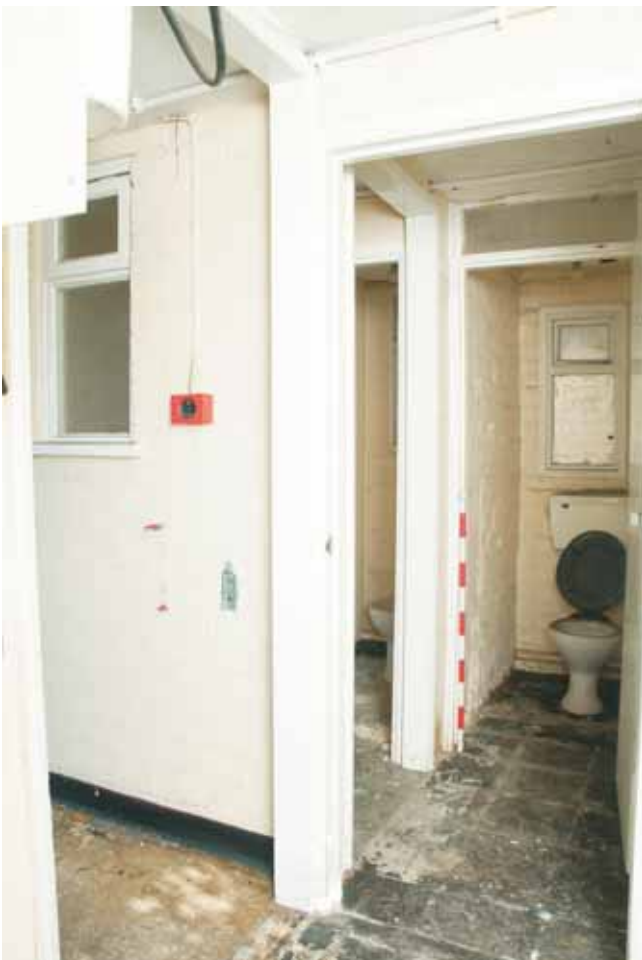
Plate 20.8: Building 20 – lavatories in the linking range, view to the south
