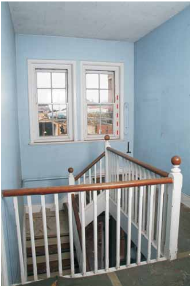
Plate 18.9: Building 18 – first floor: gallery and stairwell, view to the north
