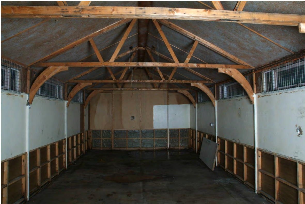
Plate 37.7: Building 37 – general view of interior, view to the north
