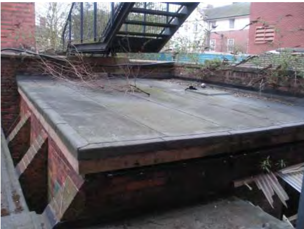
Plate 36.2: Building 36 – roof, view to the southwest
