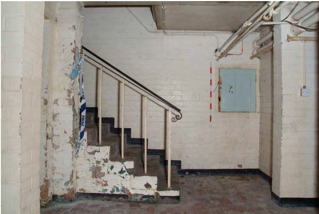
Plate 43.41: Building 43 – basement: entrance hall, view to the south
