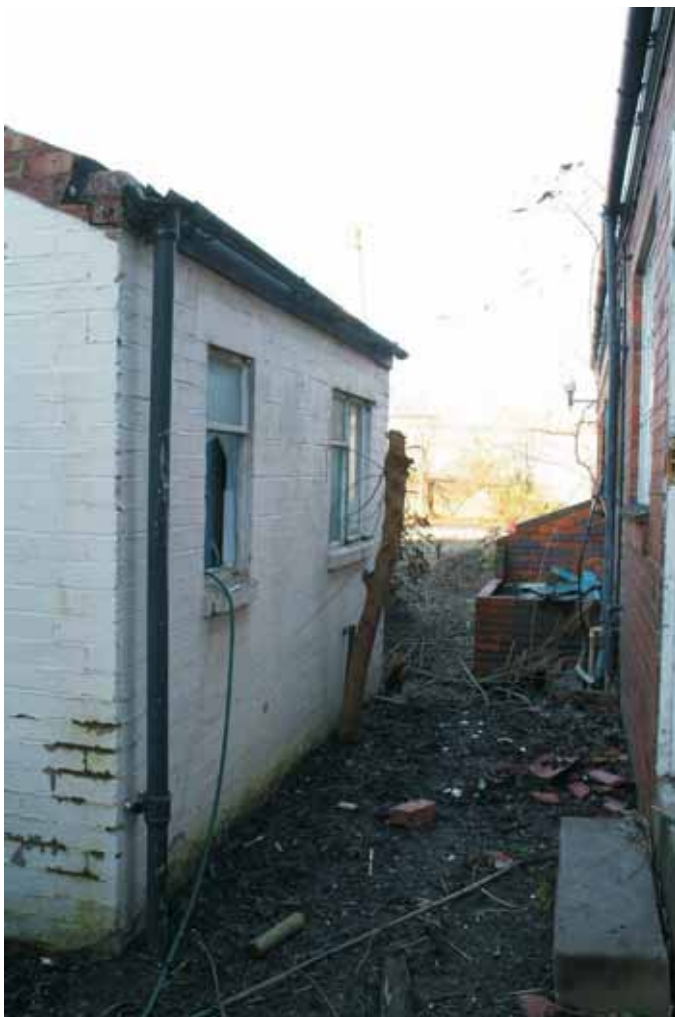
Plate 5.3: Building 5 – eastern elevation
