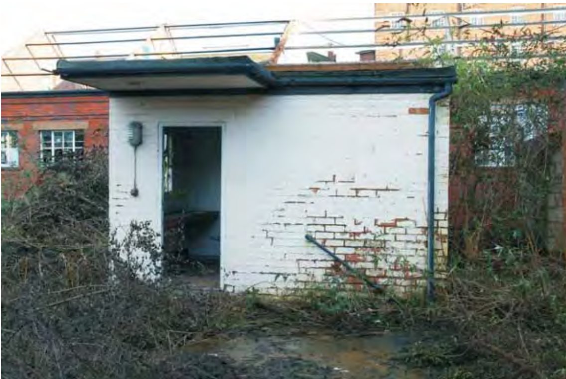
Plate 5.2: Building 5 – western elevation
