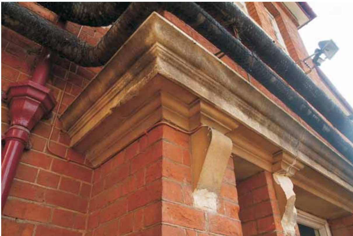
Plate 18.2: Building 18 – detail of stone cornice, view to the southwest
