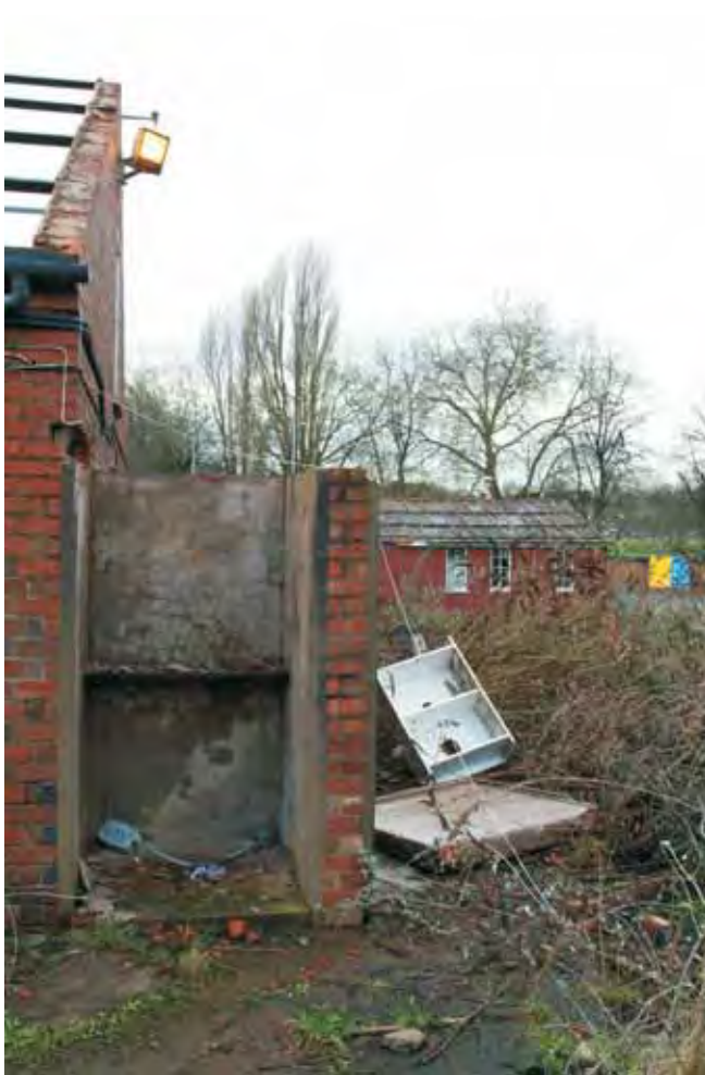
Plate 6.5: Building 6 - external store
