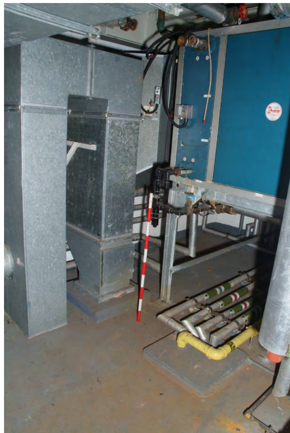
Plate 32.2: Building 32: interior of first floor plant room, view to the southeast
