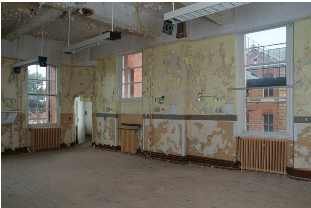
Plate 24.184: Building 24 (FF): eastern end of Ganderton Ward showing modified windows, view to the southeast
