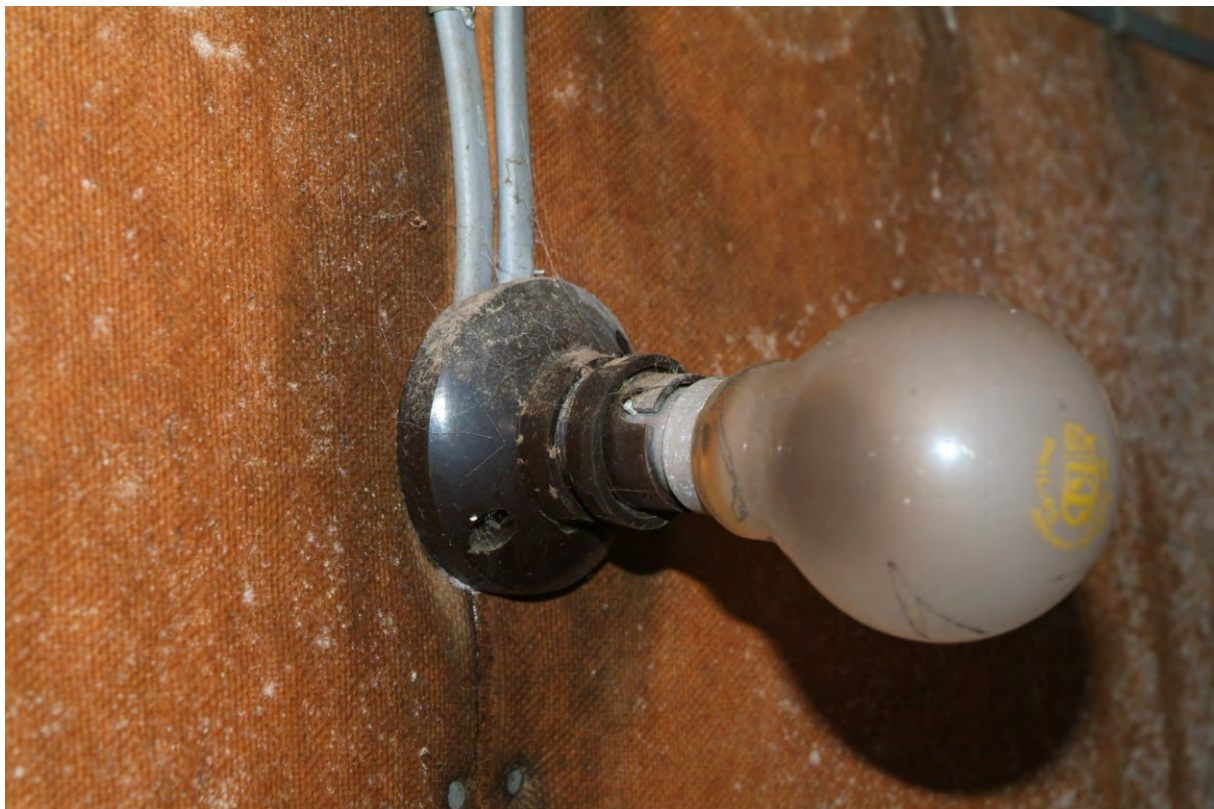
Plate 38.4: Building 38 – detail of Bakelite bulb holder, view to the southwest
