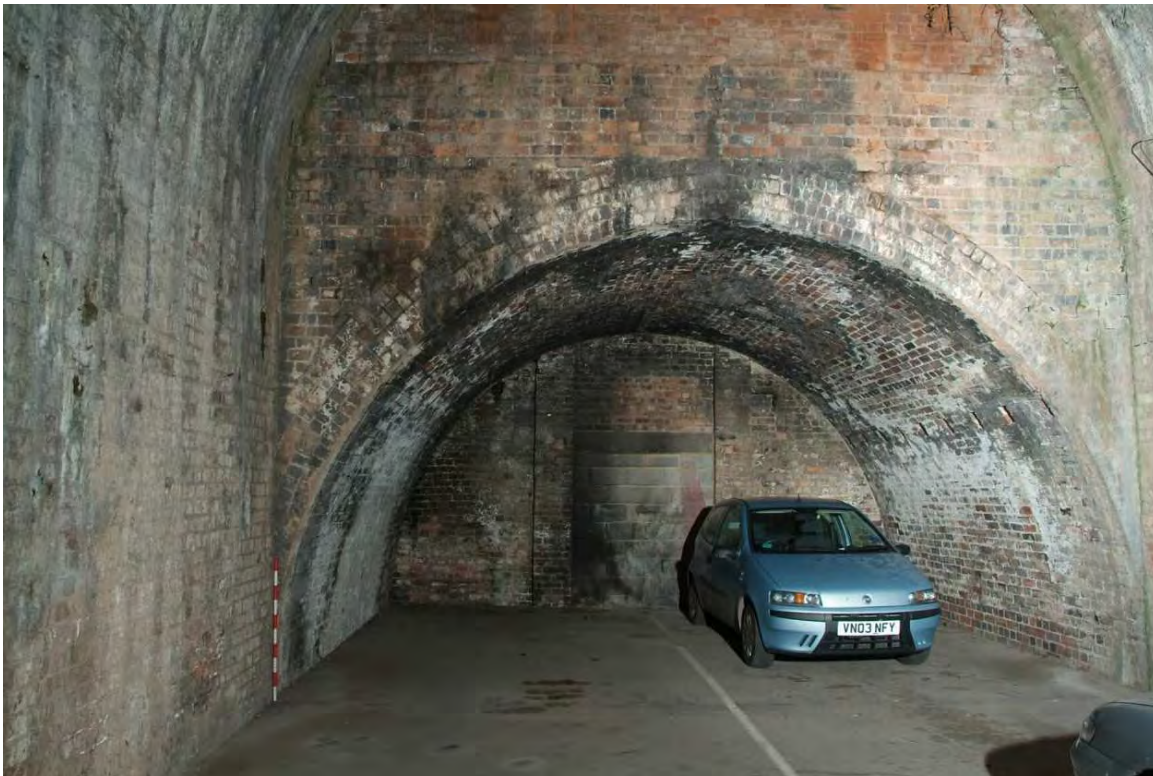
Plate 44.9: Building 44 – detail of arch structure, view to the north
