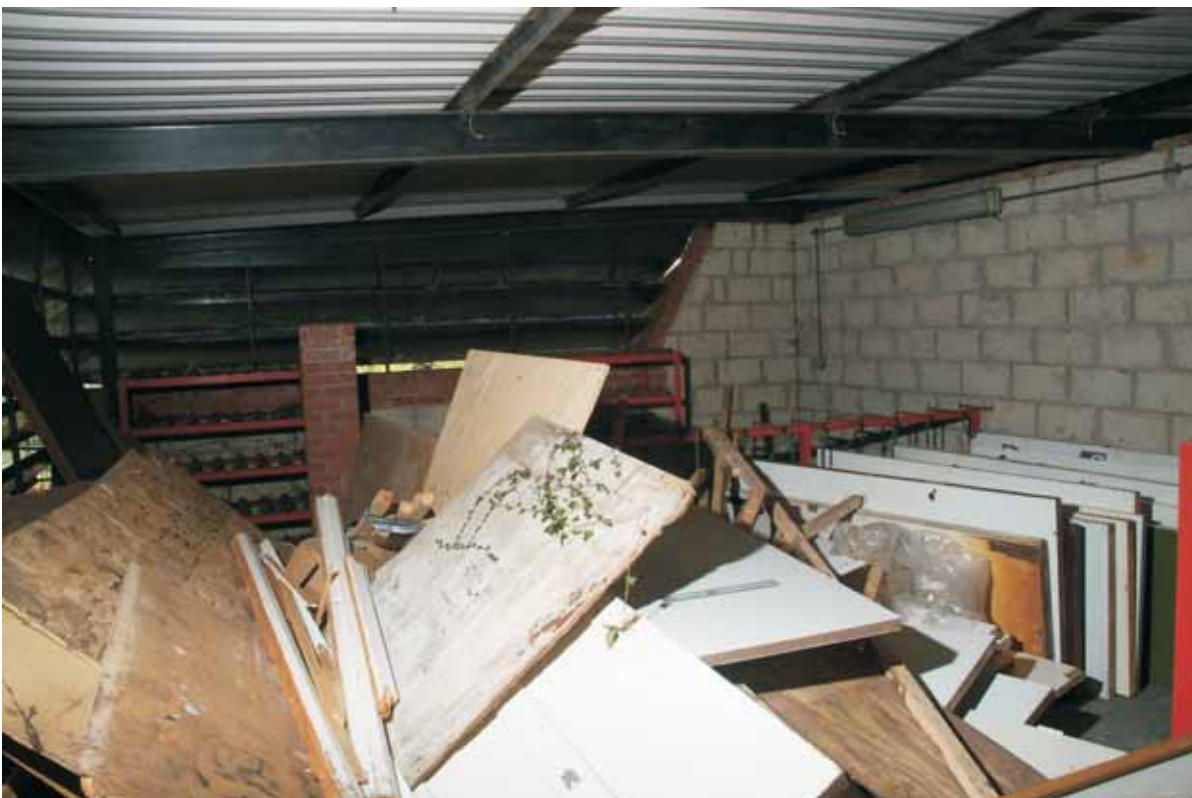
Plate 19.4: Building 19 – interior showing gas bottle racks, view to the west
