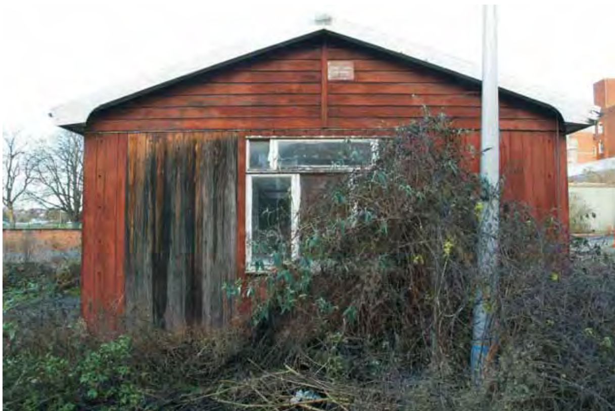
Plate 2.2: Building 2 – western elevation
