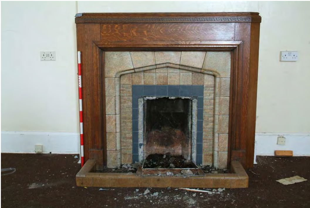
Plate 27.21 : Building 27a – ground floor: detail of 'Wellington' fireplace within sister's sitting room, view to the north
