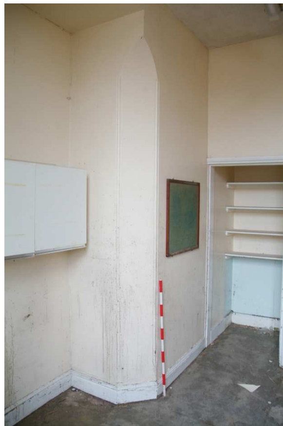
Plate 24.74: Building 24: Room 1.32, view to the east
