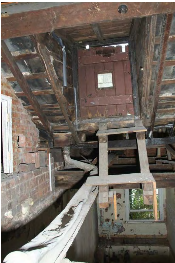
Plate 24.218: Building 24 (Room Structure): former steps to roof access dormer, view to the west
