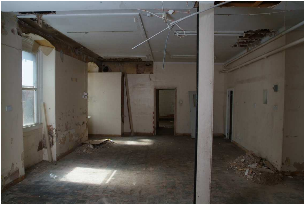
Plate 24.100: Building 24 (LGF): nursing staff changing areas [Room 109], view to the west
