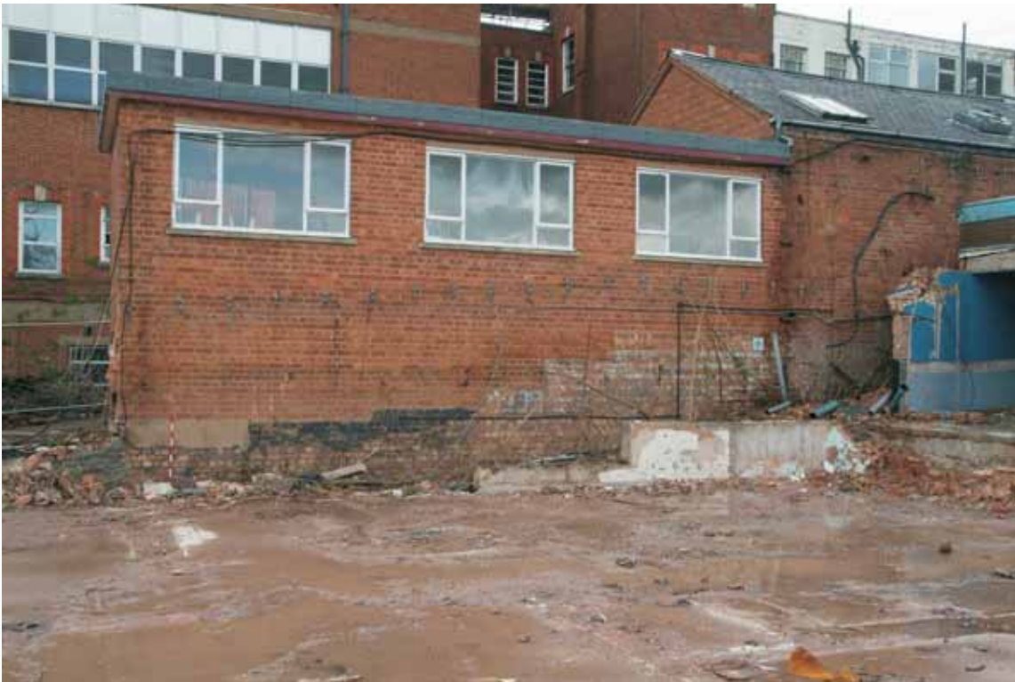
Plate 13.4: Building 13 - southern elevation showing earlier wall at base, view to the north
