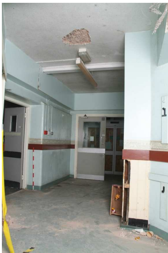
Plate 24.146: Building 24 (LGF): late 20th century entrance, lobby and doors to the ECG room in Building 72, view to the southwest
