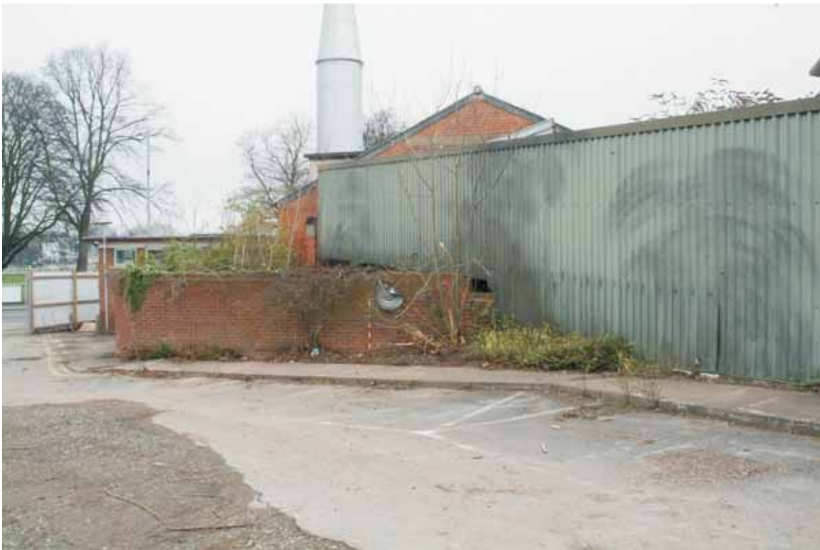
Plate 10.8: Building 10 – west side of southern elevation
