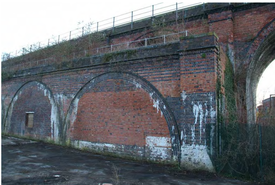
Plate 44.2: Building 44 – western end, view to the southeast
