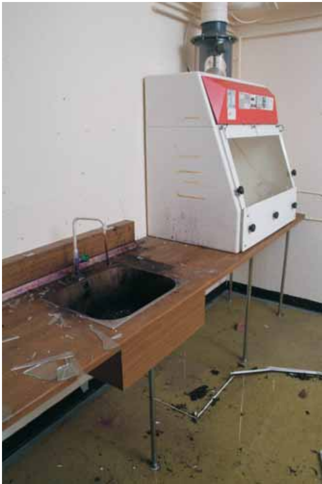
Plate 20.5: Building 20 – Interior of northern hut showing lab sink and fume cupboard, view to the northeast
