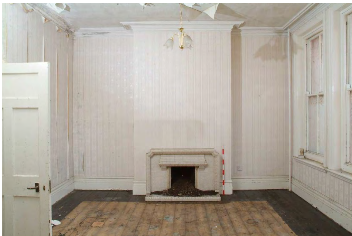
Plate 43.24: Building 43 – ground floor: lounge area showing surviving fireplace, view to the south
