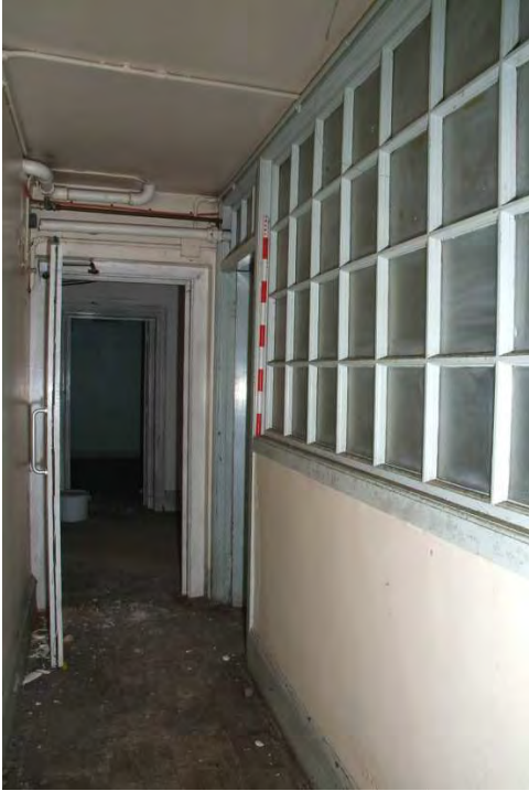
Plate 27.29: Building 27a - basement: original part glazed partition, view to the southwest
