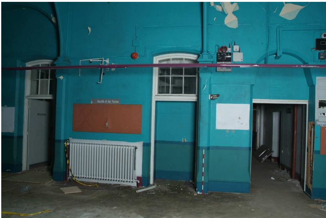
Plate 41.8: Building 41: south wall showing openings to infirmary, view to the south
