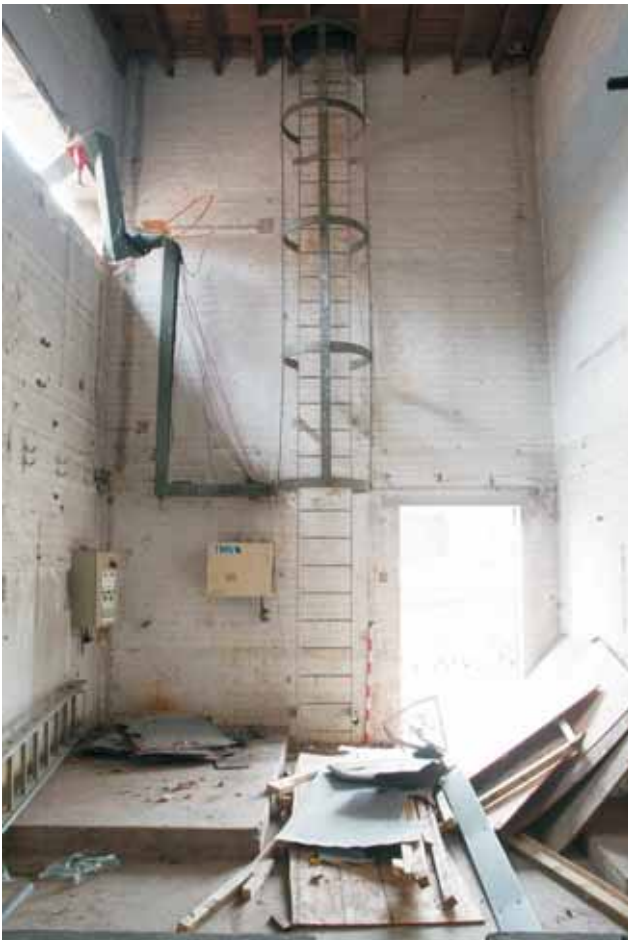
Plate 12.3: Building 12 – interior showing ladder to water tank, view to the south
