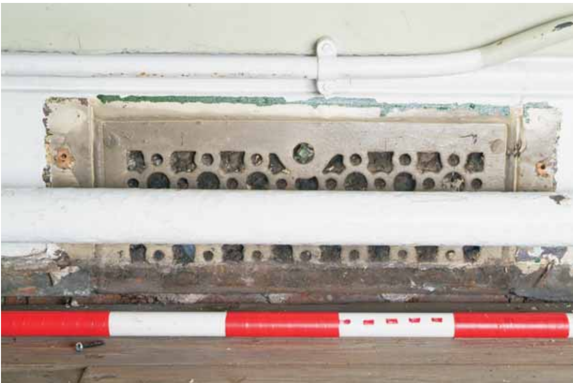
Plate 18.28: Building 18 – ground floor: detail of controllable grill in skirting board
