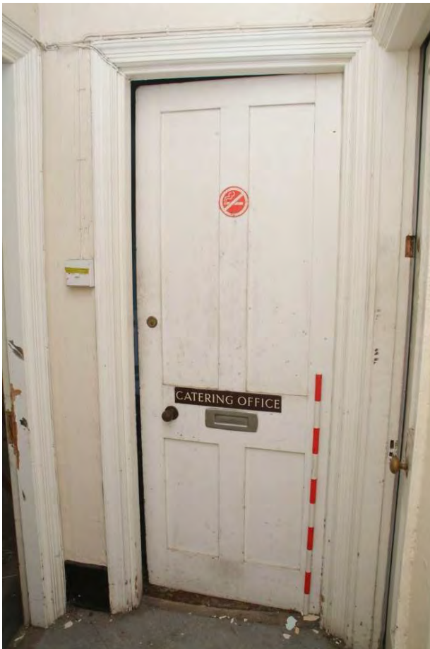
Plate 24.104: Building 24 (LGF): entrance to catering office [Room 108], view to the north
