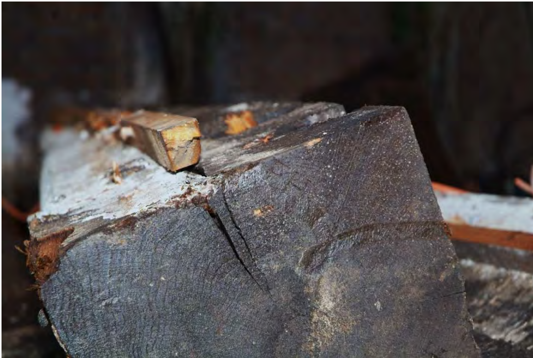
Plate 30.61: Building 30 (GF): detail of floor joist showing EH stamp in end
