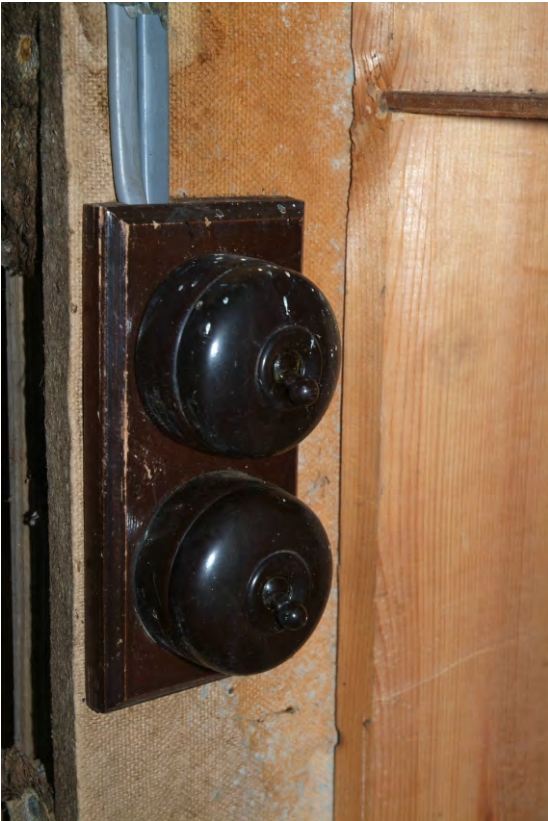
Plate 38.3: Building 38 – detail of Bakelite switches, view to the north
