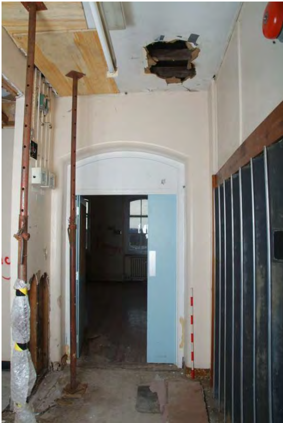
Plate 24.193: Building 24 (SF): entrance to the Maddox Ward, view to the north
