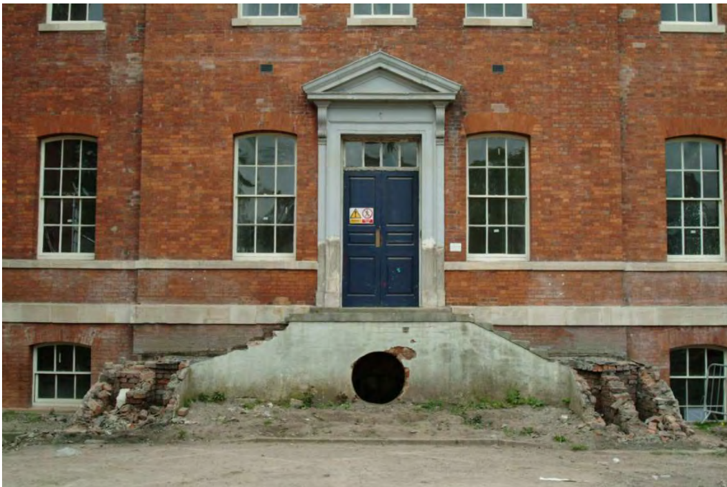
Plate 24.6: Building 24: detail showing principal entrance and steps following removal of stone treads, view to the west
