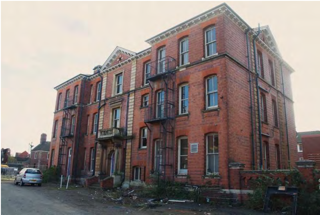
Plate 43.1: Building 43 – east elevation, view to the southwest
