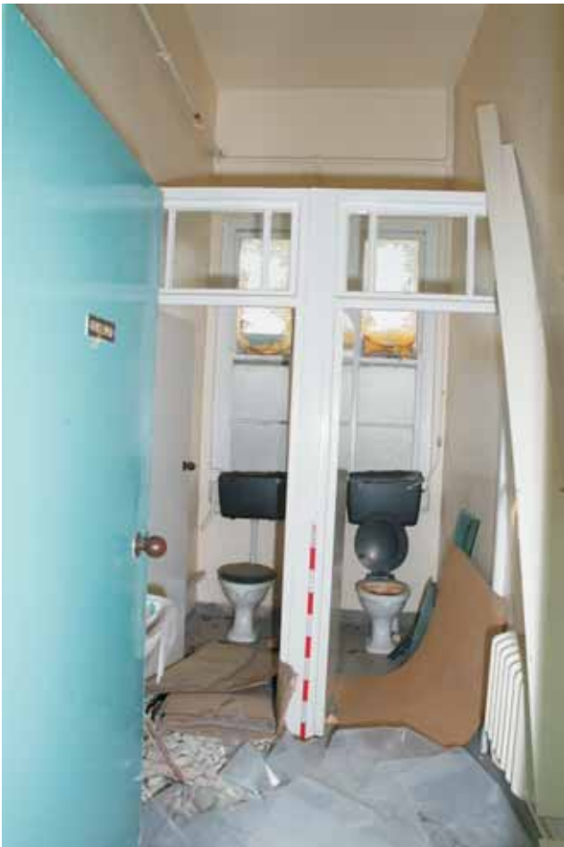
Plate 16.8: Building 16 – interior of first floor male WC, view to the south
