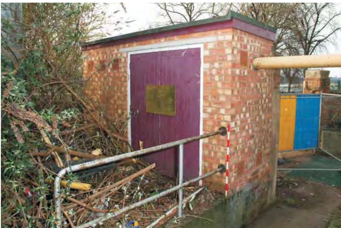
Plate 9.1: Building 9 – southern and eastern elevations
