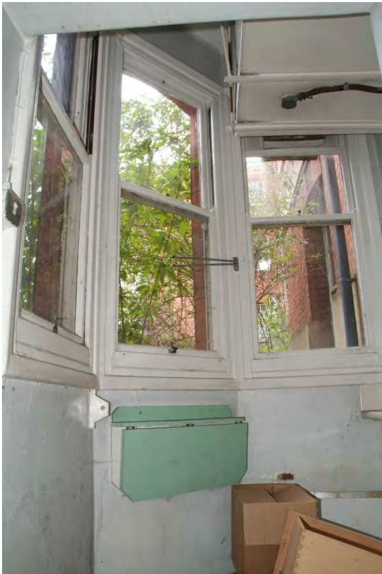
Plate 40.11: Building 40 (LGF): buffet wash-up area, view to the south
