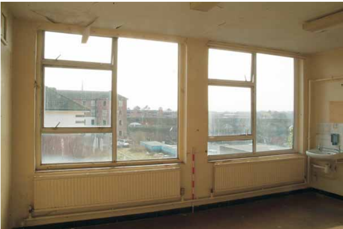
Plate 16.11: Building 16 –interior of third floor extension, view to the southwest
