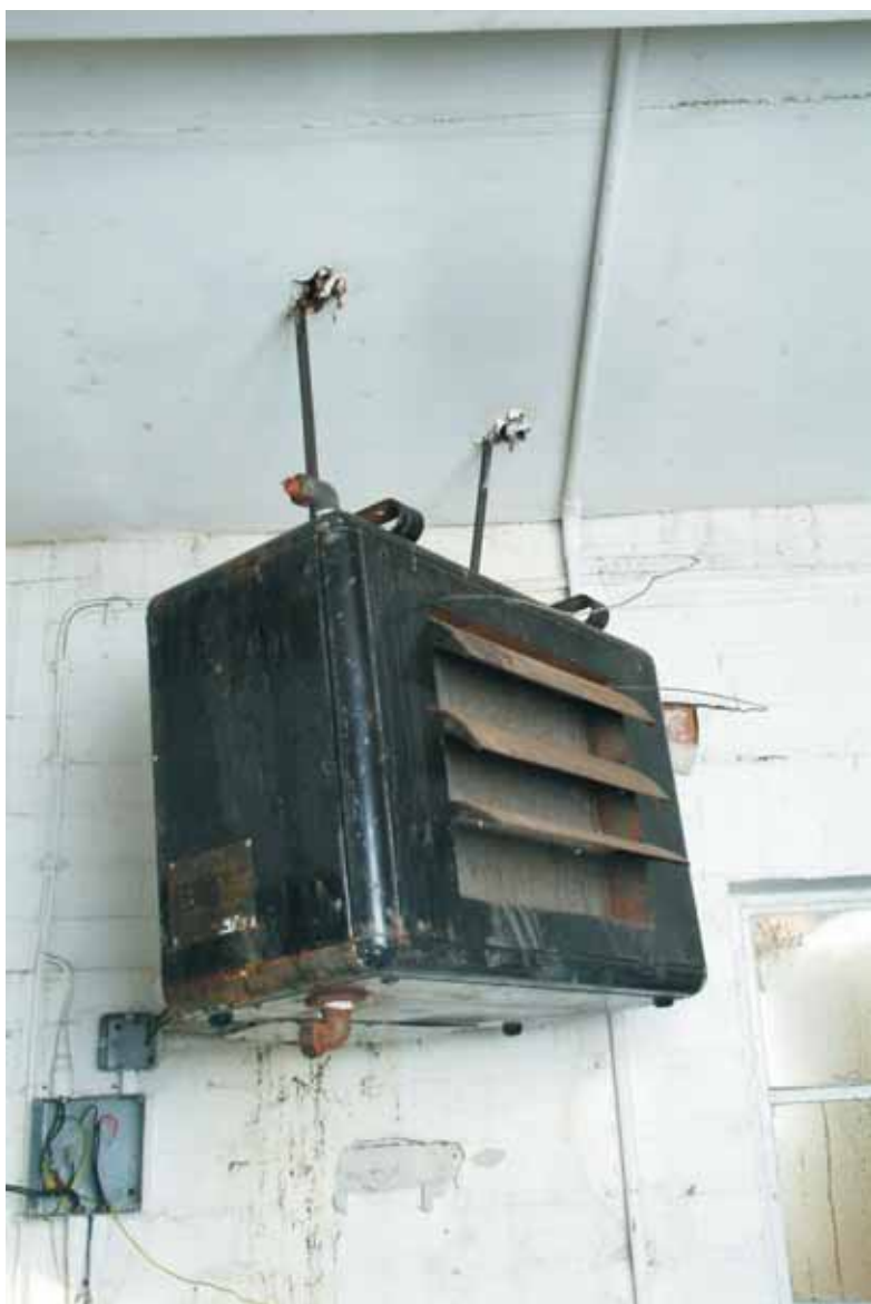
Plate 6.15: Building 6 – detail of 1950s 'Univectair' heater unit, northern workshop
