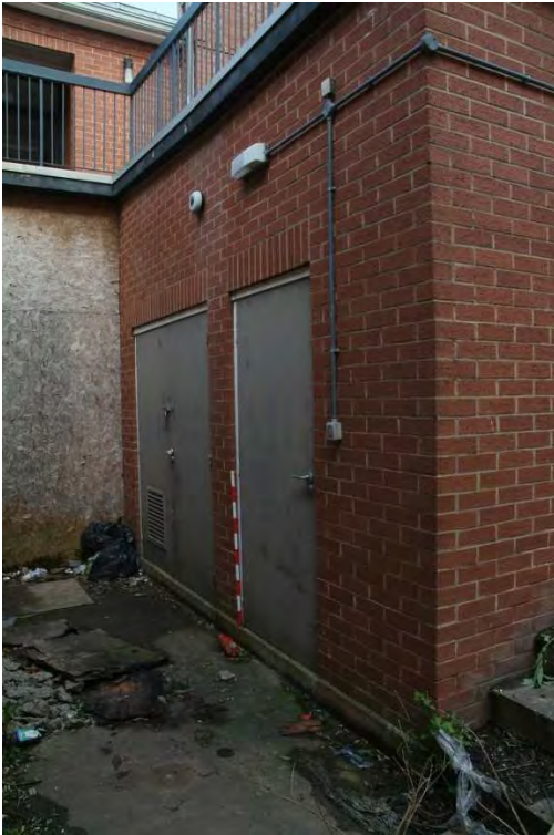
Plate 39.7: Building 39 – lower ground floor plant room, view to the southeast
