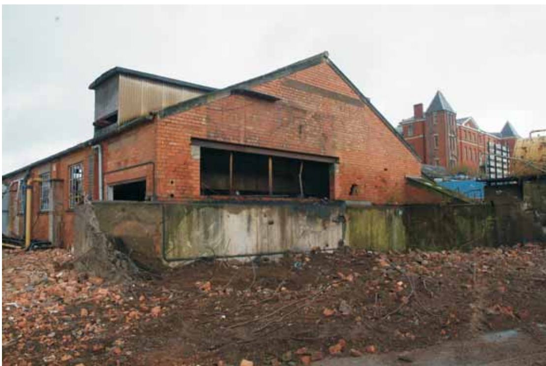
Plate 10.11: Building 10 – southern elevation following demolition of Building 25
