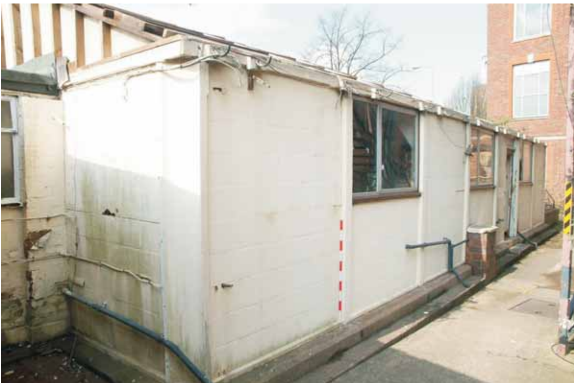
Plate 20.2: Building 20 – south and west elevations of northern hut
