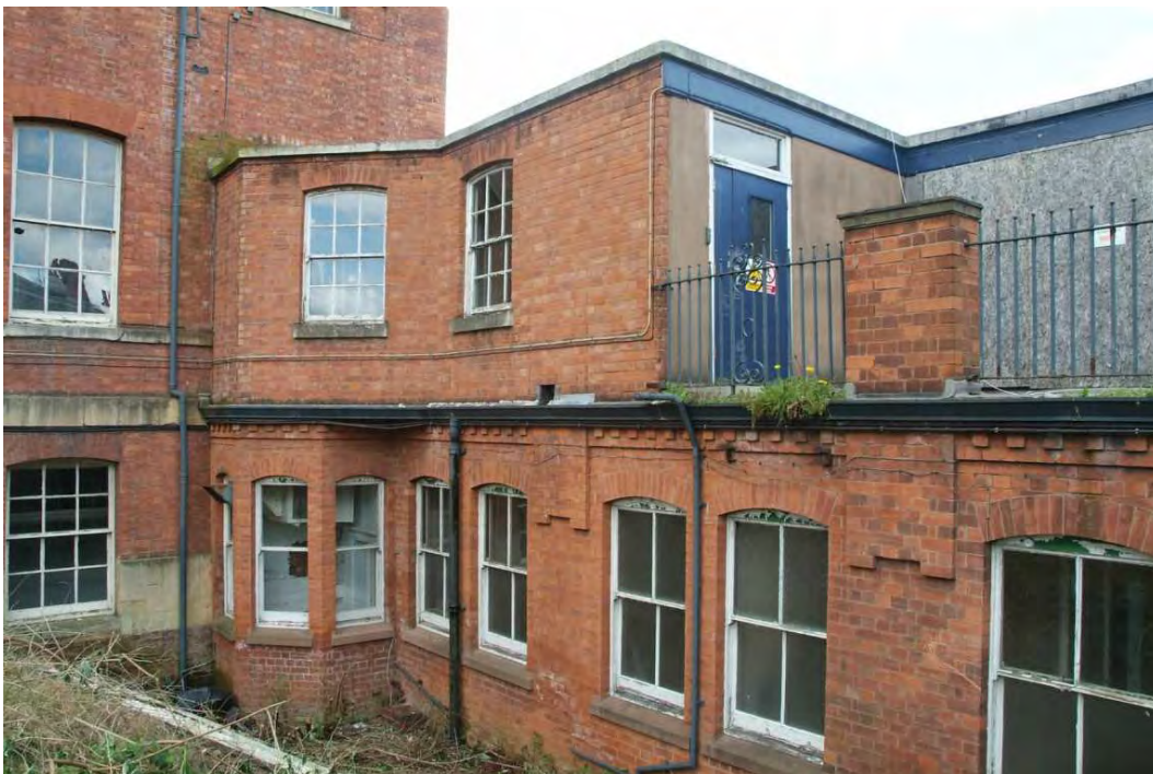
Plate 40.8: Building 40: western part of the north elevation, view to the northwest
