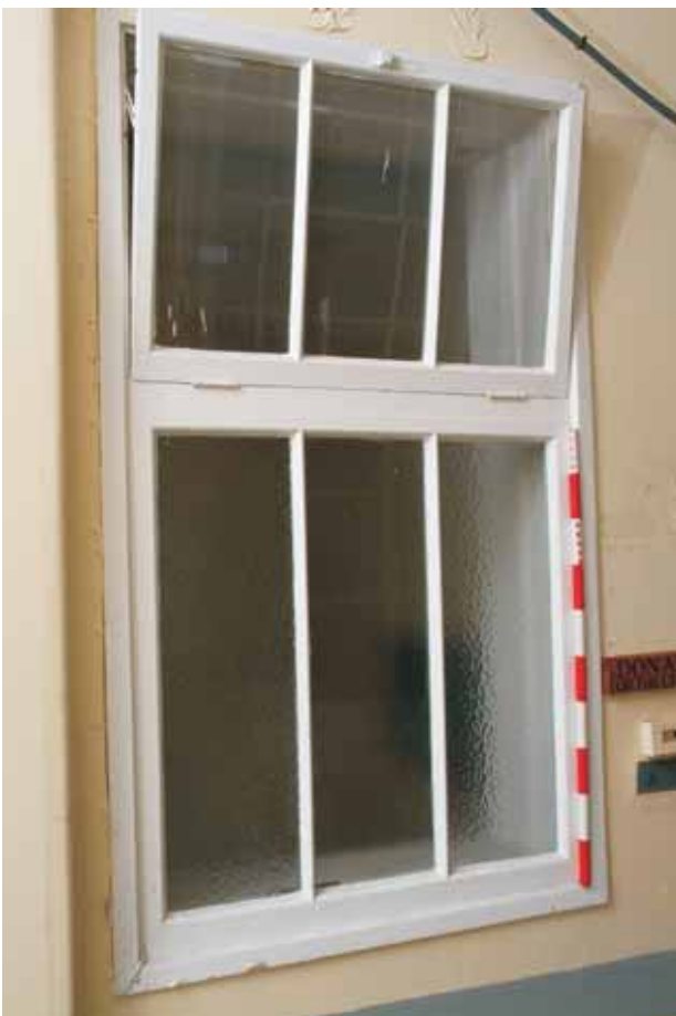
Plate 22.6: Building 22 – upper ground floor: detail of early 20th century hopperlight window, view to the northeast
