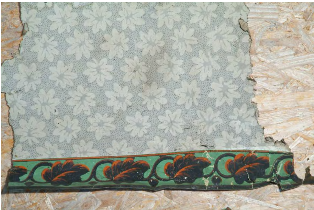
Plate 30.58: Building 30 (GF): detail of wallpaper and dado recovered from behind 1820s sash box
