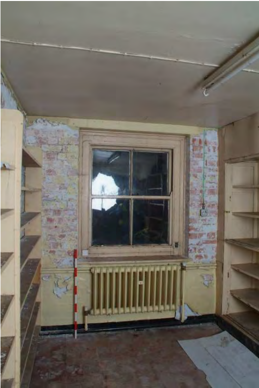
Plate 43.49: Building 43 - basement: store room, view to the north
