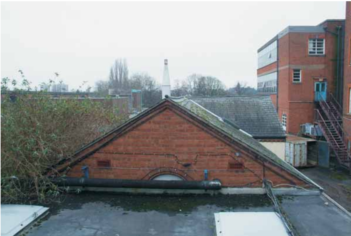
Plate 14.7: Building 14 – eastern elevation above the roof of Building 15a
