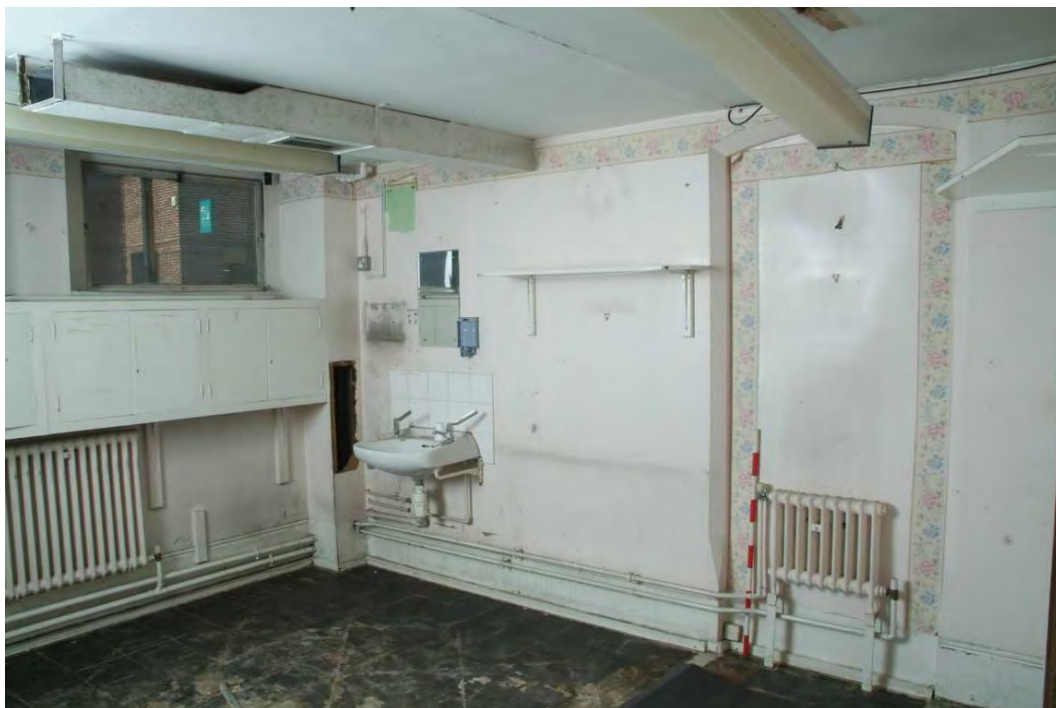
Plate 41.12: Building 41: inserted office beneath mezzanine showing blocked door, view to the northeast
