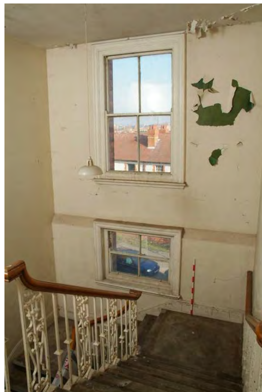
Plate 43.68: Building 43 - second floor: stairwell showing high level stairlight
