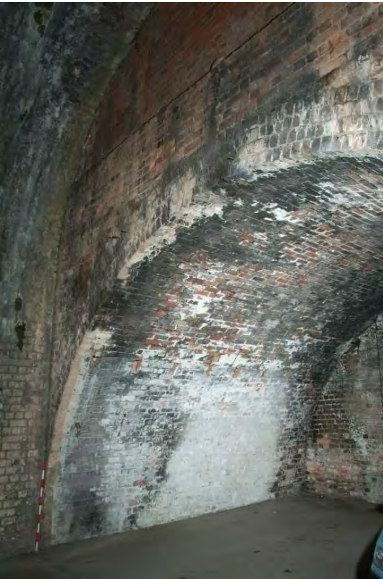
Plate 44.11: Building 44 – detail of joint between Butts Siding (right) and viaduct , view to the northwest
