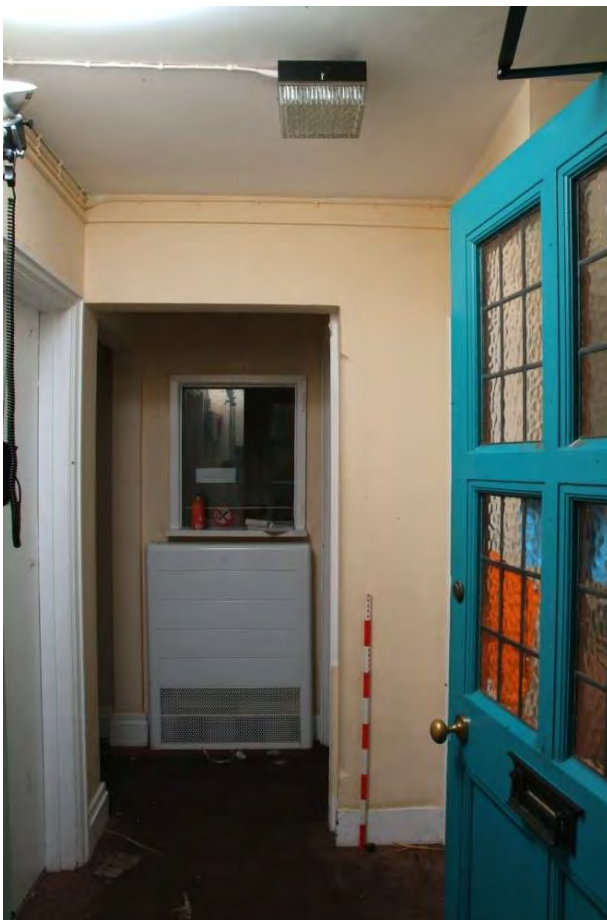
Plate 31.10: Building 31 (GF): stair hall, view to the west
