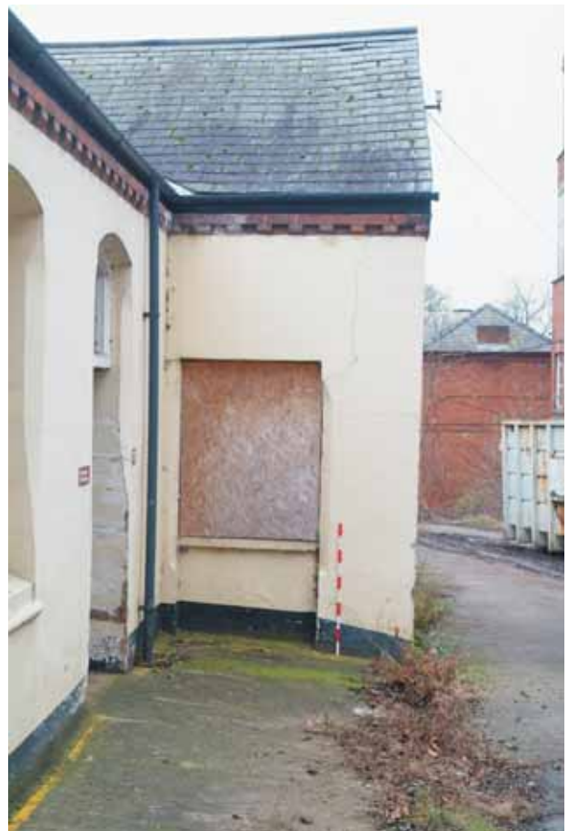
Plate 14.4: Building 14 – eastern side of central gabled projection showing blocked door, view to the west
