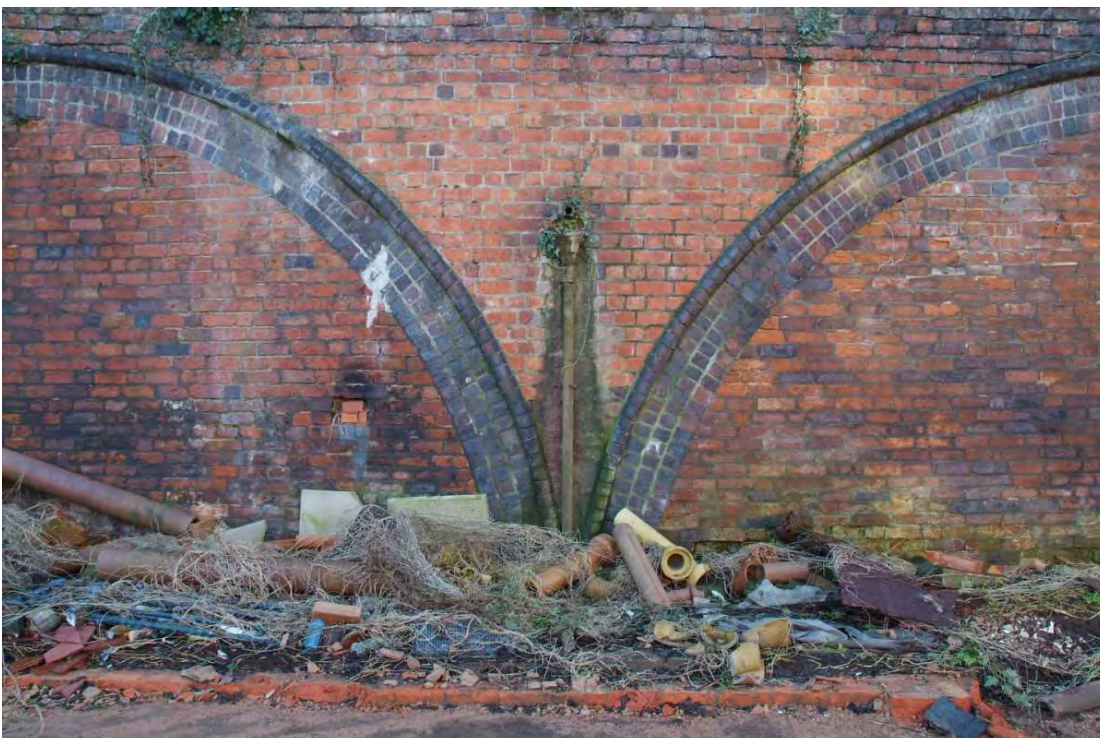
Plate 44.4: Building 44 – original drainage goods, view to the south
