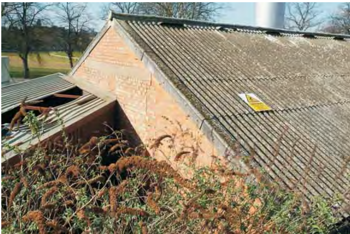
Plate 10.9: Building 10 – east side of (upper) southern elevation
