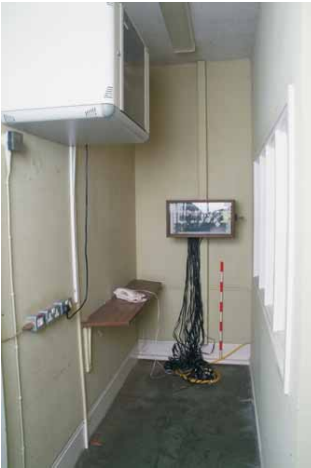
Plate 18.35: Building 18 – first floor: interior of comms room, view to the north
