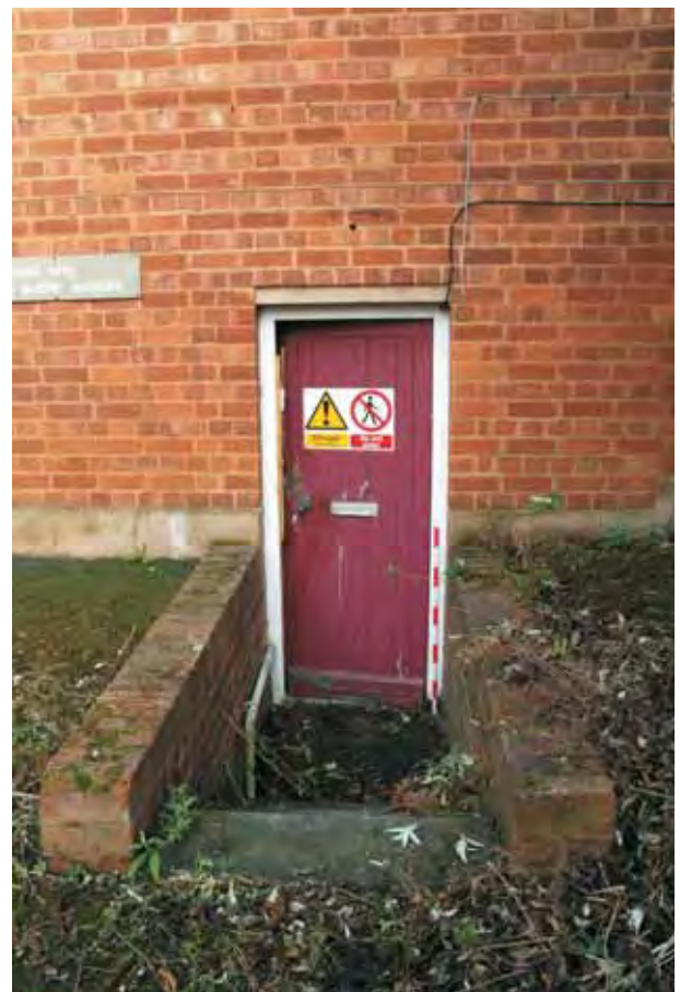
Plate 13.3: Building 13 – basement door in western elevation, view to the east
