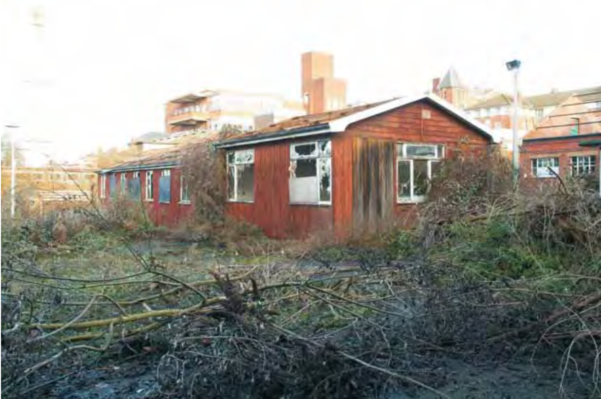
Plate 2.1: Building 2 – southern and western elevations
