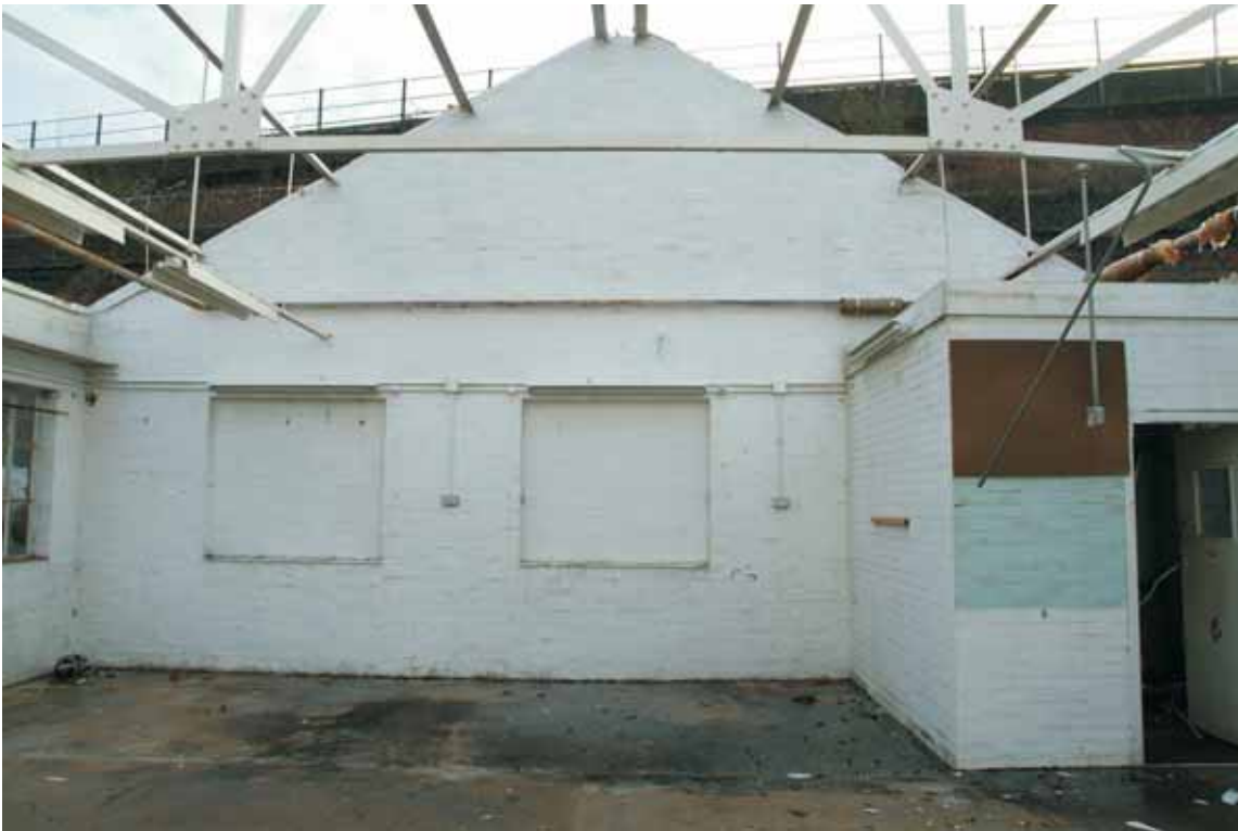
Plate 6.9: Building 6 – interior of former southernmost workshop, view to the southeast
