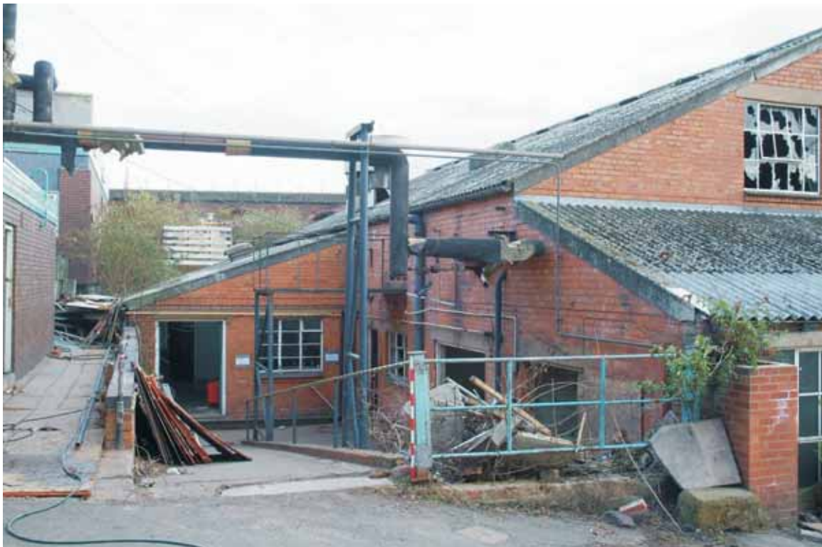
Plate 10.3: Building 10 – northern end of the east elevation, view to the south
