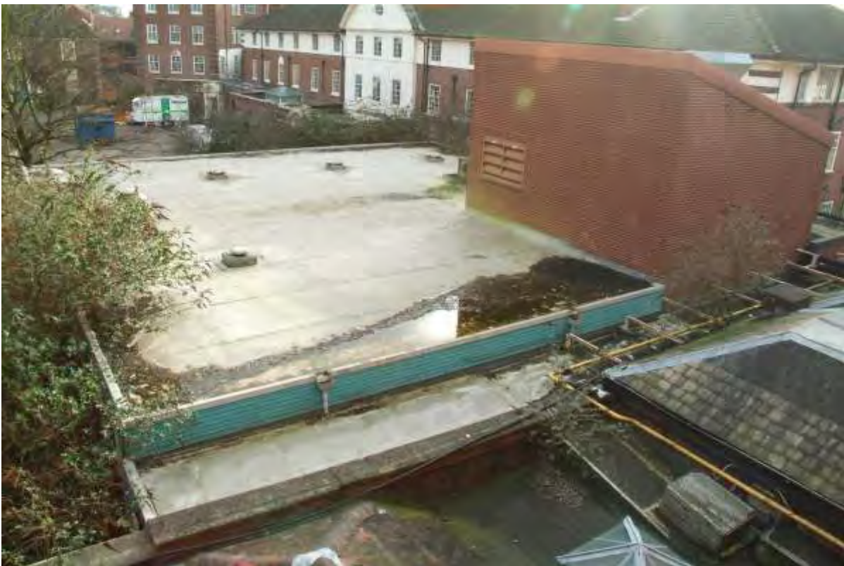
Plate 49.2: Building 49 – roof, view to the southwest
