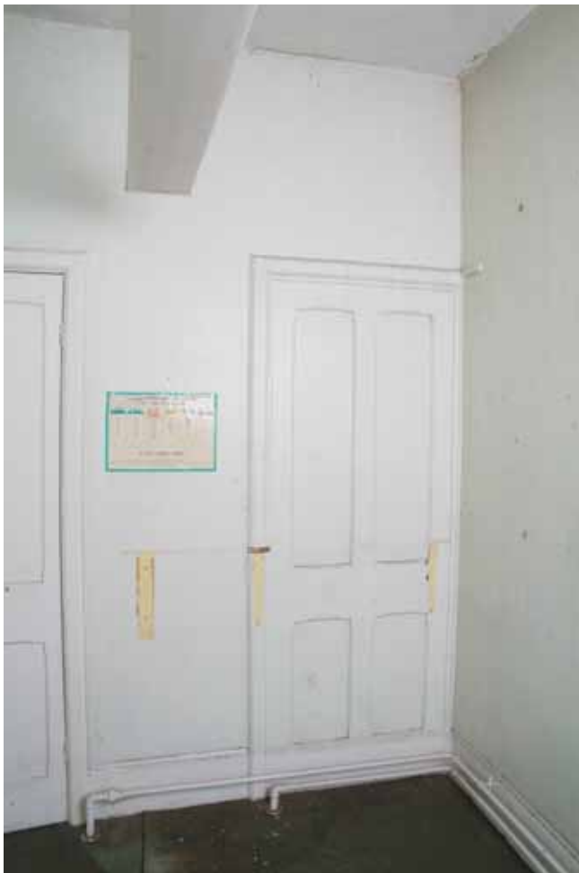
Plate 18.13: Building 18 – first floor: eastern part of partitioned duty room, view to the northeast
