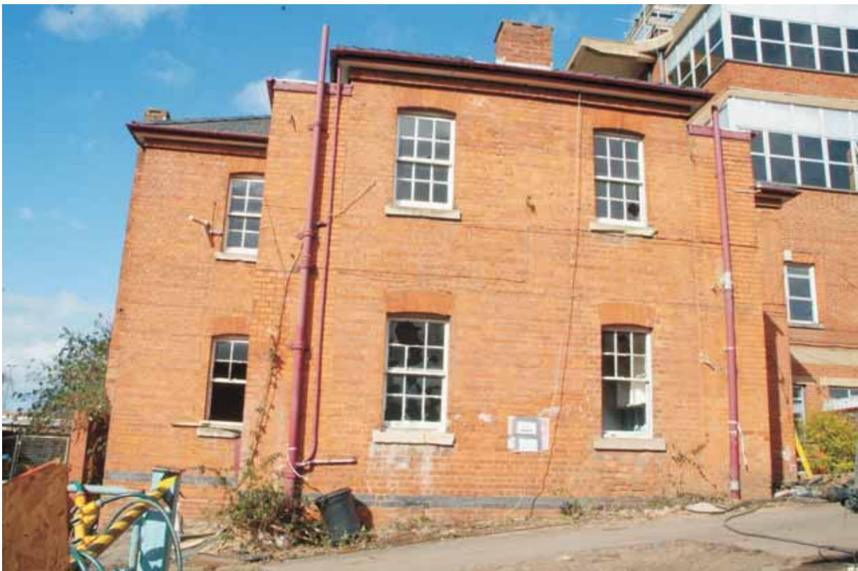
Plate 18.6: Building 18 – south elevation
