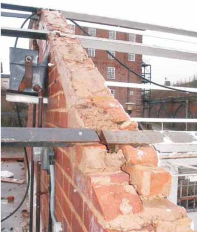
Plate 6.18: Building 6 – detail showing original metal purlins (right) and later purlins over central and northern workshops, view to the east
