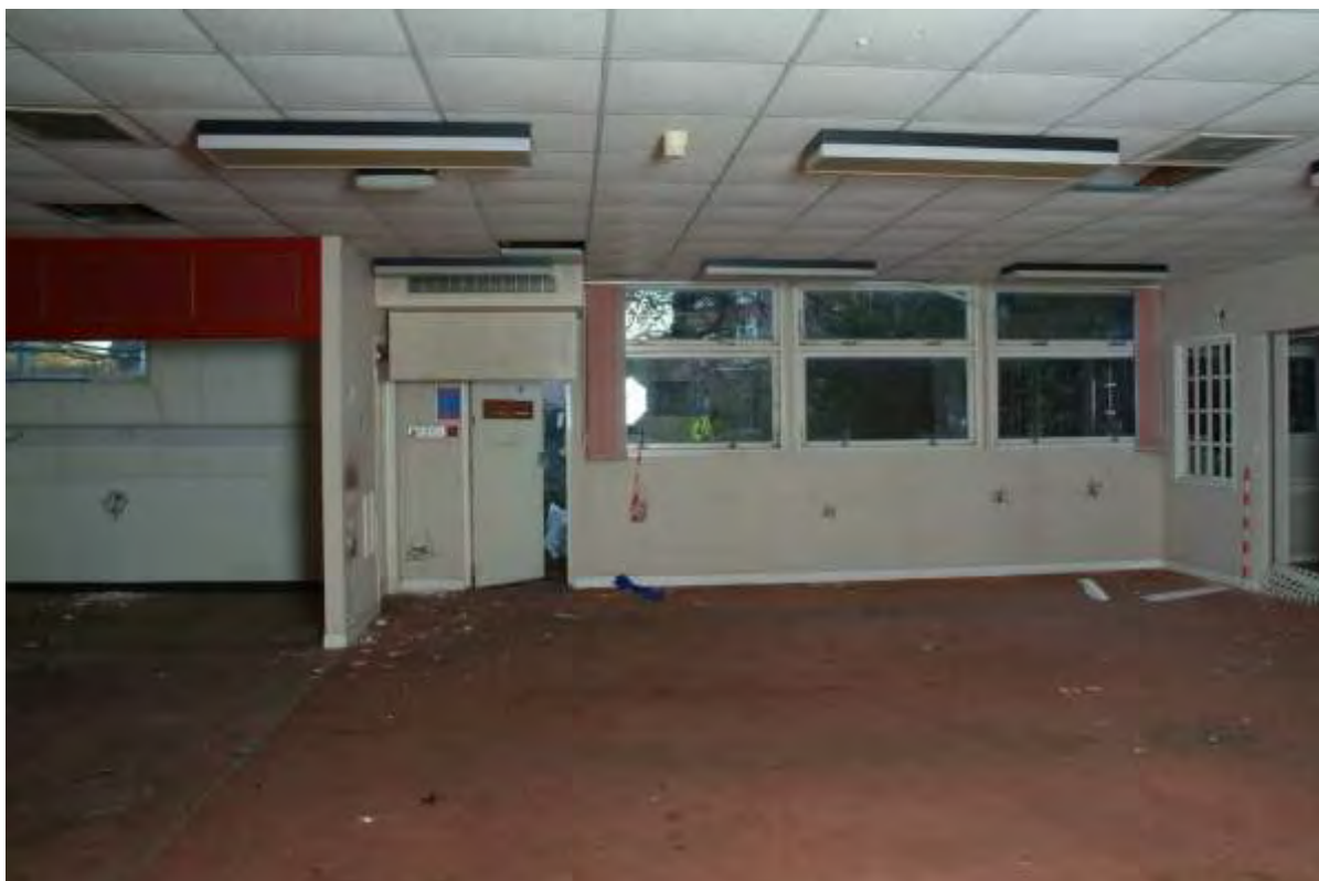
Plate 49.5: Building 49 - interior of southern dining area, view to the southwest
