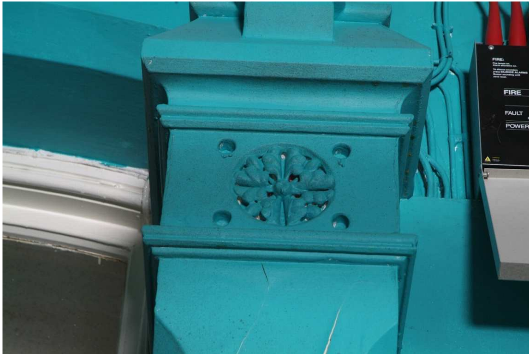
Plate 41.9: Building 41: detail of typical pilaster head, view to the south
