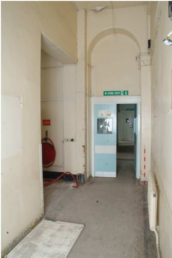
Plate 24.155: Building 24 (FF): part blocked round headed arch in central corridor, view to the north
