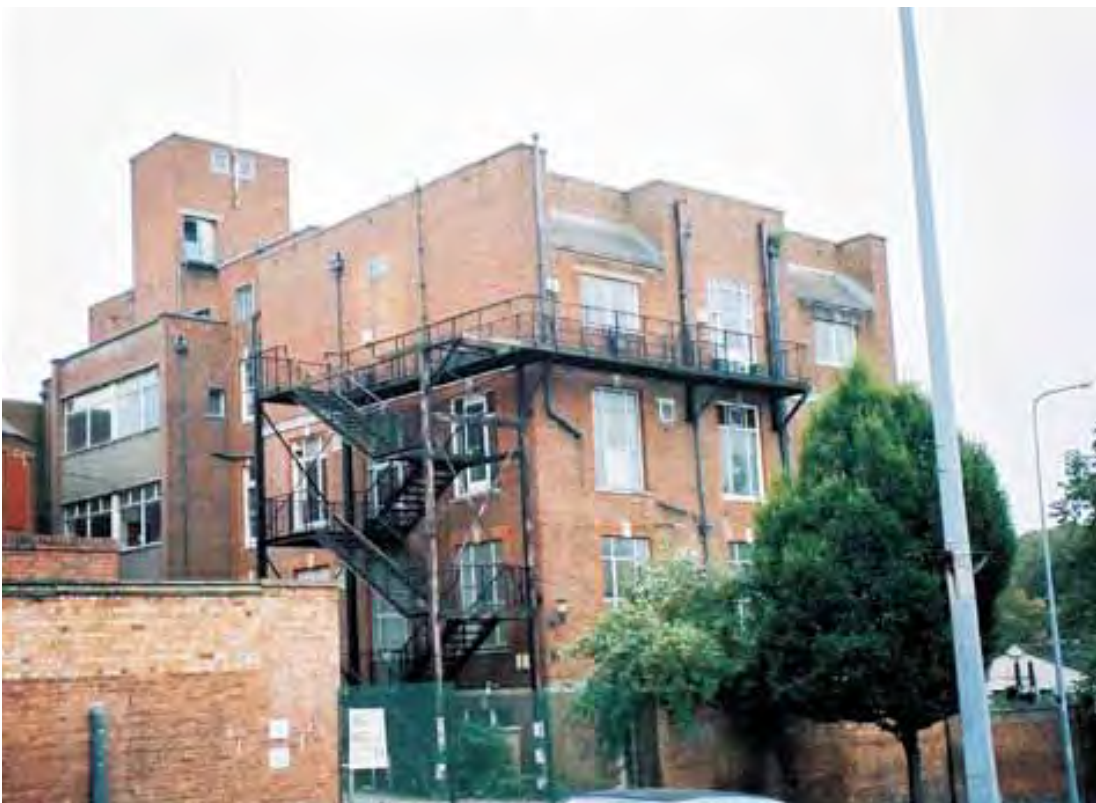
Plate 17.2: Building 17a –north elevation (right)
