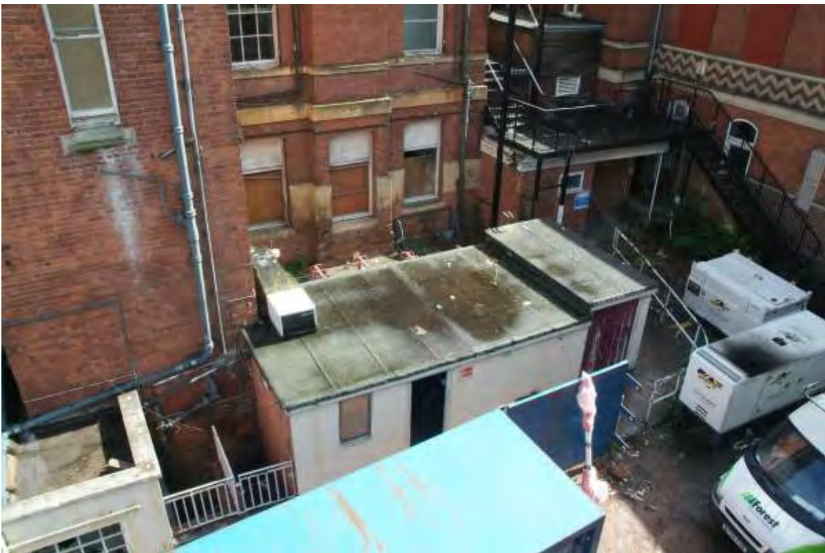
Plate 48.2: Building 48: southern part, view to the east
