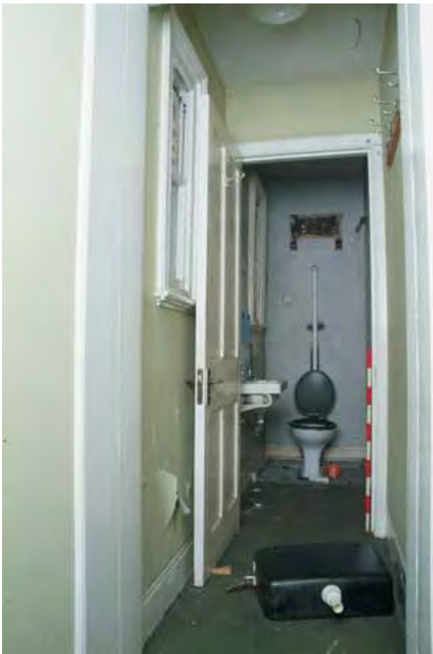
Plate 18.11: Building 18 – first floor: eastern closet wing, view to the south
