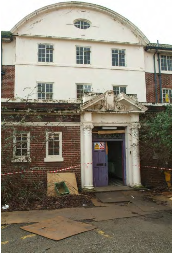
Plate 27.2 : Building 27a – detail of central part of eastern elevation
