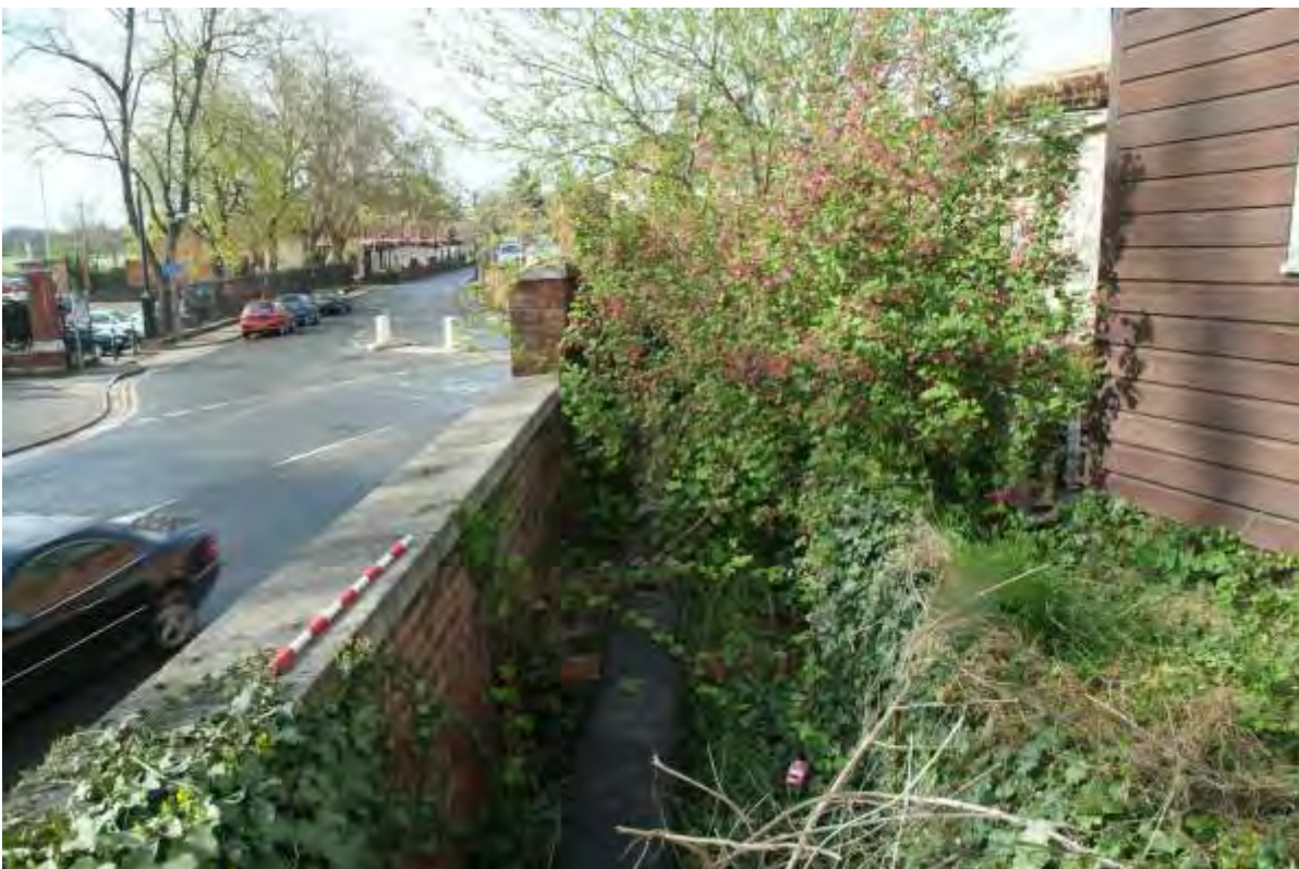
Plate 47.12: Building 47: hospital elevation 03
