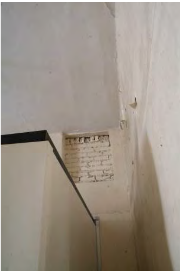
Plate 34.11: Building 34 – detail of vent in south wall, view to the south
