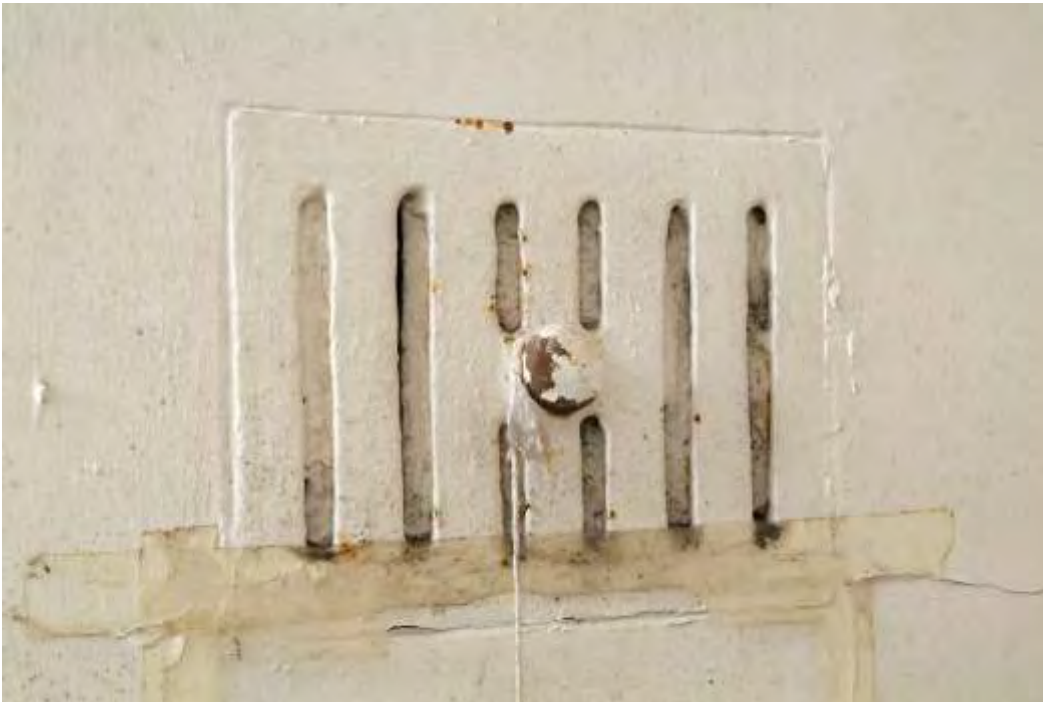
Plate 34.12: Building 34 – detail of closable vent in the northern wall, view to the north
