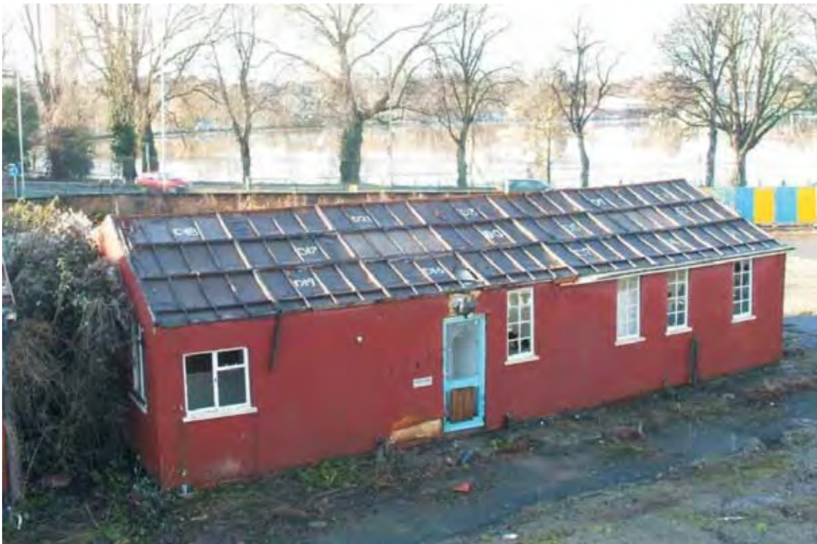
Plate 3.1: Building 3 – southern and eastern elevation (taken from B.27b)
