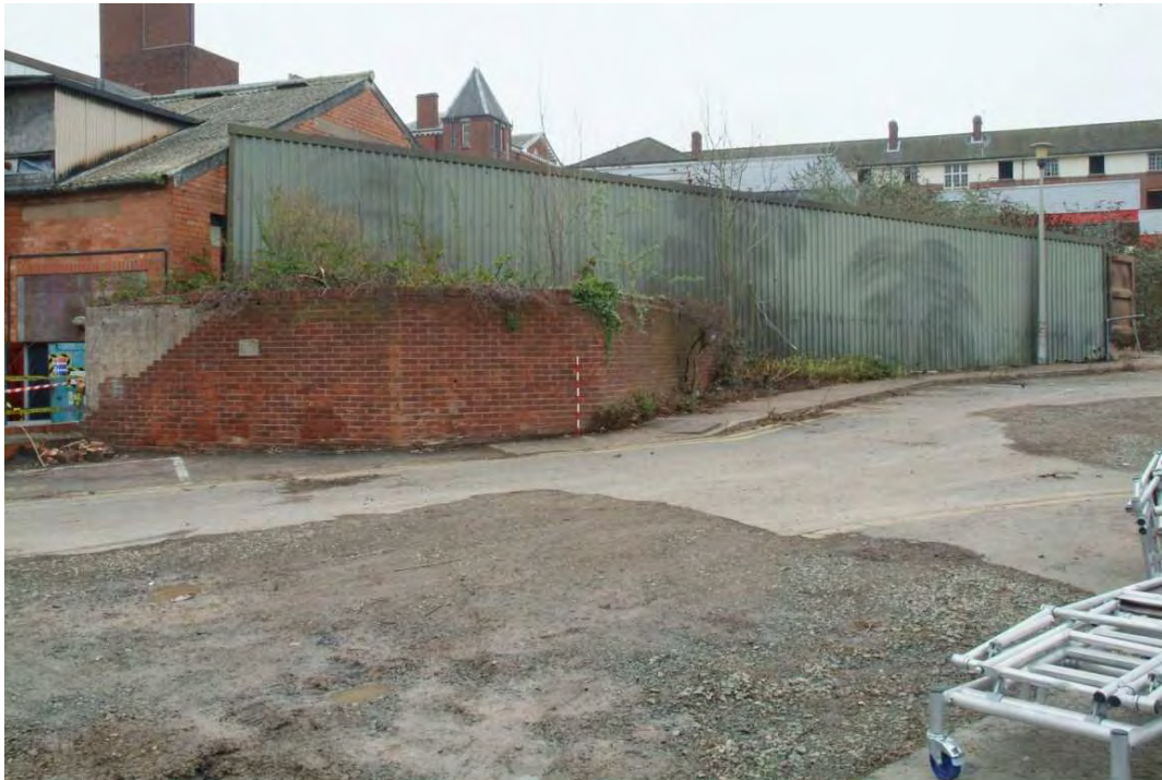
Plate 25.1: Building 25: general view of coal conveyor from the southwest
