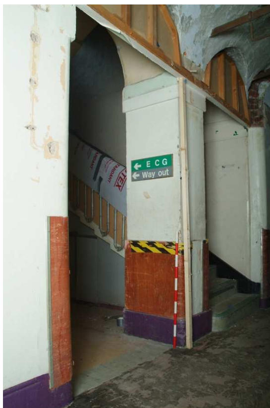
Plate 24.94: Building 24 (LGF): foot of northern stairs, view to the northwest
