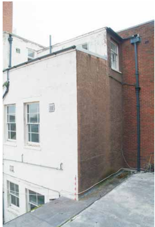
Plate 16.3: Building 16 – eastern elevation above Building 15
