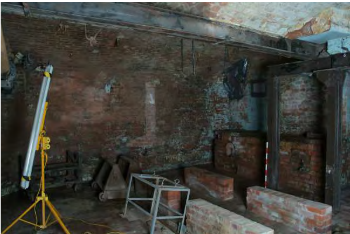
Plate 48.14: Building 48: basement – interior of main eastern part, view to the southeast
