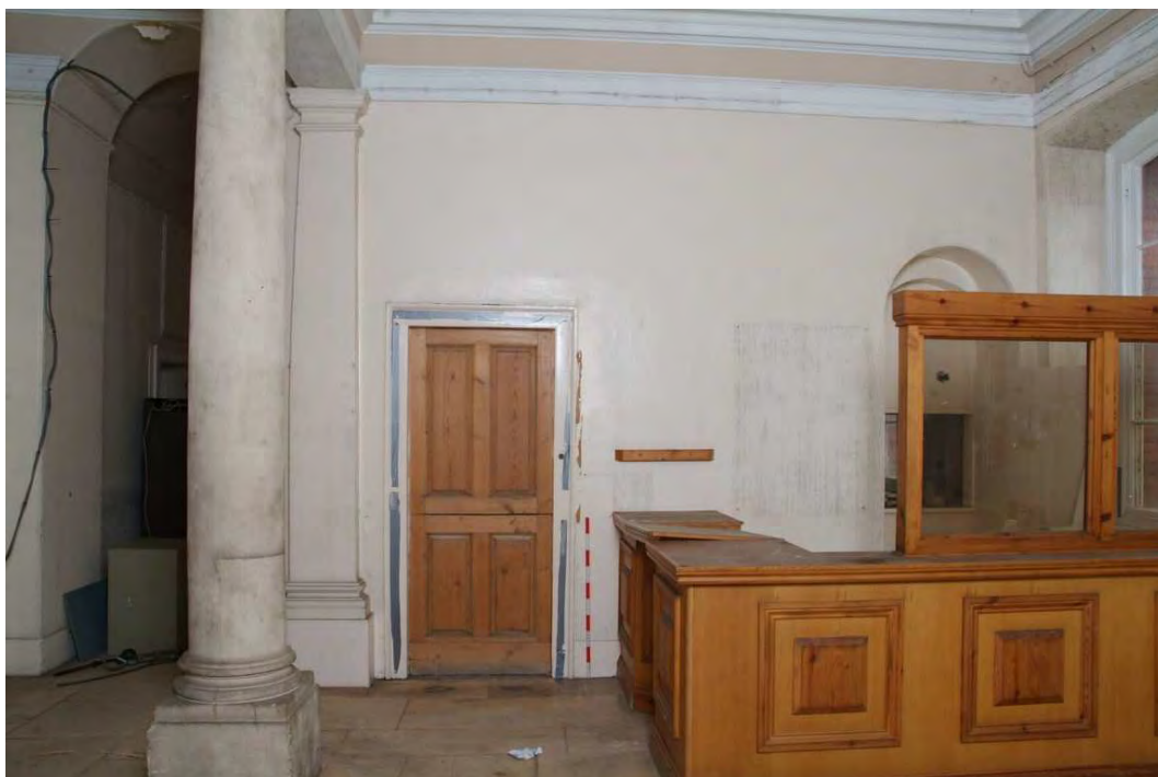
Plate 24.40: Building 24: entrance hall, view to the north
