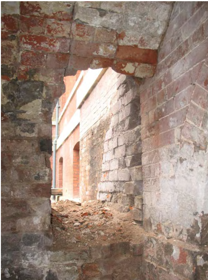
Plate 24.14: Building 24: inserted opening in south side of barrel vault
