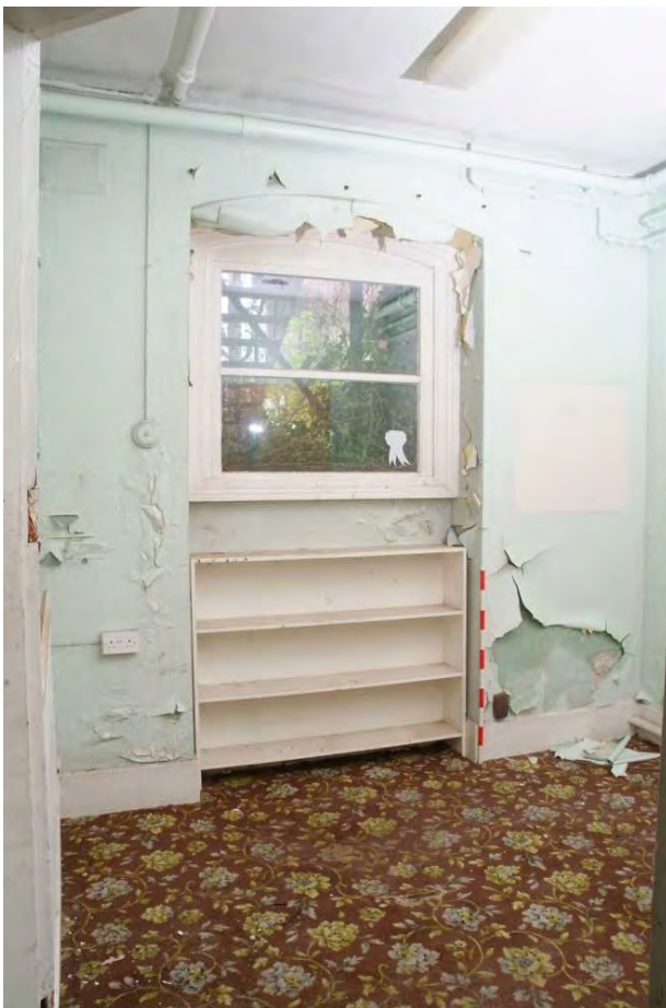
Plate 24.106: Building 24 (LGF): catering office [Room 108], view to the northwest
