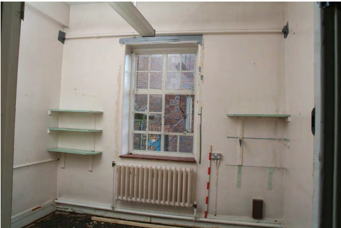
Plate 27.56: Building 27b – ground floor: typical modified bedroom, view to the southeast
