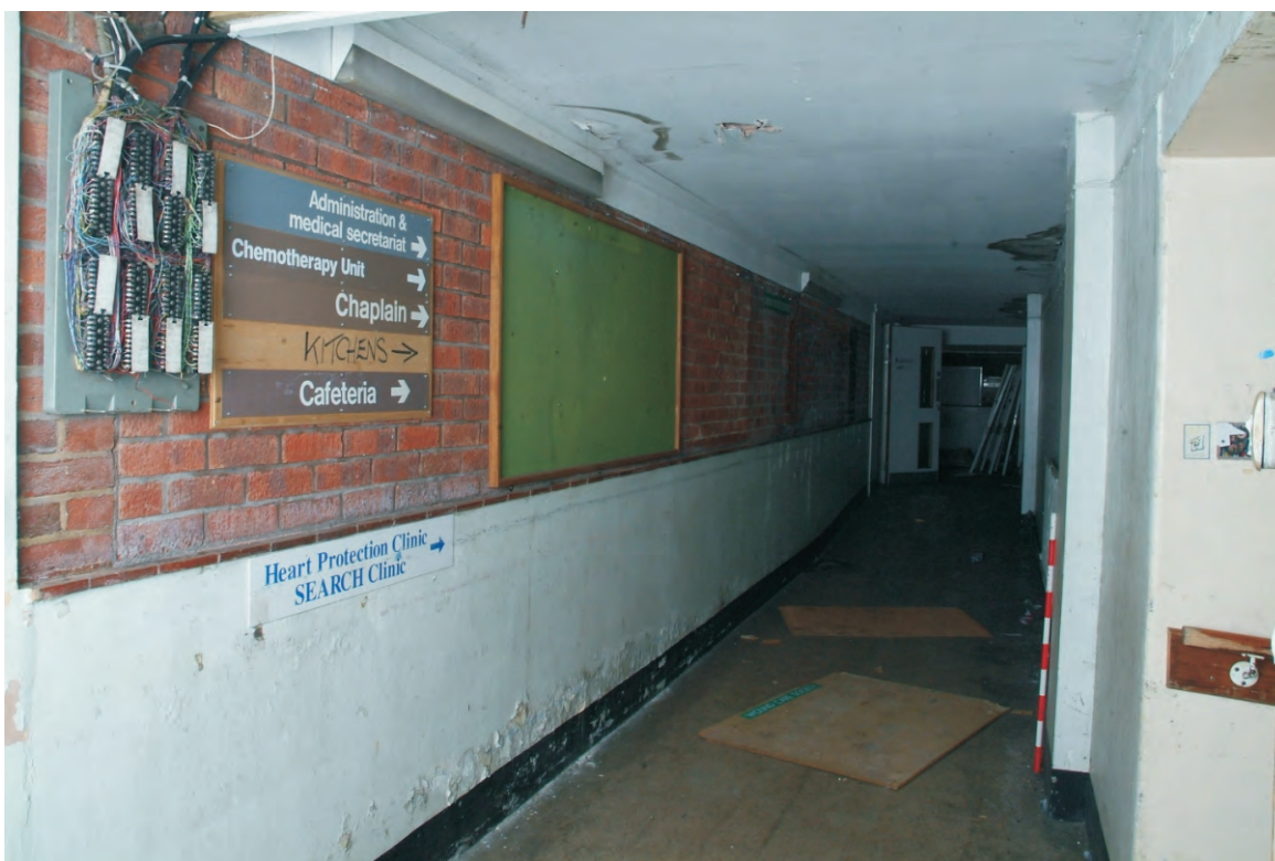
Plate 23.7: Building 23 - interior of the E - W corridor, view to the southwest
