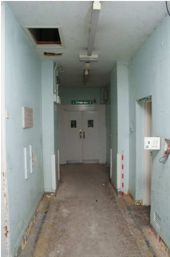
Plate 24.151: Building 24 (FF): central corridor, view to the north
