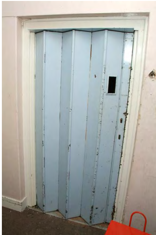
Plate 27.52: Building 27b – ground floor: inserted lift, view to the north
