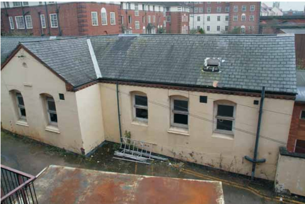
Plate 14.2: Building 14 – northern elevation (western end)
