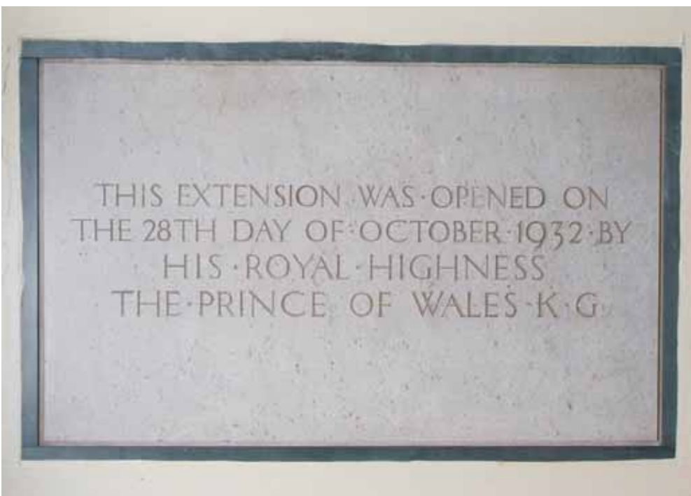
Plate 17.22: Building 17a – ground floor: detail of opening plaque, view to the north
