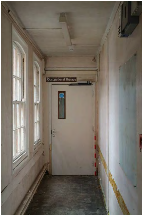
Plate 40.19: Building 40 (UGF): south corridor along western end, view to the north
