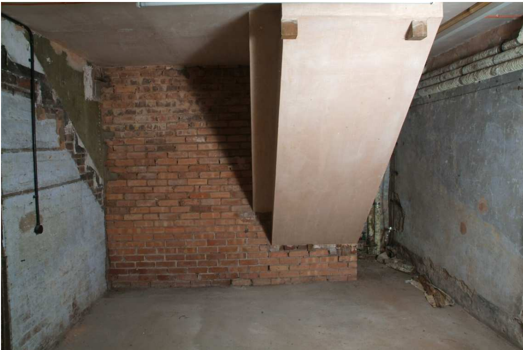
Plate 30.30: Building 30 (LGF): central part of original basement showing inserted stair enclosure and scar of former stairs, view to the south
