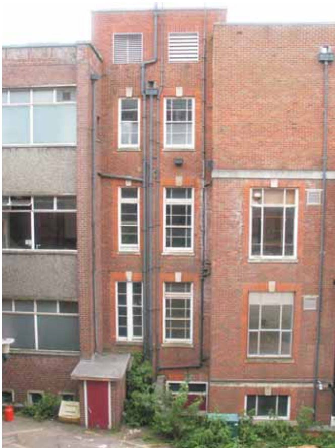
Plate 17.11: Building 17b – northern elevation of post 1938 building, view to the east
