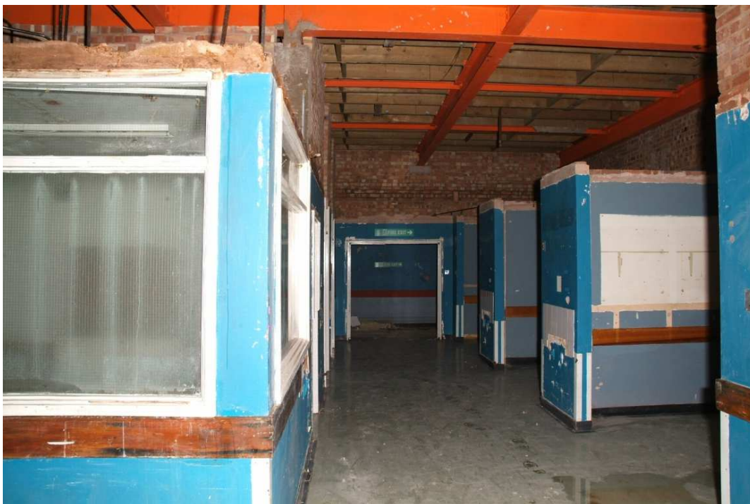
Plate 26.12: Building 26: triage area showing assessment cubicles, view to the east
