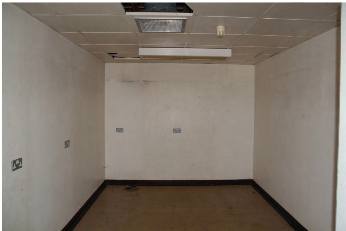
Plate 32.6: Building 32: cold store, view to the east
