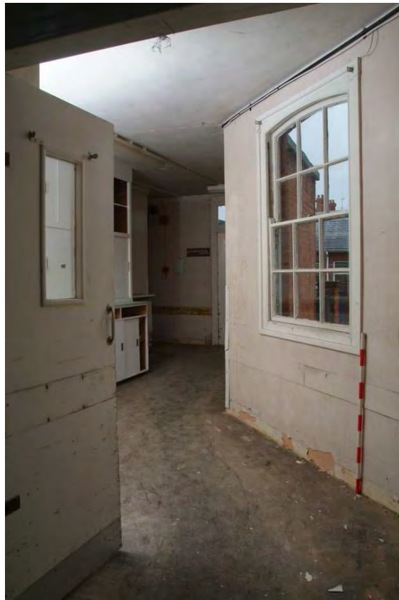
Plate 40.18: Building 40 (UGF): corridor leading from Rushout Ward, view to the southwest
