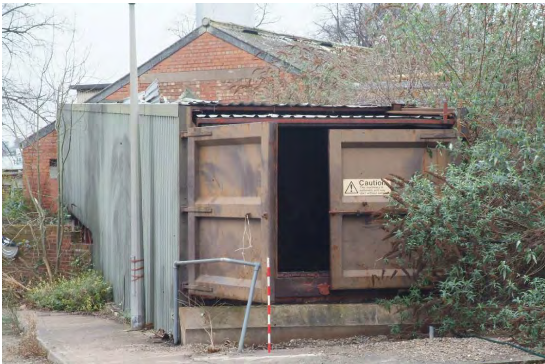
Plate 25.2: Building 25: shipping container doors at the south eastern end
