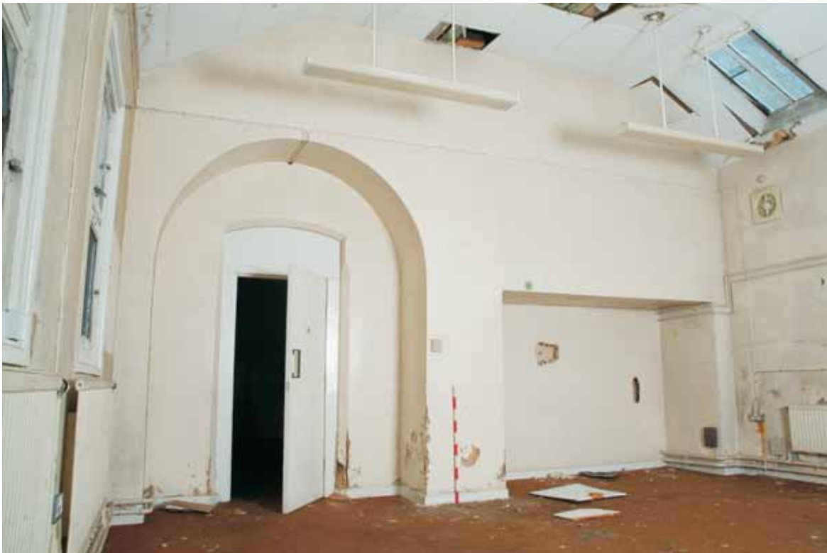
Plate 14.13: Building 14 – original showing blocked fireplace (Right) and original door (left), view to the southeast
