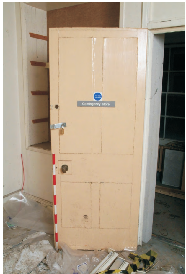
Plate 22.48: Building 22 – connecting range (LGF): door from the Building 17 link corridor to the 'Contingency Store', view to the southeast
