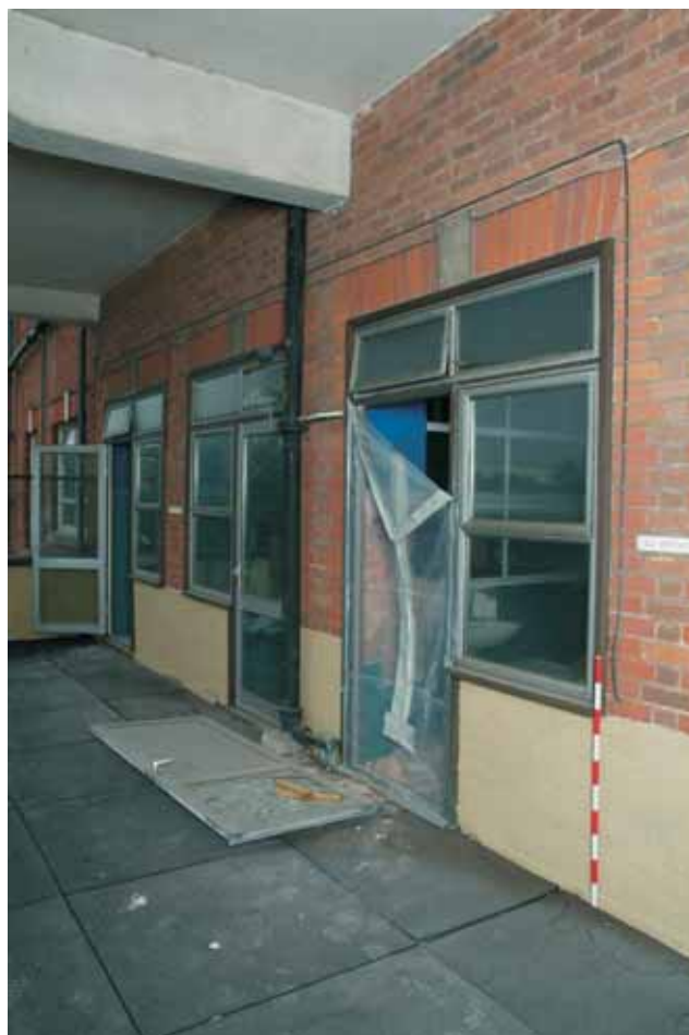
Plate 17.48: Building 17b –first floor: extended window openings on west elevation accessing balcony, view to the northeast
