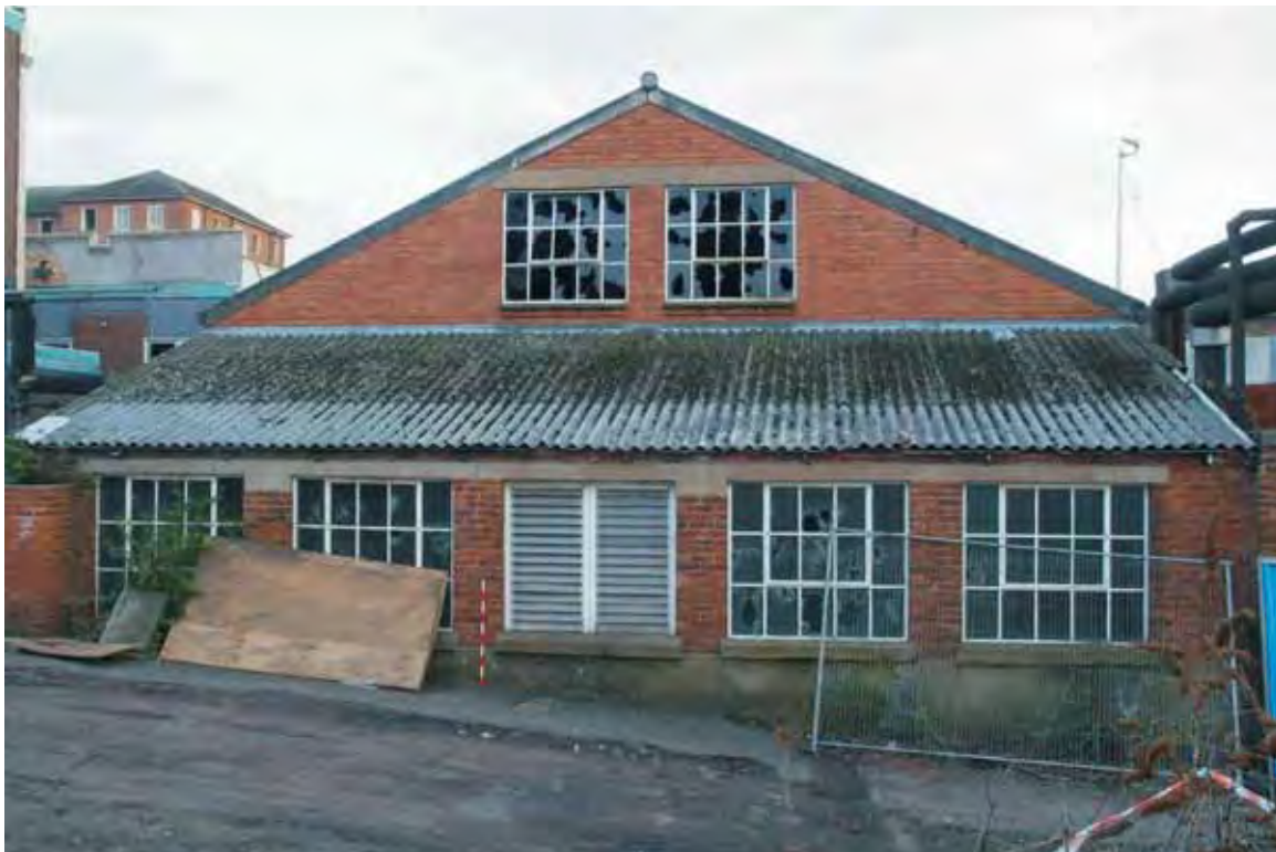
Plate 10.5: Building 10 – northern elevation
