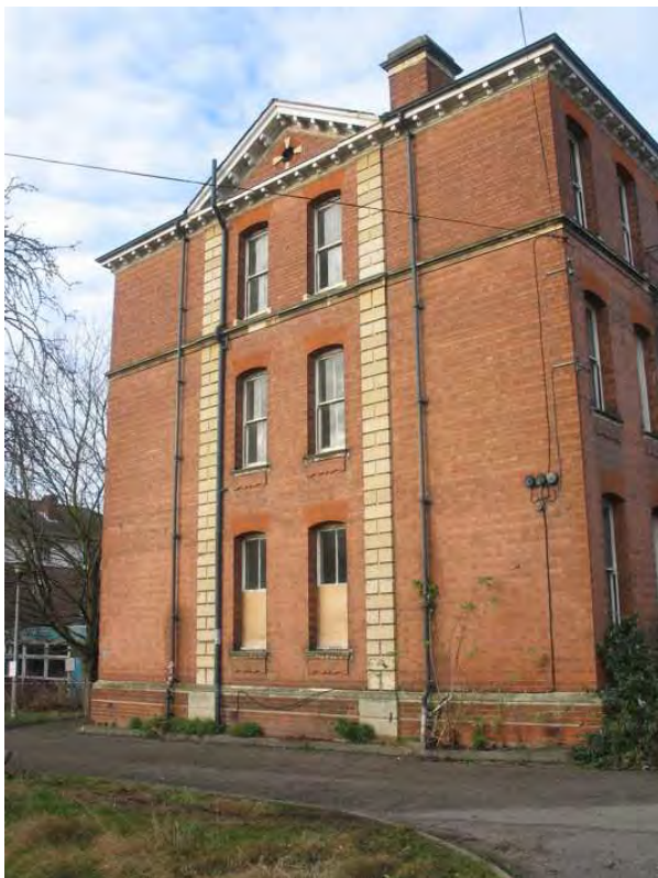
Plate 43.17: Building 43 – south elevation
