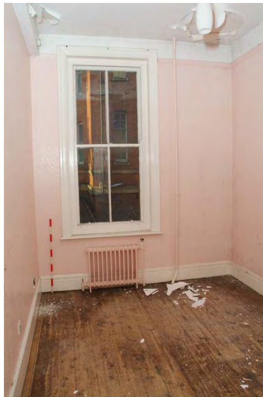
Plate 43.30: Building 43 – ground floor: eastern central bedroom in north range showing off centre window, view to the north
