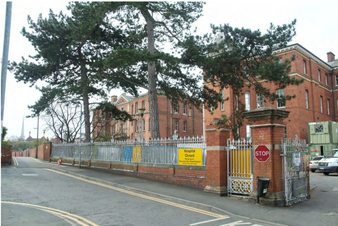
Plate 42.2: Building 42 – General view of railings to the south of the principal entrance
