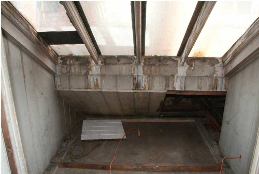
Plate 40.25: Building 40 (UGF): interior of roofspace showing rooflight over western flanking range
