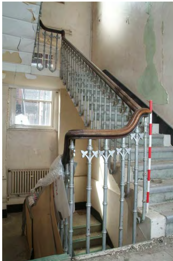
Plate 24.52: Building 24: northern staircase, view to the west
