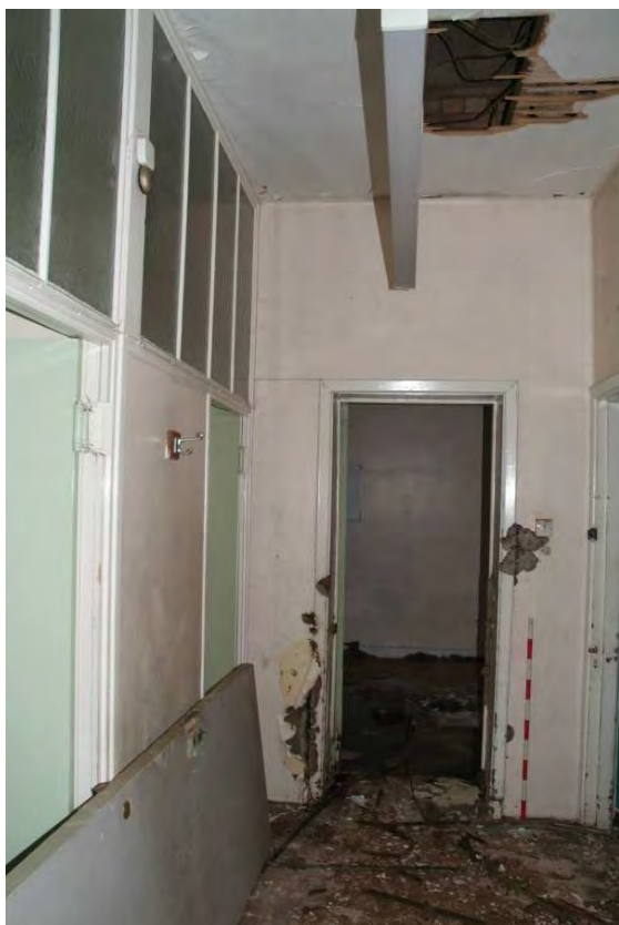
Plate 40.15: Building 40 (LGF): inserted passage [Rom 0.37] showing glazed partition, view to the east
