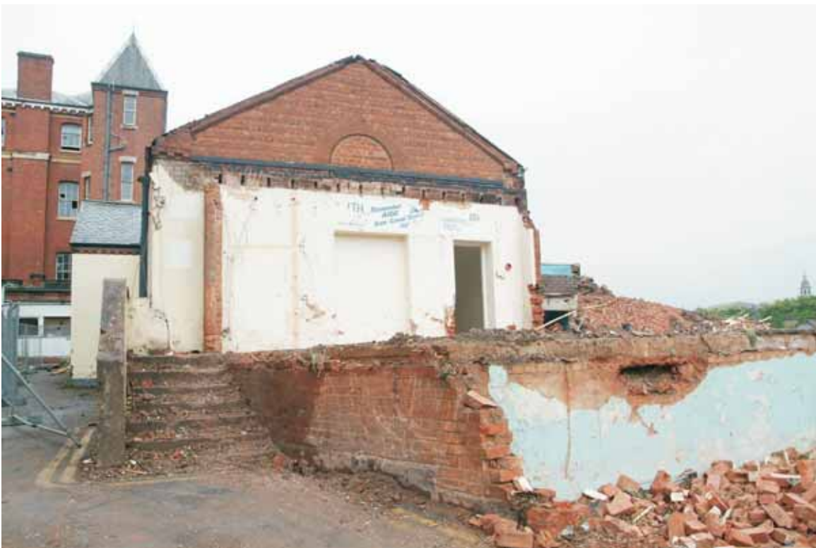
Plate 14.8: Building 14 – western elevation following demolition of Building 13
