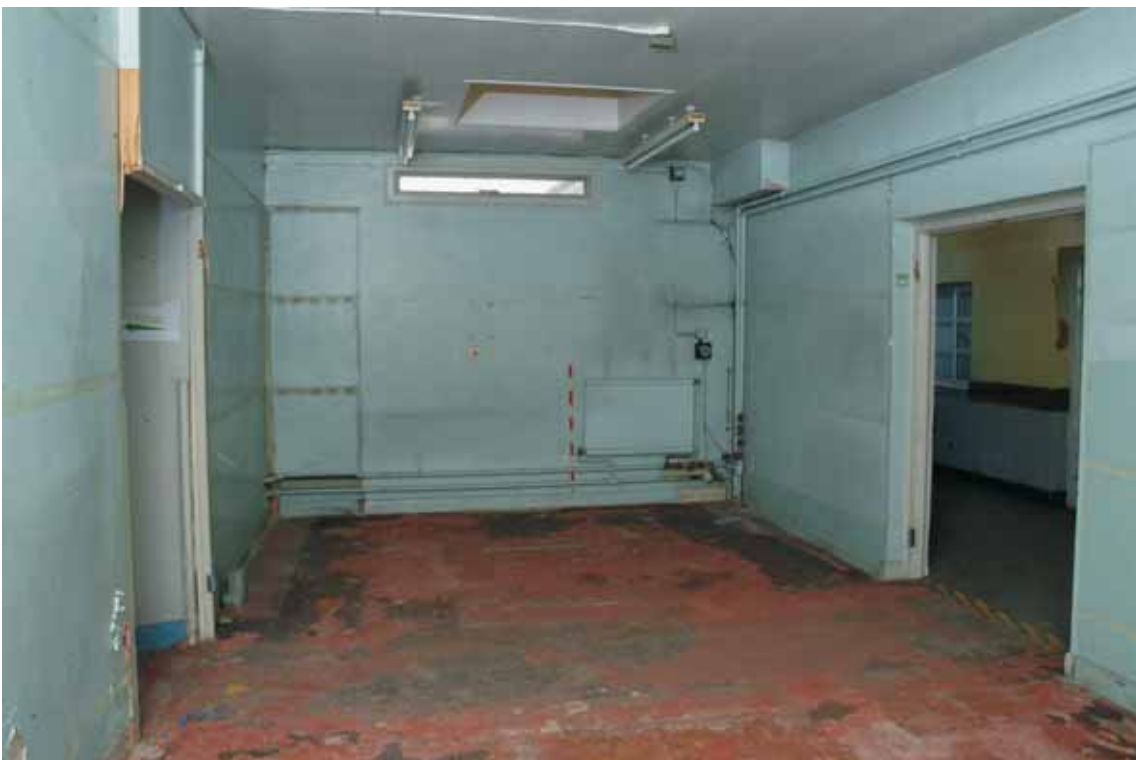
Plate 15.7: Building 15a – interior, view to the south
