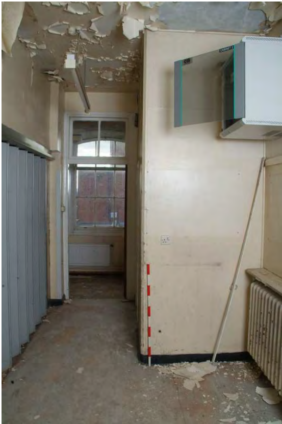
Plate 24.191: Building 24 (SF): area around southern lift, view to the west
