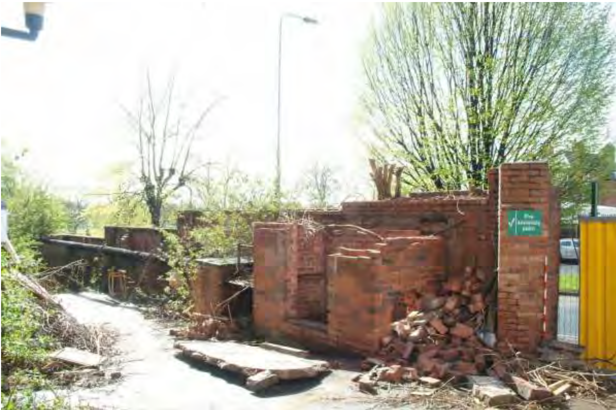
Plate 47.10: Building 47: hospital elevation 01
