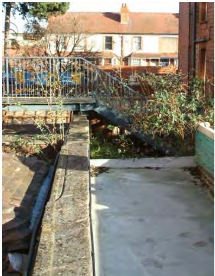
Plate 46.3: Building 46 - southern face to south of Building 35 showing concrete insert for fire escape, view to the northwest
