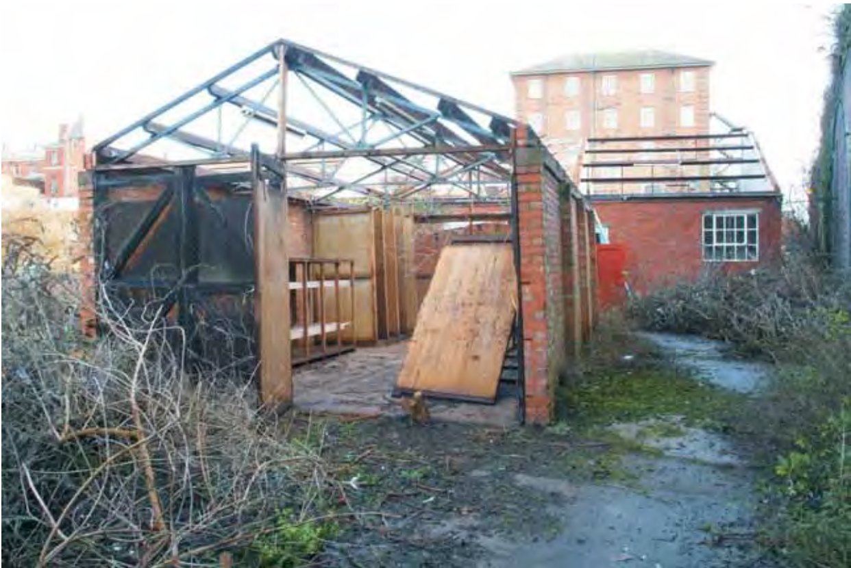
Plate 1.2: Building 1 – western elevation
