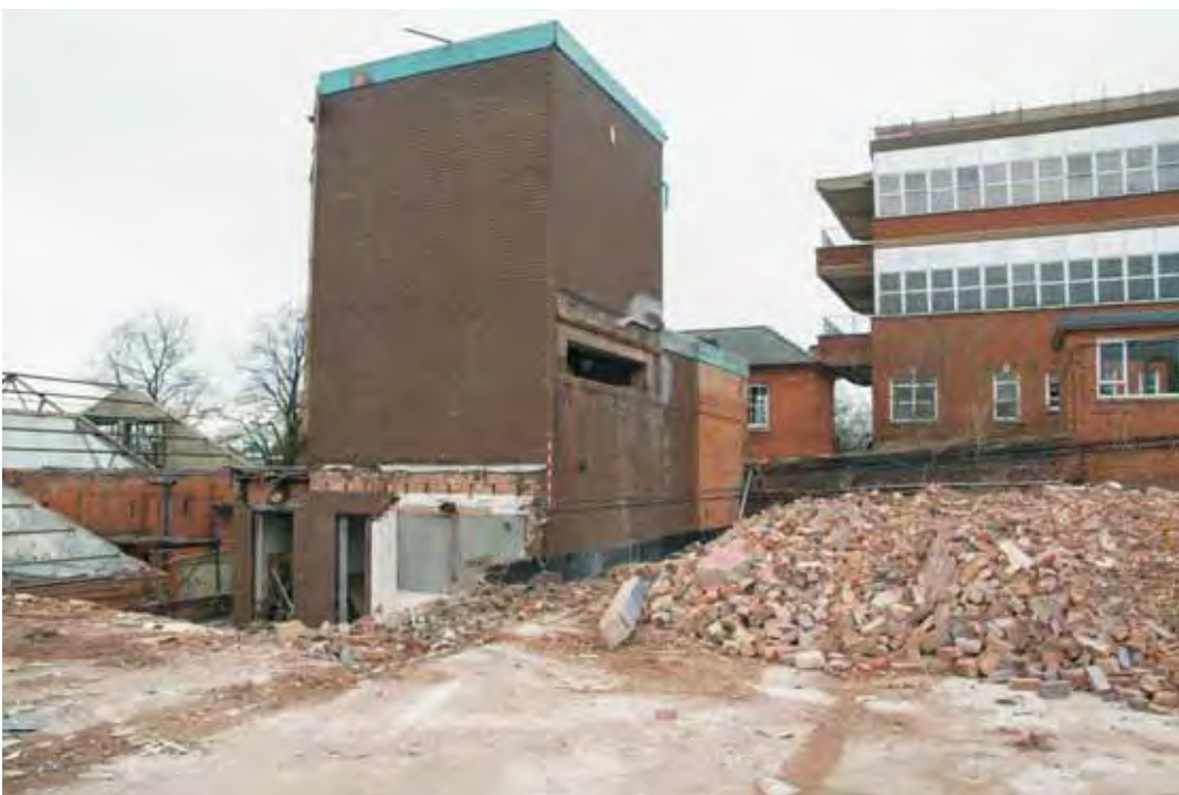
Plate 12.2: Building 12 – south and west elevation
