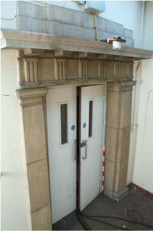
Plate 27.5: Building 27a - southern entrance on eastern elevation, view to the northwest
