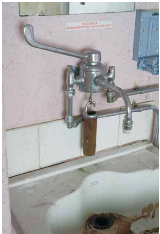
Plate 17.28: Building 17a – ground floor: detail of original sluice sink fittings
