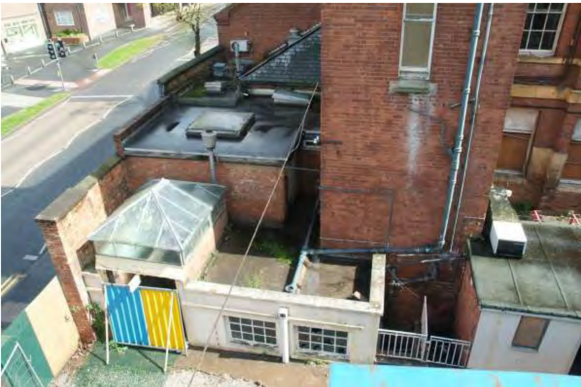
Plate 48.1: Building 48: northern part, view to the northeast
