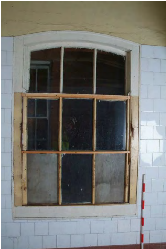
Plate 24.115: Building 24 (LGF): detail of inserted window in blocking wall across former side entrance to kitchens, view to the north
