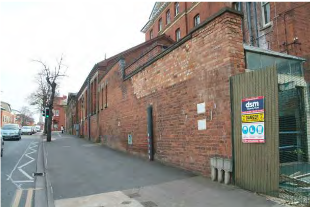
Plate 48.5: Building 48: northern elevation, view to the east
