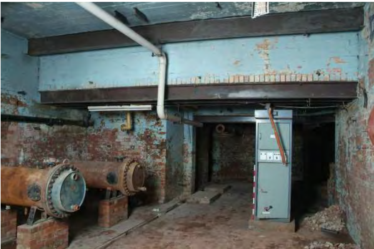
Plate 48.13: Building 48: basement – general interior, view to the northeast
