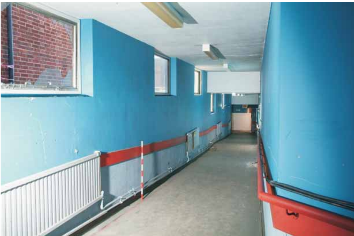
Plate 15.5: Building 15 – interior of east-west section, view to the west
