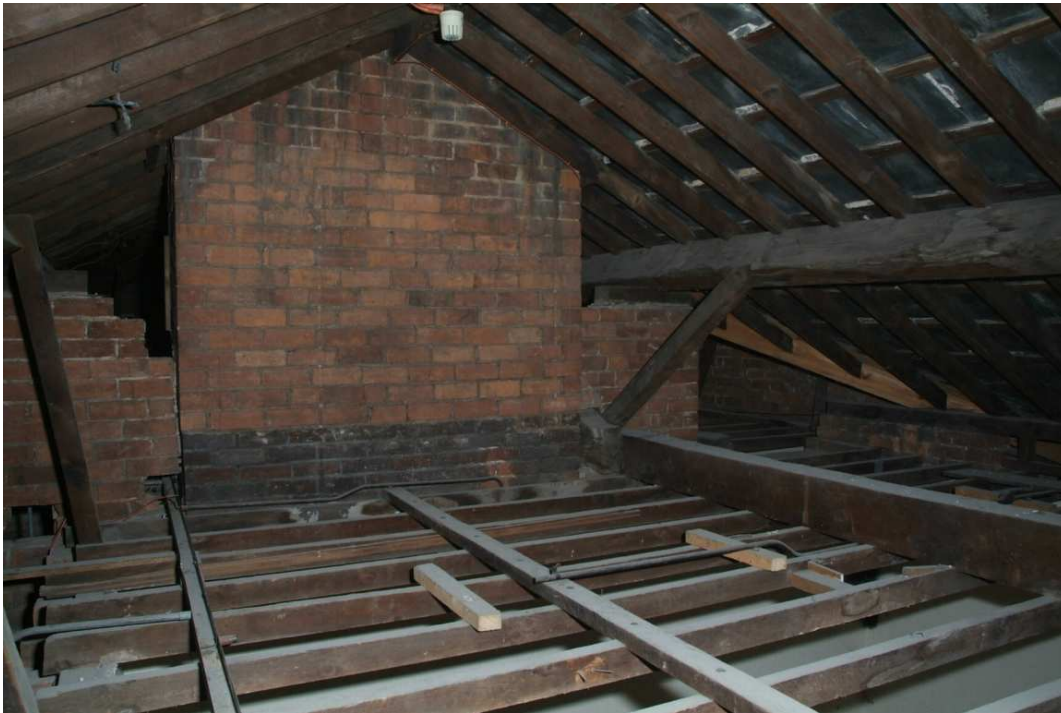
Plate 24.217: Building 24 (Room Structure): chimney showing extension, view to the south
