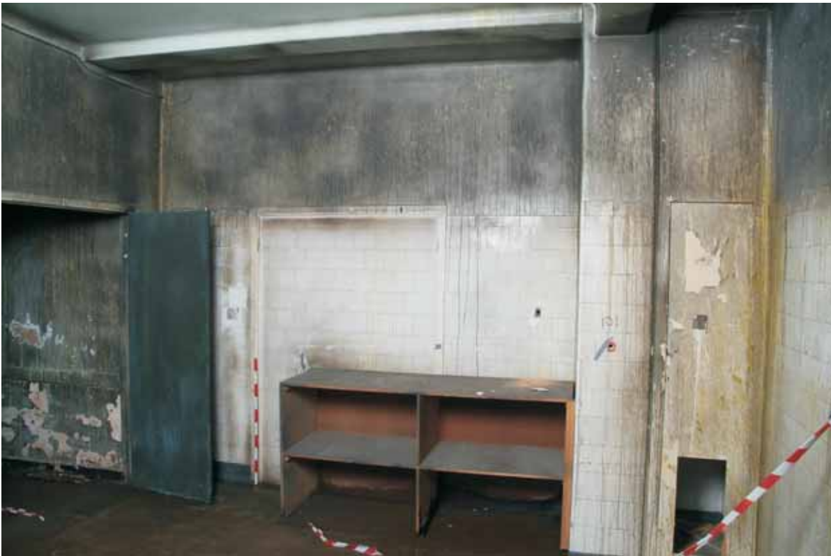
Plate 17.19: Building 17a – basement: tiled mortuary (body store), view to the southwest
