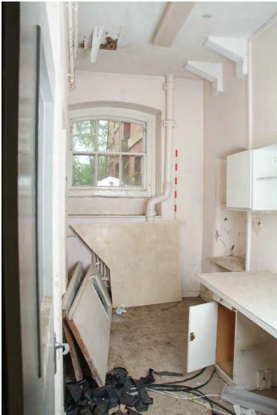
Plate 24.127: Building 24 (LGF): interior of Room 103, view to the east
