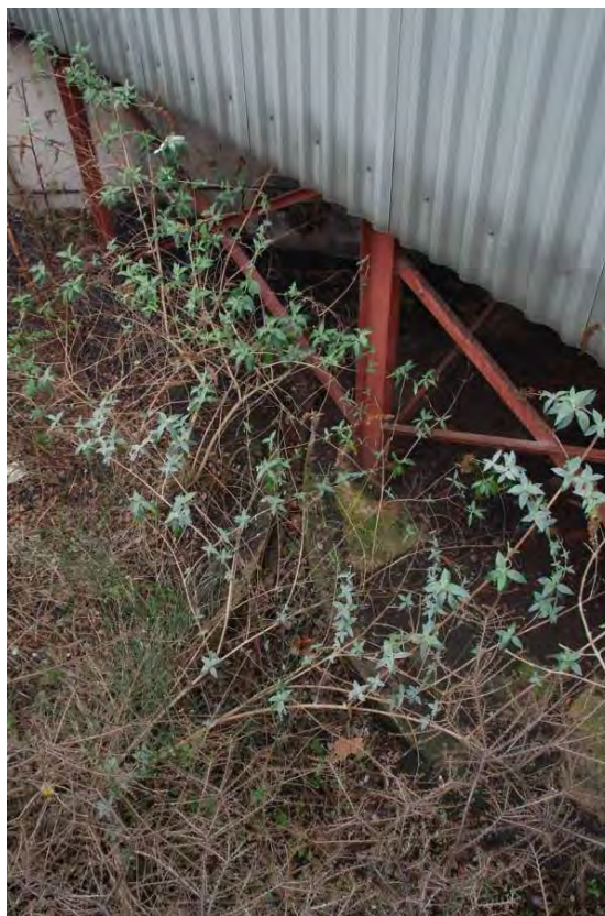
Plate 25.6: Building 25: interior of bunded tank showing conveyor trestles, view to the north
