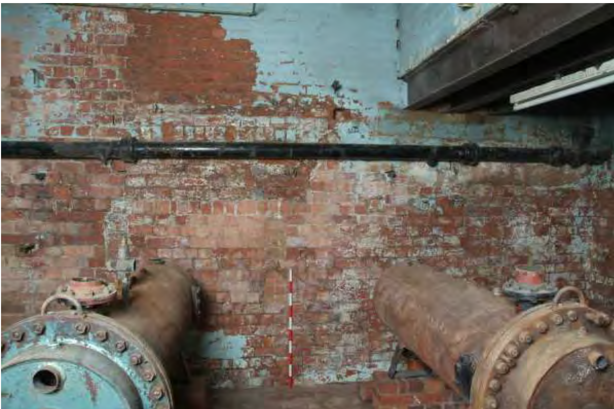
Plate 48.11: Building 48: basement – detail of north wall showing infilled arch
