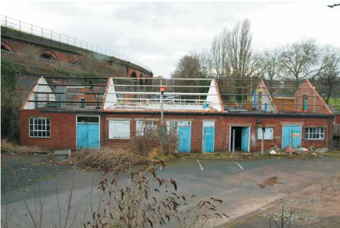
Plate 6.1: Building 6 – Eastern elevation
