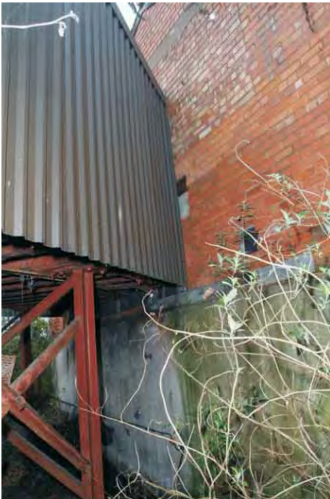
Plate 10.10: Building 10 – east side of (lower) southern elevation
