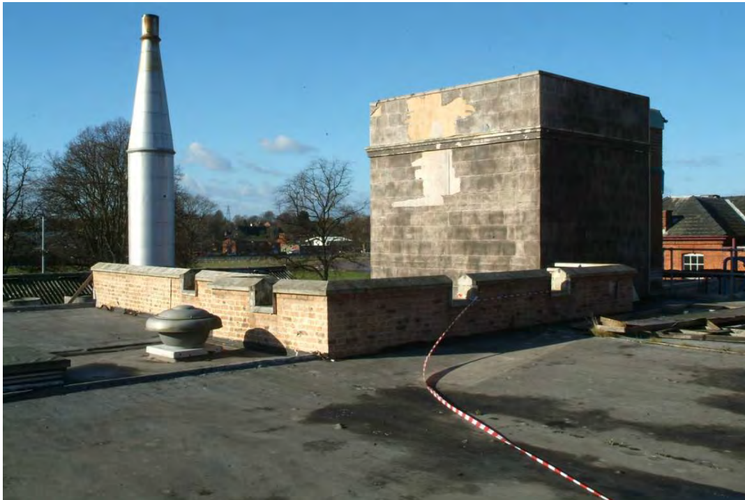
Plate 26.3: Building 26: detail of crenulated parapet, view to the northwest
