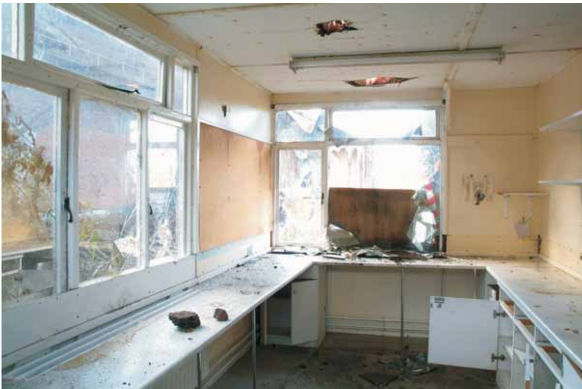
Plate 2.4: Building 2 – interior of southern part, view to the south west
