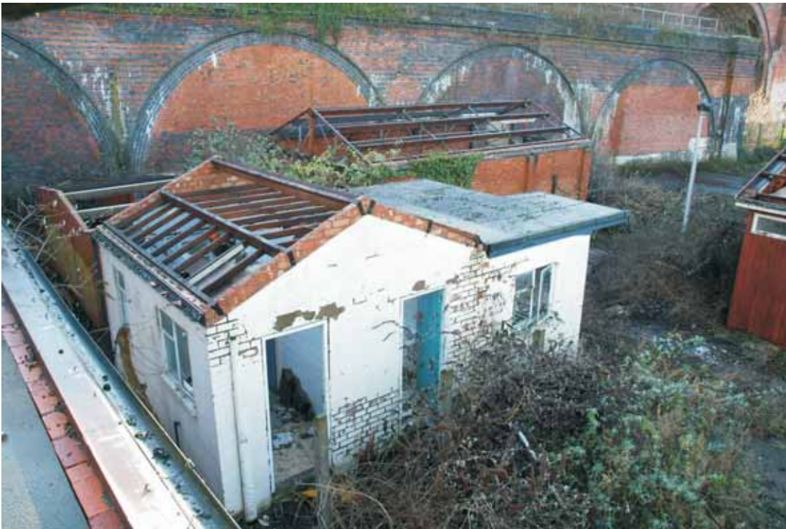
Plate 5.1: Building 5 – eastern and northern elevations (taken from B.6)
