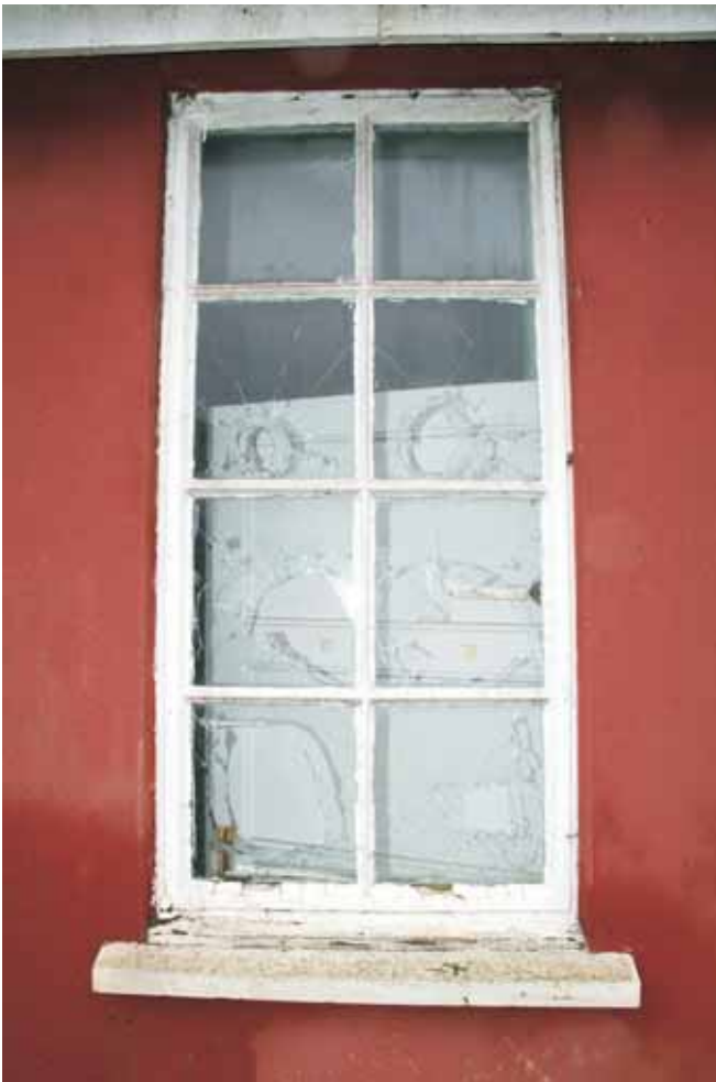
Plate 3.4: Building 3 – detail of typical window
