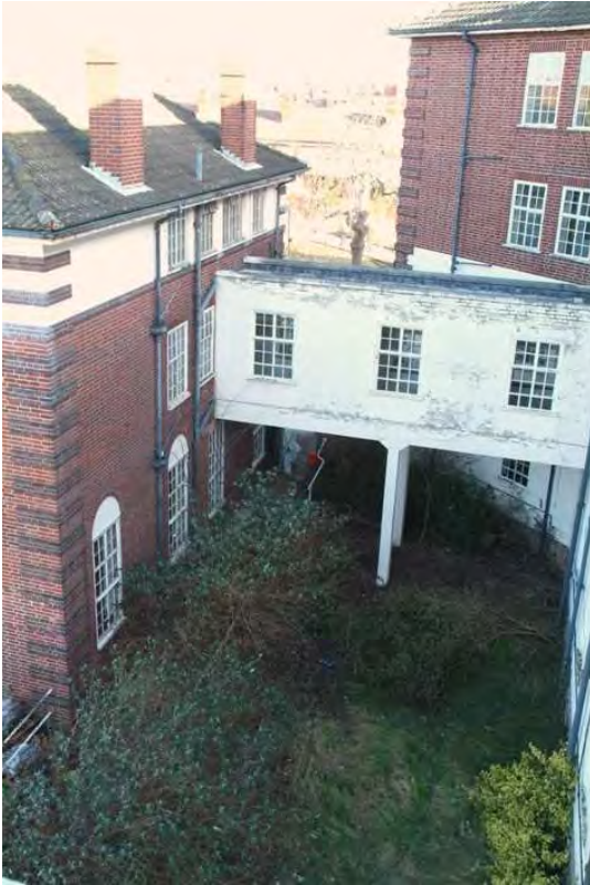
Plate 27.7: Building 27a – southern elevation, view to the northeast
