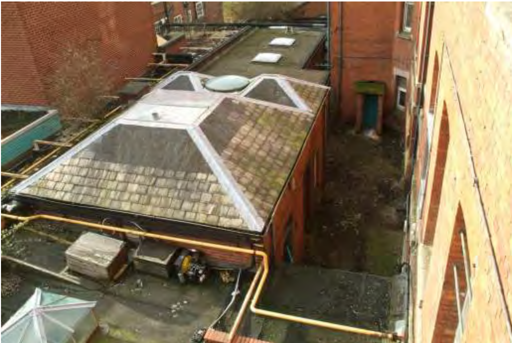
Plate 34.2: Building 34 – roof, view to the southwest
