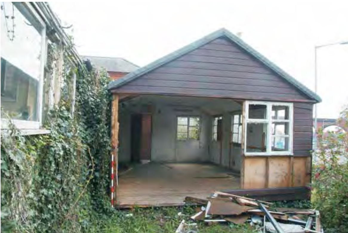
Plate 21.2: Building 21 – north elevation showing interior, view to the south
