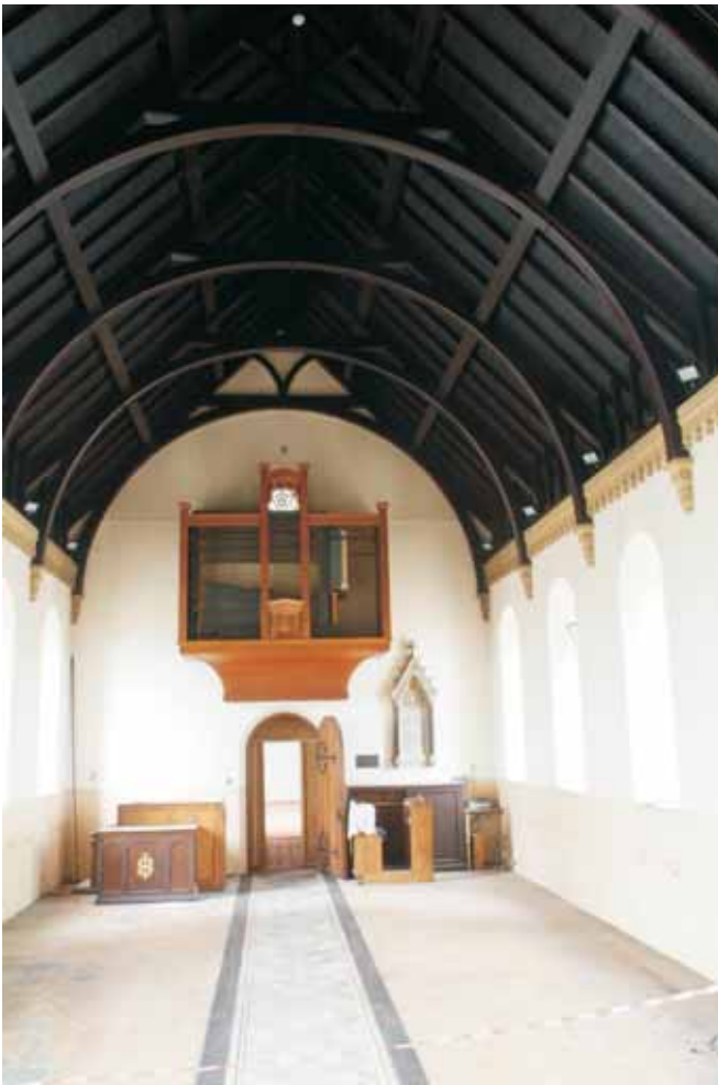
Plate 22.17: Building 22 – nave: interior, view to the east
