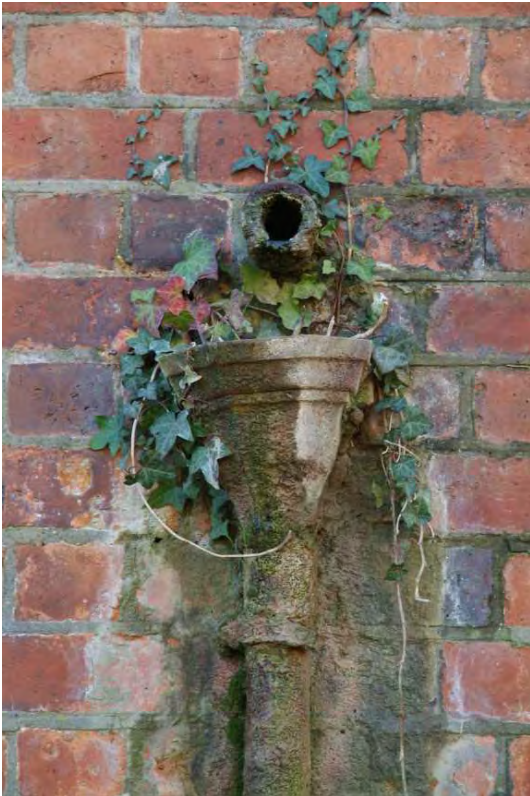
Plate 44.5: Building 44 – detail of rainwater hopper
