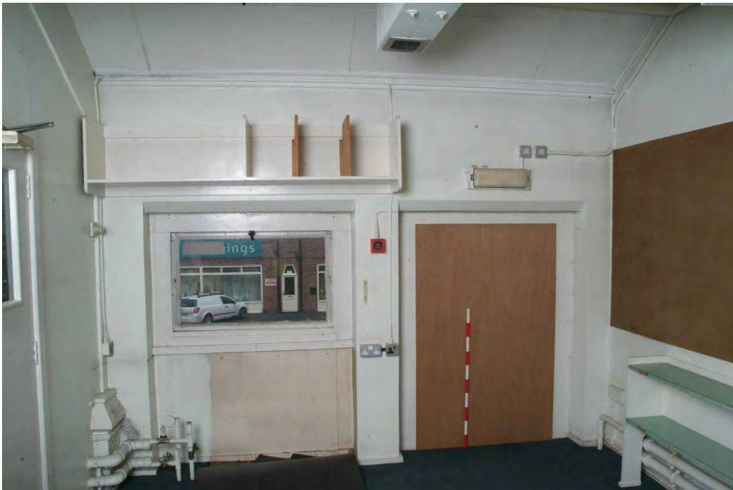
Plate 41.16: Building 41: mezzanine office showing blocked window, view to the north
