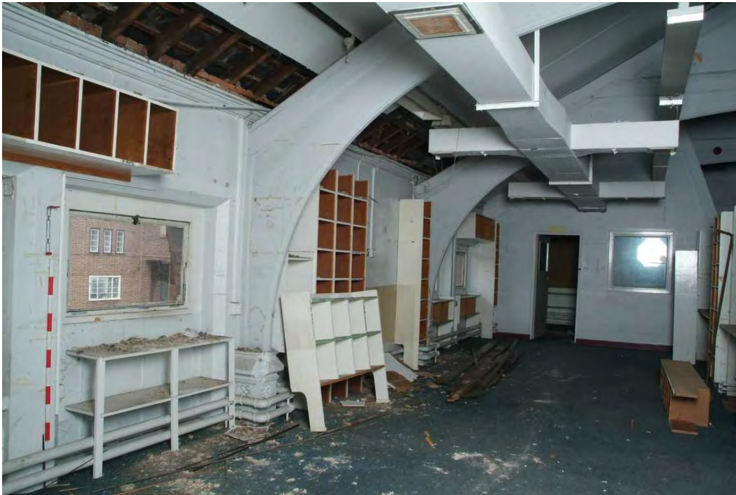
Plate 41.15: Building 41: mezzanine floor, view to the east
