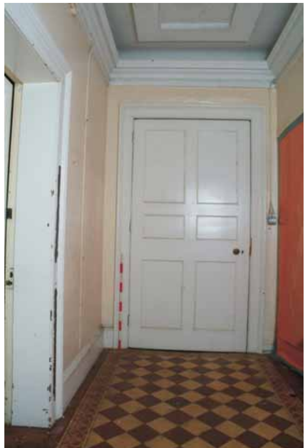
Plate 22.36: Building 22 – connecting range: central corridor on upper ground floor, view to the east
