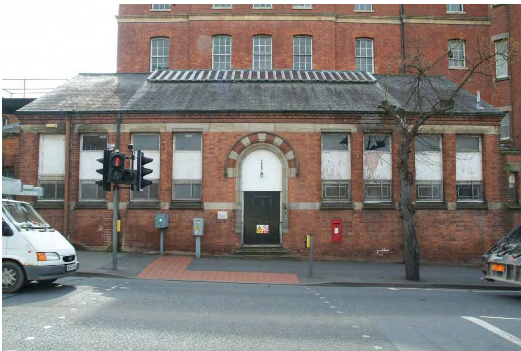
Plate 41.1: Building 41: northern elevation
