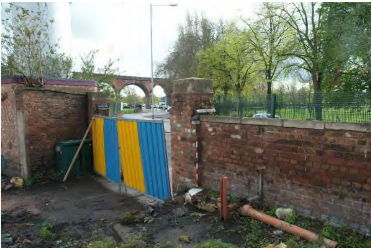
Plate 47.15: Building 47: hospital elevation 06
