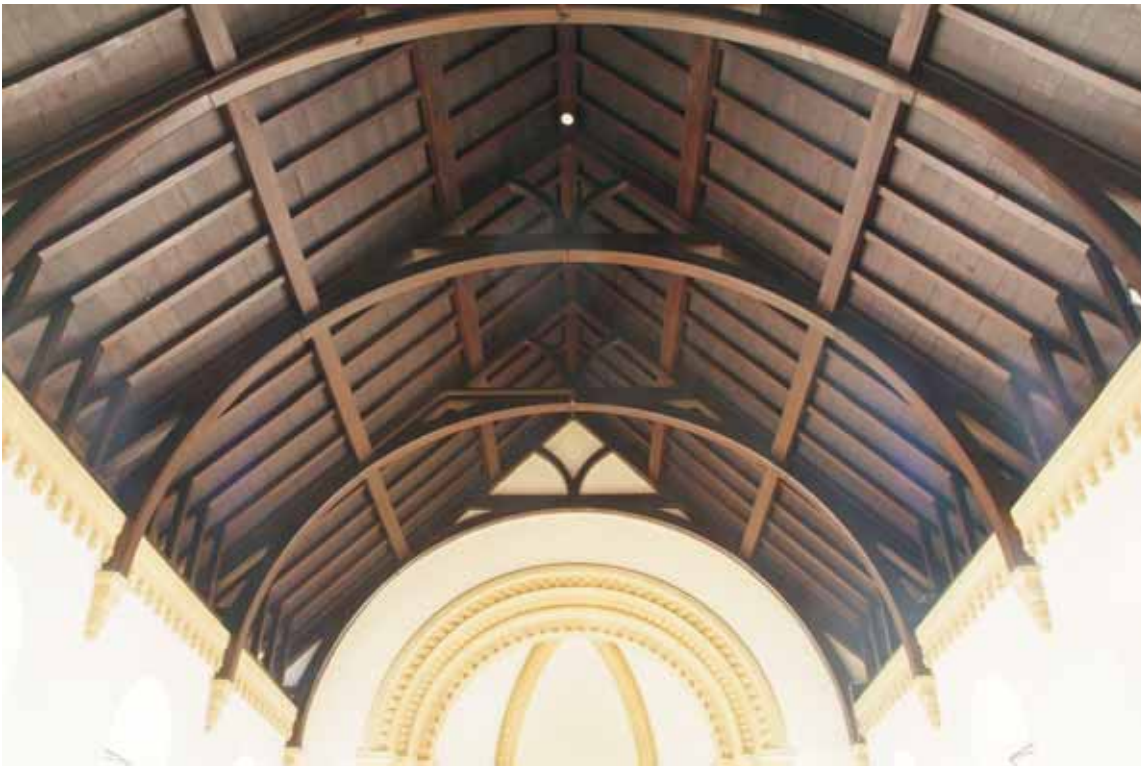
Plate 22.21: Building 22 – nave: roof structure, view to the west
