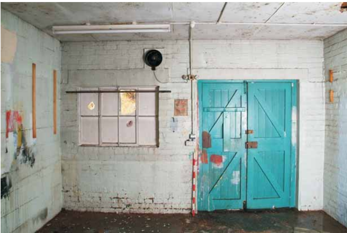
Plate 6.12: Building 6 – interior of former central workshop, view to the northeast
