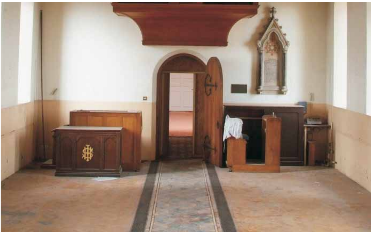
Plate 22.18: Building 22 – nave: detail of internal east elevation showing external door hinges, view to the east
