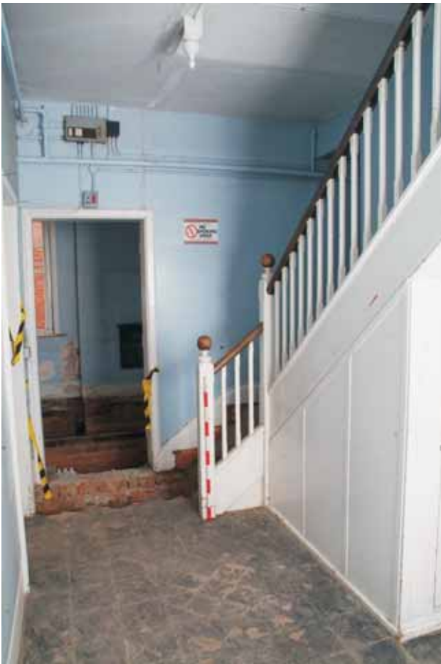
Plate 18.23: Building 18 – ground floor: duct passing beneath the floor of the entrance hall, view to the southwest
