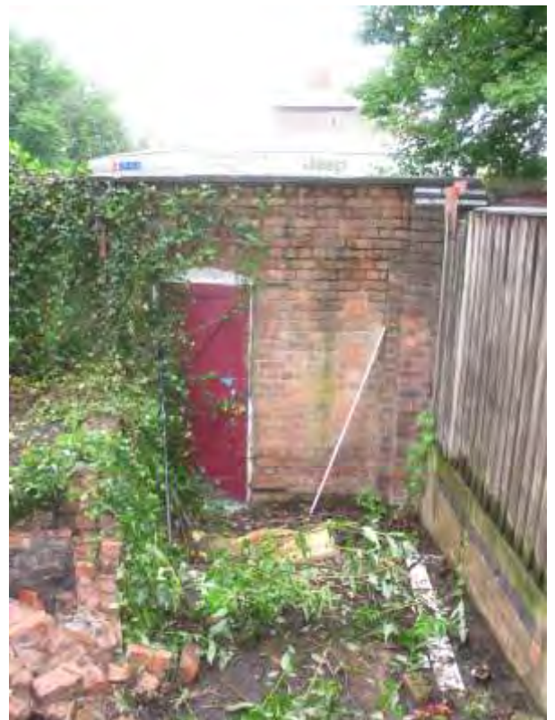
Plate 47.11 & 11a: Building 47: hospital elevation 02
