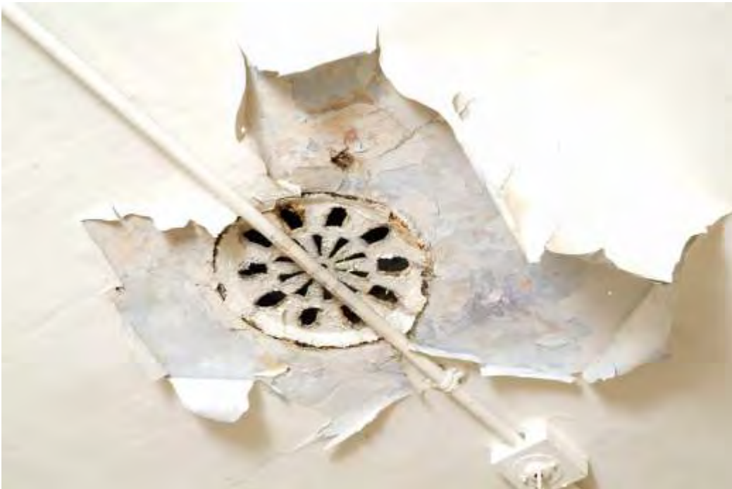
Plate 34.10: Building 34 – detail showing roof vent in eastern part
