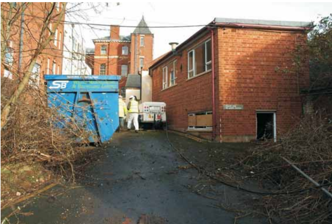
Plate 13.1: Building 13 – View east along the western access road showing the northern and western elevations
