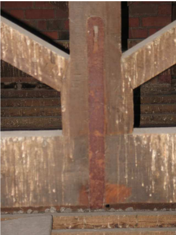
Plate 43.75: Building 43 - roof space: detail of king post attachment to tie beam
