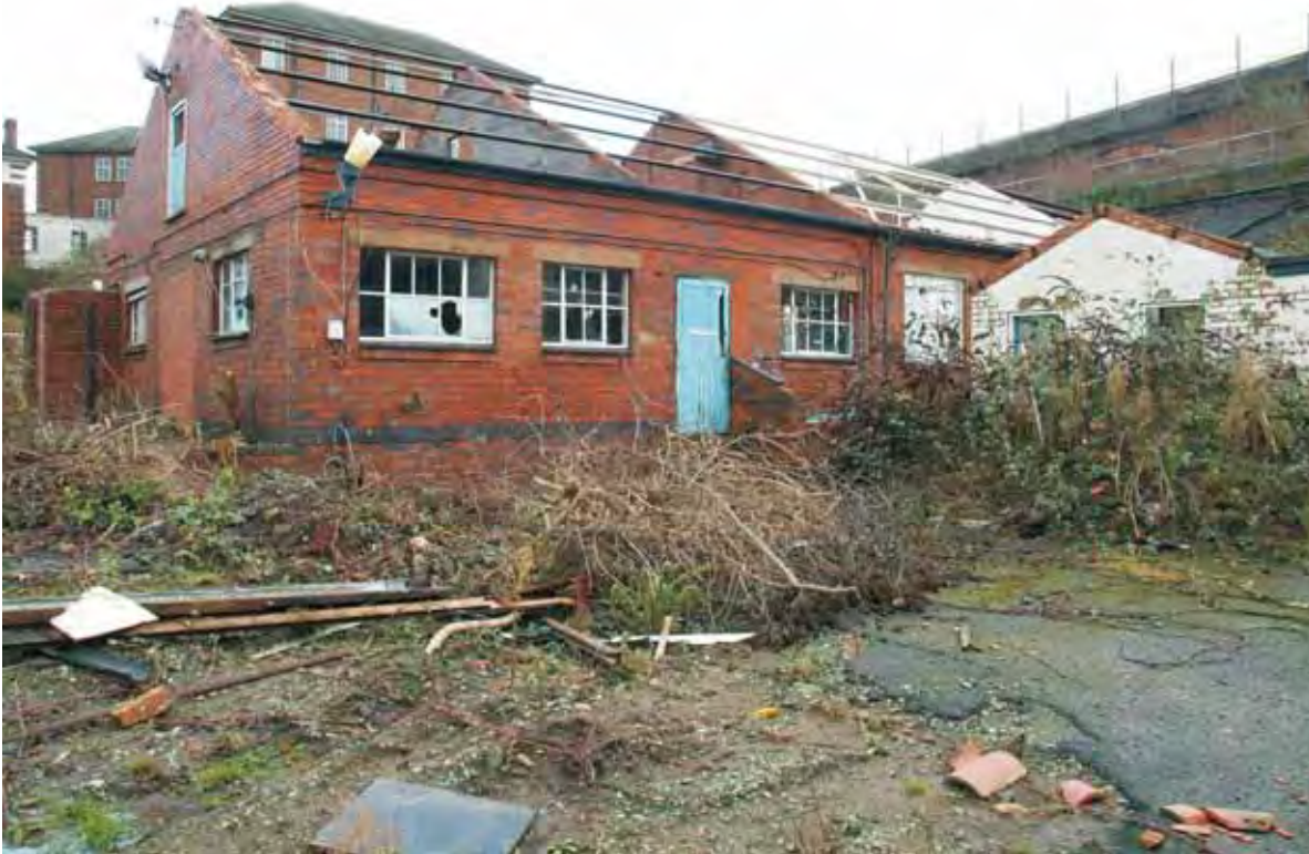
Plate 6.3: Building 6 – western elevation
