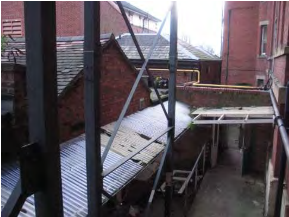
Plate 35.1: Building 35 – general view of northern elevation, view to the southwest
