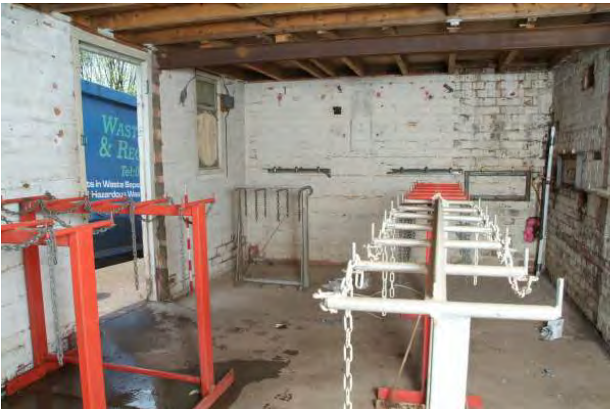
Plate 48.6: Building 48: interior of southern part, view to the north
