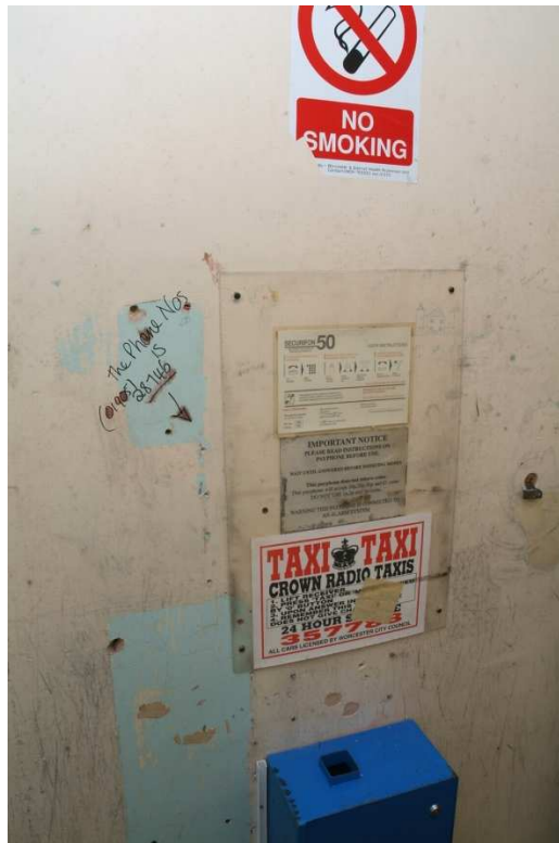
Plate 27.70: Building 27b – first floor: former payphone area showing graffiti, view to the southwest
