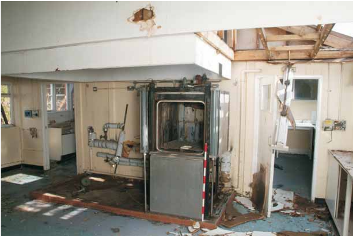
Plate 20.7: Building 20 – sterilizing equipment in the linking range, view to the south
