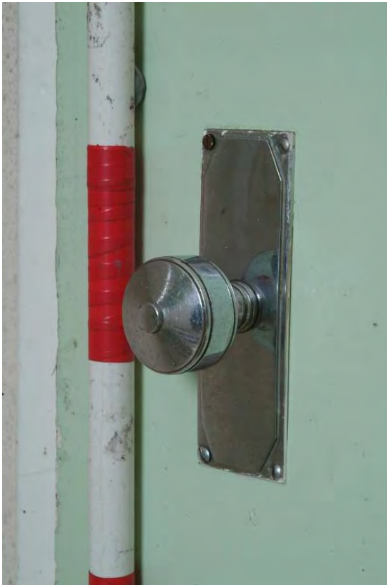
Plate 40.17: Building 40 (LGF): detail of relocated door handle in Room 0.36
