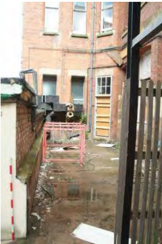
Plate 48.4: Building 48: east elevation of western part, view to the north
