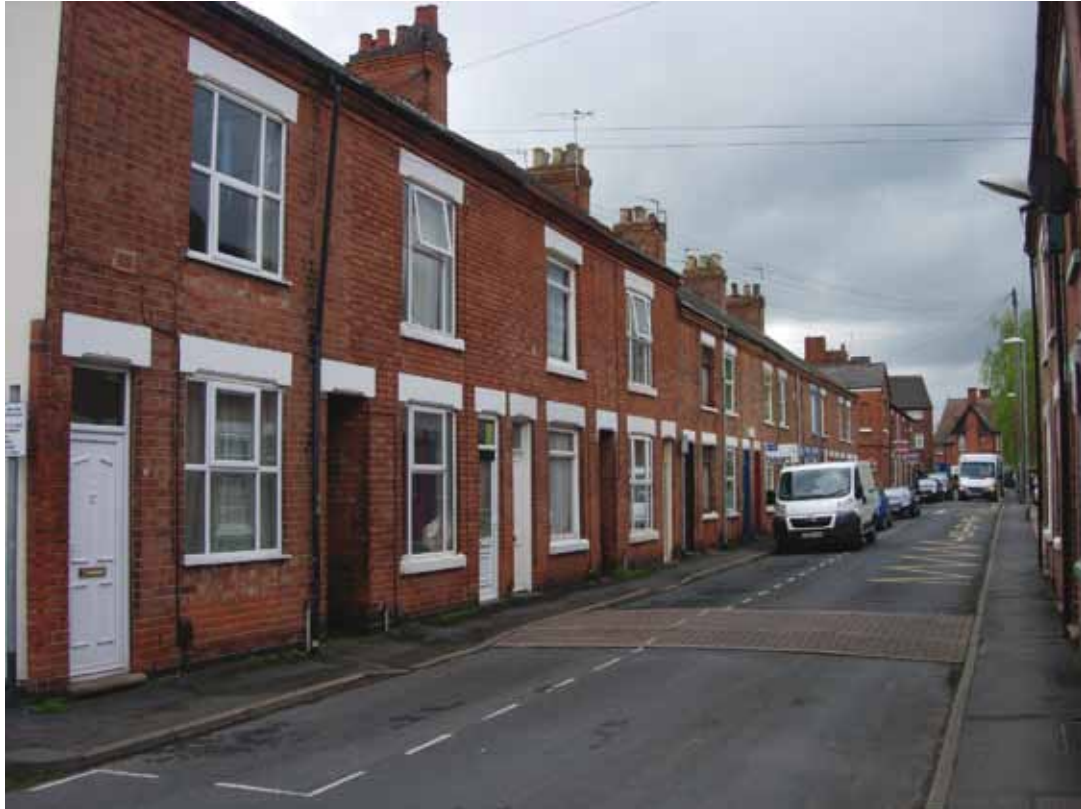
Figure 81. Pre-1880s Terrace Housing: Loughborough
