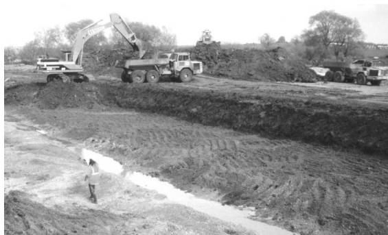
Plate 2 General view during stripping of alluvium to the north of barrow 2
