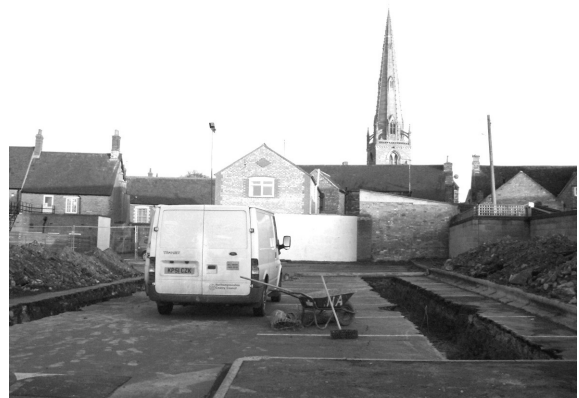
Plate 1 Trenches cut through car park tarmac
