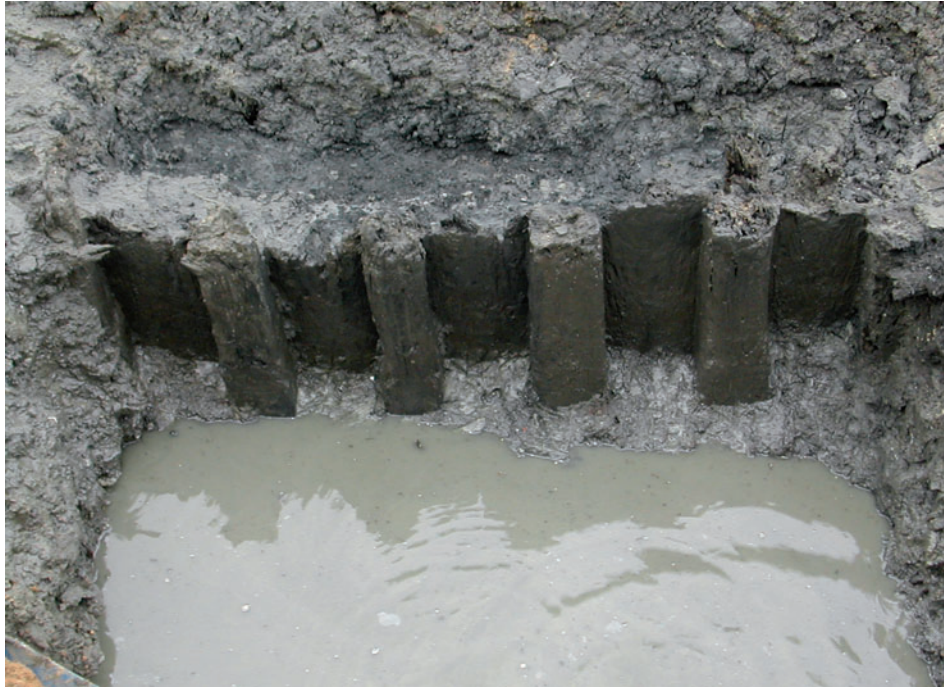
Fig 8 The exposed face of the timber and plank revetment
