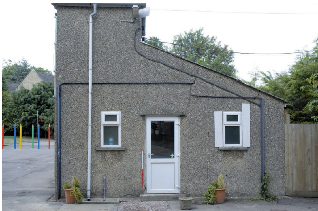
Fig 9 The eastern elevation, showing the raised water tank storage over the service rooms
