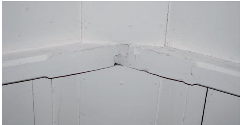
Fig 8 Detail of apex of ribs, showing halved joint and chamfering
