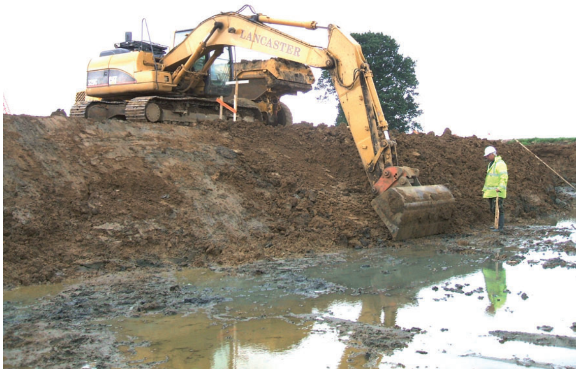
Fig 7 Machining of new river channel
