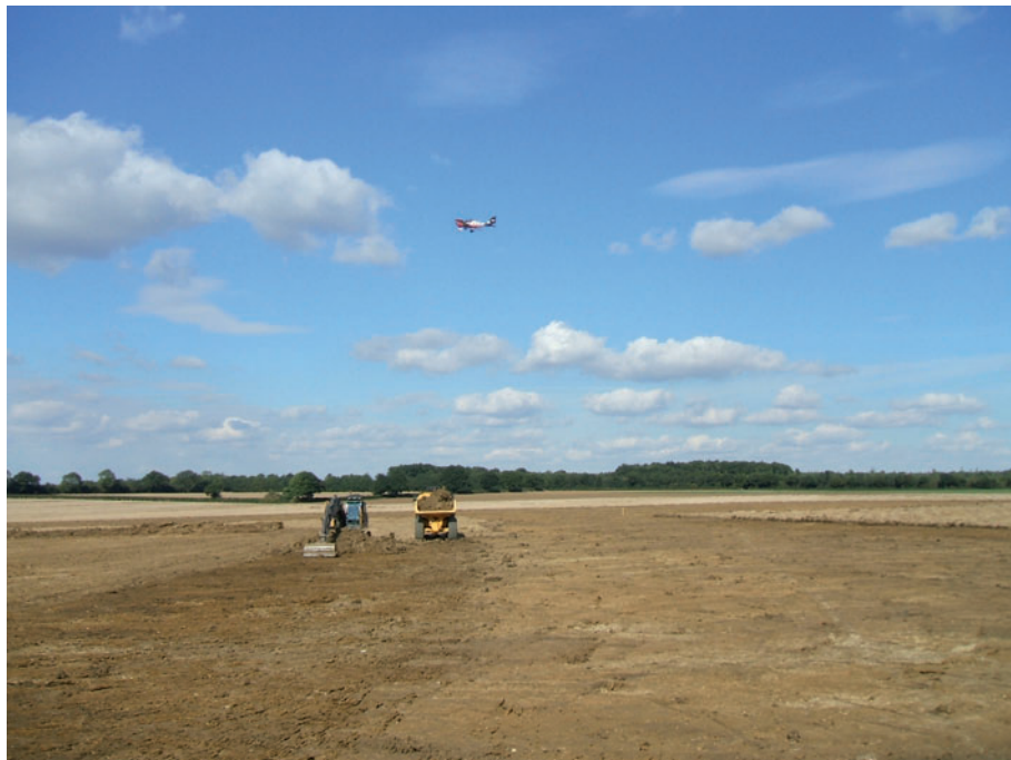
Fig 4 View of the site during topsoil stripping, looking north-east
