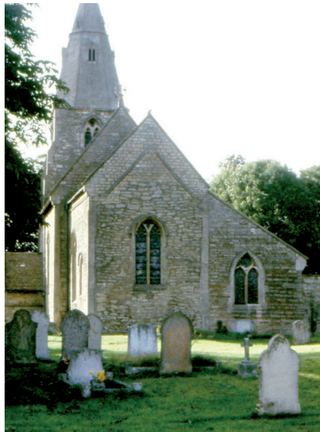
Fig 8 View of Wittering church, showing the Anglo-Saxon chancel and the later raised roof line (photograph, A Chapman)
