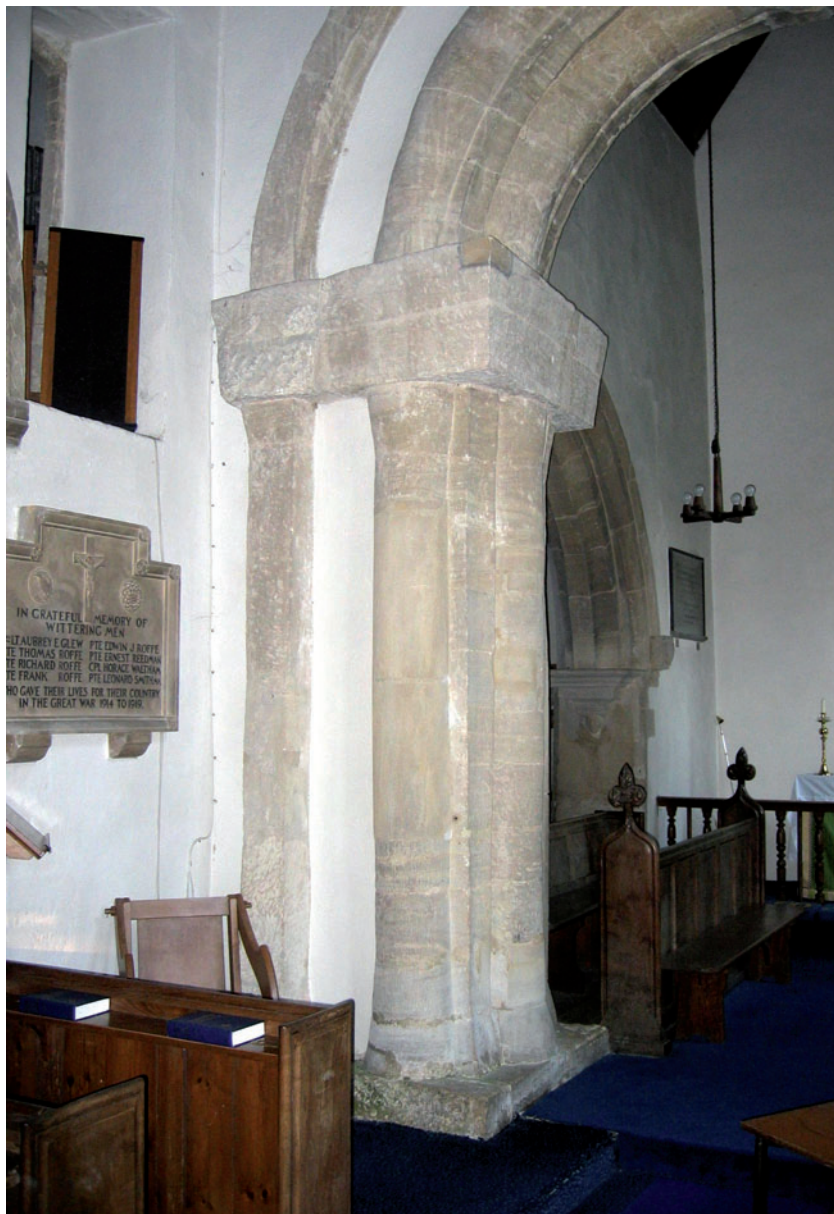
Fig 10 The north jamb of the chancel arch at Wittering, which is here viewed from the nave, exhibits typical Anglo-Saxon characteristics; however, many stones have been replaced, but the original through stone at its foot reveals that the complex carvings were created from a single stone.
