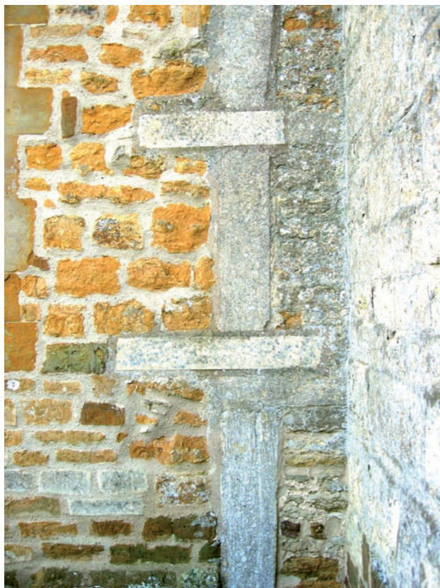
Fig 12 The north-west quoin of Pattishall church has been rebuilt to include stones of Middle Jurassic oolite to help to tie the aisle (left) to the original Anglo-Saxon nave
