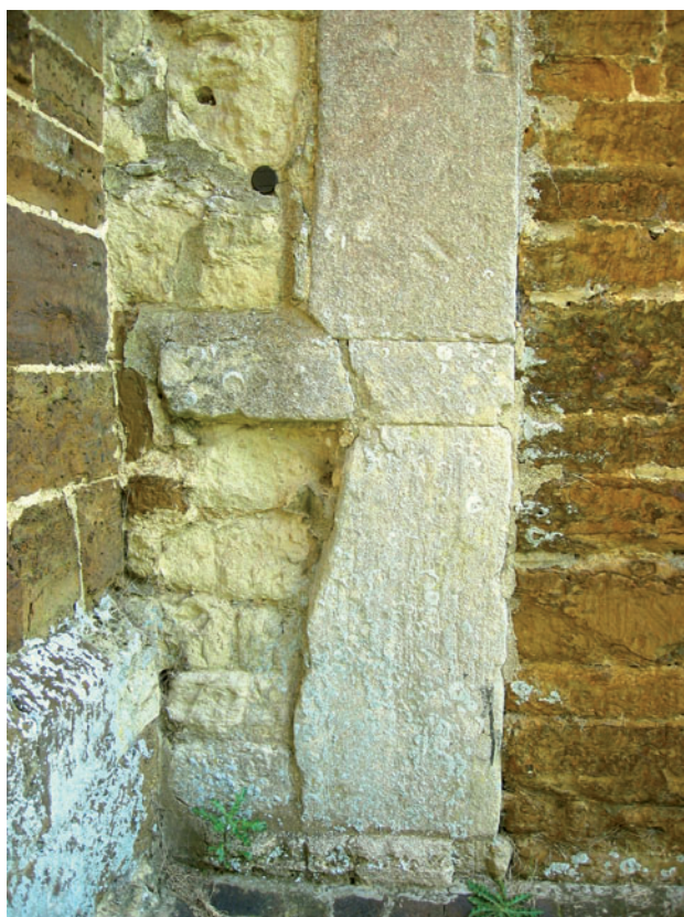
Fig 11 Three types of stone are visible in this view of the foot of the south-west nave quoin of Green's Norton church. The darker (brown) stone in the tower (left) and aisle (right) is from the Northampton Sand Formation; Anglo-Saxon stonework is represented by white limestone rubble in the nave wall, probably of local Blisworth Limestone, and its dressings in the Barnack-like Stone of the quoin, set BVFR, BH, BVFL
