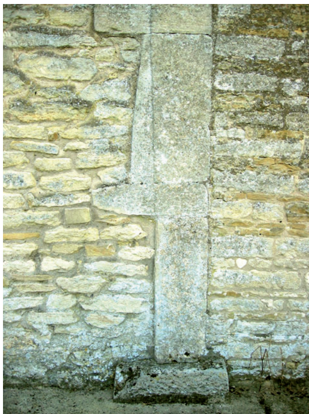
Fig 9 The stones in the north-east chancel quoin at Wittering church are set in Anglo-Saxon style; above the pedestal, stones 3, 4 and 5 have been cut back and stone 4 (BVFL) might be described as 'pear-shaped', and the quoin does not sit squarely on the plinth
