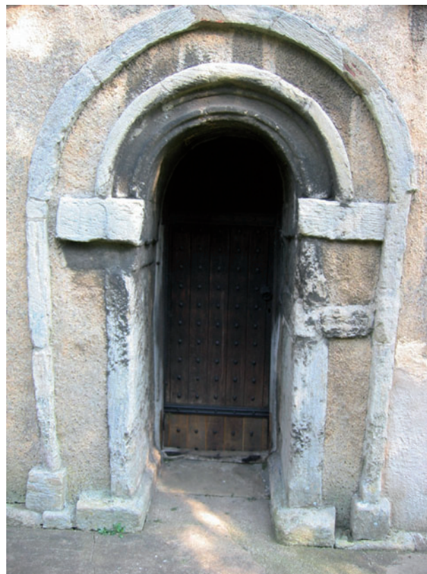
Fig 14 The stone orientations in the west doorway of Earls Barton tower support its Anglo-Saxon origin
