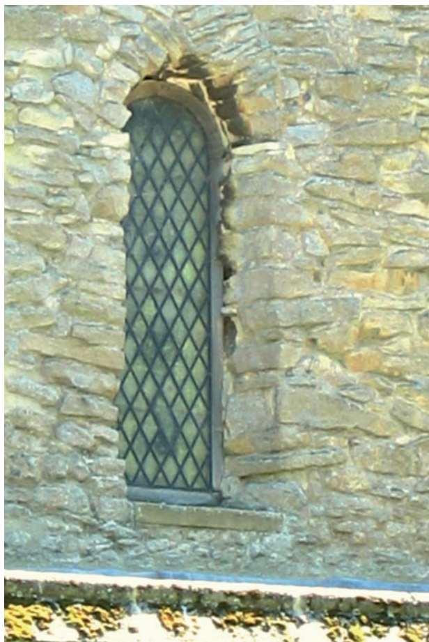
Fig 16 From the external view, the double-splayed window on the northern wall of the tower at Brigstock church shows evidence of having been replaced; note that the jamb stones (all BH), fit irregularly into the wall and that the sill stone is new
