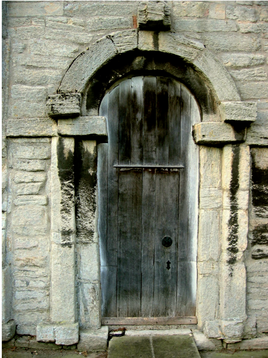
Fig 6 The south doorway of Barnack church has its vertically orientated stones set in Anglo-Saxon style (BVFIA and BH)
