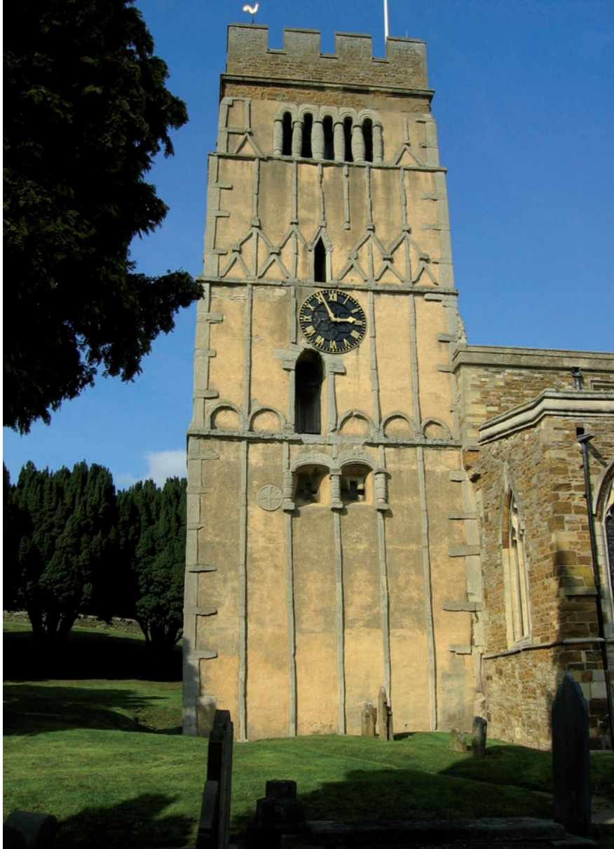
Fig 13 The south face of the Earls Barton, tower; note that the quoin stones are of variable width
