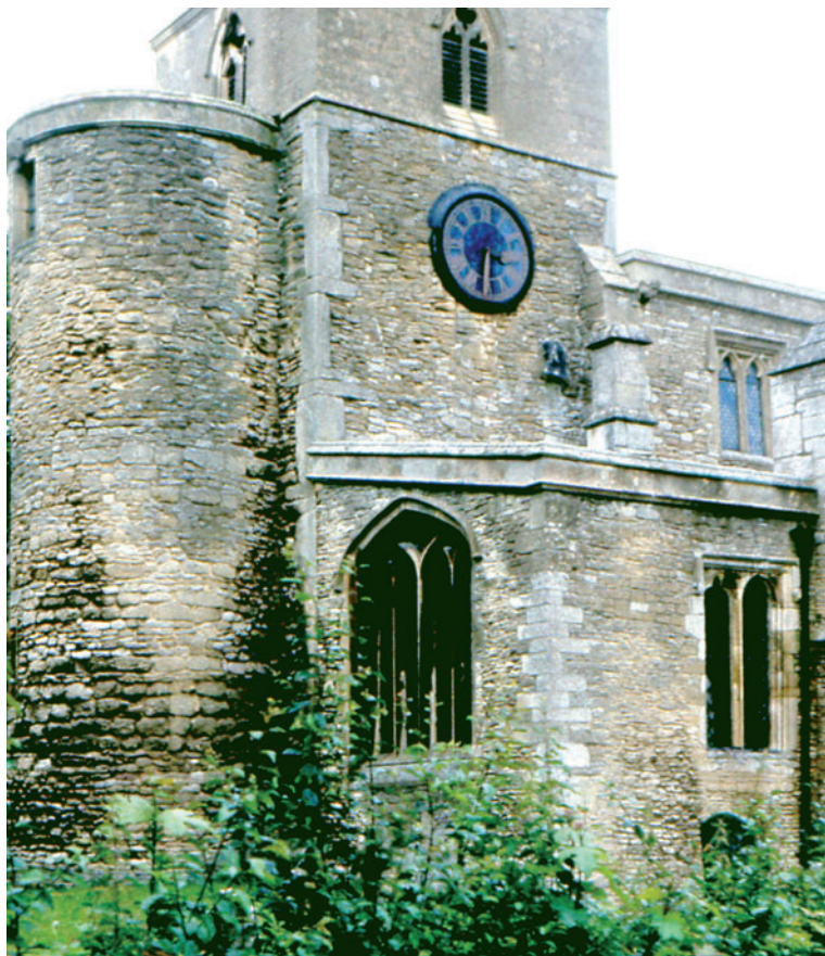
Fig 15 View of the Anglo-Saxon tower at Brigstock church, abutted by the circular stair turret, left, and a later aisle, right, (Photograph, A Chapman)
