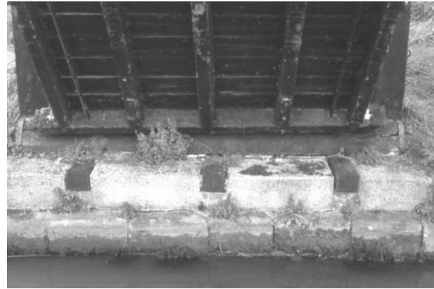
Fig 6 Detail of bank structure below the raised footbridge, looking west
