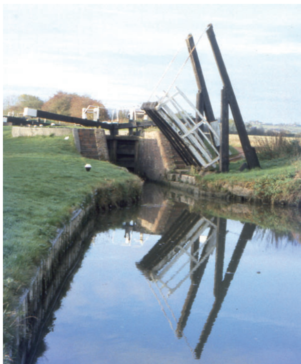
Fig 1 Rothersthorpe Lift Bridge GN5 in the up position, and lock number 5, looking south-west
