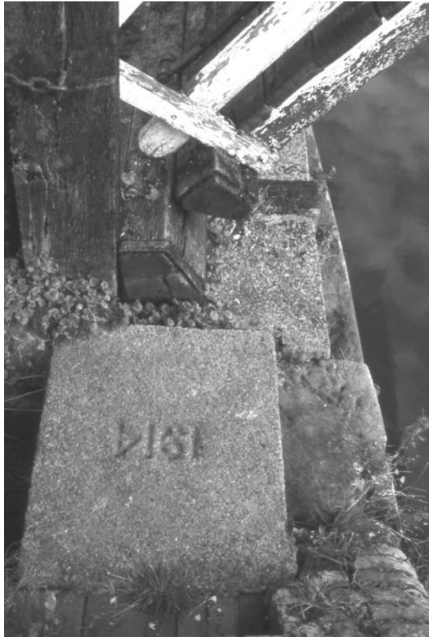
Fig 5 The date stone (1914) of the rebuild of bank surrounds, looking west
