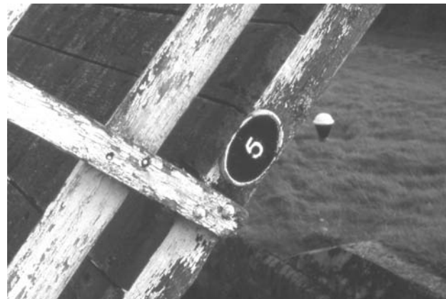
Fig 8 Detail of the footbridge assembly and cast number plate
