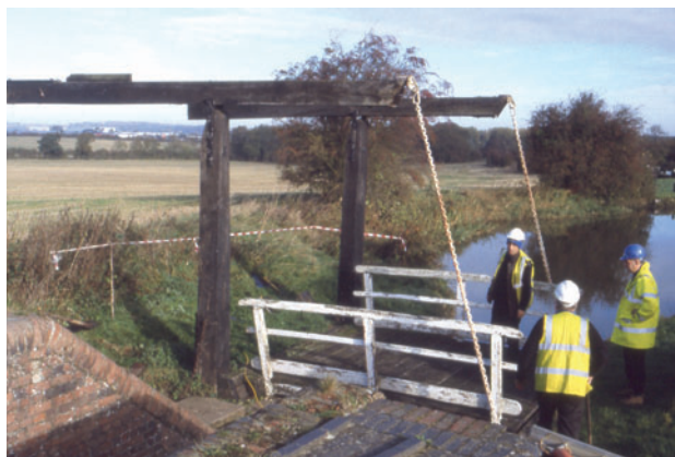
Fig 7 Lift Bridge GN5 in the lowered position, during dismantling, looking north-east
