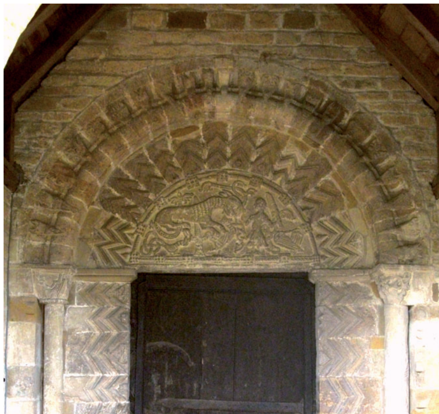
Fig 2 Pitsford, showing the tympanum over the south door
