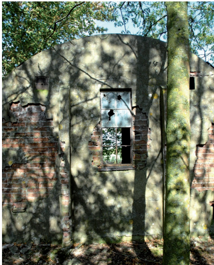
Fig 20 Hut 145, showing the steel-framed window
