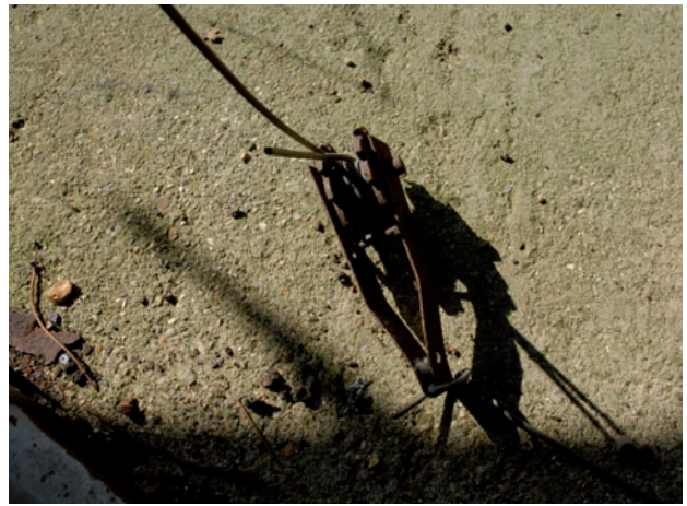
Fig 17 Straining ratchet on Hut 143
