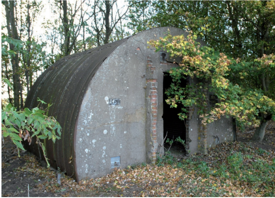
Fig 19 Hut 145, showing front wall and doorway, looking north-east
