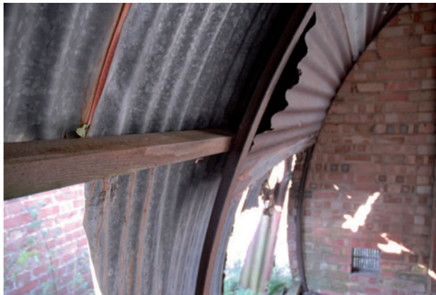
Fig 15 Wooden purlin in Hut 143
