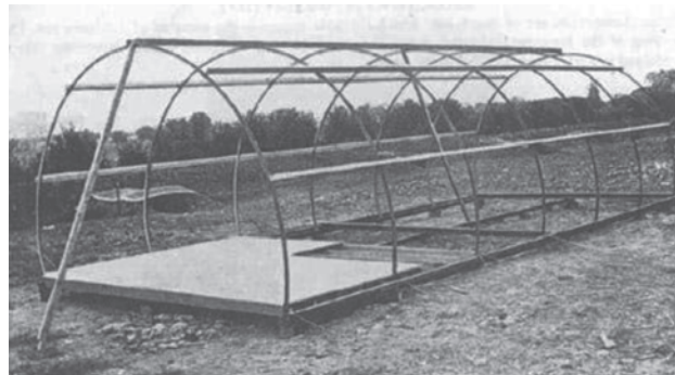
Fig 4 Wooden joists, screwed to the bearers, support wooden floor panels
