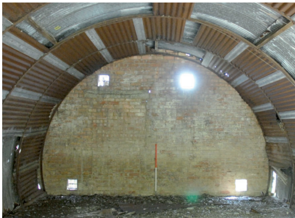
Fig 10 Interior of Hut 141, showing blocked door (left of the 1m ranging pole), looking south
