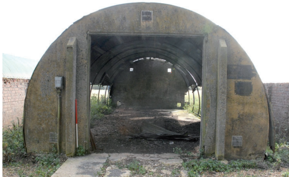
Fig 12 Front wall of Hut 143, looking south
