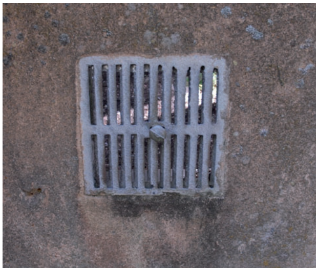
Fig 16 Detail of metal grille over wall vent
