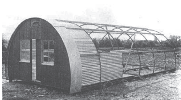
Fig 5 The hut is clad in corrugated iron
