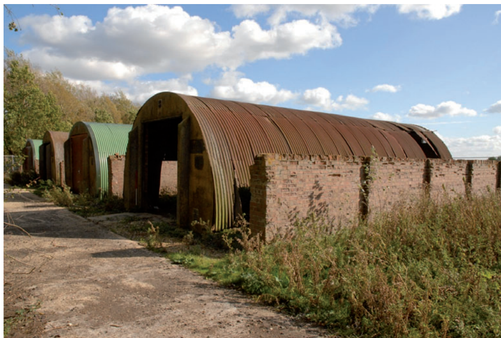
Fig 6 View of Nissen huts 141-144, looking east
