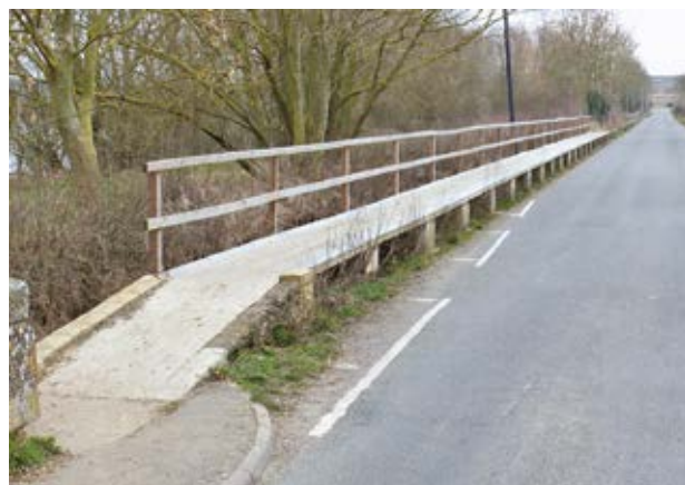
Fig 9 Ringstead, the northern end of the boardwalk, looking south-east
