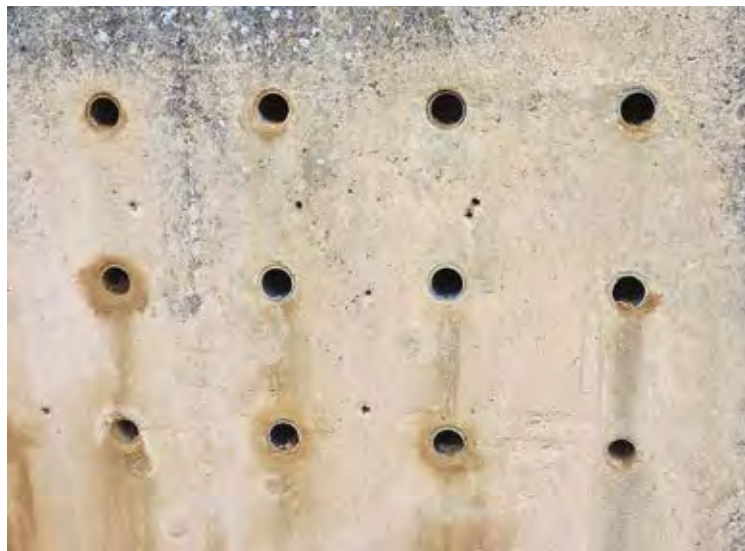
Fig 4 Detail of the newly drilled and lined nest holes
