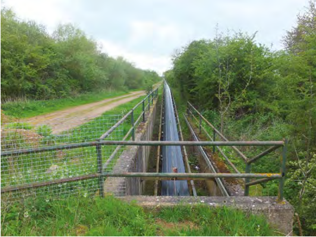
Fig 5 A quarry conveyor west of Hardwater Crossing (at SP 8804 6349), looking west
