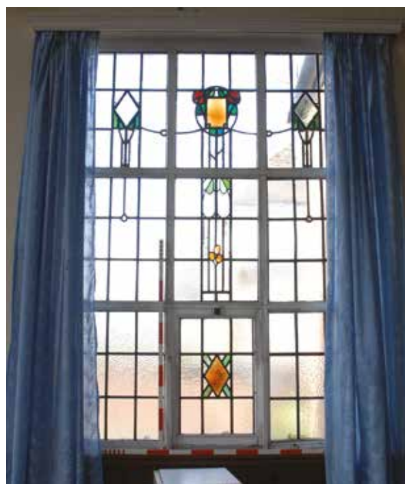
Fig 2: Side windows at Cogenhoe Baptist church
