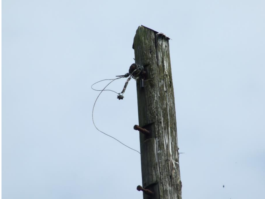
Figure 3 - Telephone/Telegraph Pole from Building A
