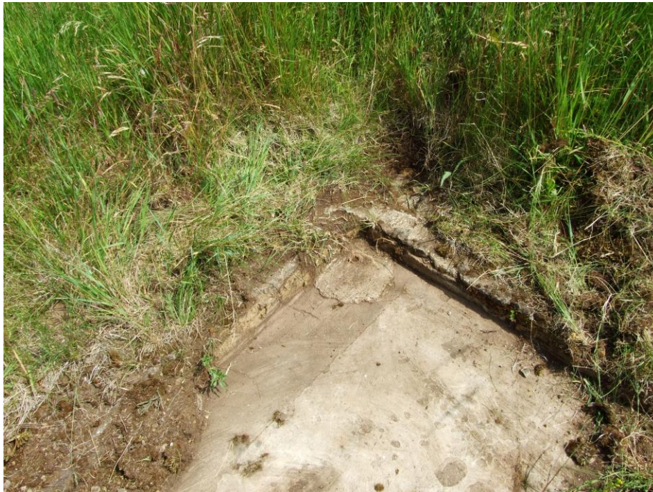
Figure 10 - Base of Building D.
