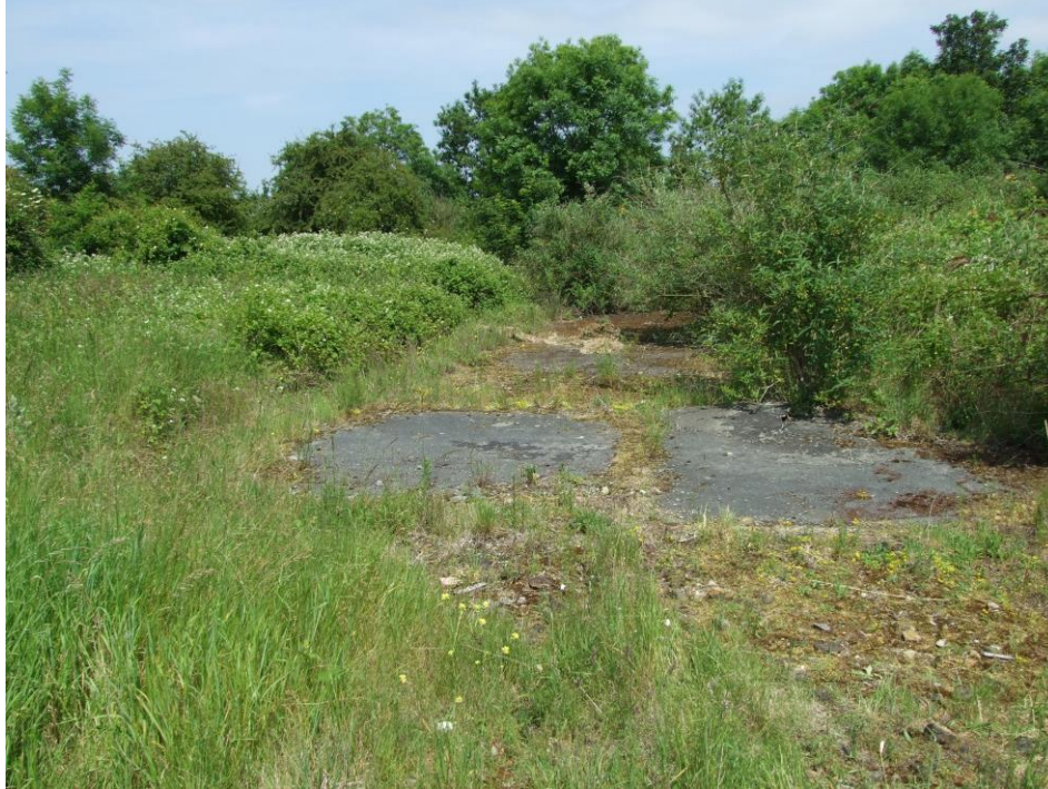
Figure 23 - Base of Building H (Boiler House). (looking north)
