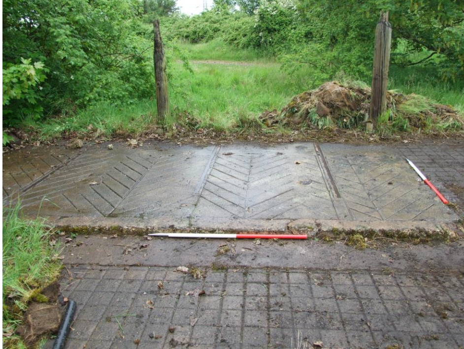
Figure 11 - Tram Car bays on southern side of entrance slope on western side of the shed. (looking west).
