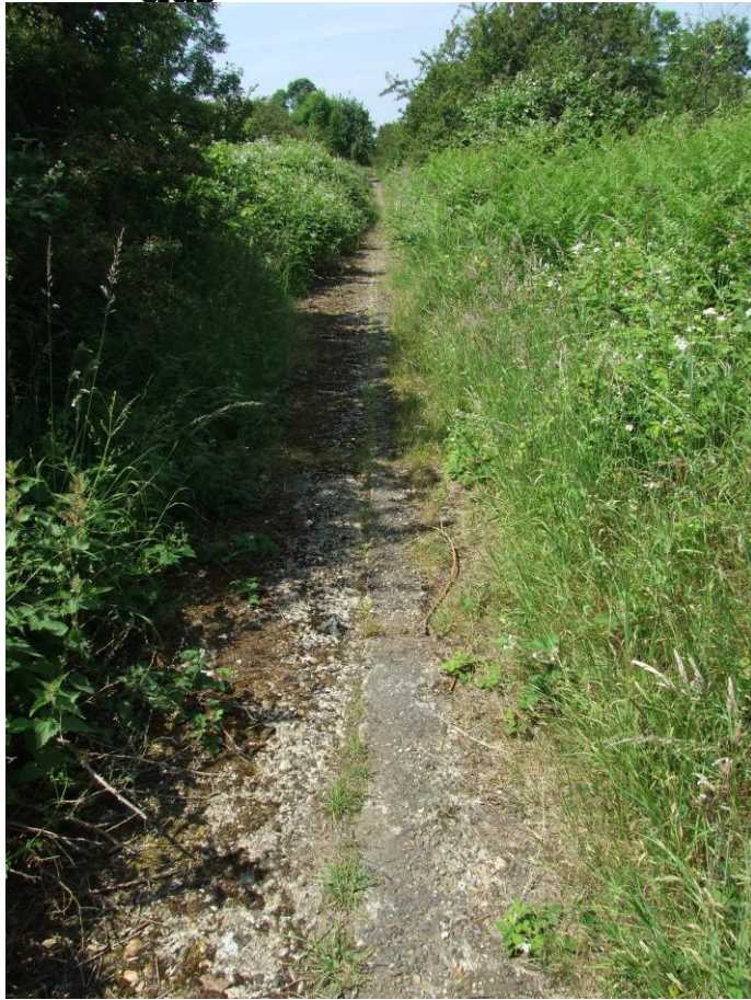
Figure 33 - Tramway running through centre of hospital site.
