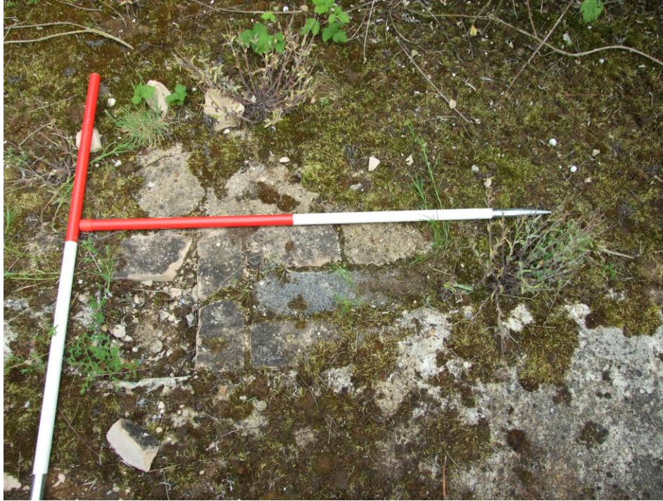
Figure 25 - Brick edge of drain from Boiler House (building H)
