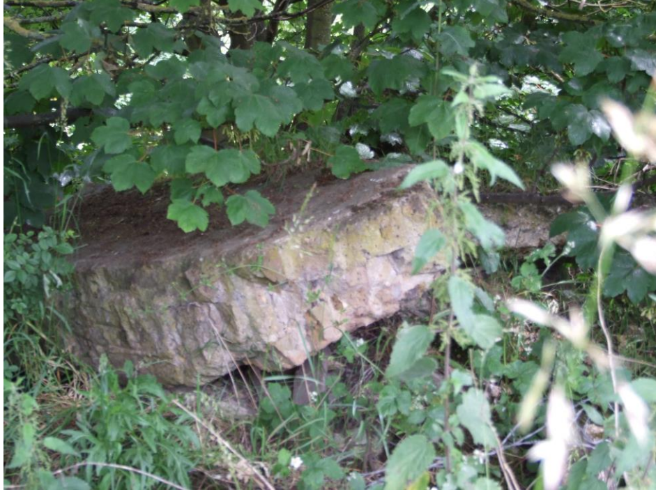
Figure 7 - Building rubble from next to Building C
