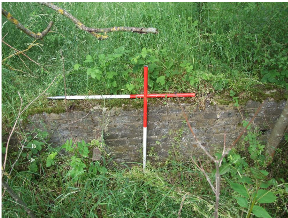
Figure 28 - North retaining wall for gully (Feature I)
