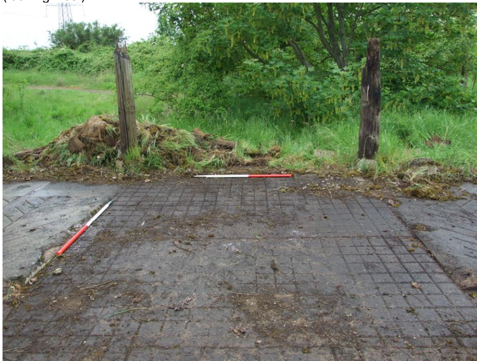
Figure 12 - Entrance slopeway on western side of the tram shed. (looking west).
