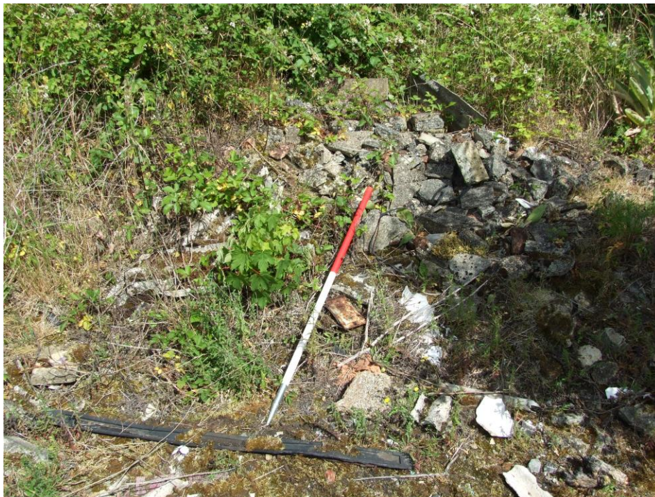
Figure 30 - Building rubble beside the turning circle at the western end of the hospital tramway.
