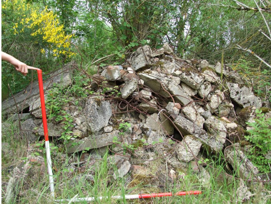
Figure 27 - Building rubble from Boiler House (building H)
