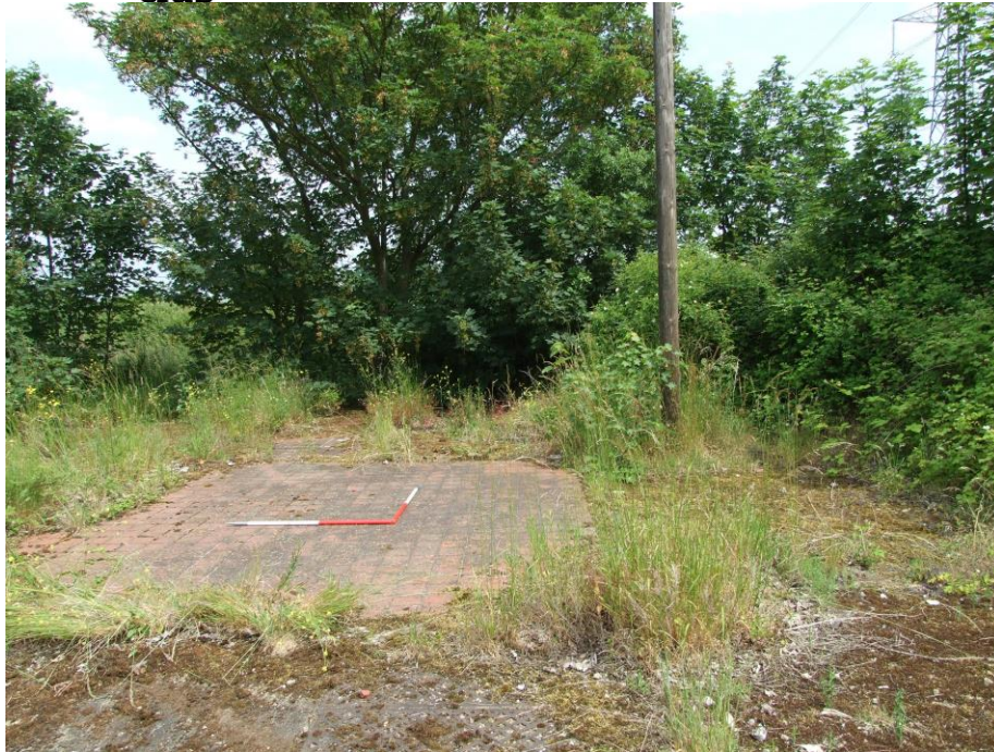
Figure 5 - Tiled floor of Building A (looking east).
