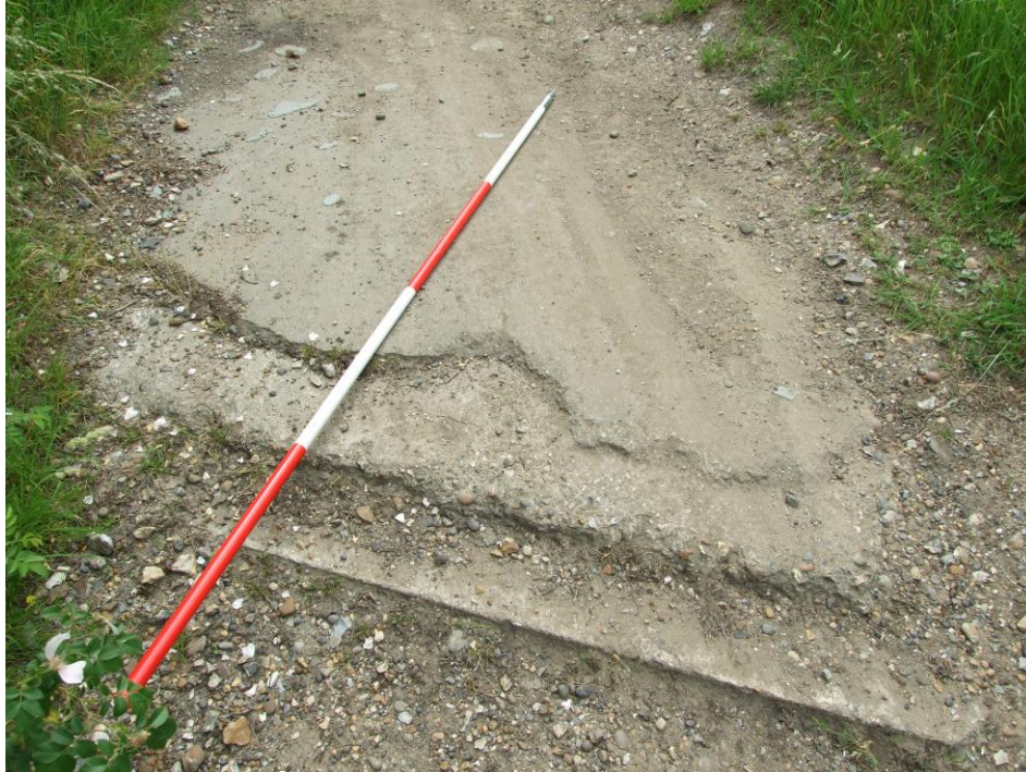
Figure 9 - Base of Building C.
