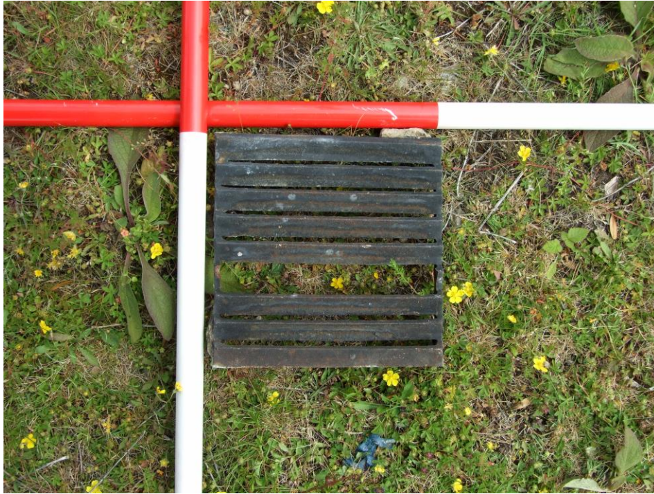
Figure 19 - Metal grill from the wall of Building G.
