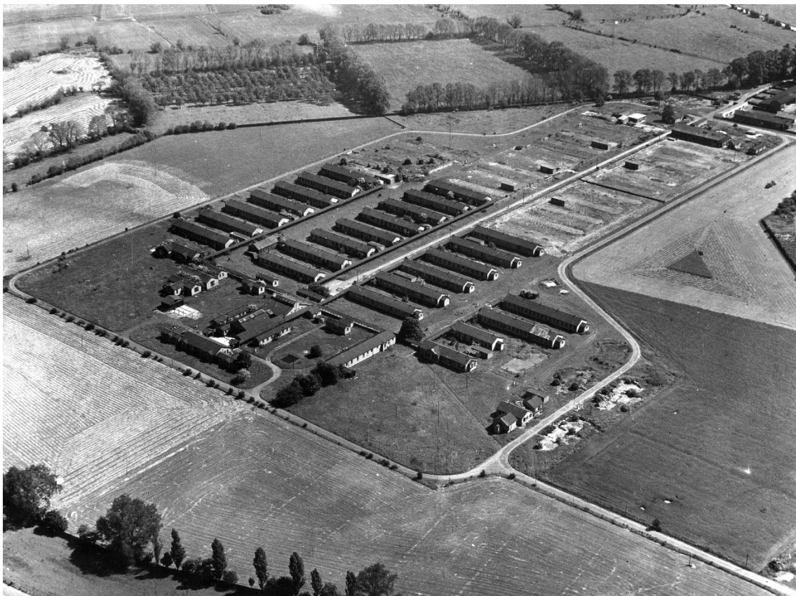
The Orchard post WW2, showing bomb damage.
