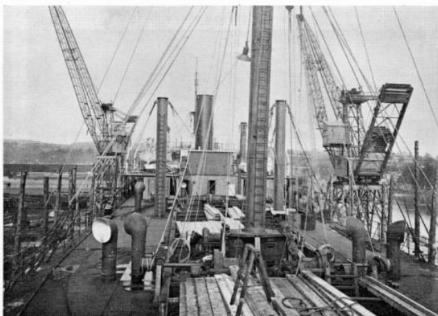
Deck view of 'N' type ship No. 2 berth, looking forward (Photo by courtesy of E. J. T. Wiles, Esq.)
