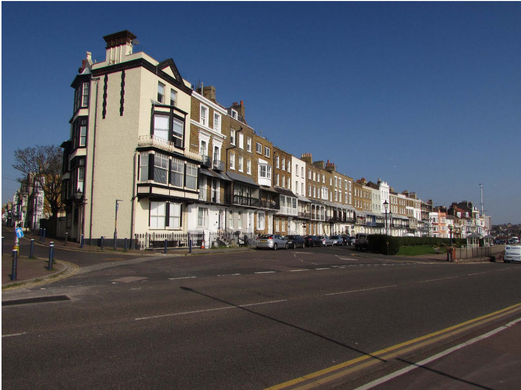
Photograph 5: Townhouses on Nelson Crescent
