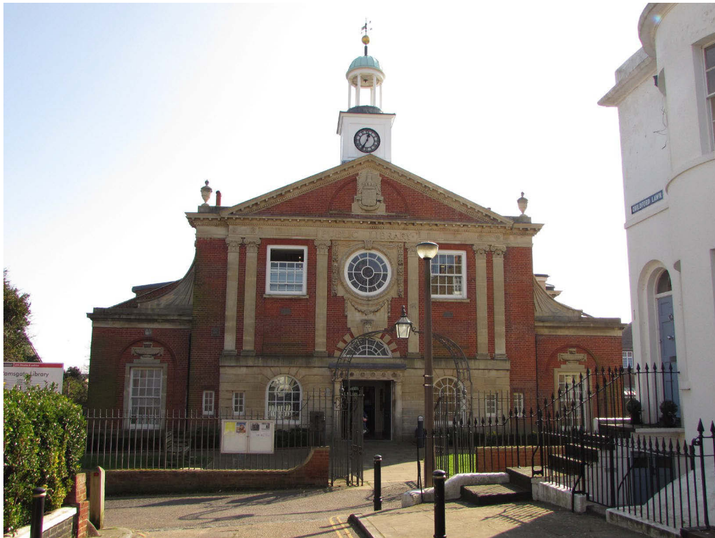
Photograph 10: Ramsgate Public Library (Listed Grade II)
