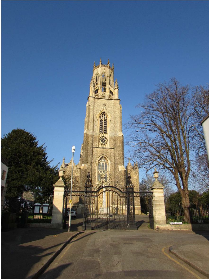
Photograph 7: Church of St. George, Ramsgate (Listed Grade I)
