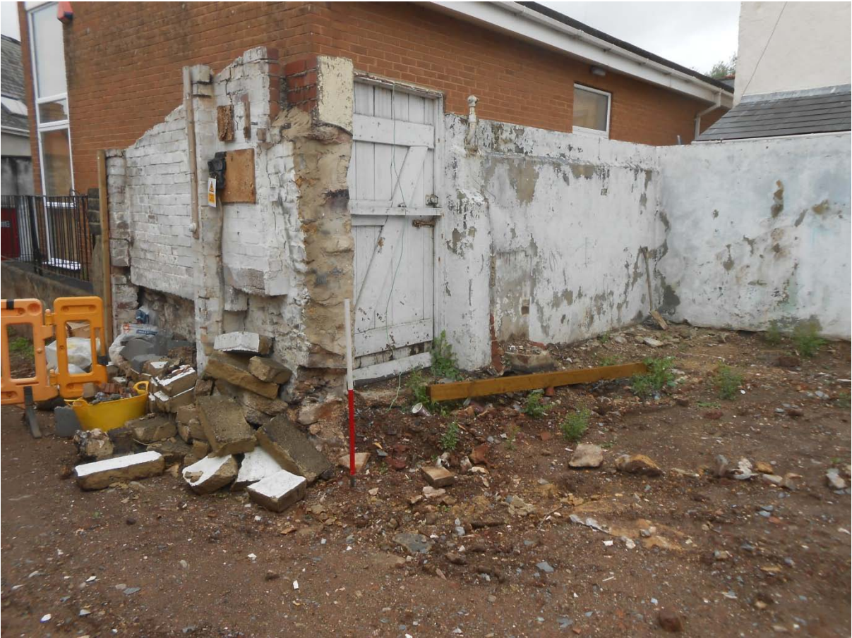
Fig. 7 View of the northern boundary wall before demolition.
