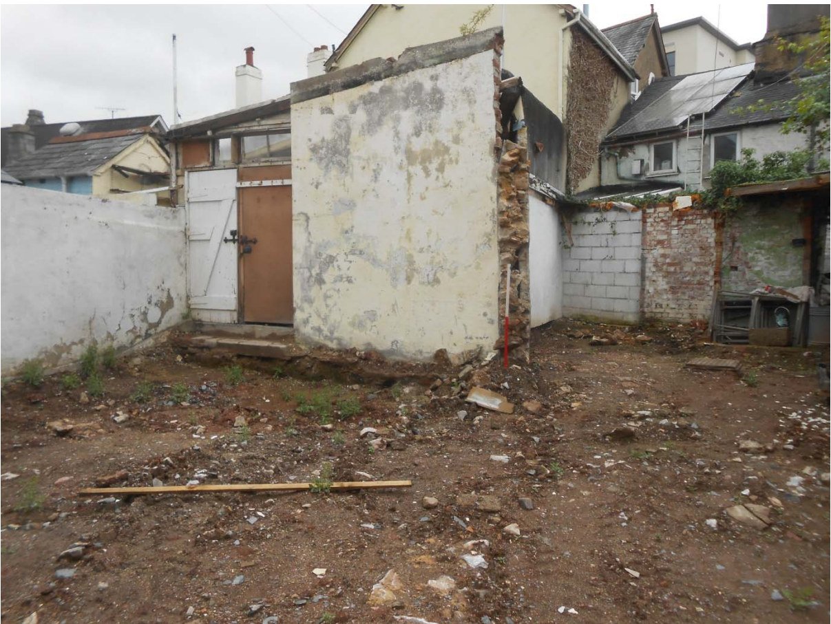
Fig. 8 view of the southern boundary wall before demolition.
