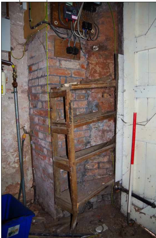
Plate 5: East elevation entrance showing breccia blocks with brick support pillars. View to northeast (scale 1m)
