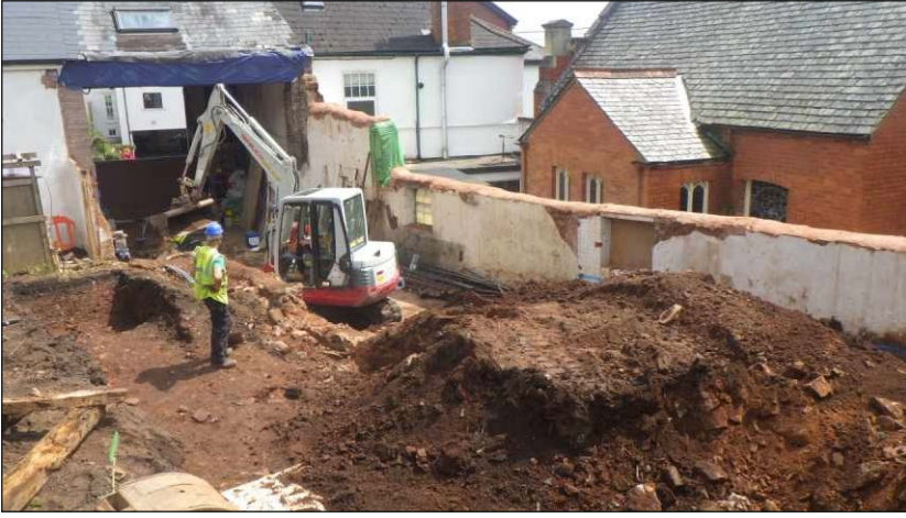
Plate 13: General working view during groundworks following demolition of workshop range. View to southeast
