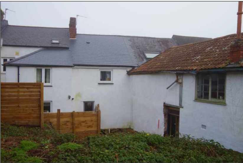
Plate 2: Showing rear of 8 Cockpit Hill with workshop range to the right. View to southeast (scale 1m)
