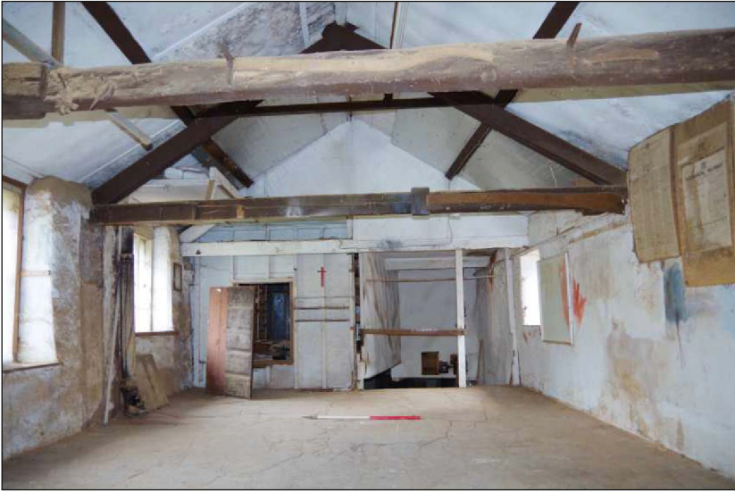
Plate 11: First floor workshop, view to northeast (scale 1m)
