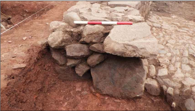
Plate 18. Showing section of wall S104. View to northwest (scale 0.4m)
