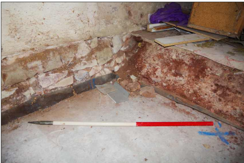
Plate 8: Showing reduced floor level and wall scar. View to south (scale 1m)
