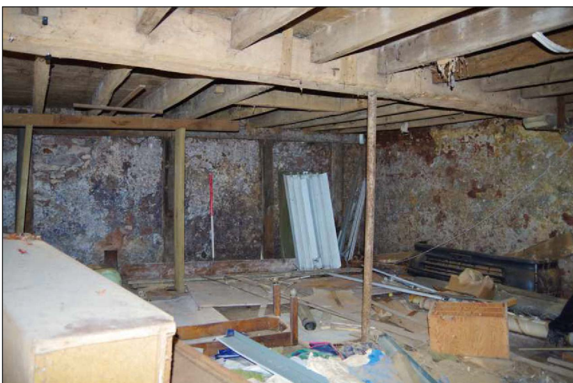
Plate 6: Ground floor store room, view to west (scale 1m)
