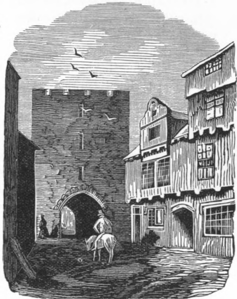
CLOSE GATE, EASTERN SIDE, REMOVED 1797.
