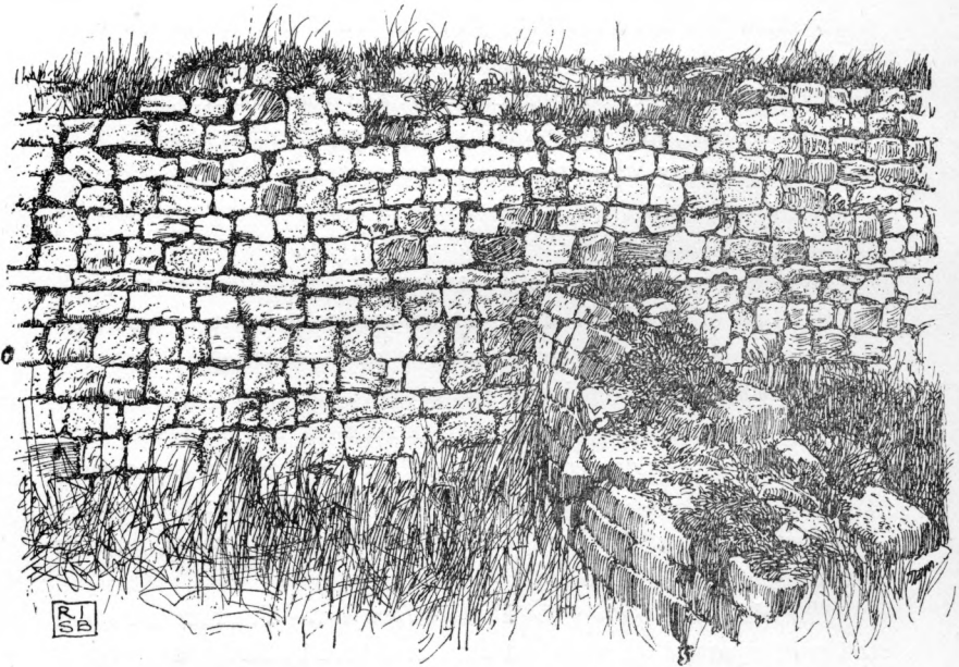
FIG. 21.—THE CAMP-WALL NORTH OF THE EAST GATE, SEEN FROM INSIDE.
