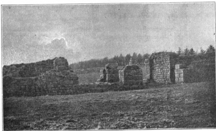
FIG. 2.—THE WEST GATE FROM THE INSIDE. (Excavated by Mr. John Clayton.)
