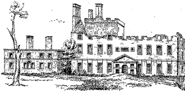
Fig 3. WEST SIDE, OLD BENWELL TOWER.
