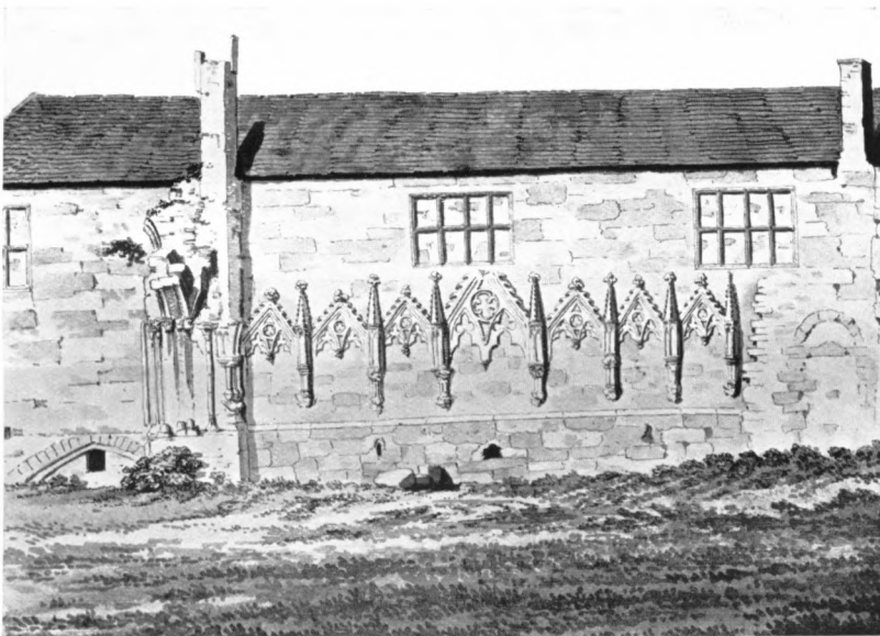
THE FRATER DOORWAY AND LAVATORY FROM THE CLOISTER.
