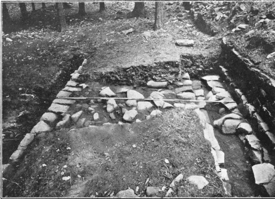
FIG. 3.—VIEW OF THE FOUNDATIONS OF THE EARLY RAMPART IN COCKMOUNT HILL WOOD, LOOKING EAST.
