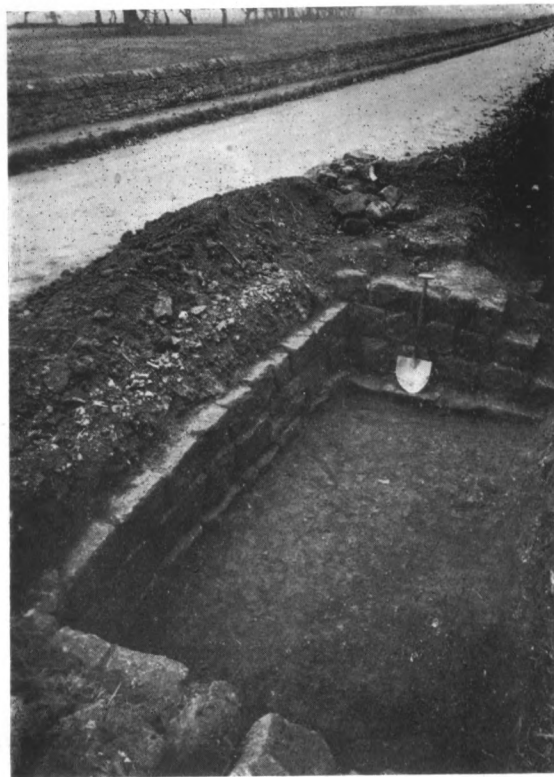
FIG. 2—INTERIOR OF TURRET NO. 12A, FROM THE WEST.
