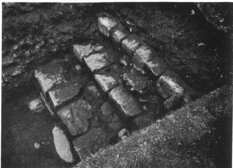
FIG. 1—SOUTH FACE OF THE WALL BETWEEN TURRET NO. 39B AND MILECASTLE NO. 40.
