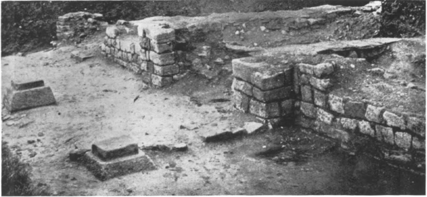
FIG. 1.—BUILDING V, SOUTH SHIELDS.
