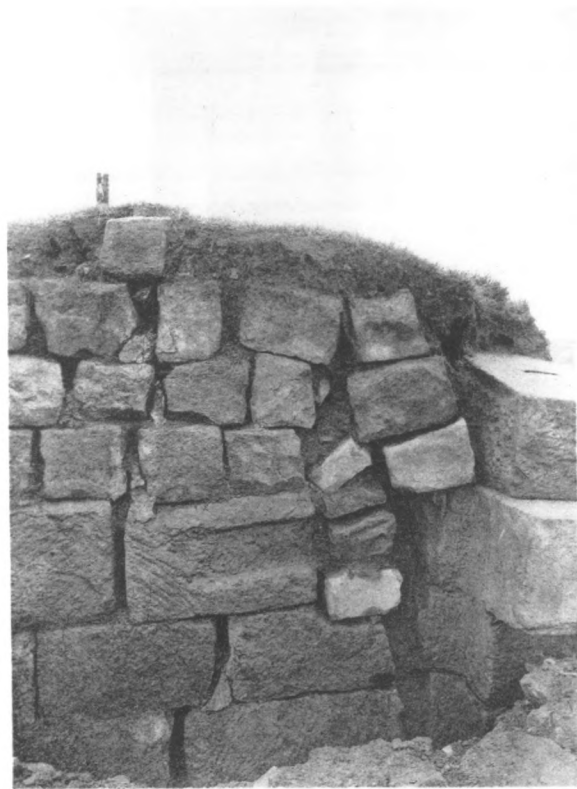
Fig. 2. N. GATE, SHOWING DISPLACEMENT OF N.W. PIER.
