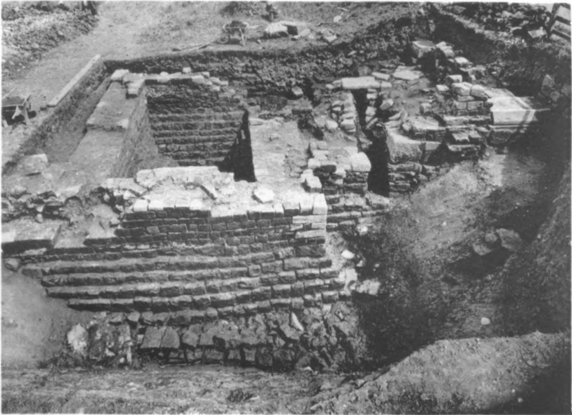
FIG. 1. HALTON CHESTERS: FOUNDATIONS OF MAIN WEST GATE. BUILT ACROSS THE DITCH OF THE GREAT WALL.
