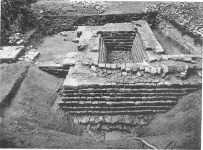
FIG. 2. HALTON CHESTERS: FOUNDATIONS OF MAIN EAST GATE. BUILT ACROSS THE DITCH OF THE GREAT WALL.
