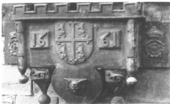
Fig. 2. LEAD HEAD ON EAST WALL OF BLACK STAIR.
