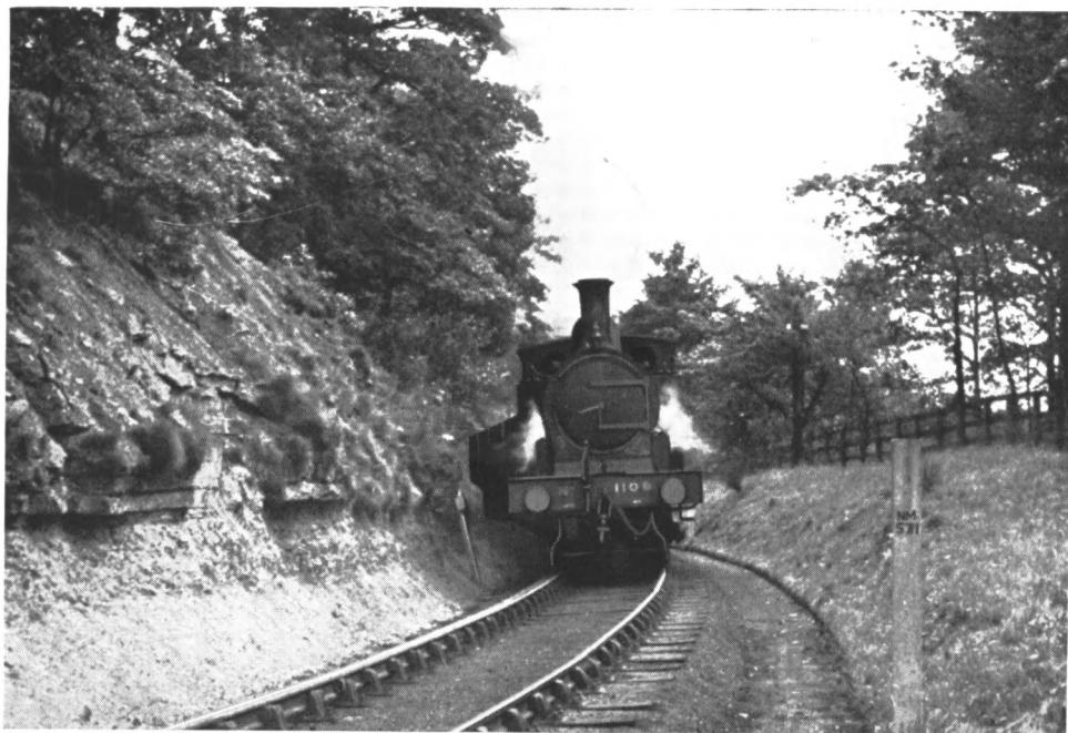
Mineral train, headed by ex-North Eastern Railway 0-6-2 tank engine, on the Tanfield Wagonway, now a branch of British Railways.
