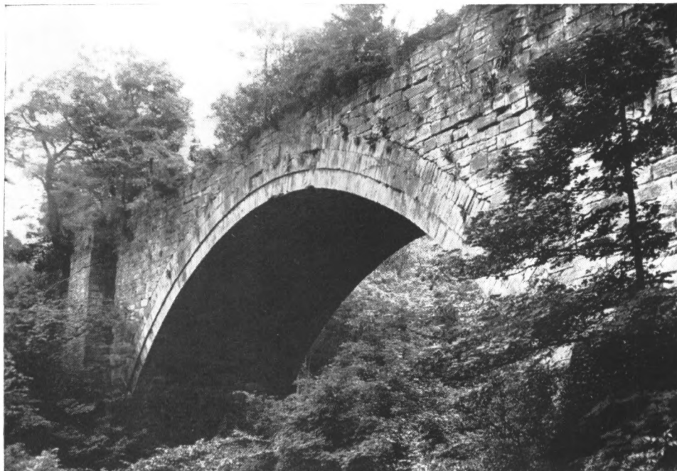
Modern view of the Causey arch, County Durham, which was built about 1727 to carry a double-track wagonway of 4-ft. gauge. It is probably the oldest surviving railway bridge in the world, and was scheduled in 1935 as an Ancient Monument of national importance.
