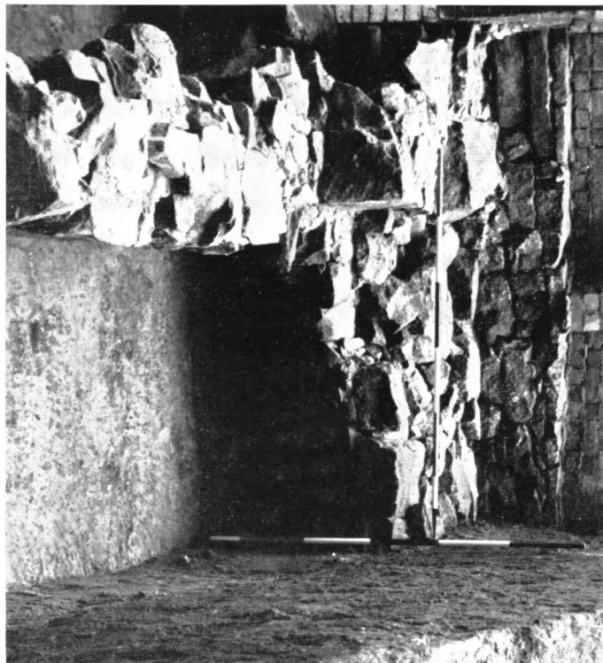
Fig. 1. Junction of tower wall and town wall
