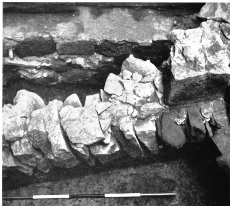
Fig. 2. Foundations of tower wall beneath one block of ashlar
